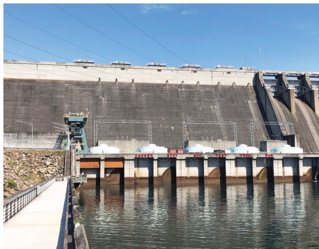
Hartwell Powerplant is the most upstream of three Federal hydroelectric stations on the Savannah River.
