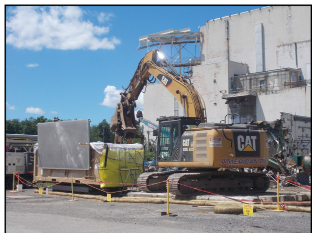
Waste loading with shielding for worker protection
