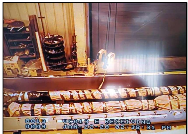
Vessel 4C-1 size-reduction and repackaging inside the Remote Handled Waste Facility (RHWF)
