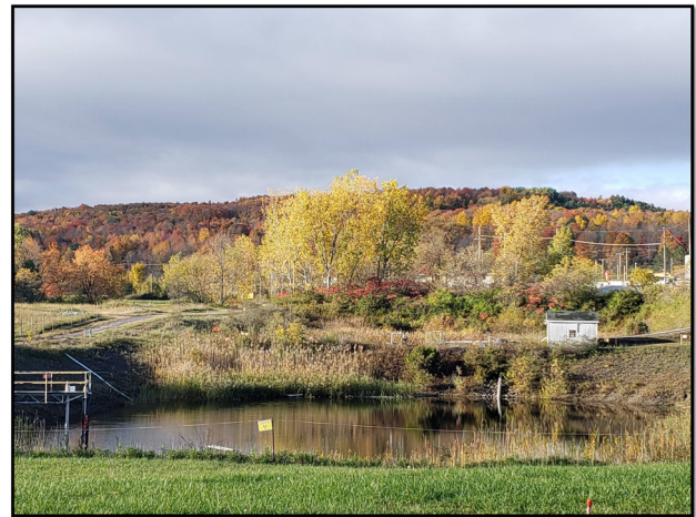
Controlled SPDES discharges occur from Lagoon 3
