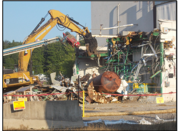
MPPB Utility Room (UR) demolition in progress
