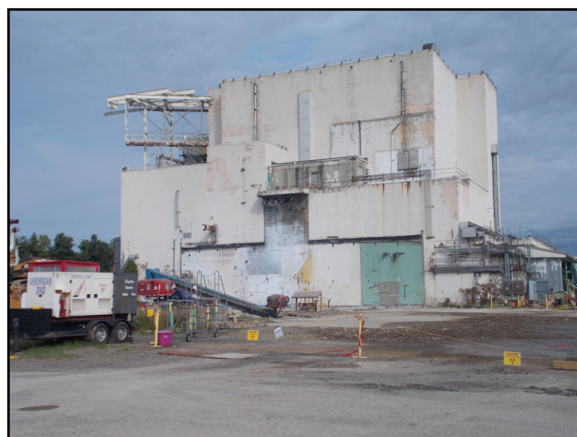
Utility Room (UR) after demolition
