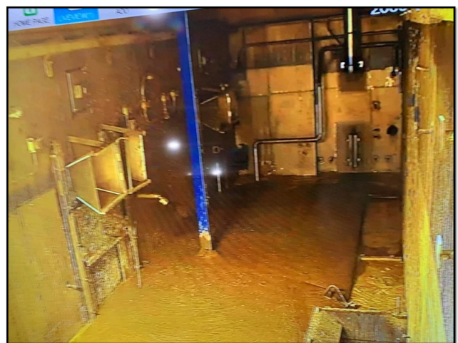
Grouting below ground portion of the General Purpose Cell (GPC)
