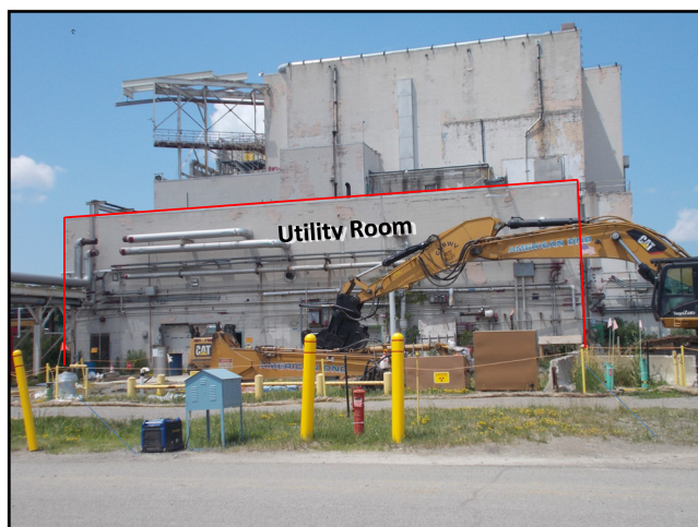
Utility Room (UR) before demolition
