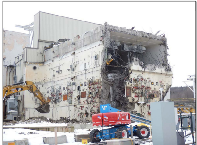
Early stages of demolition of the VF process cell
