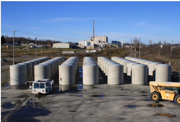
Canisters stored in Vertical Storage Casks (VSCs) relocated from within the MPPB
