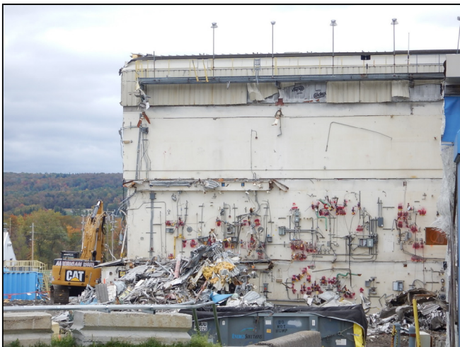
VF demolition of the outer access aisles
