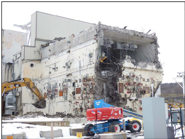
VF demolition in progress
