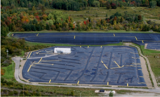
NRC-Licensed Disposal Area (NDA)
