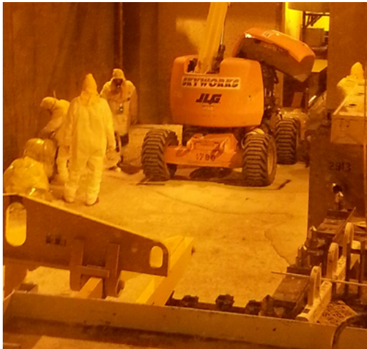
Debris removal in the Vitrification Facility (VF)
