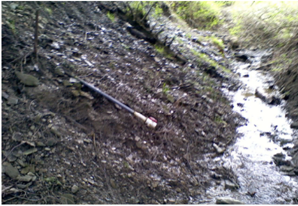
Seep monitoring discharge pipe
