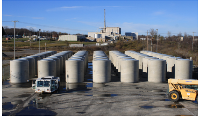
All 56 casks were relocated to the interim HLW Cask Storage Pad by November 2016
