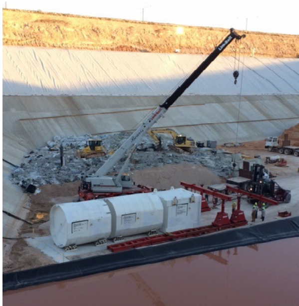
Burial of legacy LLW components at the permanent disposal site in Andrews, Texas
