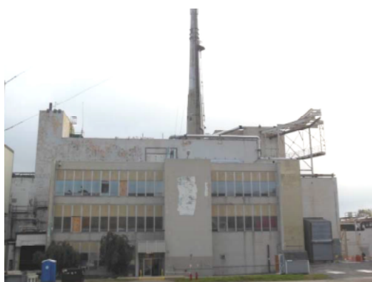
Main Plant Process Building (MPPB)
