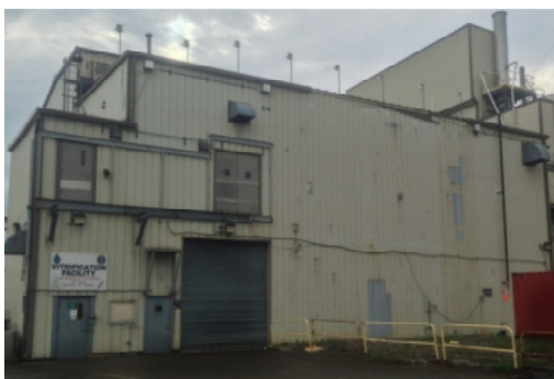
Vitrification Facility (VF)
