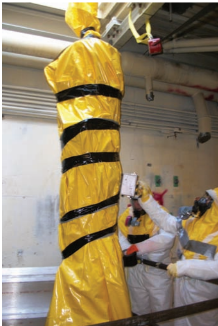
Removal of process vessels from the MPPB in preparation for demolition
