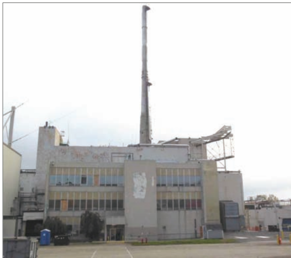
Main Plant Process Building
