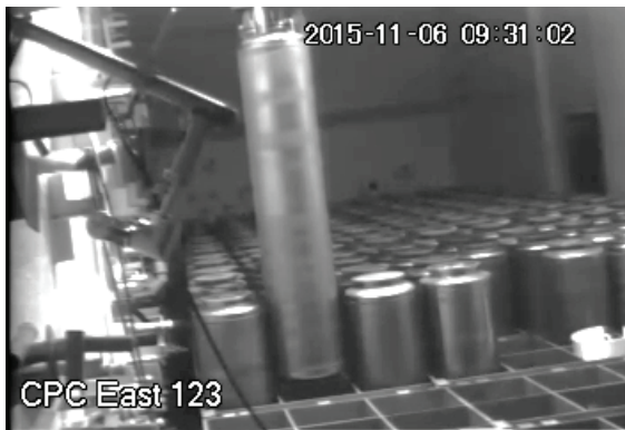
Removal of a HLW canister from the MPPB storage rack using remote-controlled equipment
