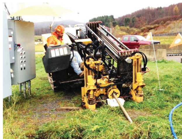
Installation of new drinking water line
