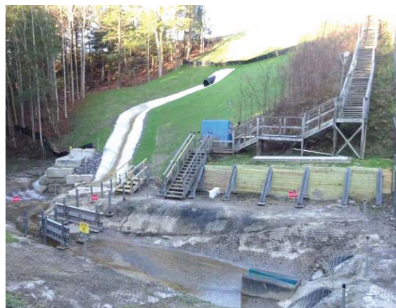
Rerouted S09 storm water outfall discharge
