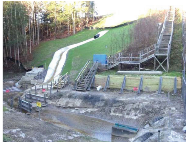
Rerouted S09 storm water outfall discharge
