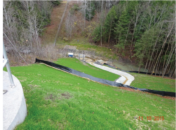
Rerouted S09 storm water outfall discharge
