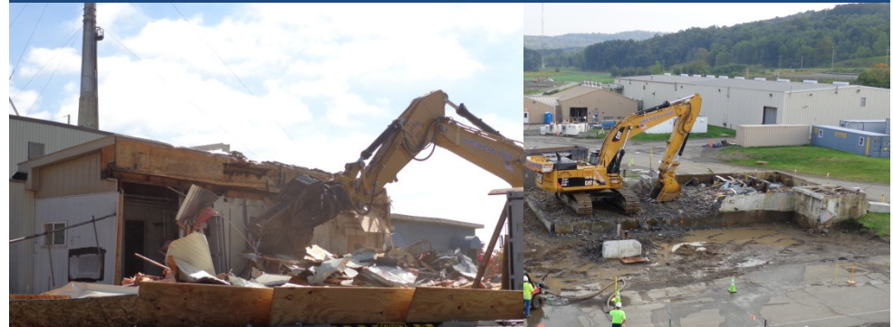
Vit Hill Trailer & New Cooling Tower Demo
