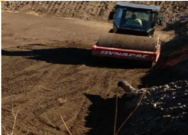
~ 300 deliveries (10,885 tons) of fill placed
