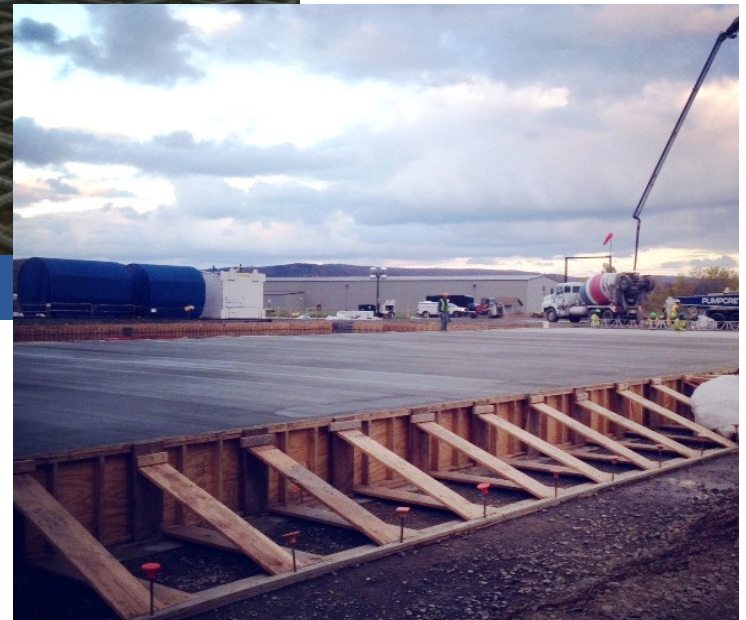
~1,800 cu-yds of concrete
