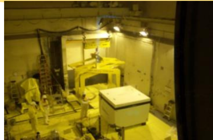
EDR Operations Supporting the Removal of HEC Drums from CPC Removal
