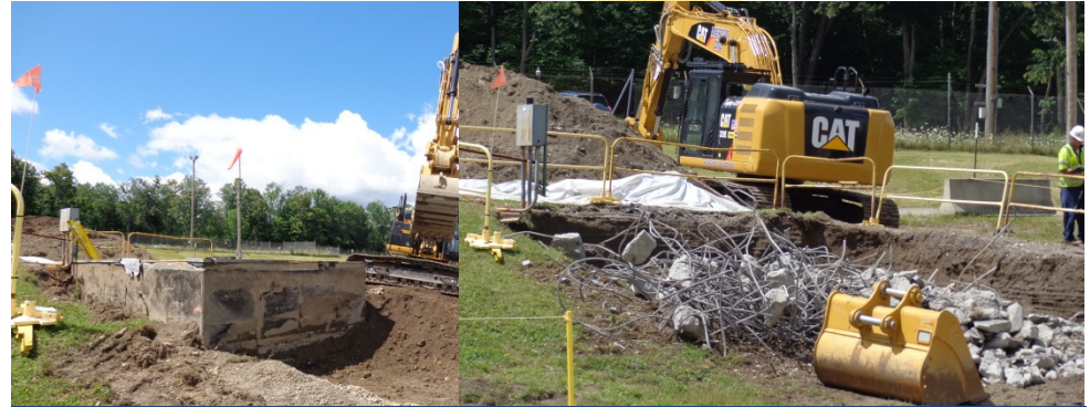
Vit Diesel Fuel Oil Pad – Before & After Demo
