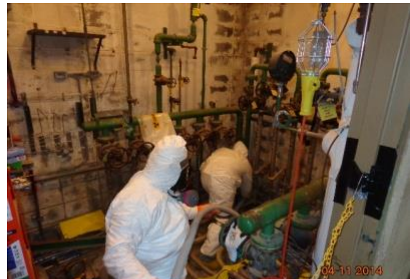
Con-Ed Building Lead Removal
