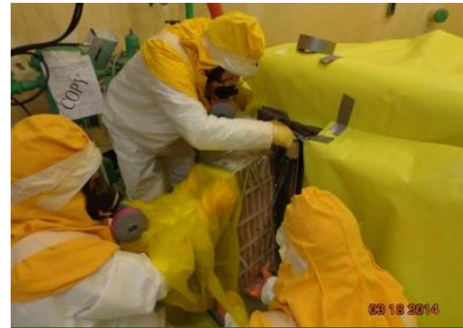
Roughing Filter Changeout
