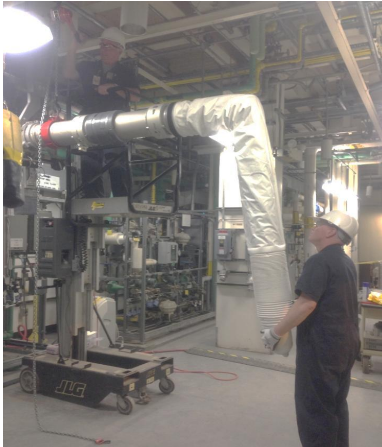
Master Slave Manipulator (MSM) Replacement
