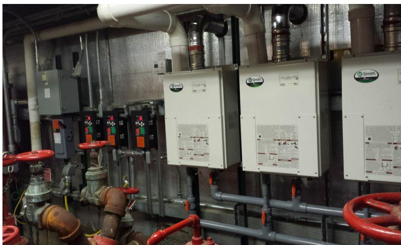
Installation of Heating System for Tank 32D-1 in Fire Pump House
