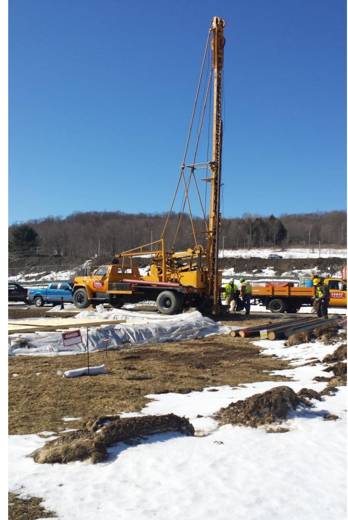
Drilling New Site Groundwater Well 1
