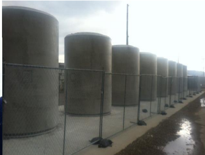
8 Add'l Vertical Storage Casks (VSCs) Being Constructed
