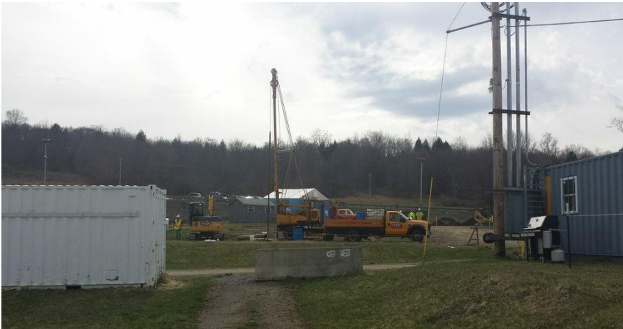
Drilling New Site Groundwater Well 2
