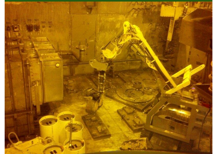
Main Floor after Vacuuming
