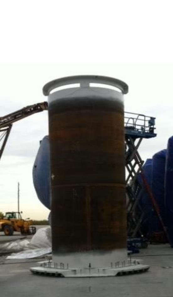
Cask Liners Being Fabricated
