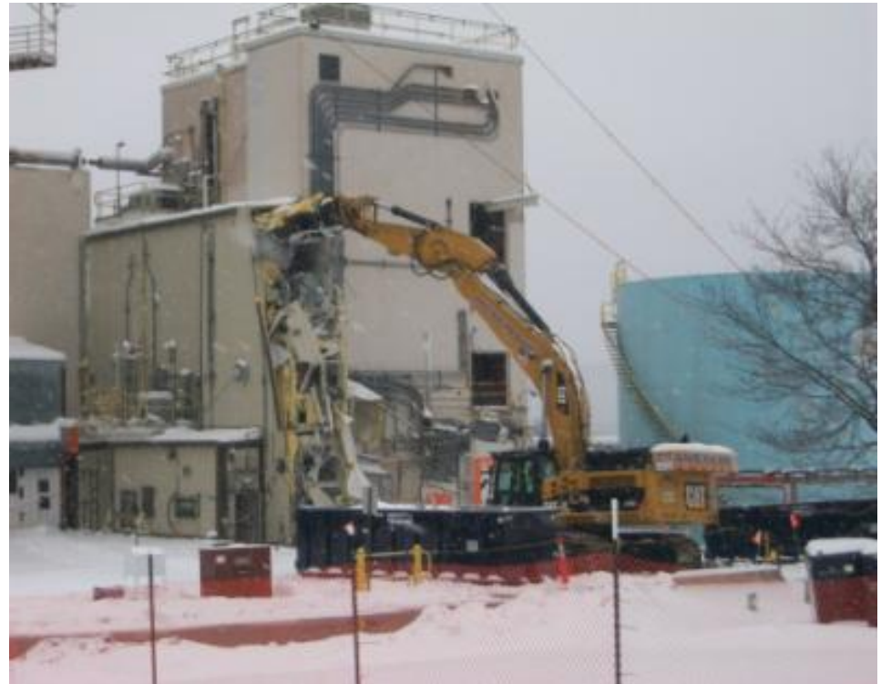
Demolition of North Side of 01-14 Building
