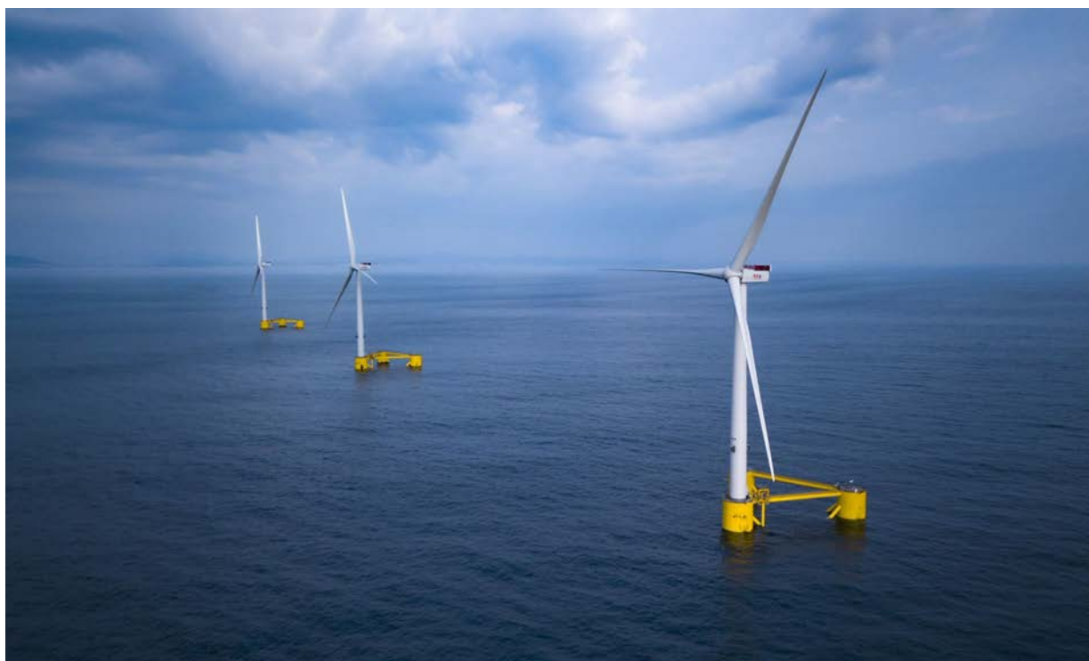
Figure 20. Kincardine 47.5-MW floating offshore wind plant. Photo courtesy of Principle Power, Inc.
