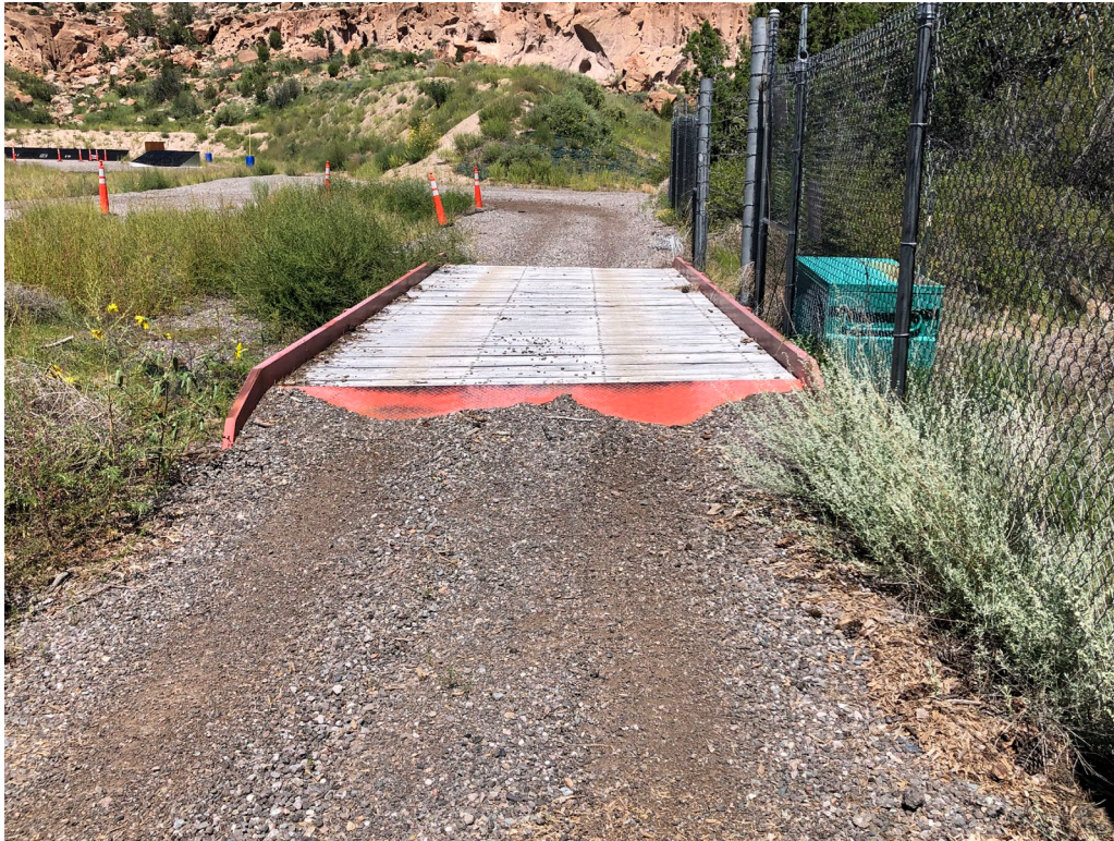
Figure 4. Proposed Location of Gate #3 East Perimeter Fence Looking North.
