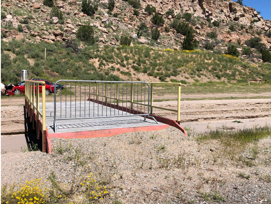
Figure 2. Proposed Location of Gate #1 Northwest of Building 72-0011 Looking North.
