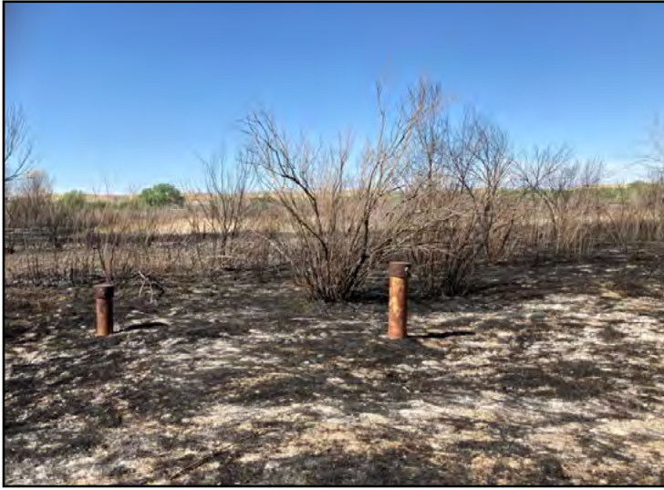
A wildfire engulfed some of LM’s monitoring wells last year at the Shiprock disposal site in New Mexico. After a fire is contained and the area is safe, teams assess infrastructure for potential damage from the heat.
