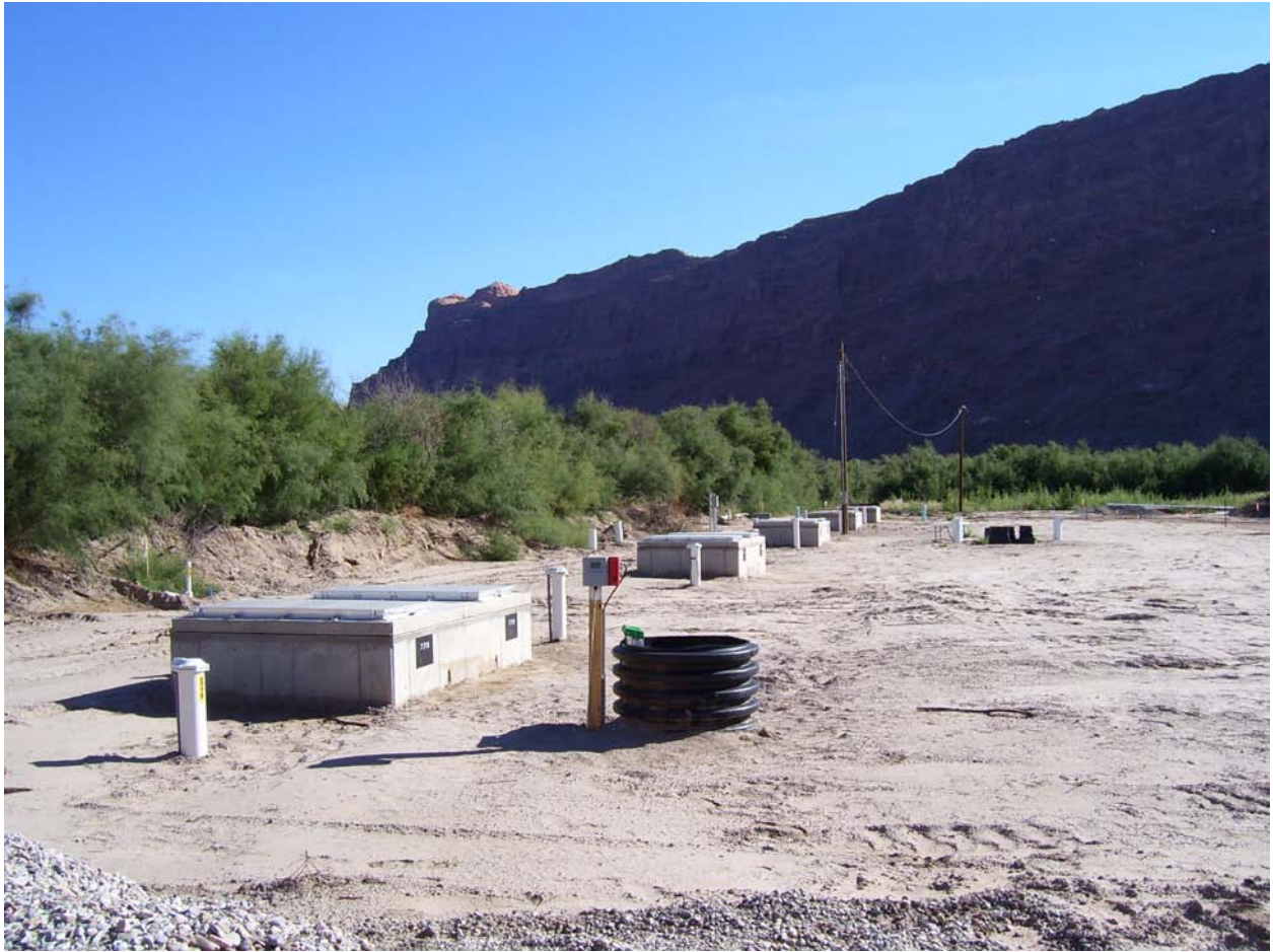
Interim Action Well Field Configuration 4 Wells
