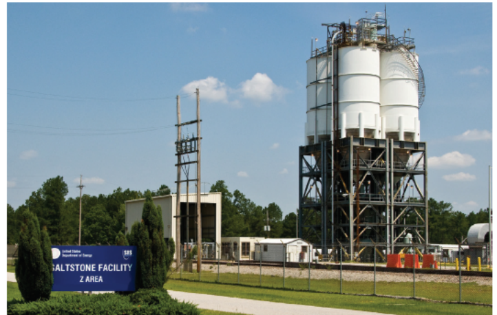
SPF contains the tanks and equipment necessary to process saltstone grout.
