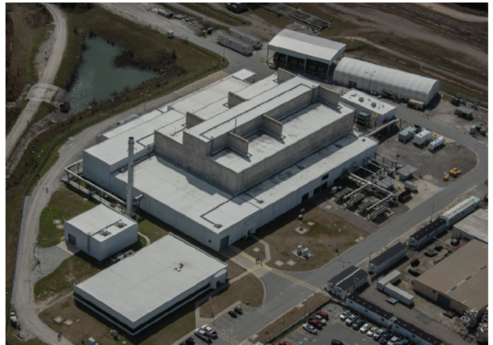
SWPF will process the majority of the Site’s salt solution waste.
