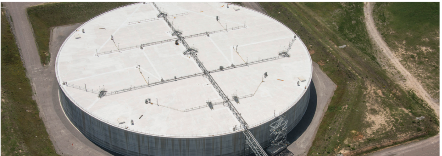
The mega-volume units are designed for the larger decontaminated salt solution stream that will be produced by the site's Salt Waste Processing Facility.
