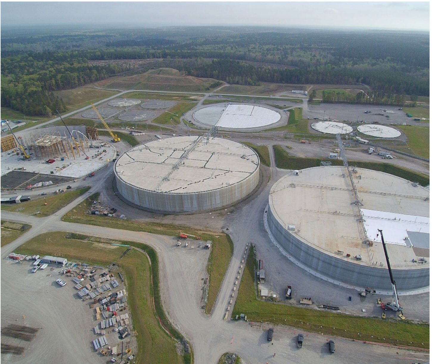
Saltstone Disposal Units are permanent disposal units at the Savannah River Site. The smaller SDUs can be seen in the top right and left portion of the photo, while the larger, mega-volume SDUs to the bottom and top middle.
