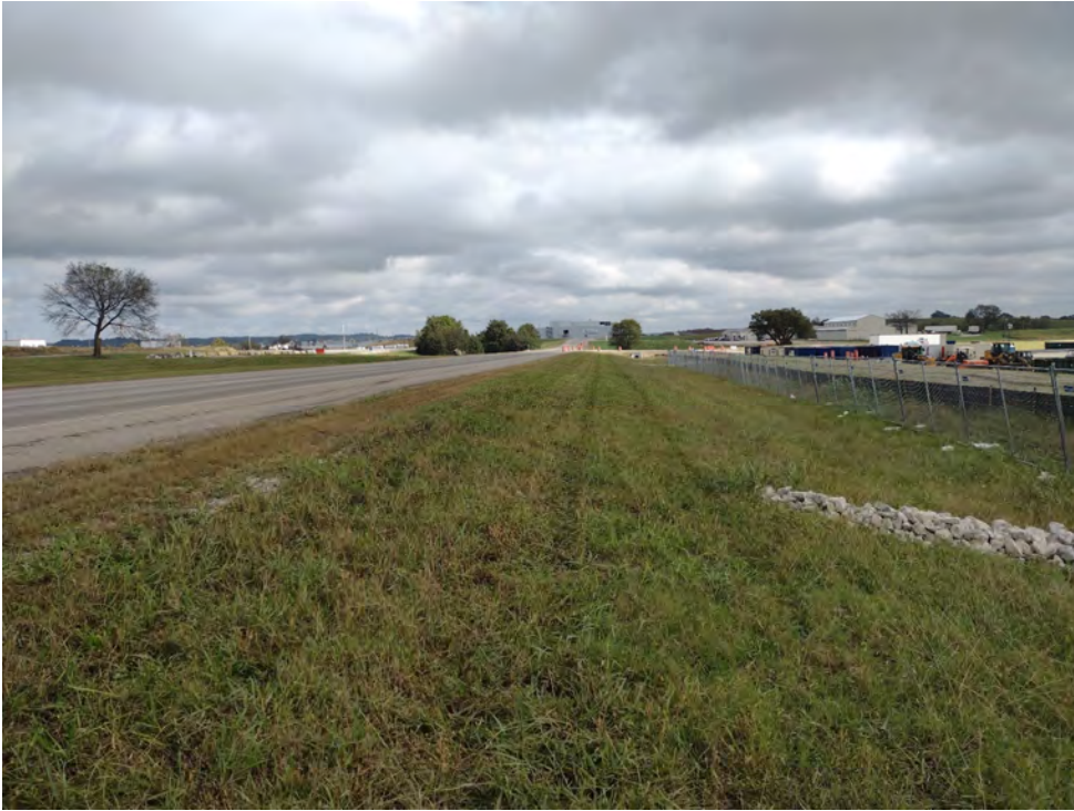
Photograph 1. Overview of Area 3 (southeast edge), facing northeast.
