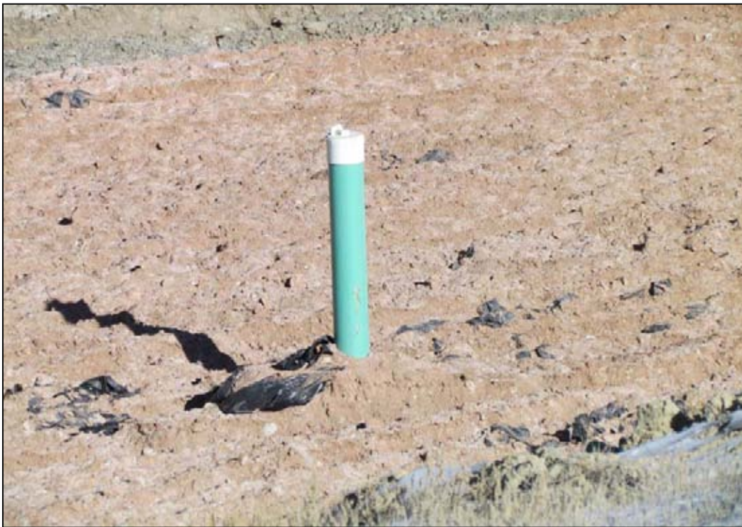
Photo 67. Standpipe with Placed RRM January 6, 2012
