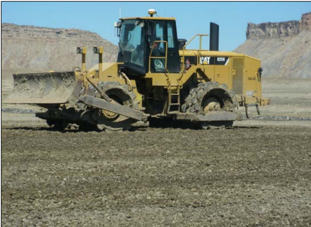
Photo 48. Frost Protection Layer Compaction June 21, 2011
