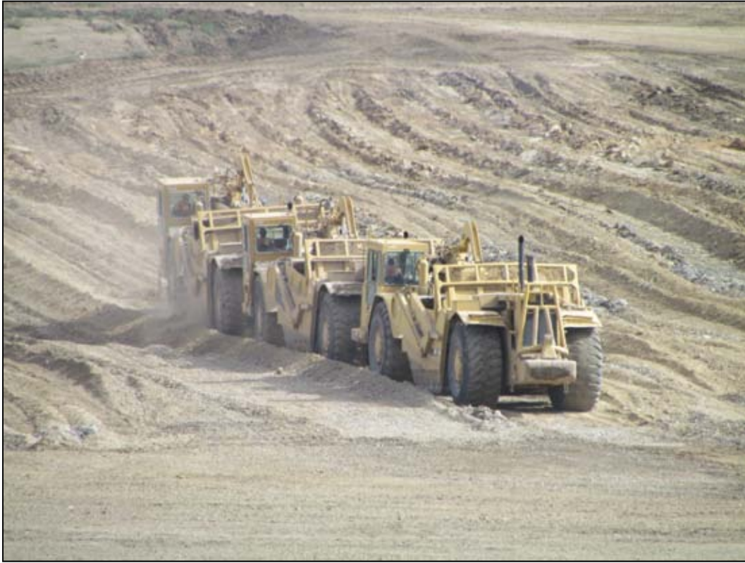
Photo 11. Cell Excavation July 19, 2011
