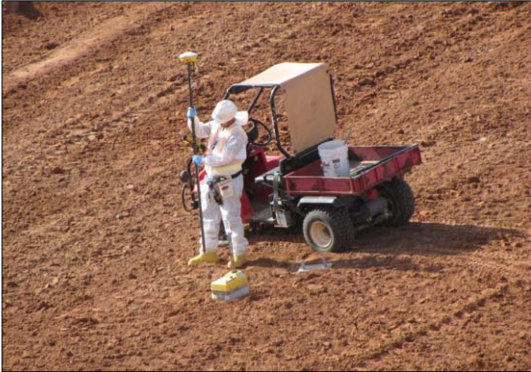
Photo 14. Density Test June 2, 2009
