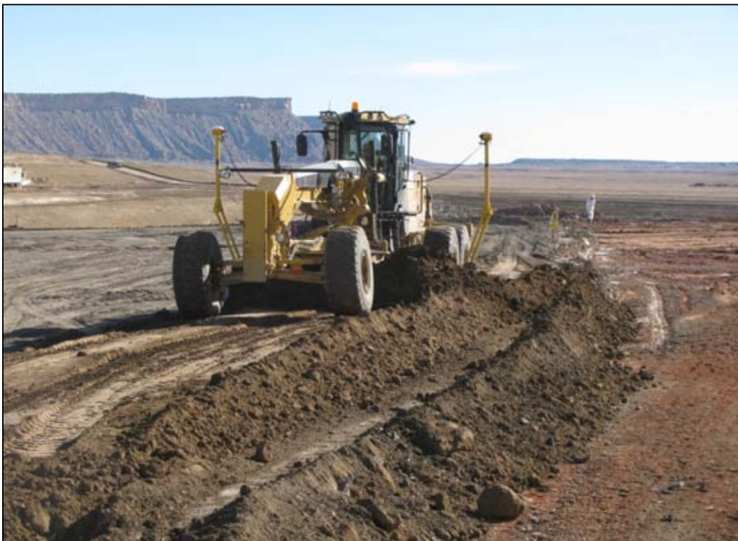
Photo 25. Interim Cover Placement March 1, 2011
