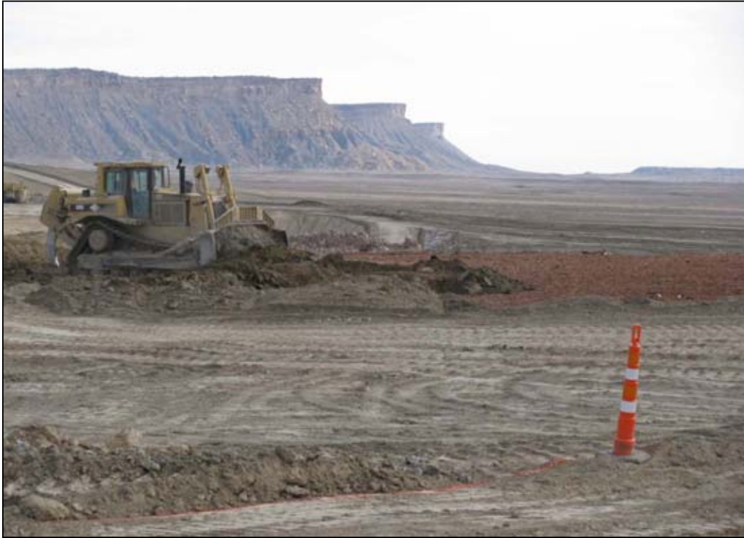
Photo 26. Interim Cover Placement March 7, 2011
