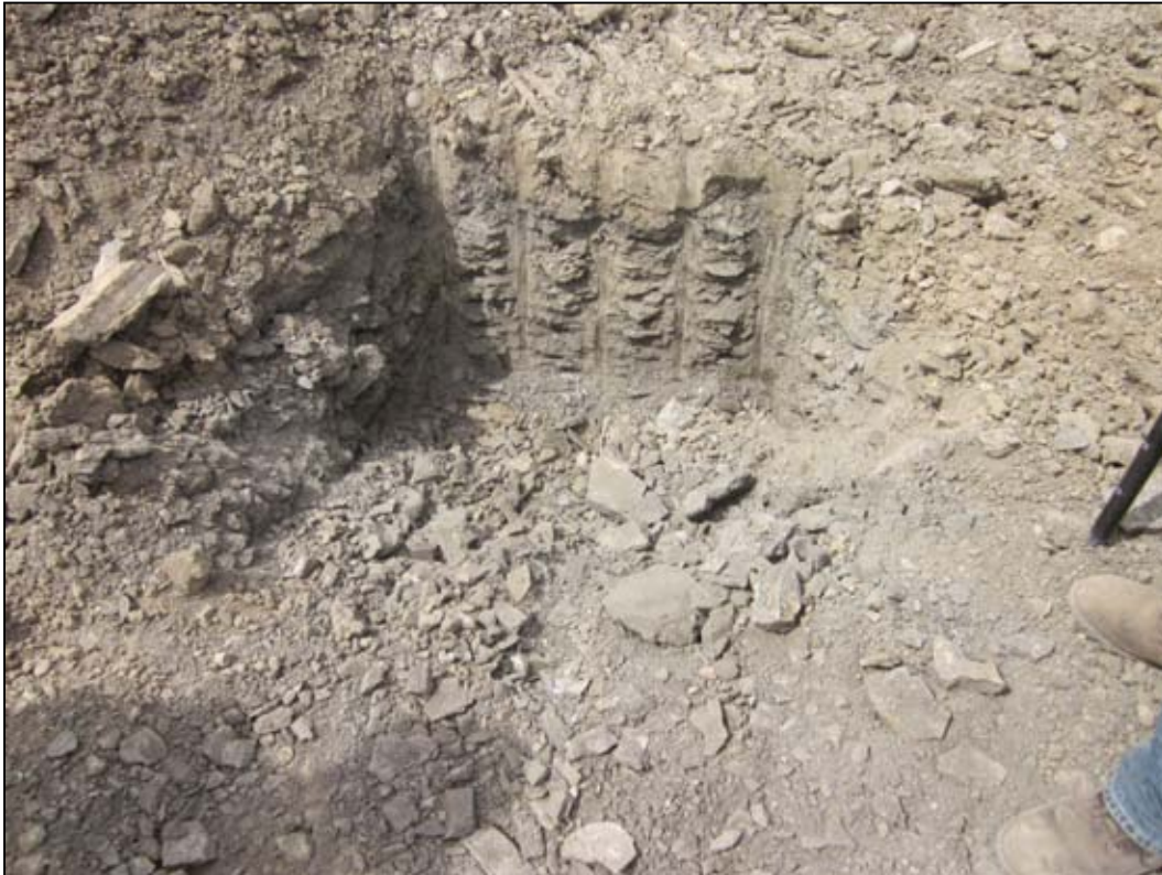
Photo 65. Standpipe Sump June 3, 2011
