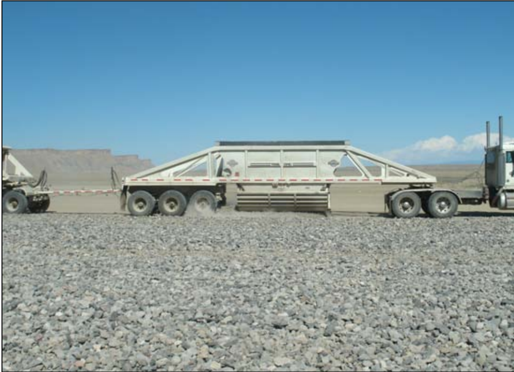
Photo 54. Cap Rock Placement August 11, 2011
