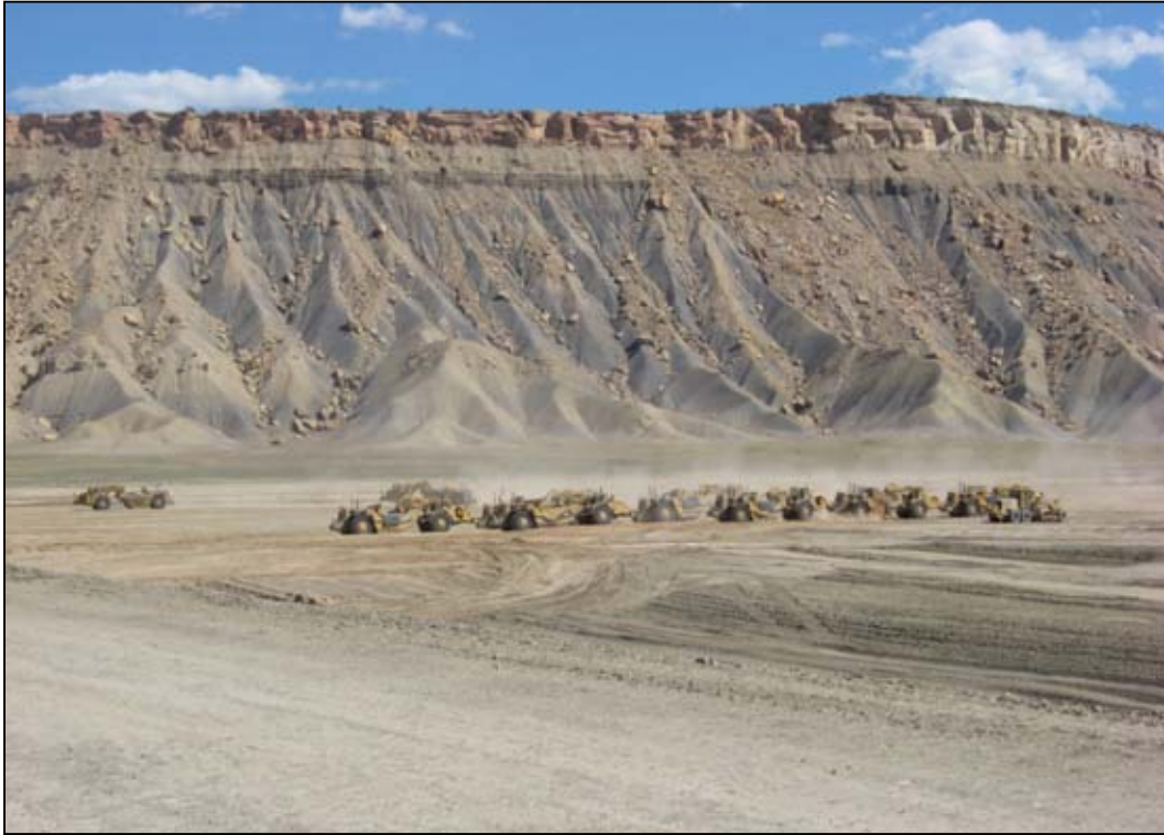
Photo 5. Cell Excavation August 18, 2008
