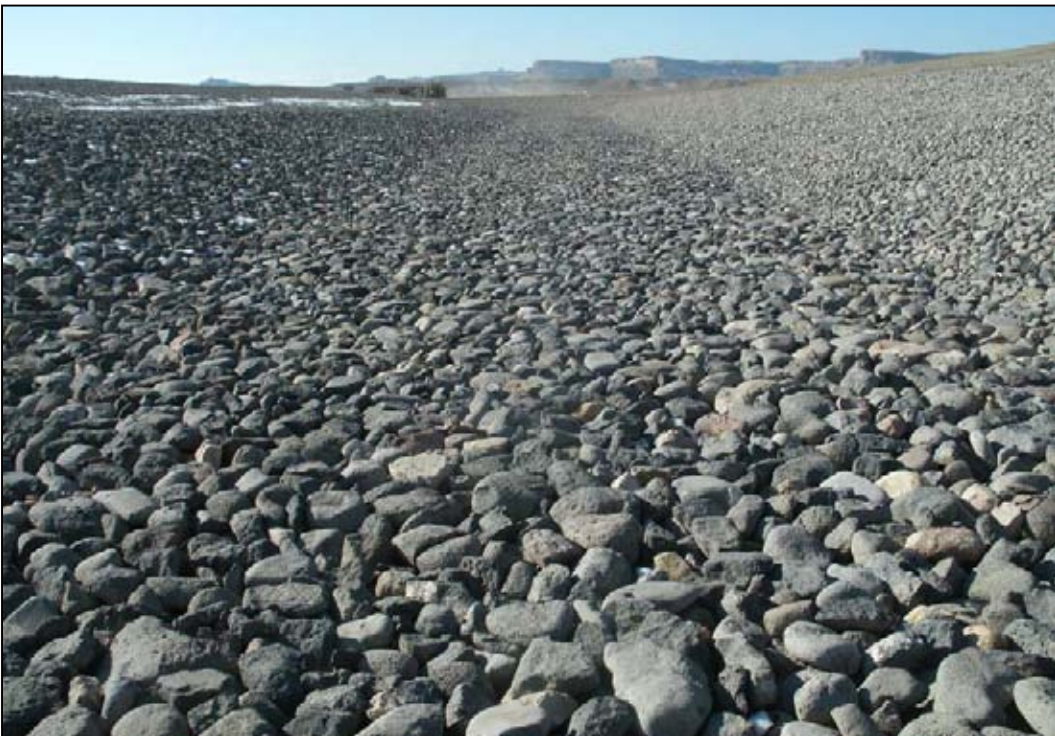
Photo 61. Northern Apron Armor Placement December 21, 2011
