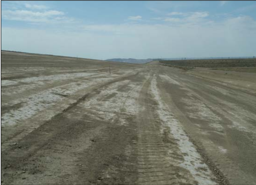
Photo 50. Western Embankment Prepared for Armor July 6, 2011
