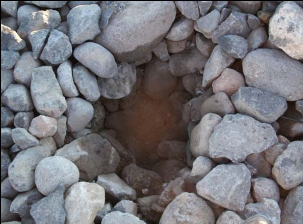
Photo 60. Northern Apron Thickness Verification Test Hole December 20, 2011
