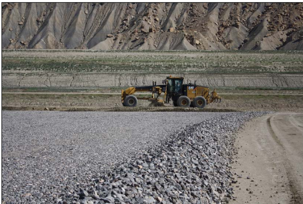
Photo 46. Frost Protection Layer Grading June 23, 2011
