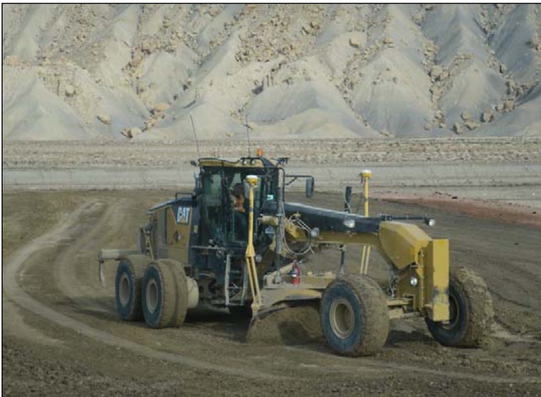
Photo 31. Grading Interim Cover December 1, 2011
