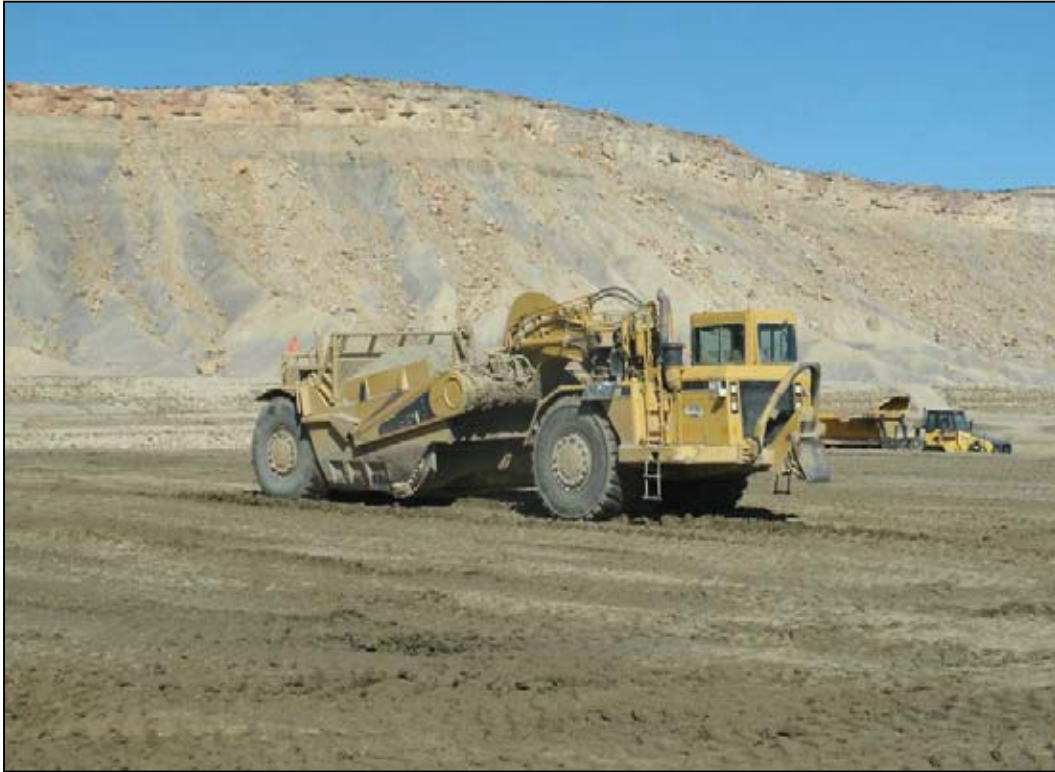
Photo 38. Radon Barrier Compaction with Scraper October 20, 2011
