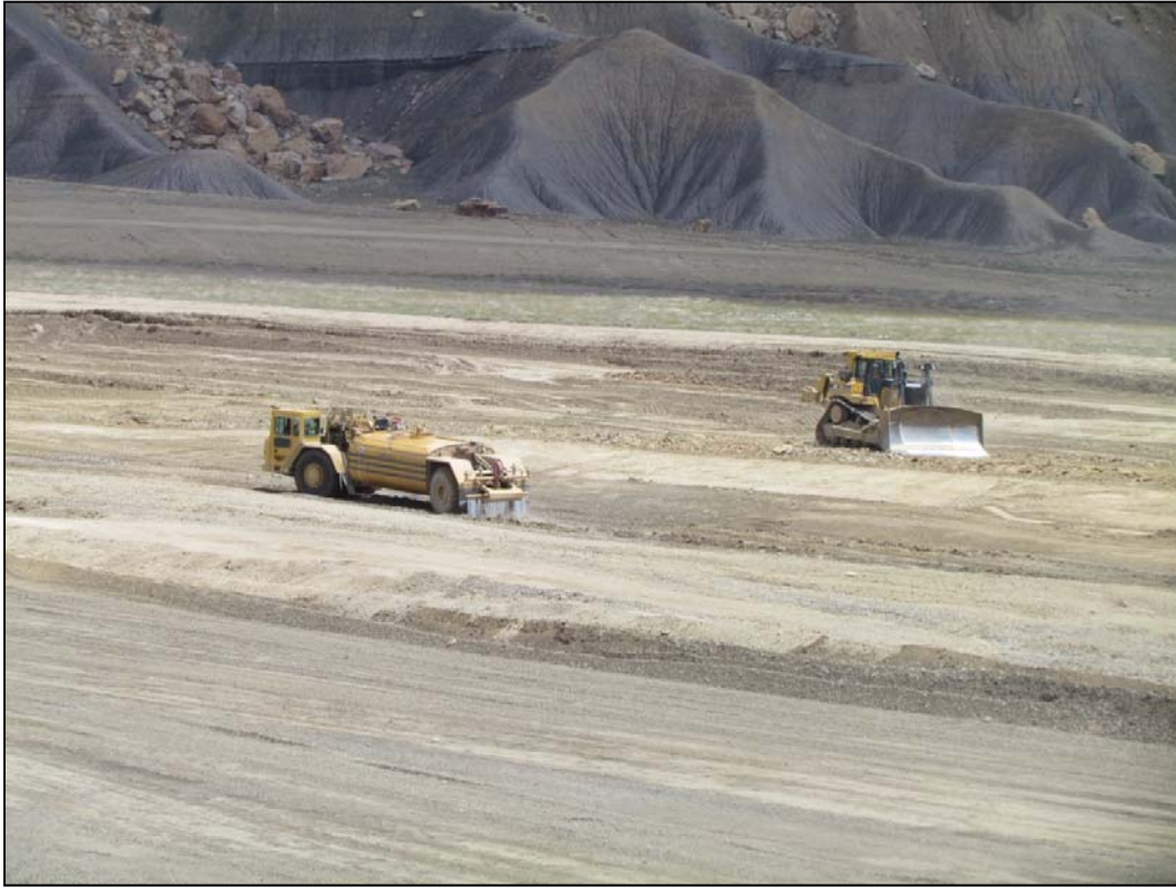
Photo 32. Radon Barrier Material Processing May 9, 2011
