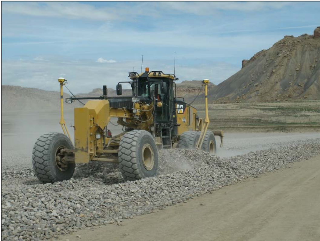
Photo 42. Infiltration and Biointrusion Barrier Grading June 17, 2011
