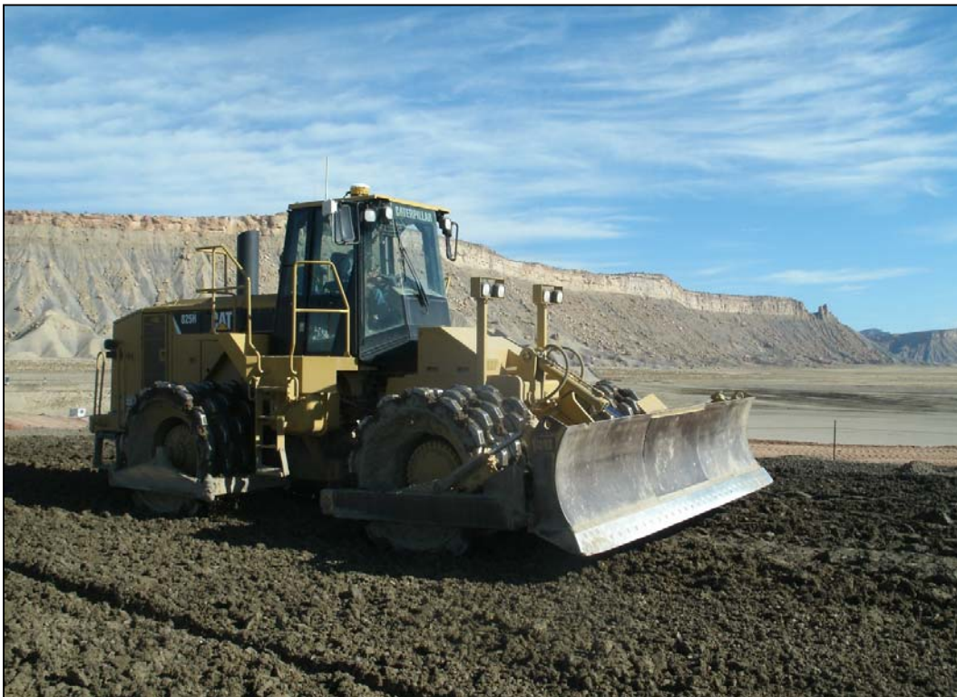
Photo 39. Radon Barrier Compaction October 21, 2011
