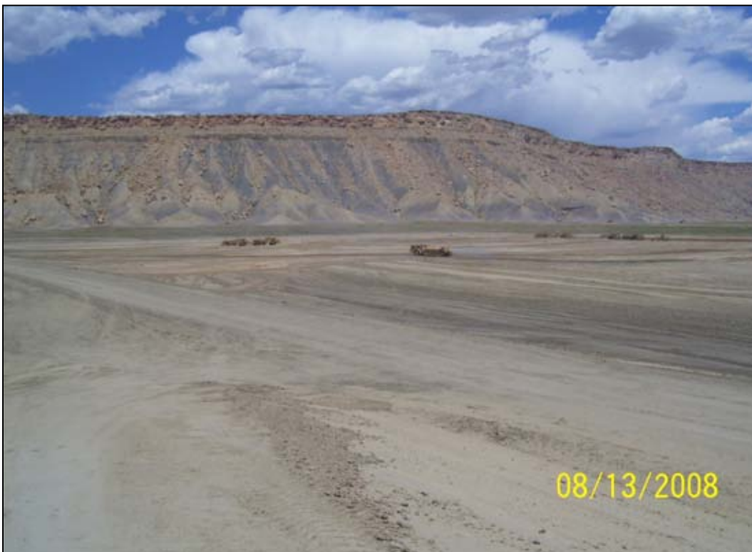
Photo 4. Cell Excavation August 13, 2008
