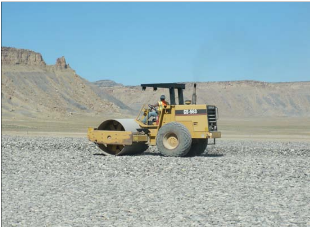
Photo 55. Cap Rock Compaction August 11, 2011
