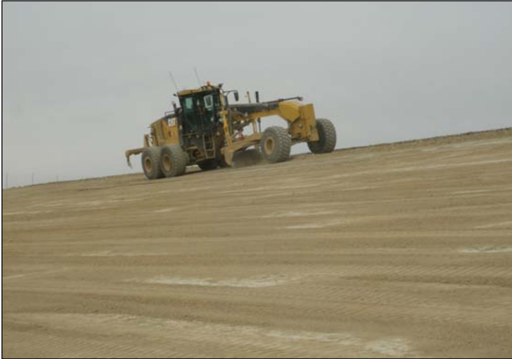
Photo 62. Southern Embankment Preparation for Armor December 12, 2011
