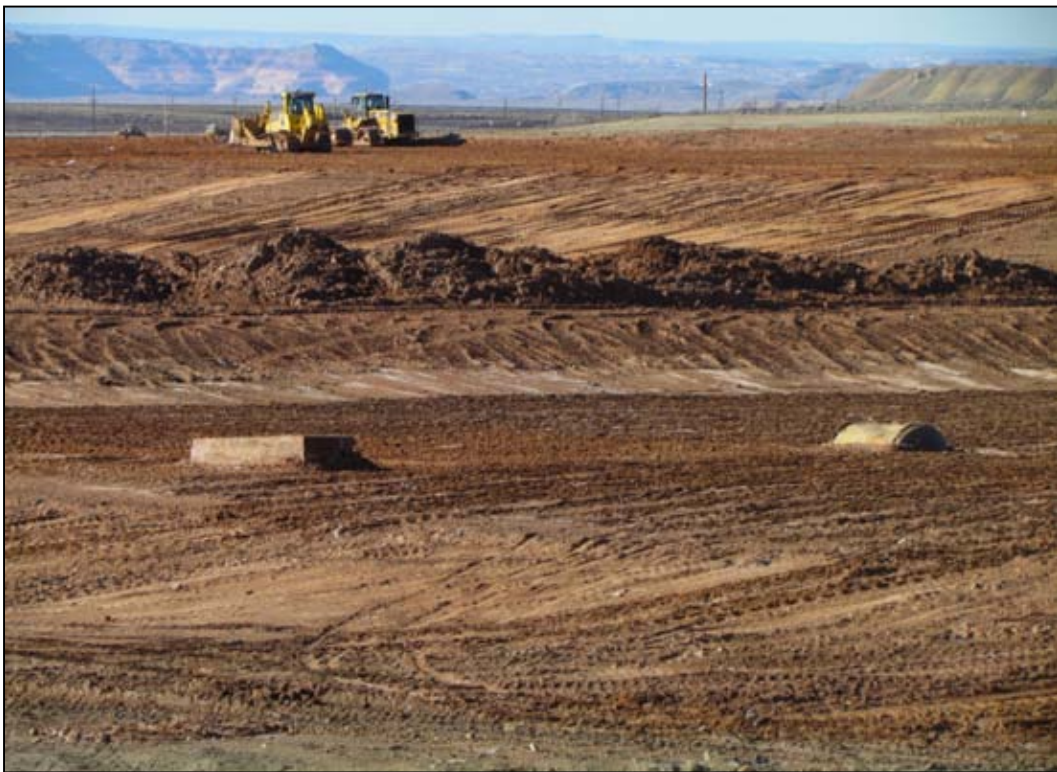
Photo 21. Oversized Debris Placement March 9, 2011
