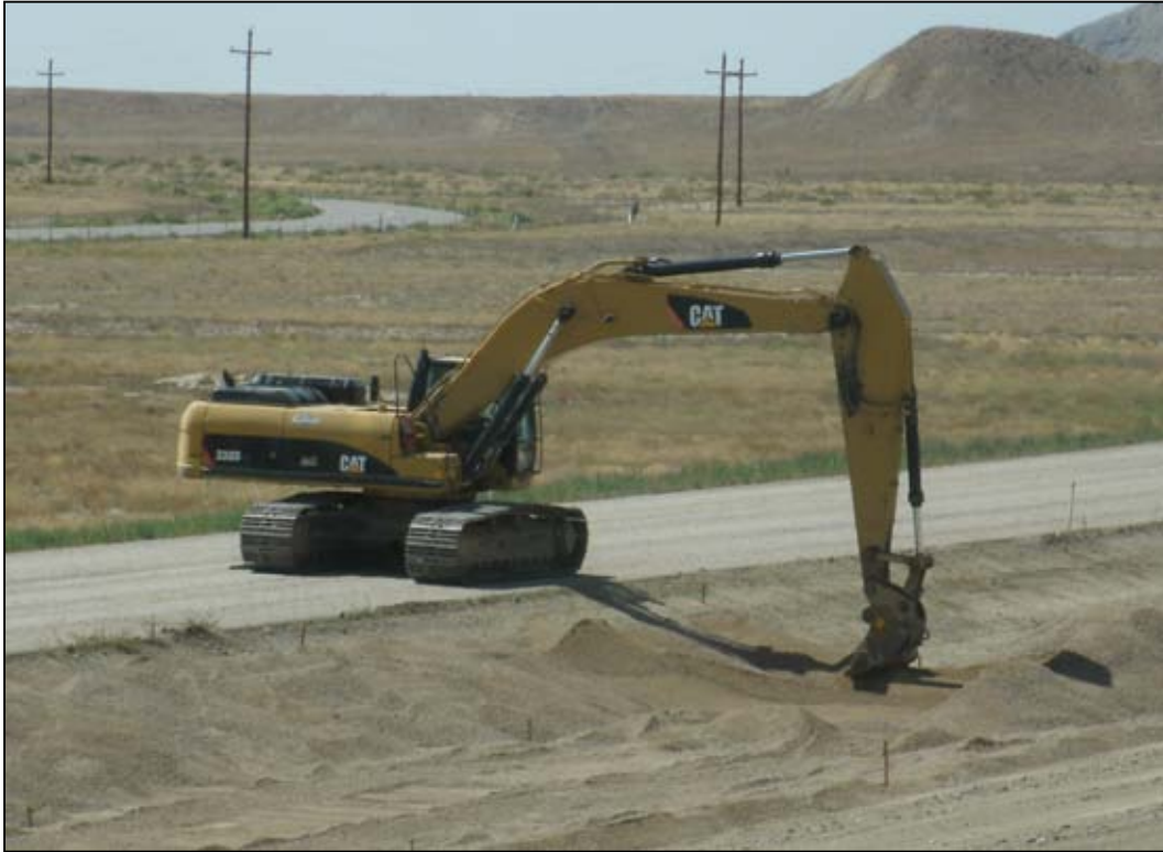
Photo 56. Southern Apron Bedding Placement September 8, 2011
