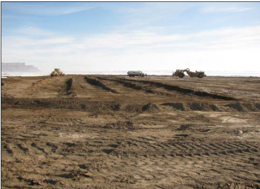
Photo 8. Cell Excavation January 13, 2010
