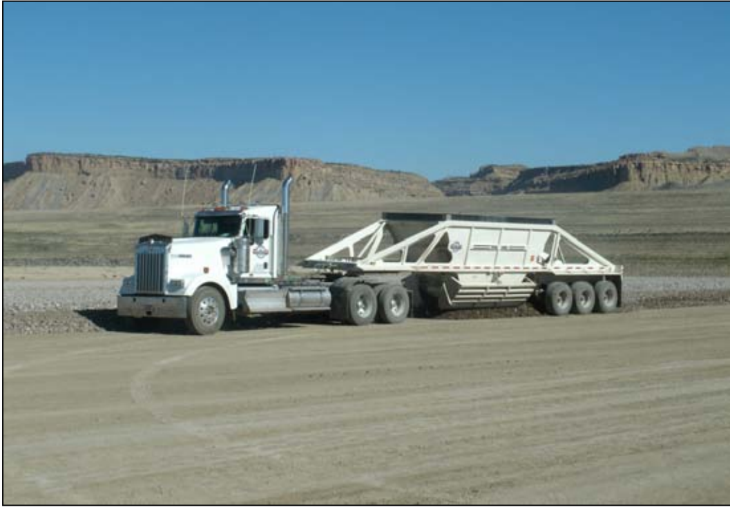
Photo 41. Infiltration and Biointrusion Barrier Placement June 15, 2011
