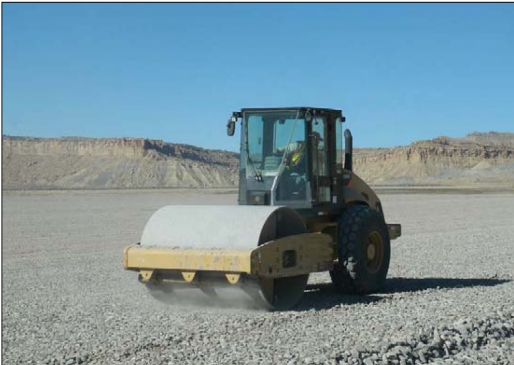
Photo 44. Infiltration and Biointrusion Barrier Smooth Drum rolling for Buyoff November 3, 2011
