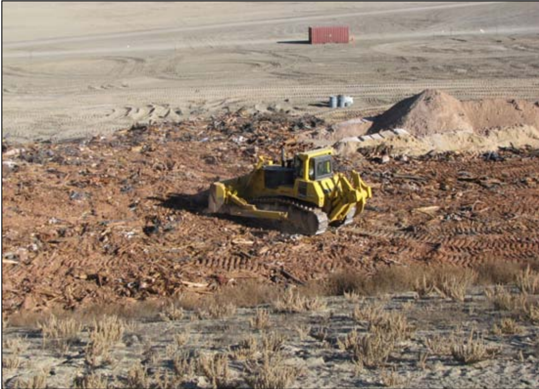
Photo 16. Debris Being Spread Out Across the Lift Area November 30, 2009
