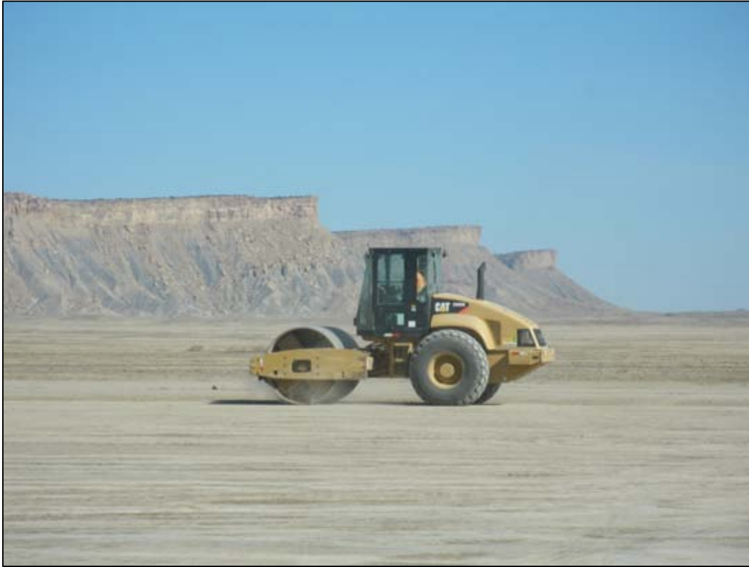
Photo 40. Radon Barrier Smooth Drum Rolling for Buyoff
