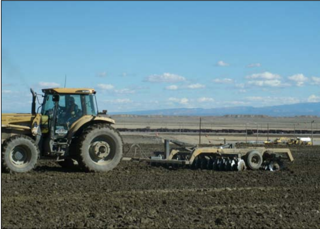
Photo 36. Radon Barrier Material Preparation October 11, 2011
