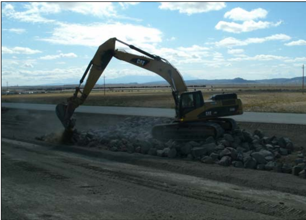
Photo 57. Southern Apron Armor Placement September 12, 2011
