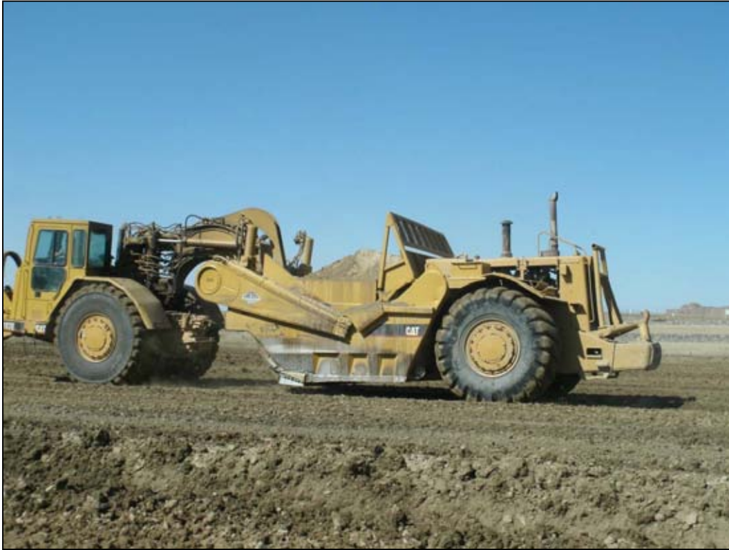
Photo 34. Radon Barrier Placement August 24, 2011
