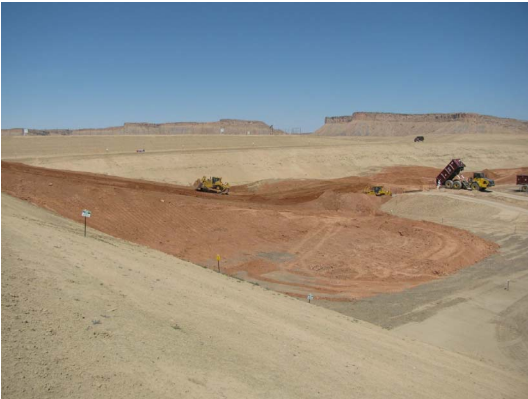
Photo 13. RRM Placement May 18, 2009
