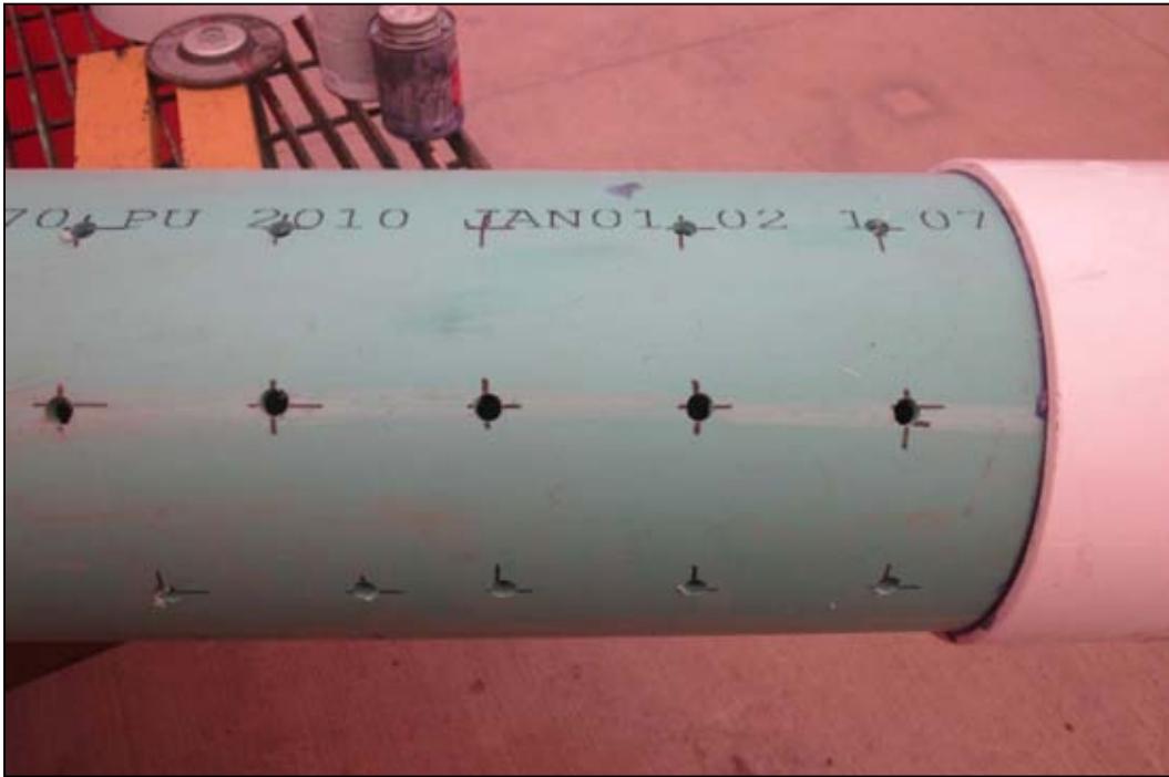
Photo 64. Standpipe Screen Perforations June 2, 2011
