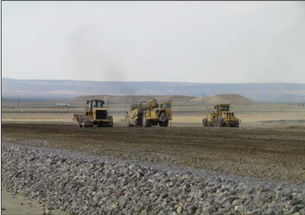
Photo 47. Frost Protection Layer Placement, Grading, and Compaction June 29, 2011
