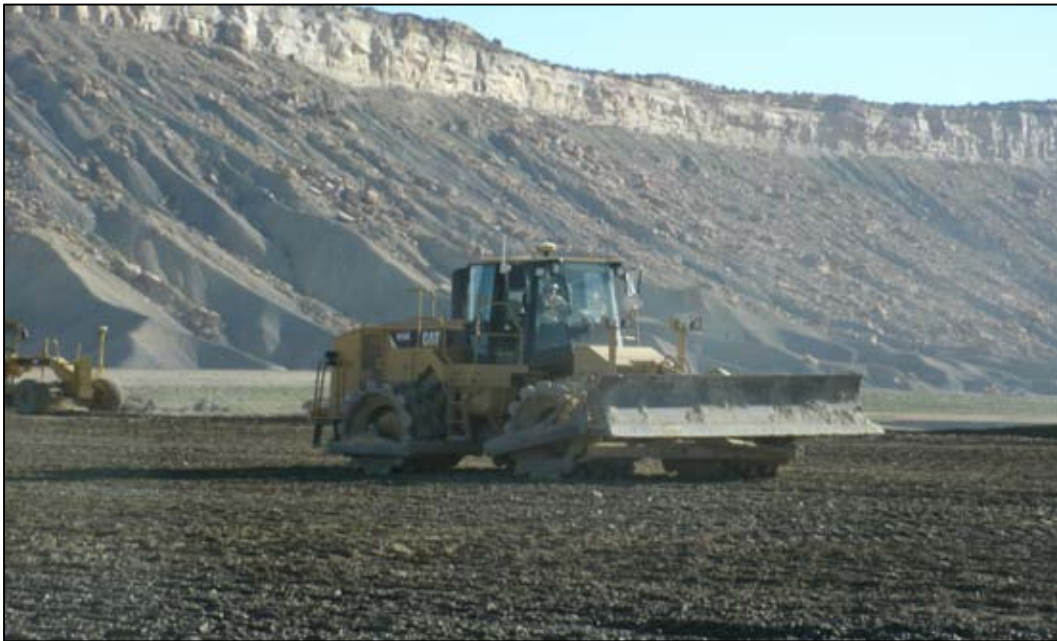
Photo 29. Interim Cover Compaction August 10, 2011
