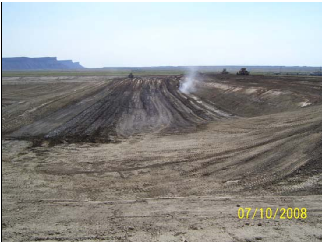
Photo 2. Cell Excavation South Perimeter Embankment Placement July 10, 2008
