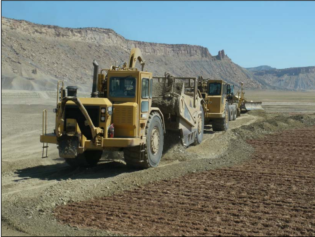
Photo 28. Interim Cover Placement August 8, 2011
