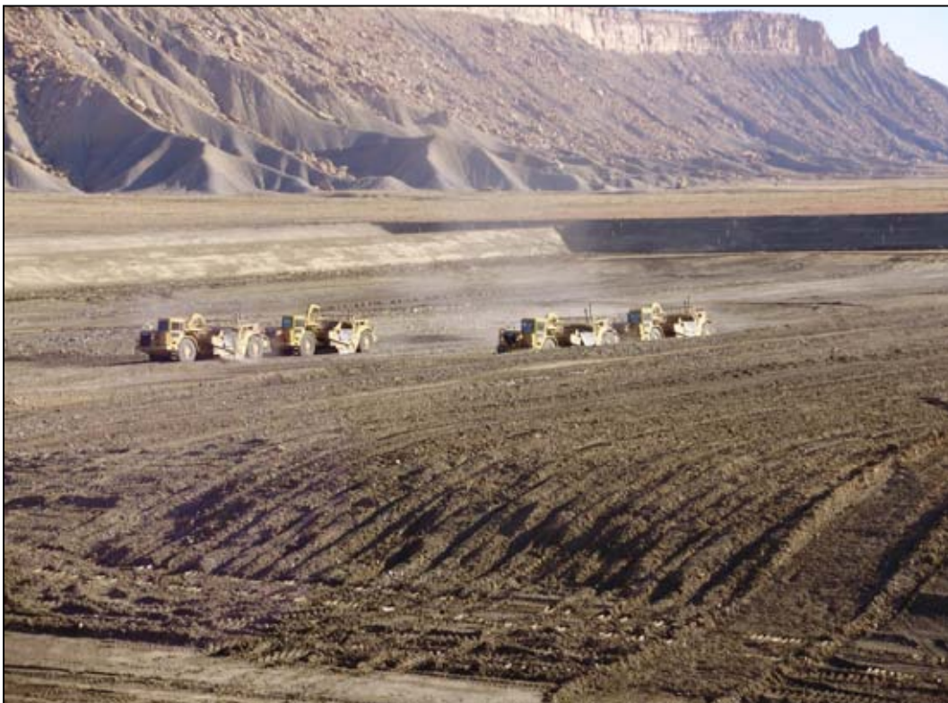
Photo 6. Cell Excavation October 6, 2008
