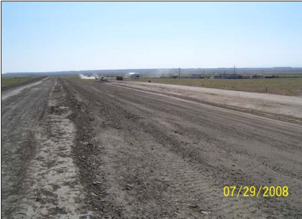
Photo 3. South Embankment Final Grade July 29, 2008
