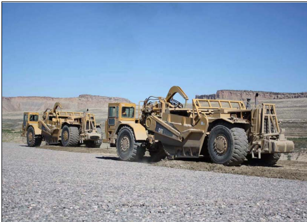
Photo 45. Frost Protection Layer Placement June 22, 2011
