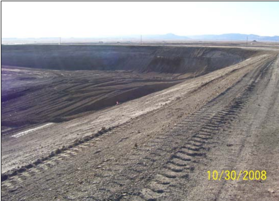
Photo 7. Cell Excavation October 30, 2008
