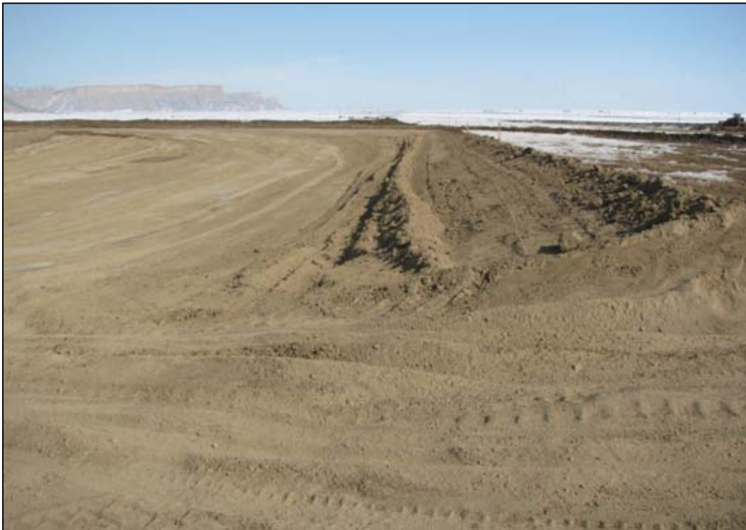
Photo 10. Cell Excavation February 17, 2010
