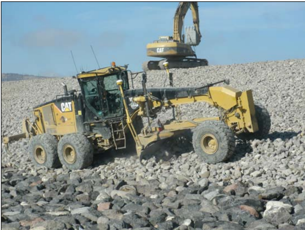
Photo 63. Southern Embankment Armor Grading December 16, 2011
