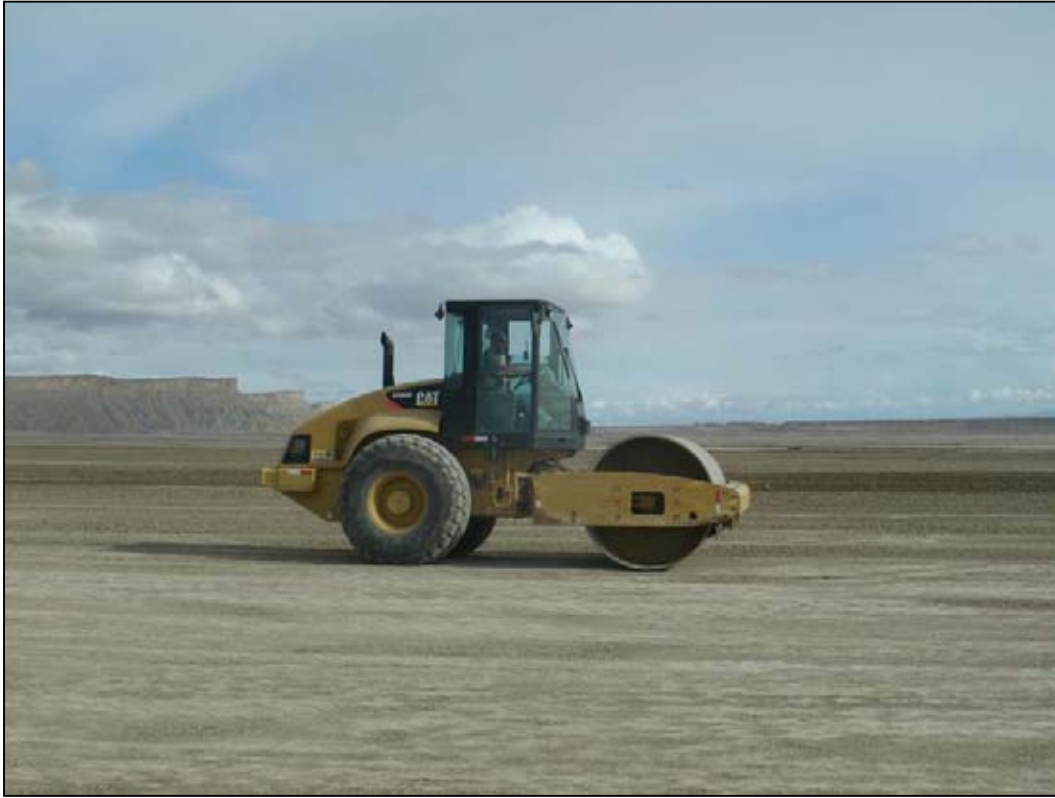
Photo 49. Frost Protection Layer Smooth Drum Rolling for Buyoff November 21, 2011
