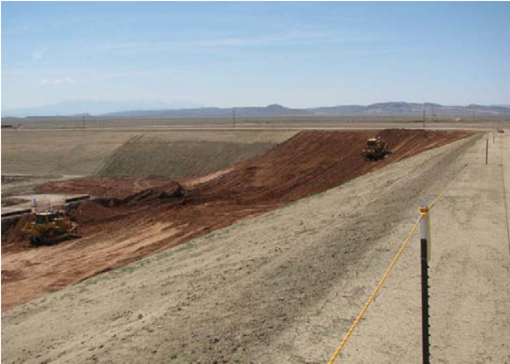
Photo 12. RRM Placement May 18, 2009
