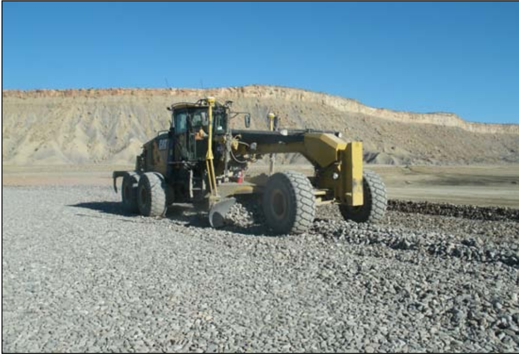
Photo 58. Cap Rock Grading August 29, 2011
