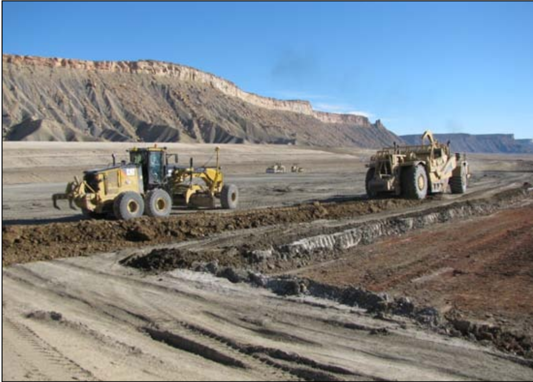
Photo 24. Interim Cover Placement March 1, 2011
