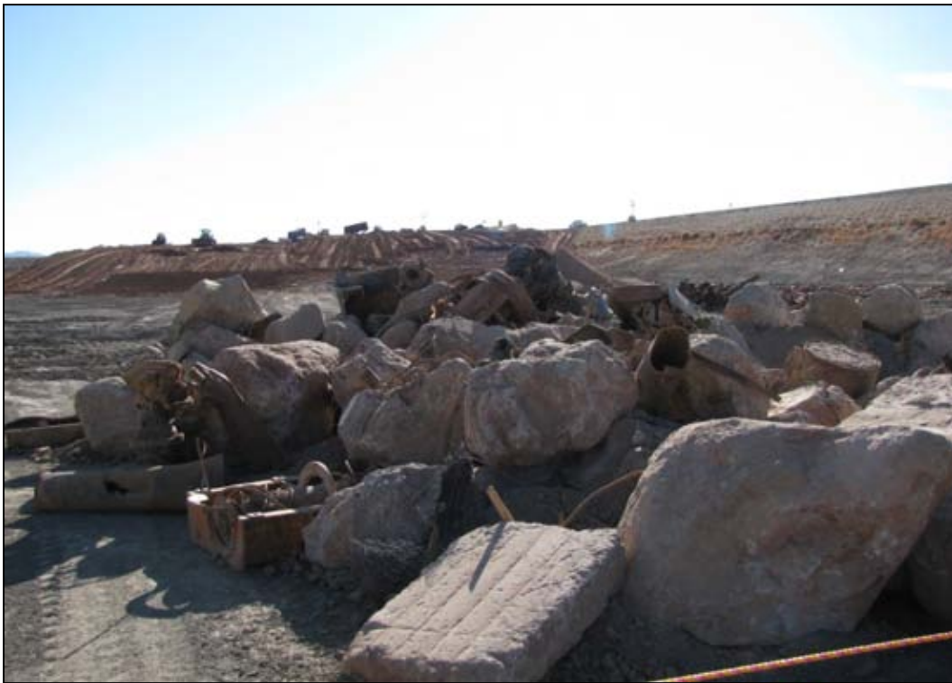
Photo 17. Oversized Debris for Sizing Before Placement December 1, 2009
