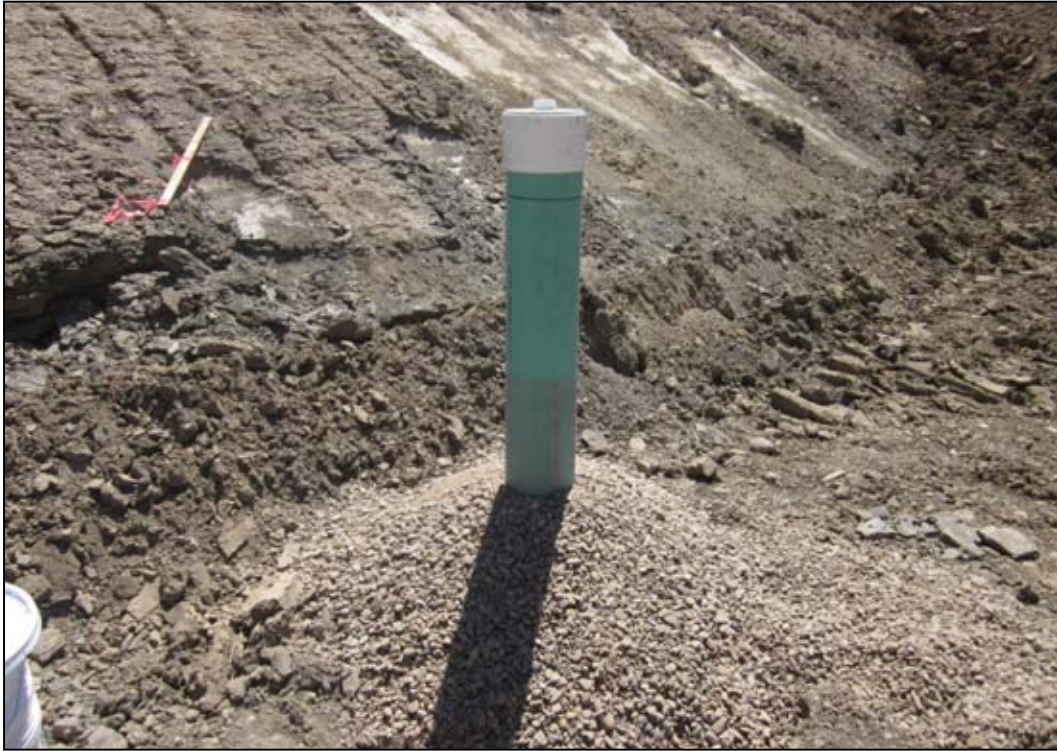
Photo 66. Standpipe Placed with Sandpack June 3, 2011
