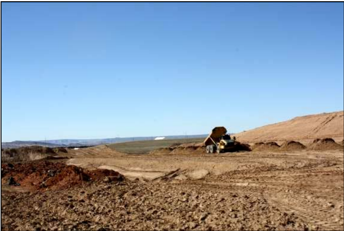
Photo 22. Unloading Material for Compaction April 2019
