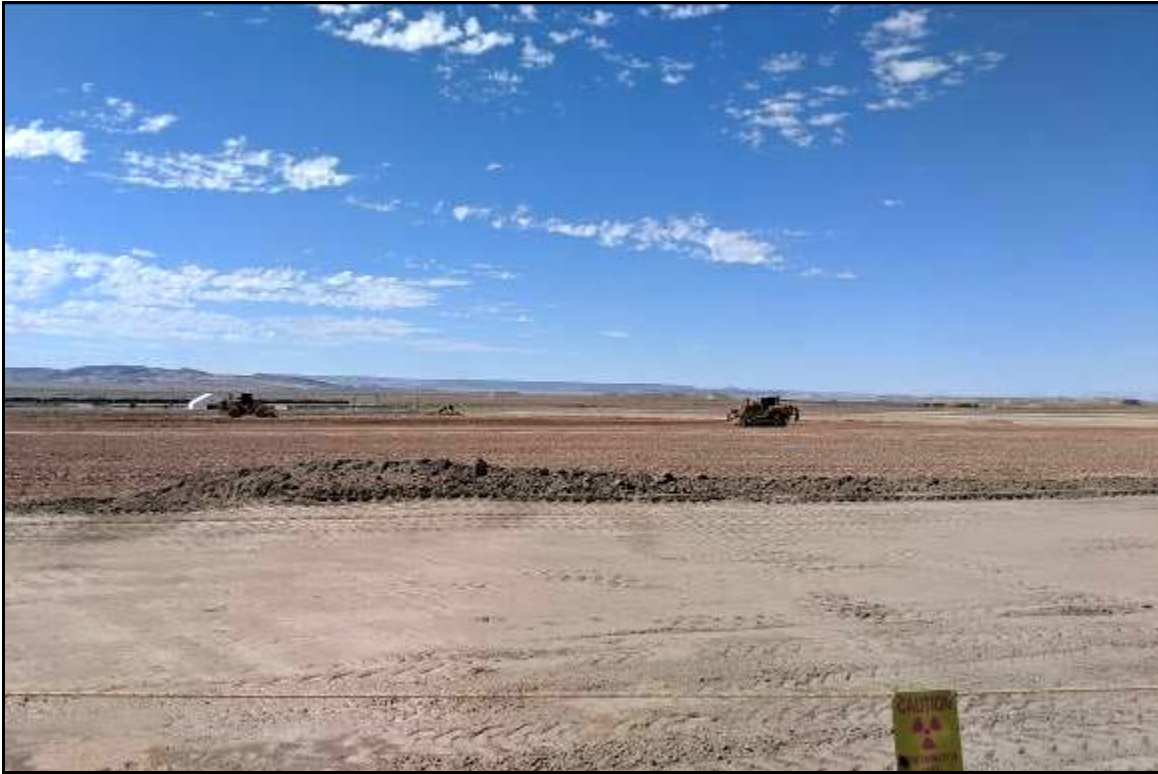
Photo 28. Bulldozer Cutting Final Grade of RRM June 2019
