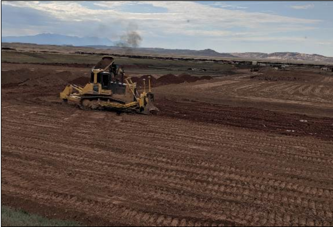
Photo 30. Bulldozer Pushing Material Over Debris July 2019
