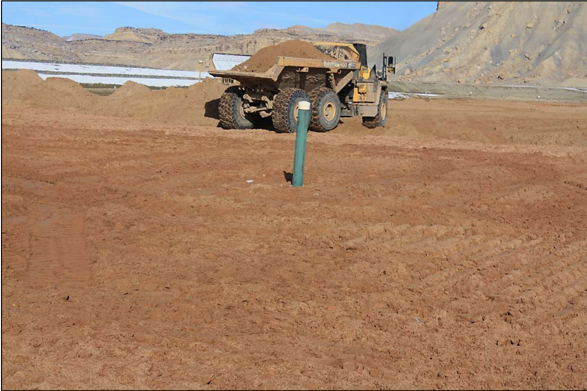
Photo 15. Material near Standpipe after Compaction January 2019
