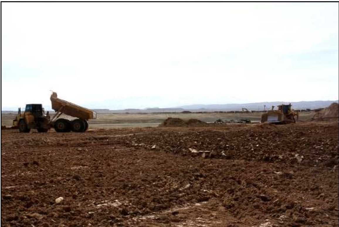
Photo 20. Unloading Material for Compaction March 2019
