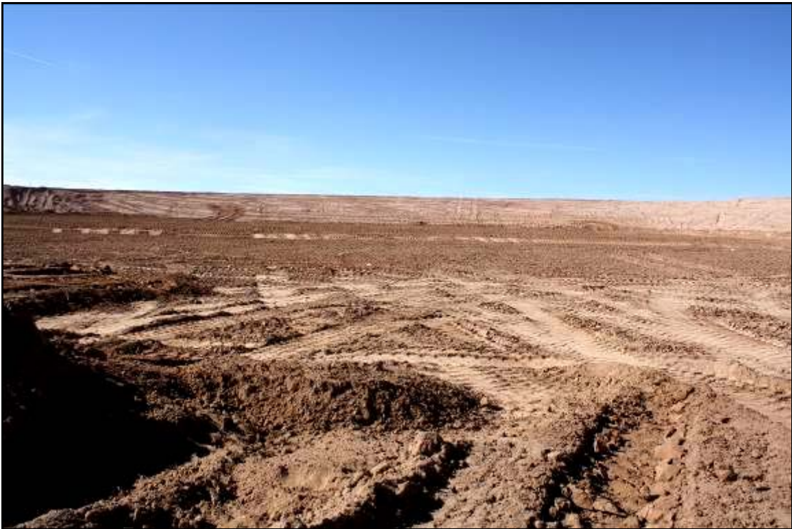
Photo 8. Lift Areas Ready for Placement November 2018
