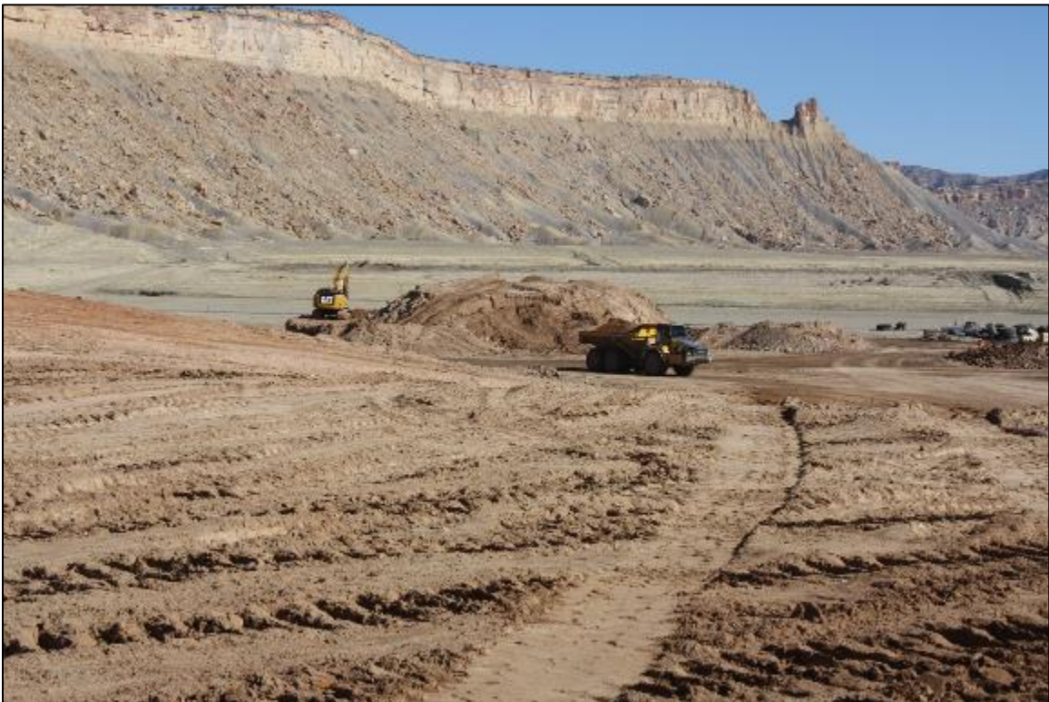
Photo 6. Loading and Hauling Stockpiled Material November 2018
