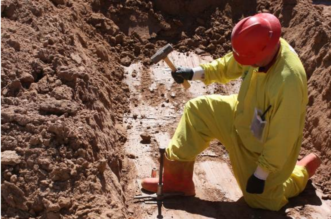
Photo 3. Quality Control Preparing In-place Density Test October 2018
