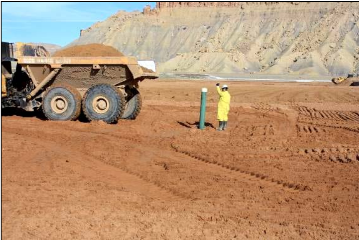
Photo 14. Compacting near Standpipe with Loaded Haul Truck January 2019
