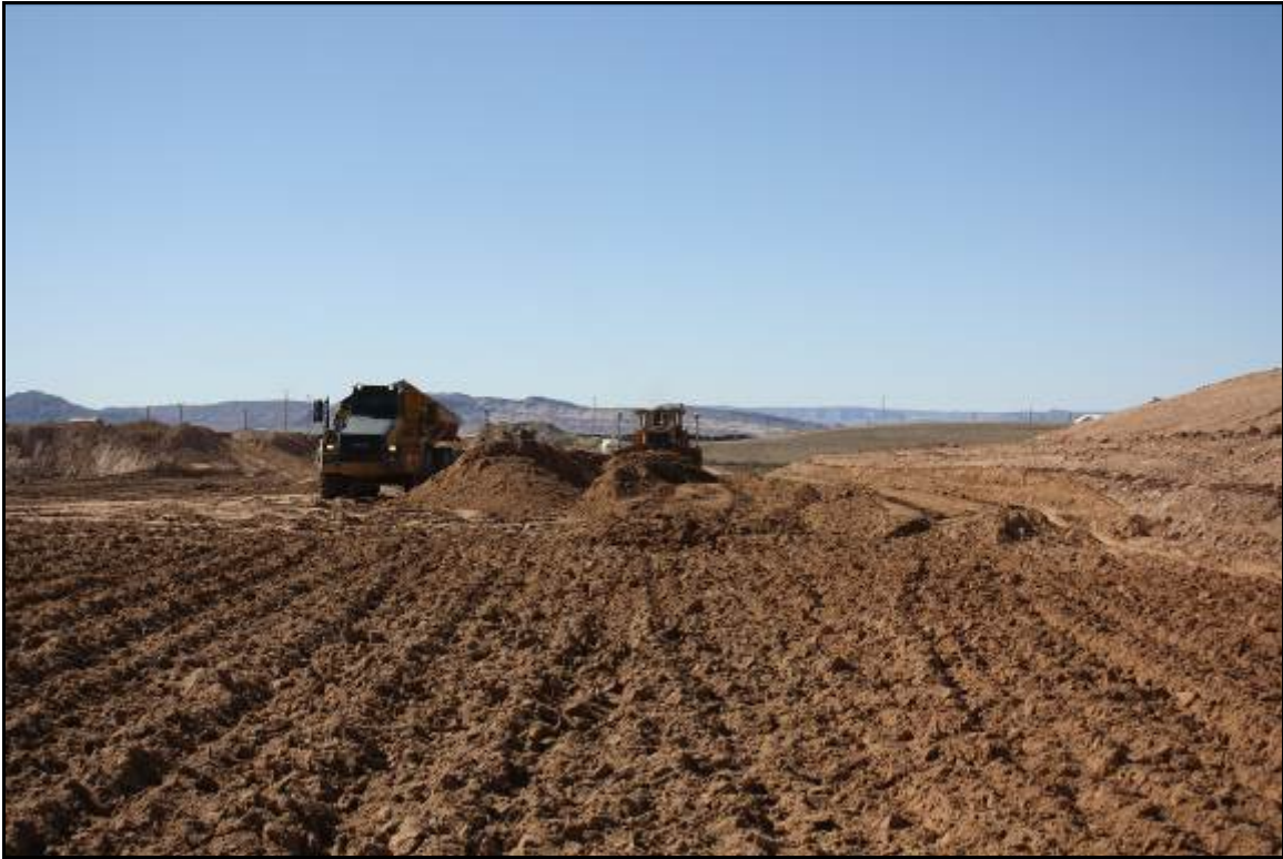
Photo 23. Placing Material with Bulldozer April 2019
