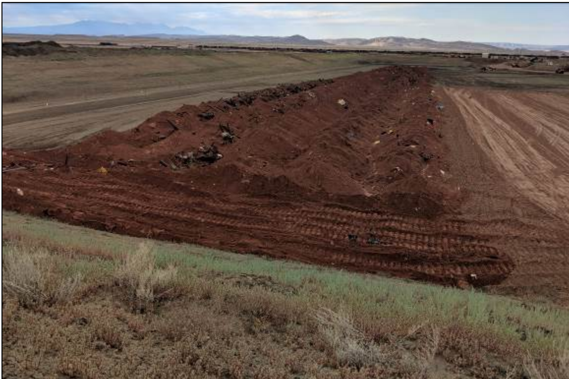
Photo 31. Beginning Placement of Sacrificial Lift July 2019
