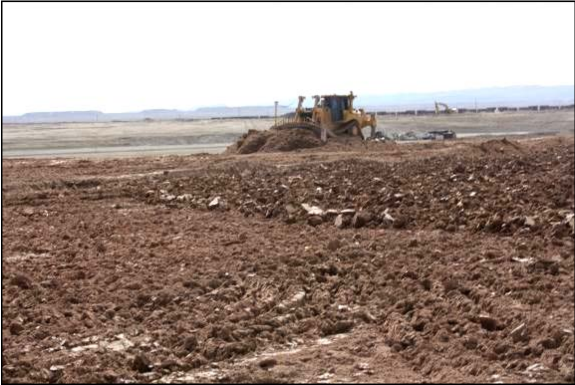
Photo 19. Placing Material with Bulldozer March 2019
