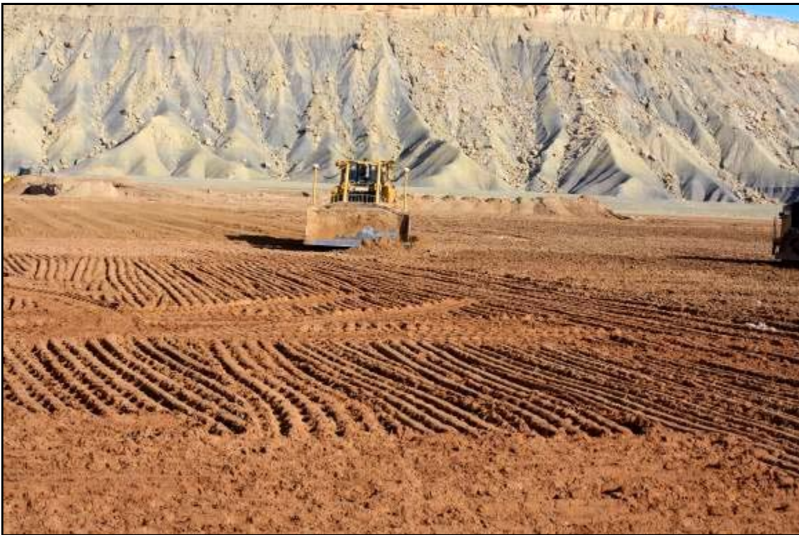
Photo 12. Placing Material with Bulldozer January 2019
