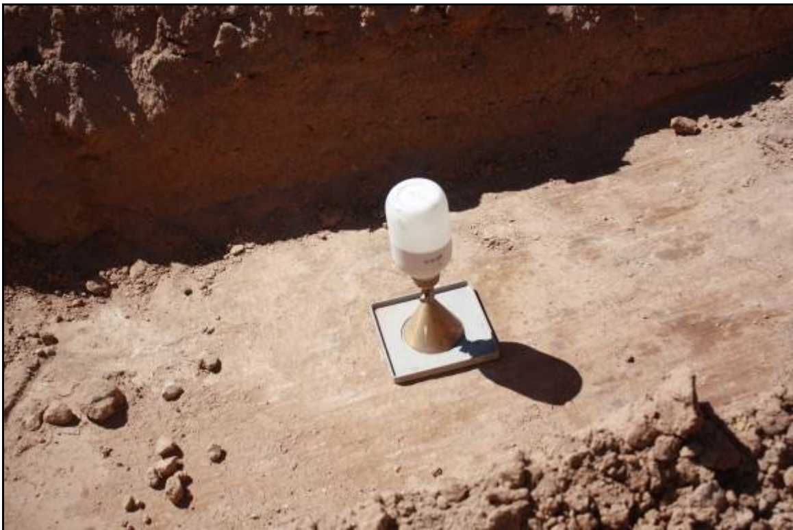
Photo 4. Quality Control Performing In-place Density Test October 2018
