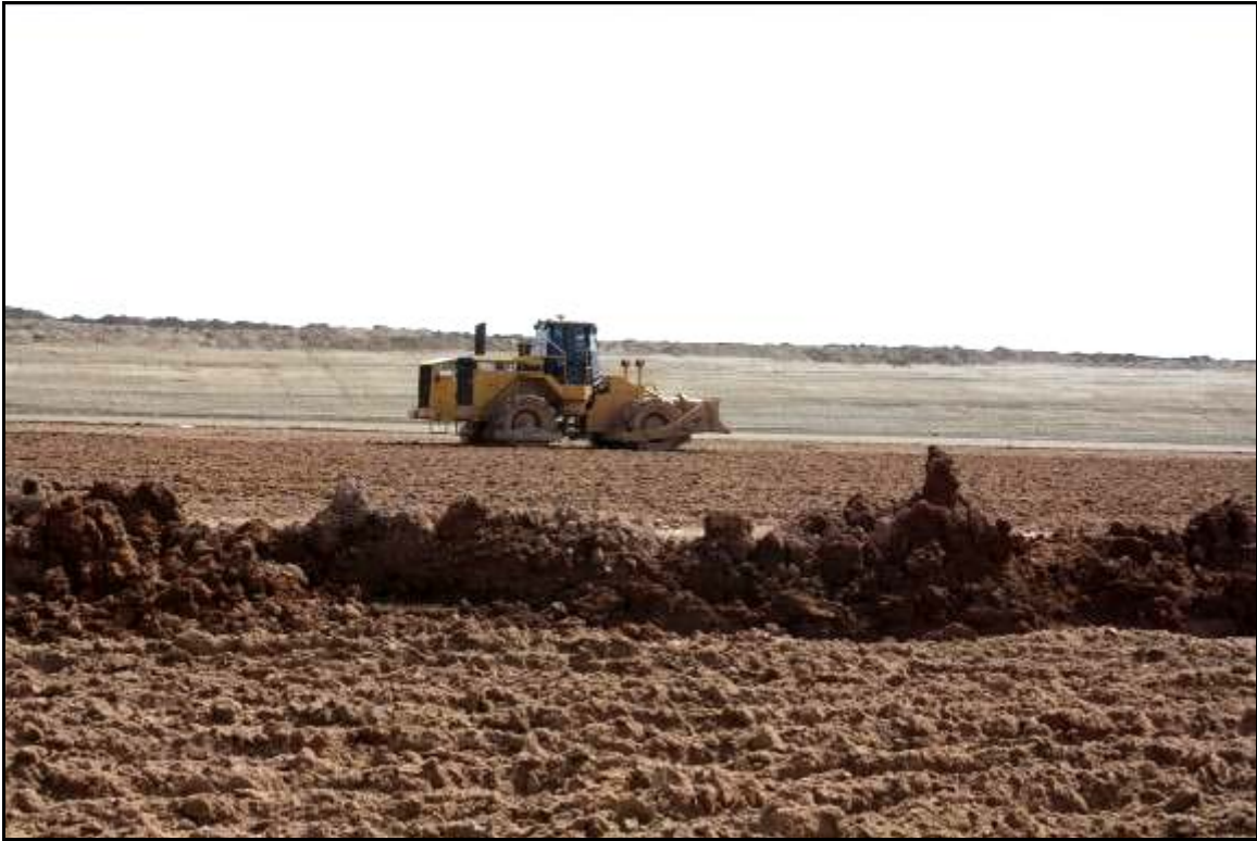
Photo 21. Compacting Lift with Sheepsfoot March 2019
