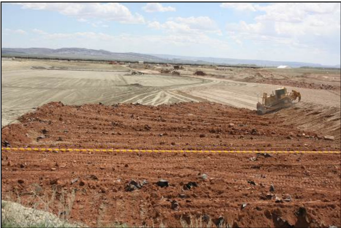
Photo 26. Bulldozer Pushing Debris in a Two-foot Lift May 2019
