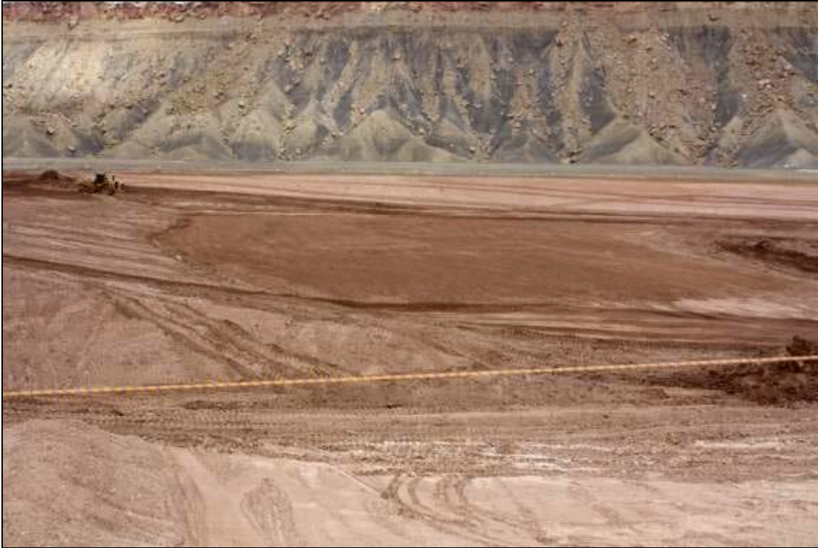
Photo 17. Finished RRM Lift February 2019
