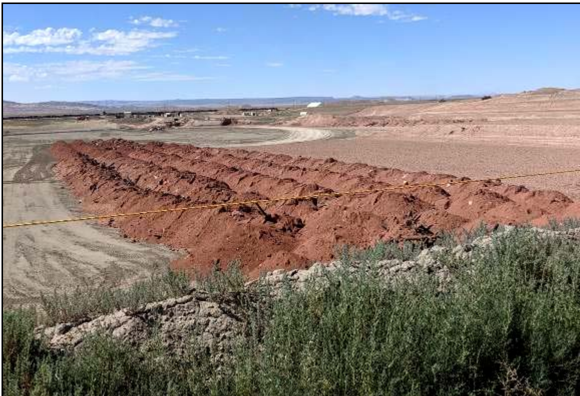
Photo 29. Debris Ready for Placement in Sacrificial Lift June 2019
