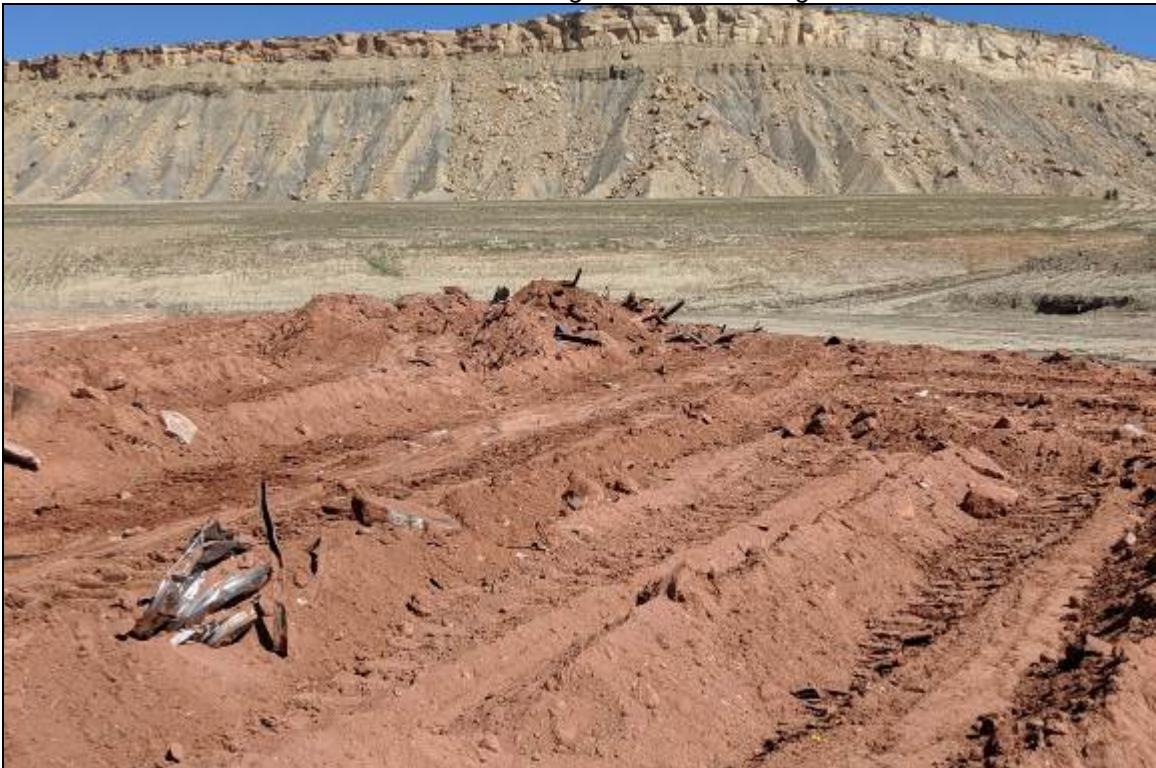
Photo 33. Placement of Sacrificial Lift August 2019
