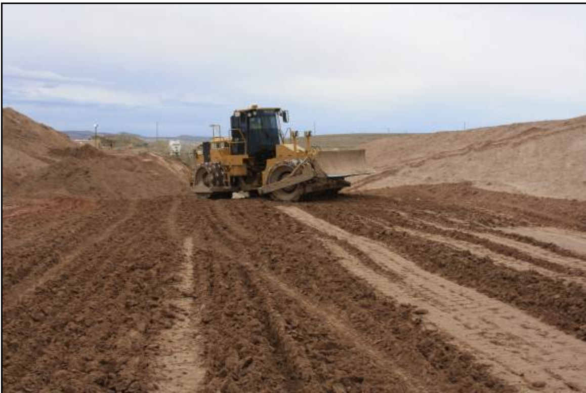
Photo 2. Sheepfoot Compacting a Lift Area October 2018
