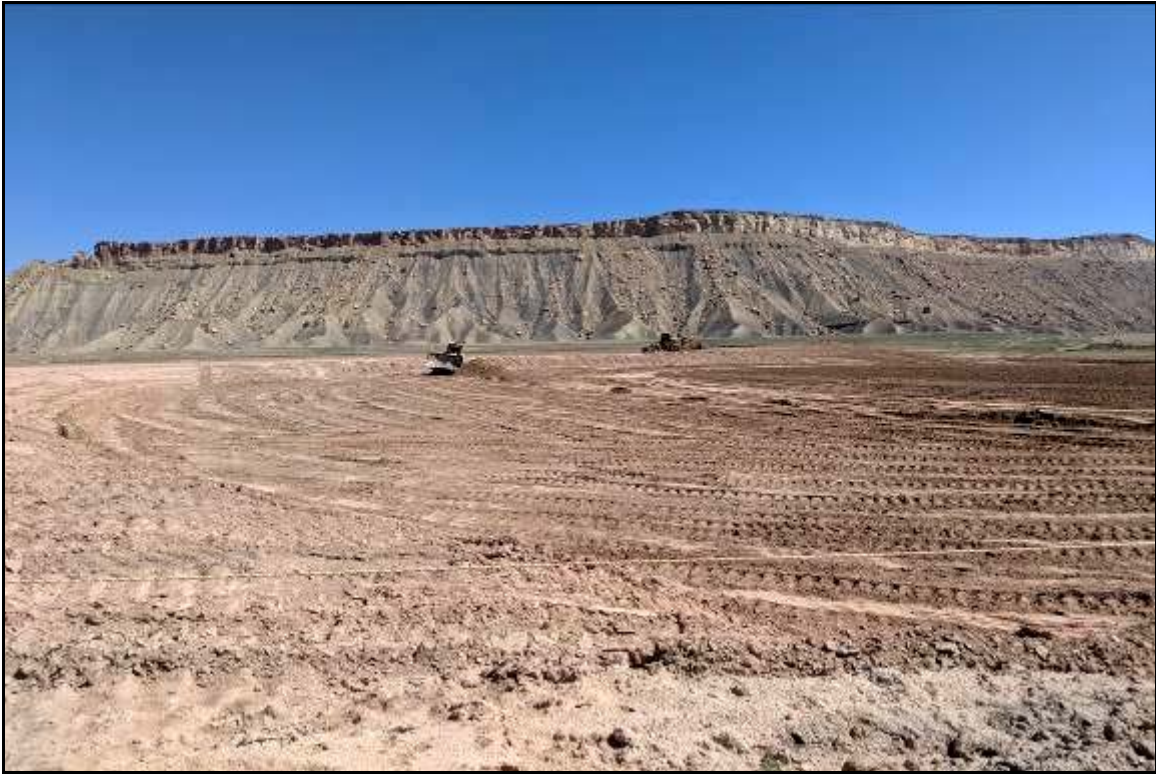
Photo 27. Placement of Last Seven Feet of Design Grade June 2019
