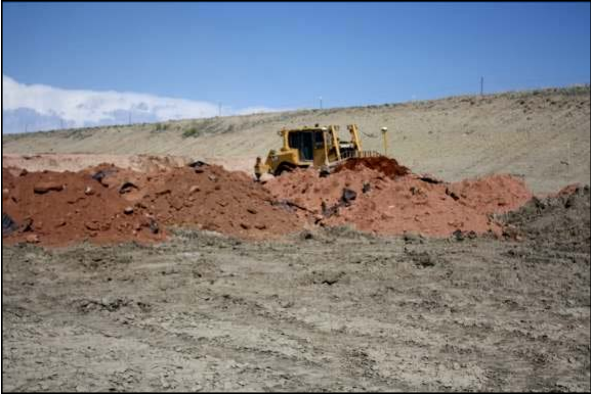
Photo 25. Pushing Debris with Bulldozer May 2019
