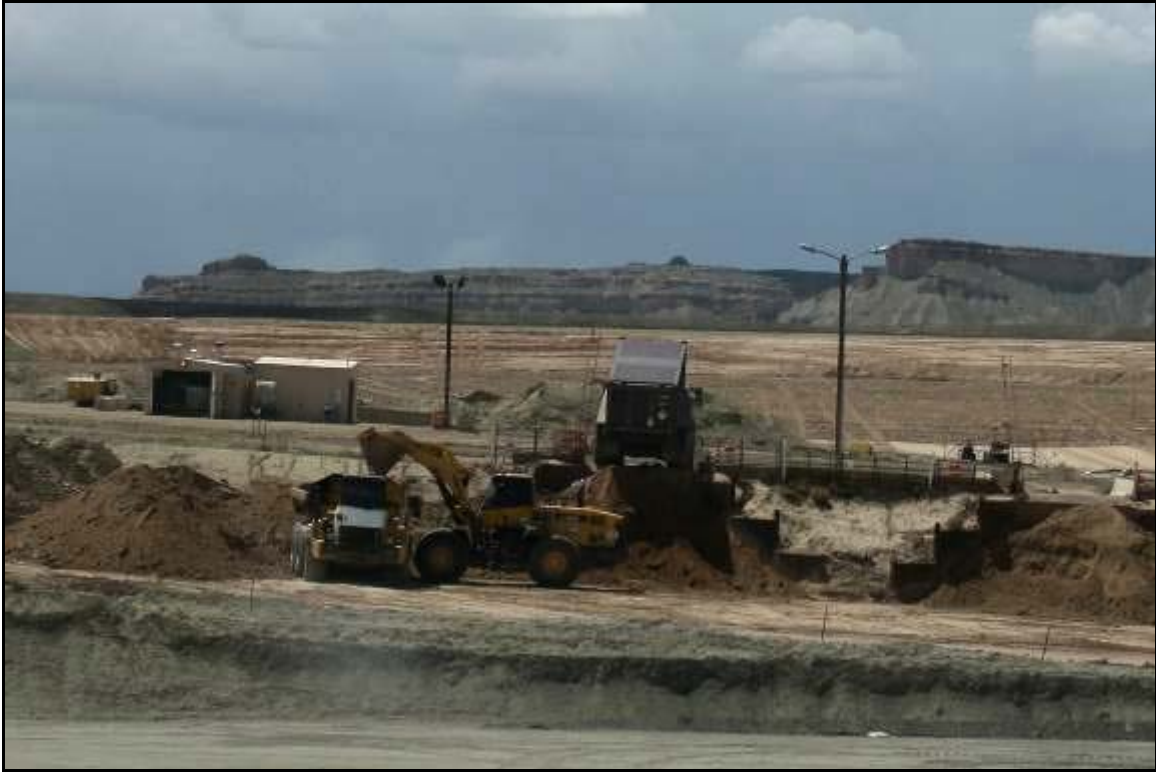
Photo 9. Loading Material for Placement December 2018
