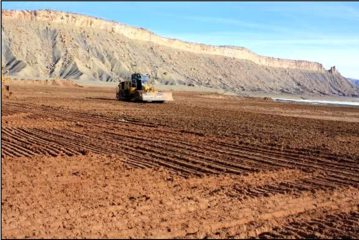
Photo 13. Compacting Lift Area with Sheepsfoot January 2019
