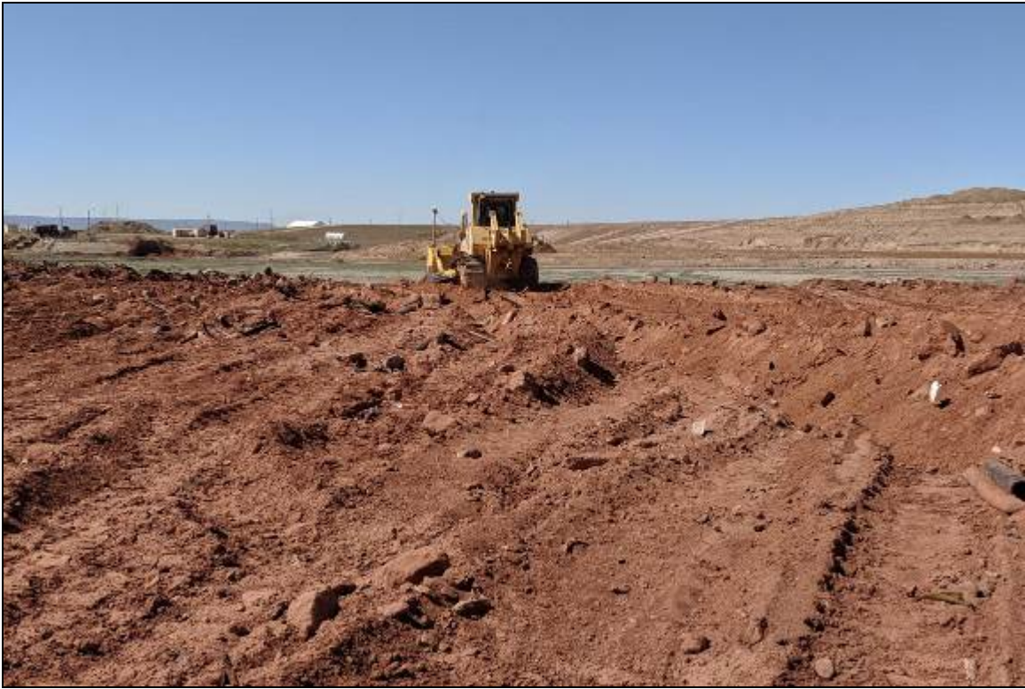
Photo 32. Bulldozer Pushing Sacrificial Lift August 2019
