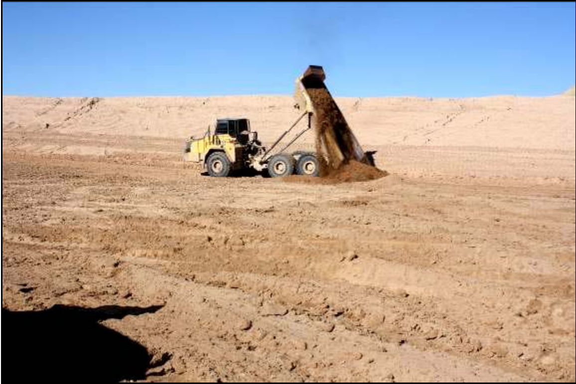
Photo 7. Haul Truck Dumping RRM November 2018
