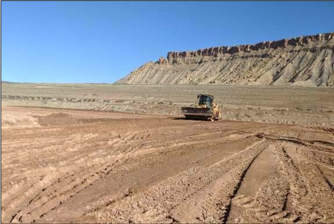
Photo 34. Sheepsfoot Compacting Lift Area September 2019
