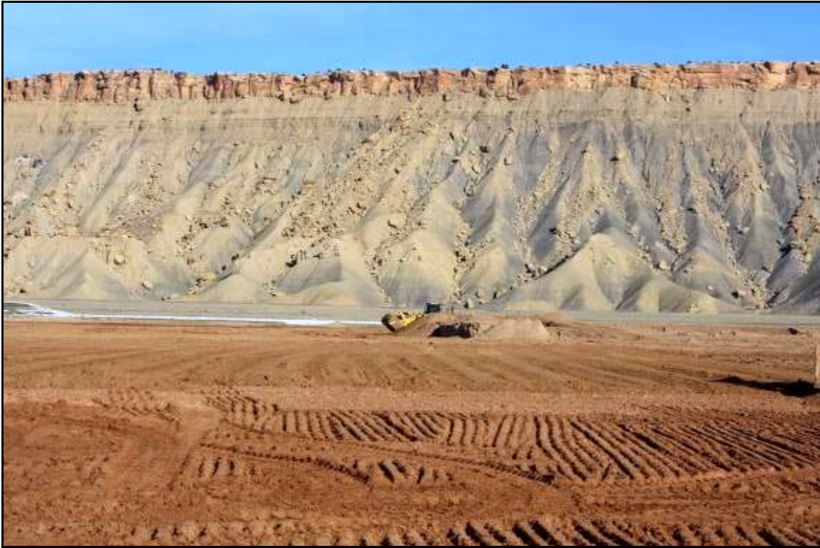
Photo 11. Loading Stockpiled Material for Lift Placement January 2019
