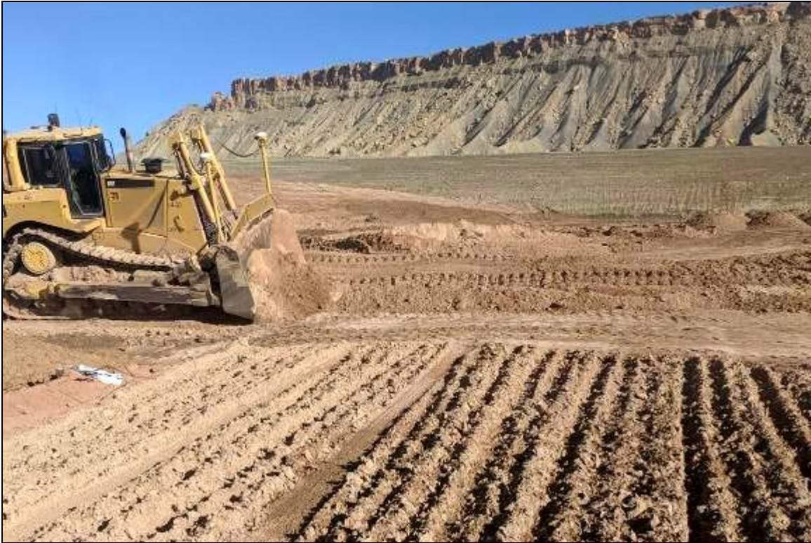
Photo 36. Bulldozer Placing Material September 2019
