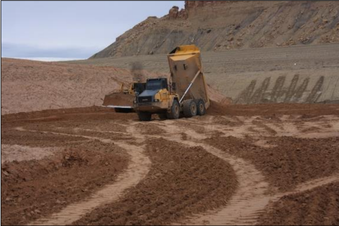
Photo 1. Operations Placing a Lift October 2018
