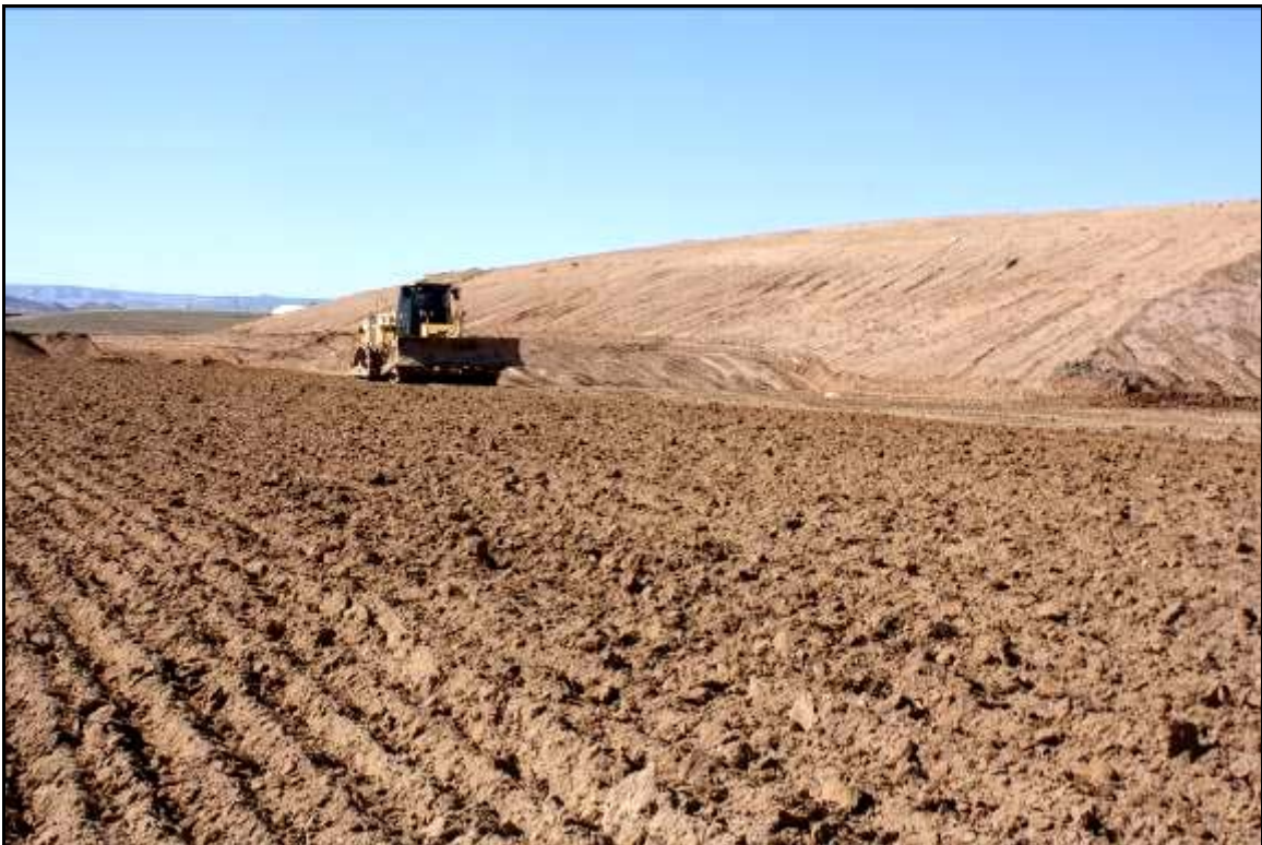
Photo 24. Compacting Lift Area with Sheepsfoot April 2019
