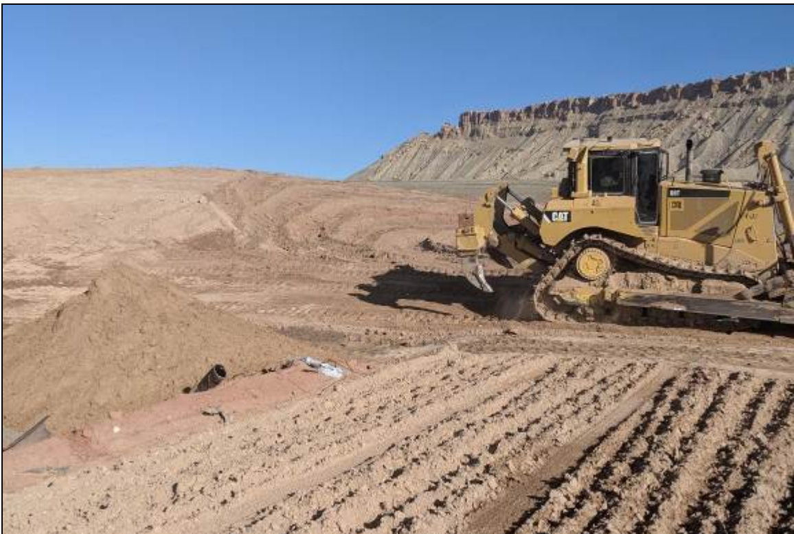
Photo 35. Bulldozer Cleaning Up Slopes September 2019
