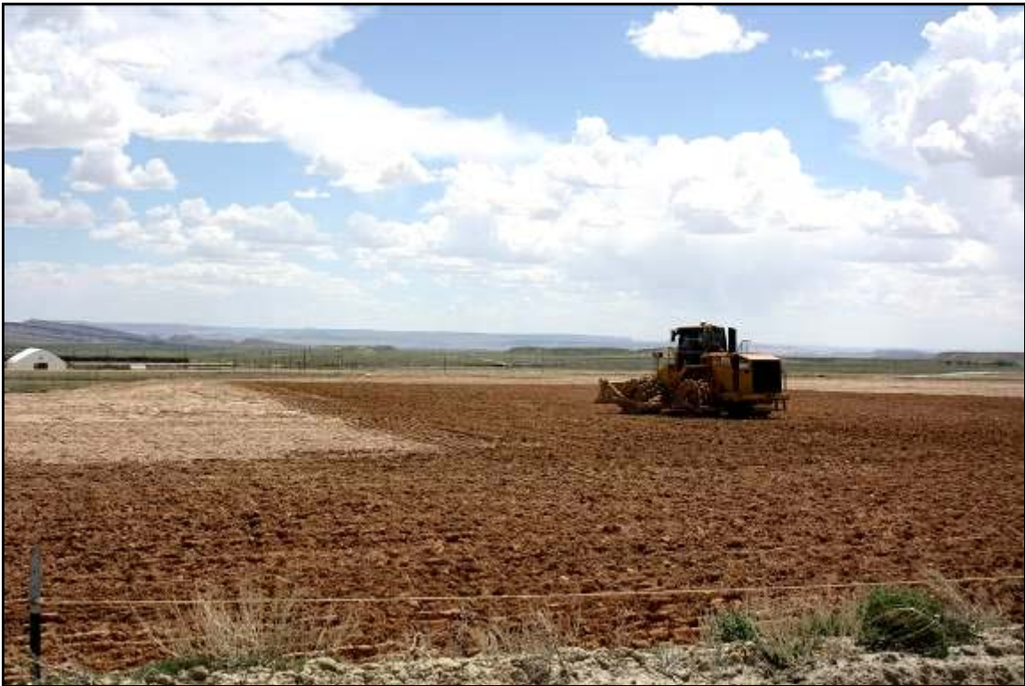
Photo 10. Sheepsfoot Compacting Lift December 2018
