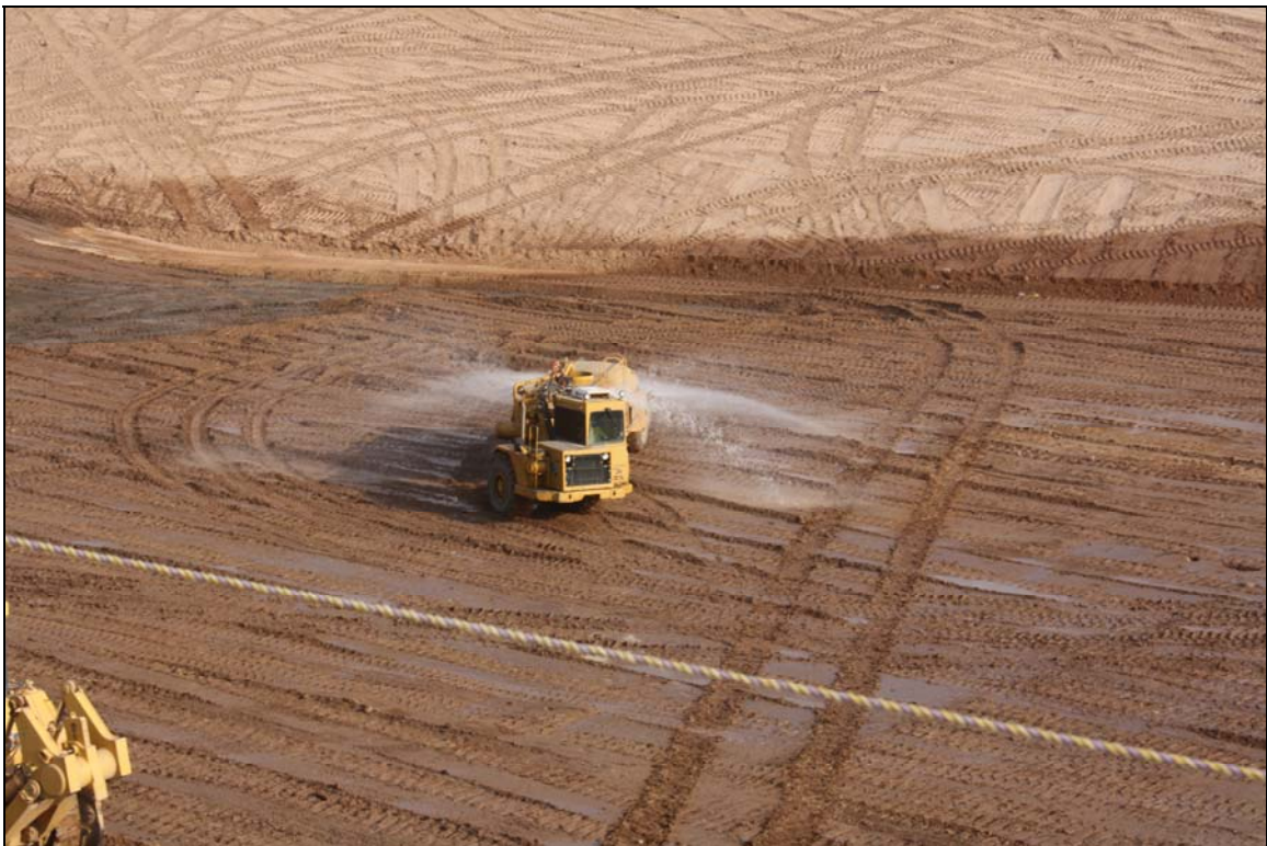
Photo 54. Watering Down of Lift Area August 2018
