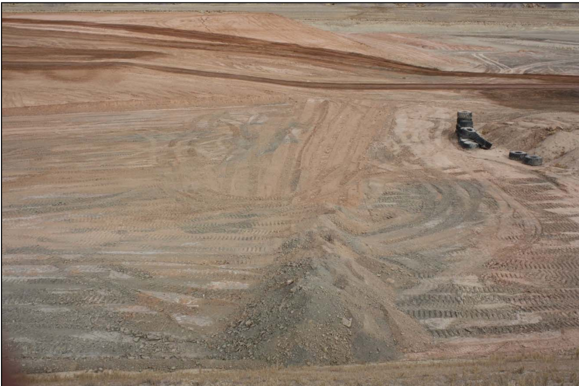
Photo 12. Water Diversion Bar in Cell November 2017
