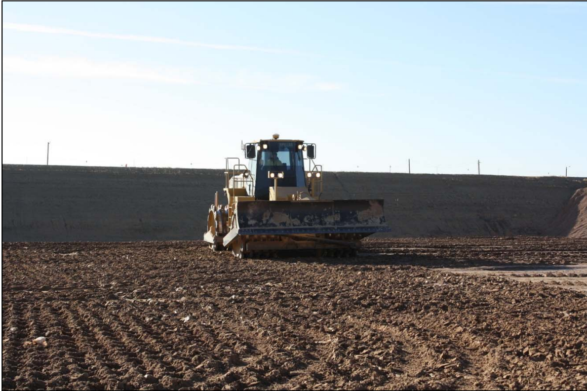
Photo 13. Compaction of Lift Area December 2017
