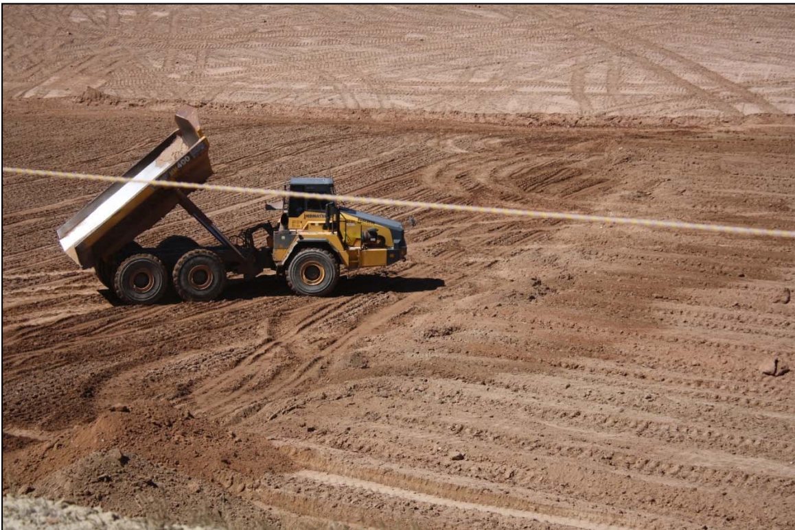
Photo 58. RRM Hauled to the Lift and Placed in Piles September 2018
