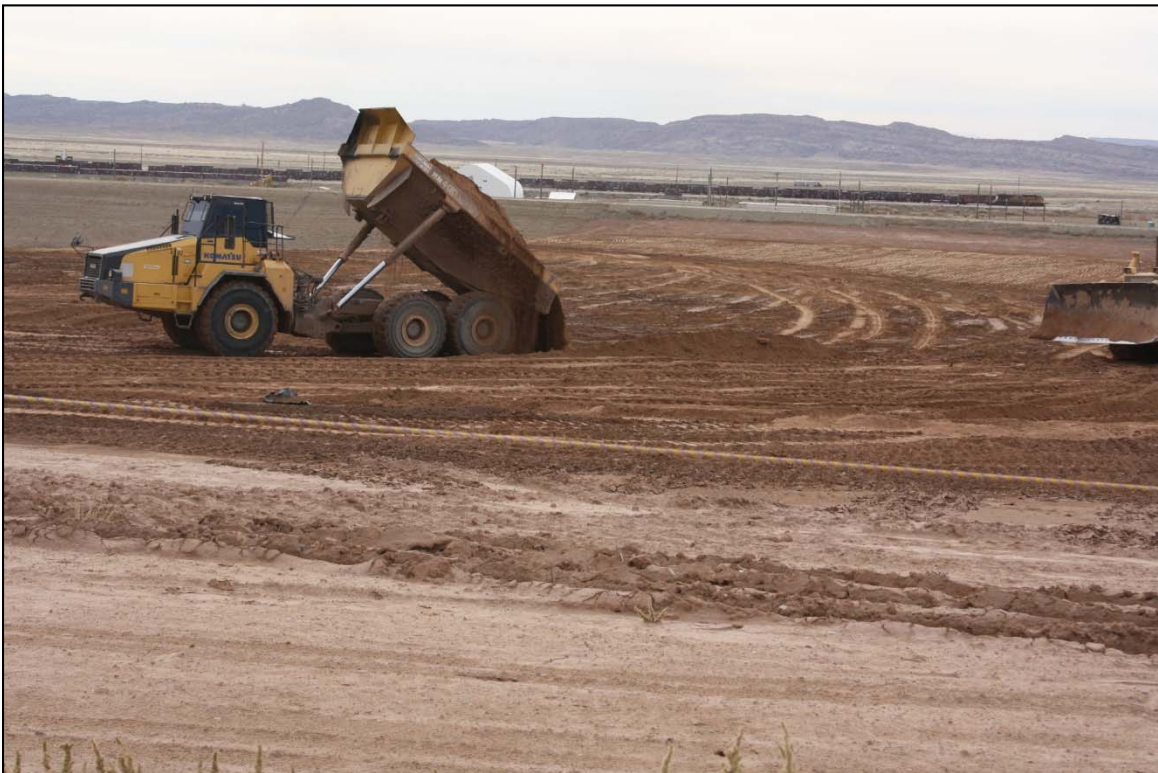
Photo 10. Haul Truck Dumping Material November 2017
