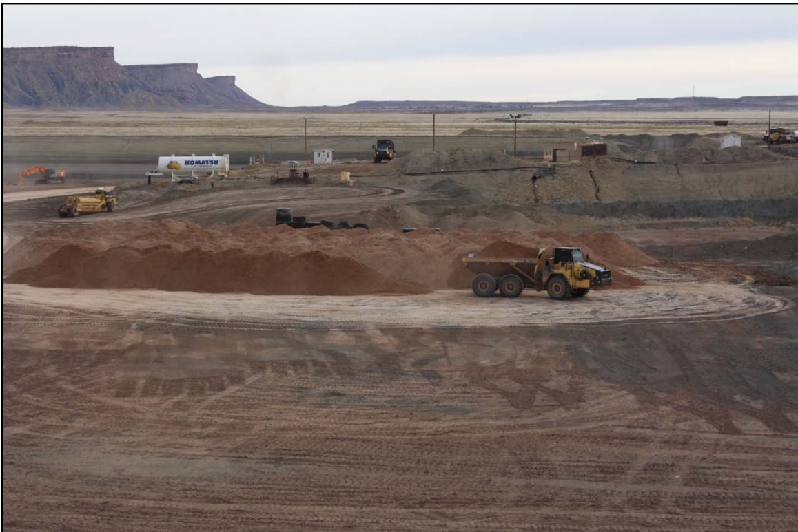
Photo 22. Stockpiled RRM February 2018
