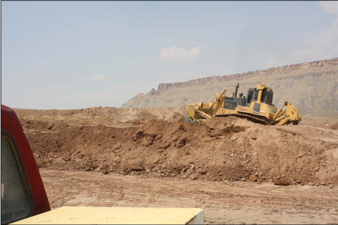
Photo 57. Dozer Working Stockpile August 2018
