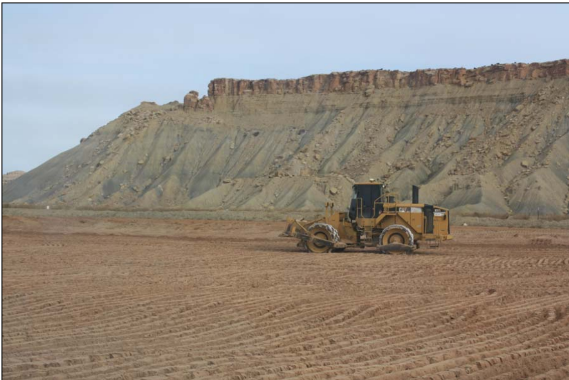
Photo 24. Sheepsfoot Scarifying Lift Area for Placement February 2018
