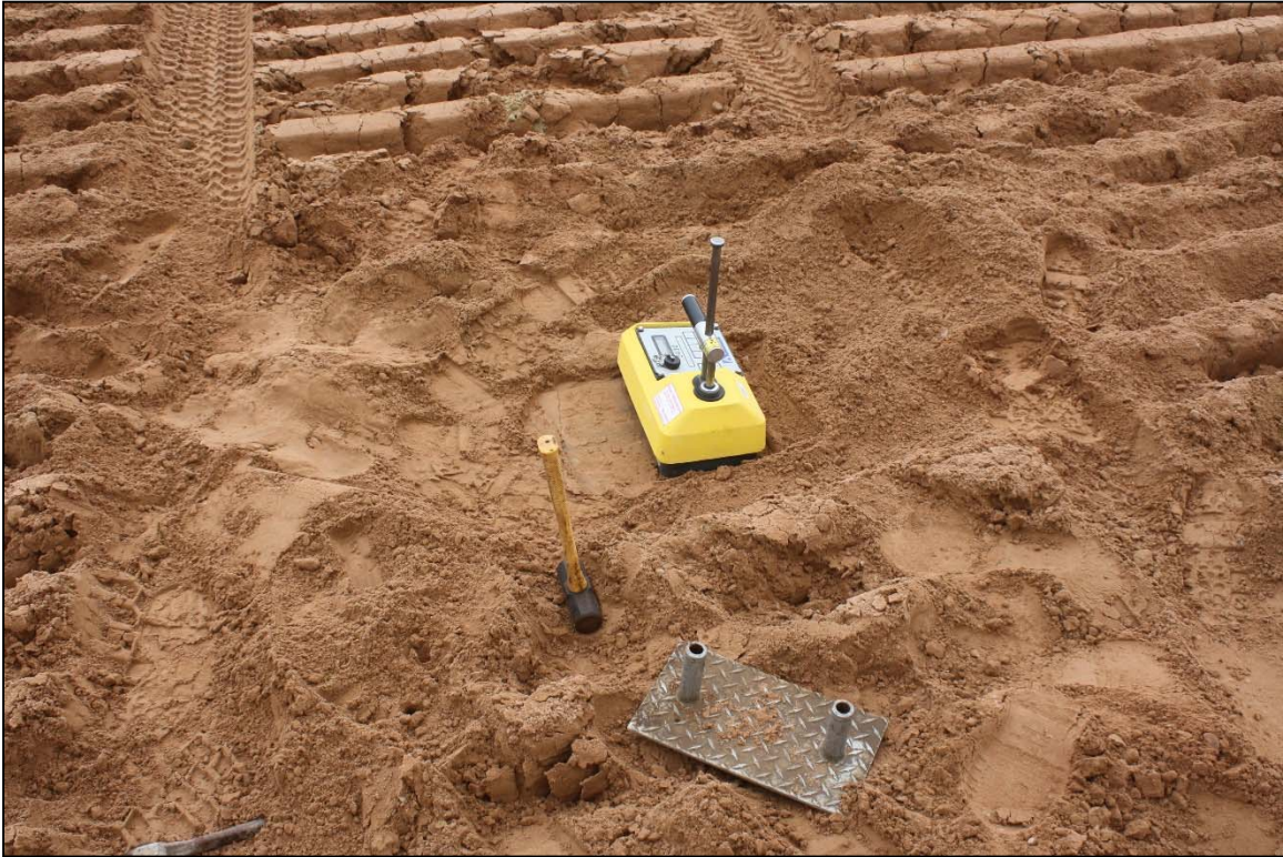
Photo 33. Moisture Density Test in Progress March 2018
