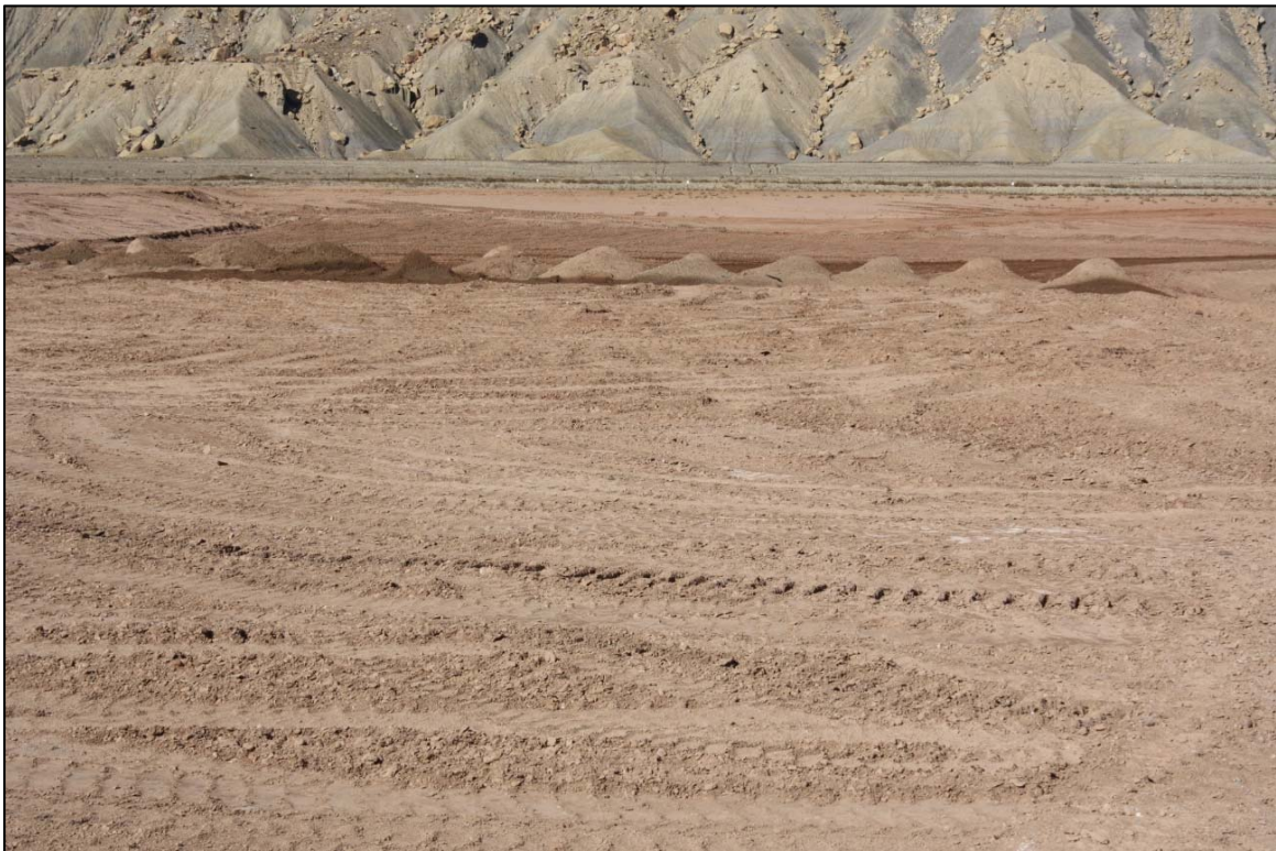
Photo 4. Piles of Tailings on Lift Area October 2017
