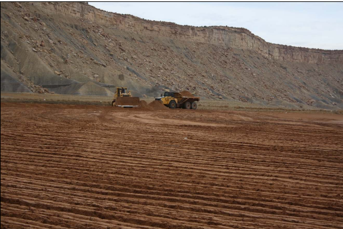
Photo 28. Dozer Placing Material on Lift Area March 2018
