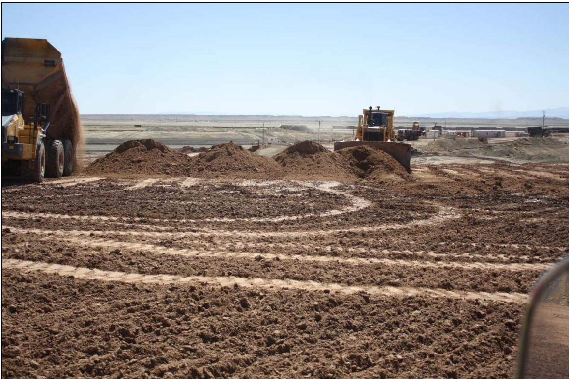
Photo 36. Dozer Placing Material on Lift April 2018
