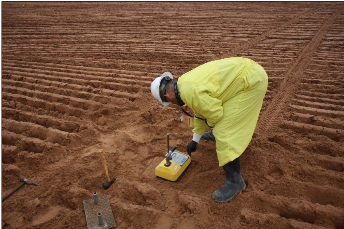
Photo 32. Moisture Density Test Start March 2018
