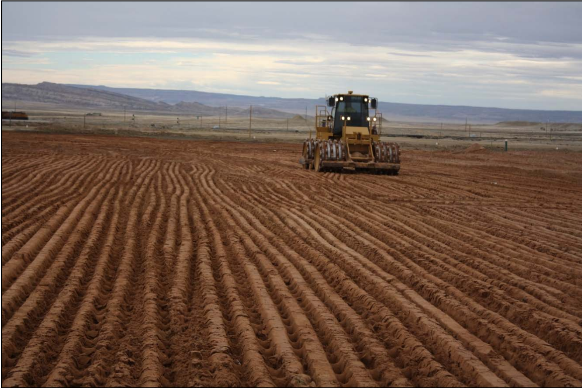
Photo 29. Compaction of Lift by Compactor March 2018
