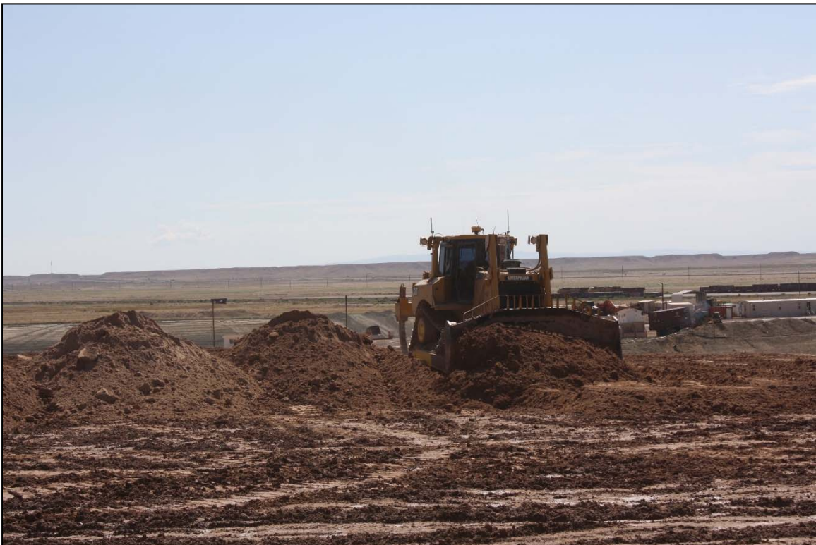
Photo 52. Placement of RRM by Dozer July 2018
