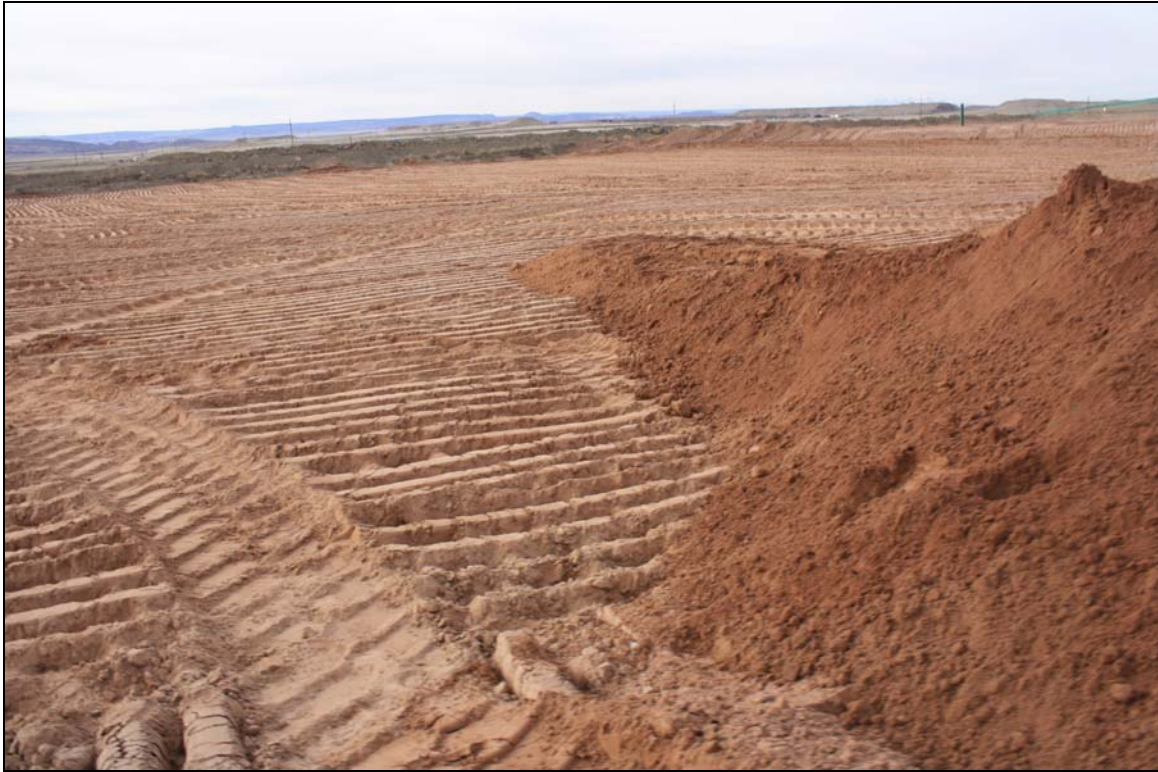
Photo 25. Underlying Lift Area Scarified for Placement February 2018
