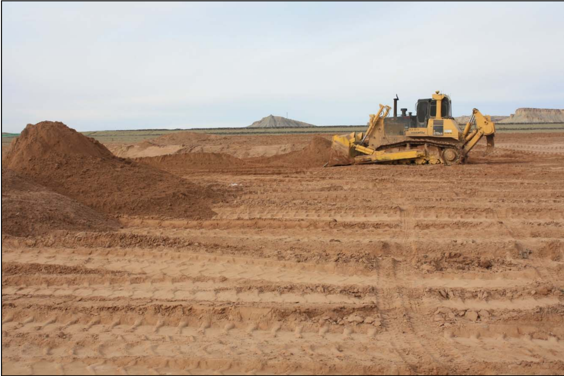
Photo 23. Bulldozer Pushing RRM for Placement February 2018
