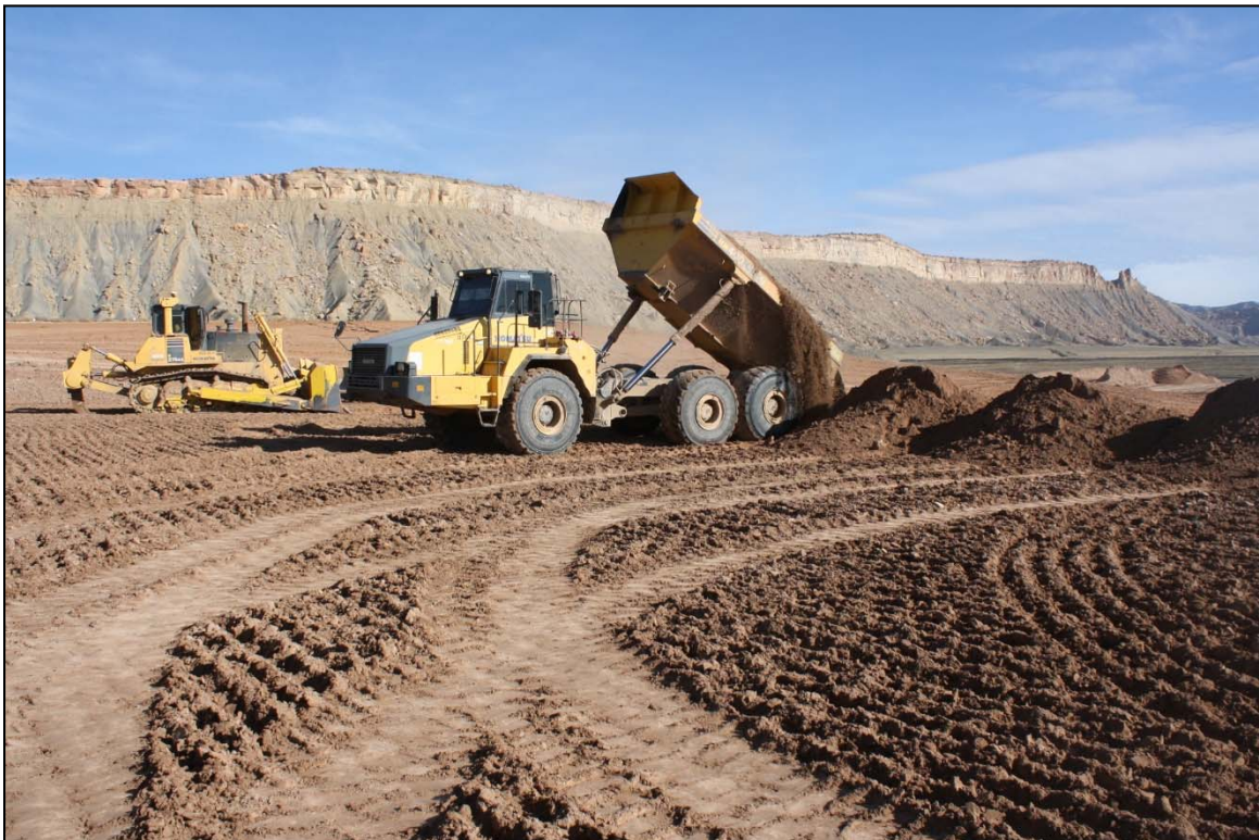
Photo 18. Truck Dumping Material on Lift Area January 2018
