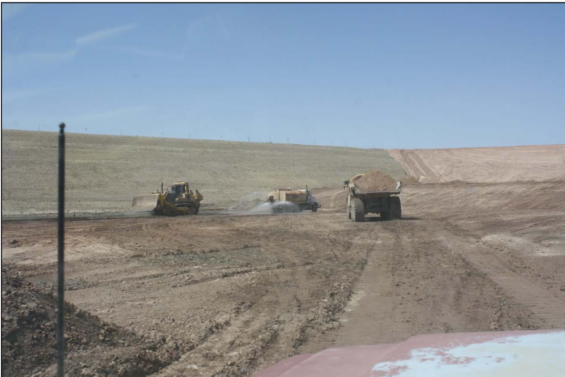
Photo 48. Prepping Cell Floor for RRM Placement June 2018
