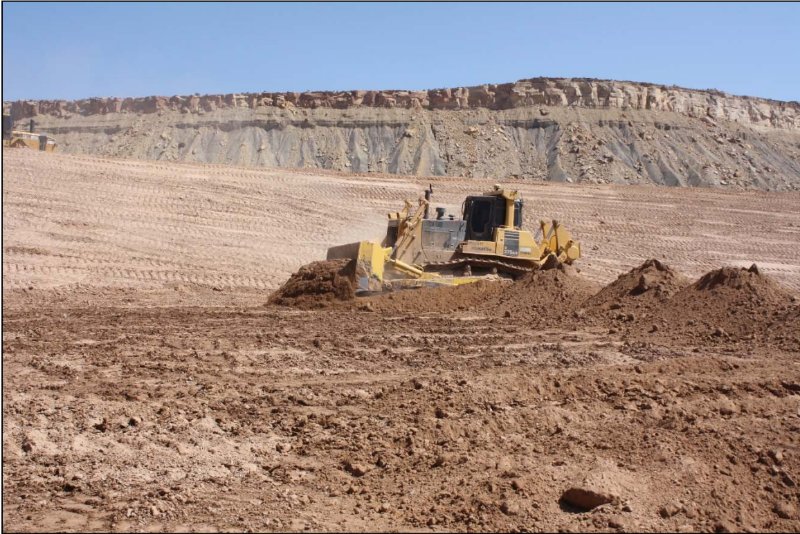
Photo 45. Dozer Placing RRM on Active Lift Area June 2018
