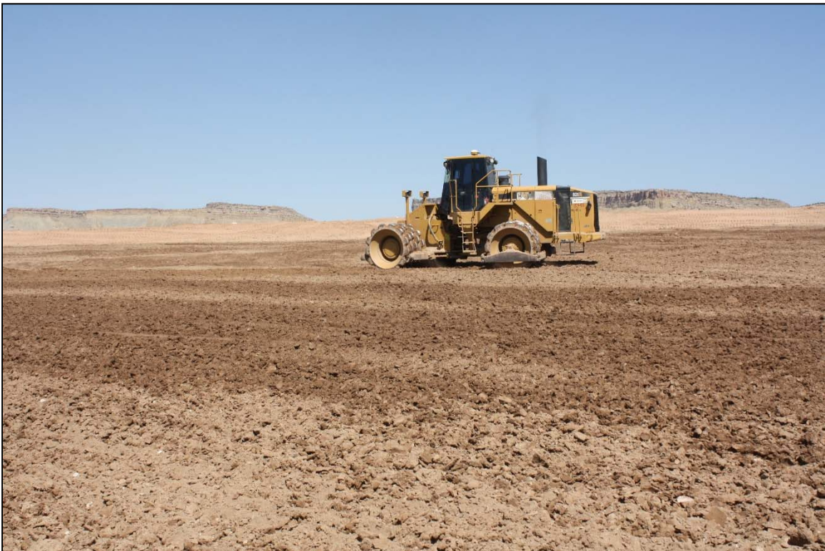
Photo 46. Compaction of Lift Area by Compactor June 2018
