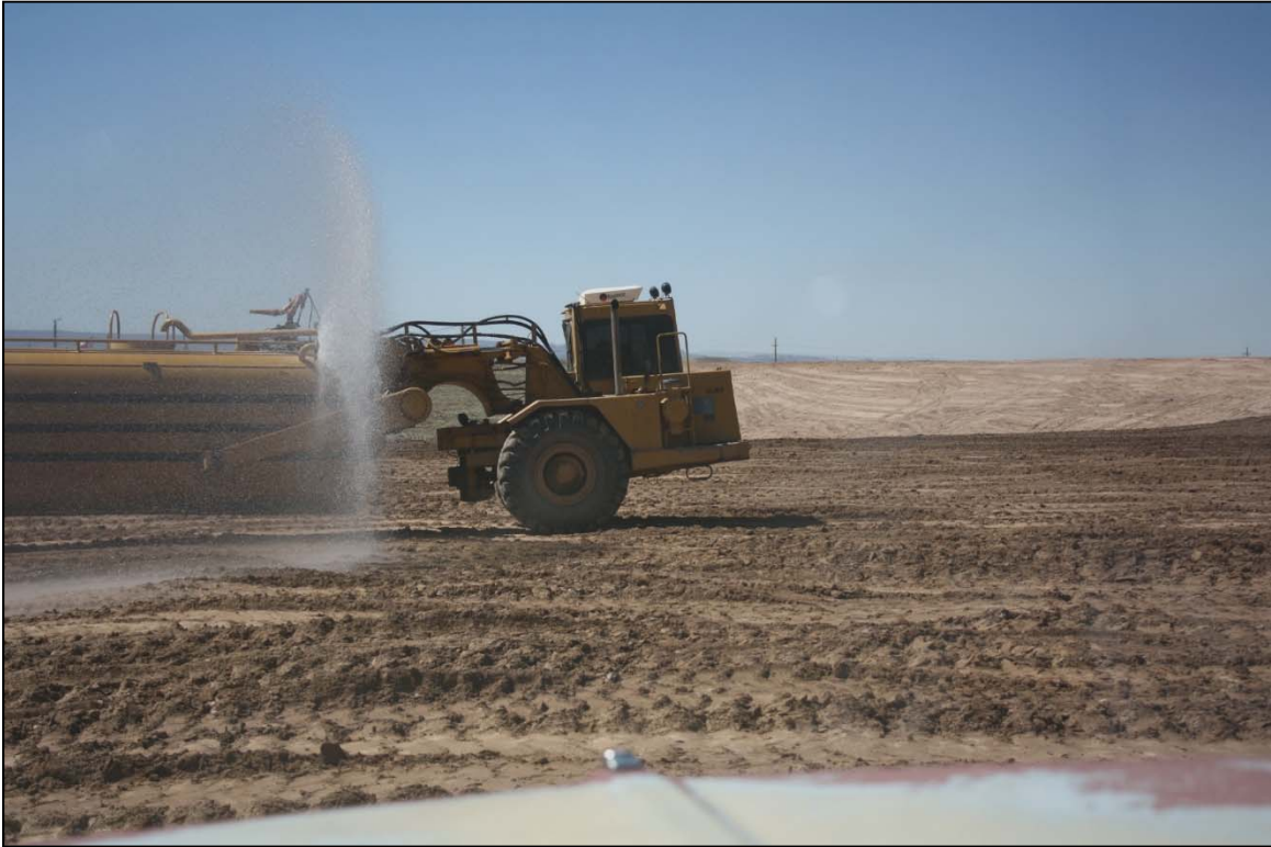
Photo 41. Watering of Lift Area May 2018
