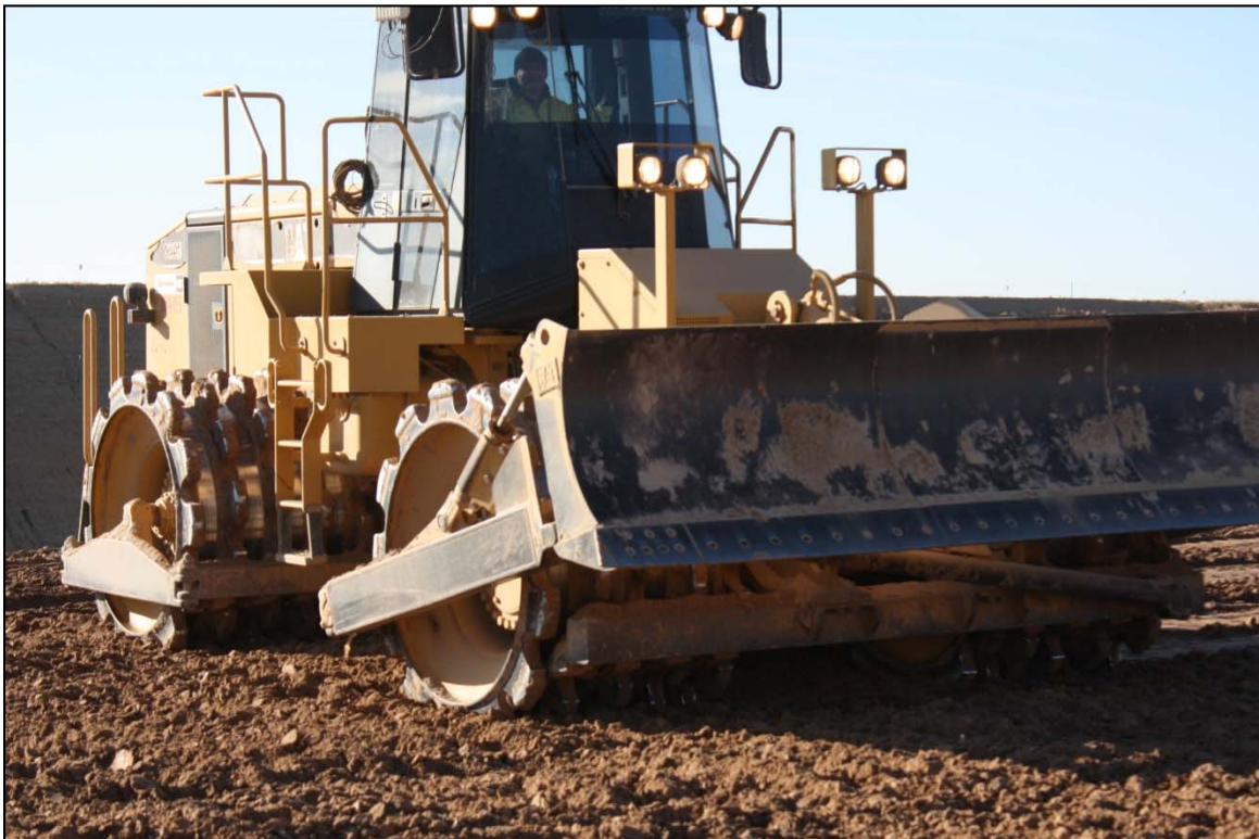
Photo 14. Compactor in Operation December 2017
