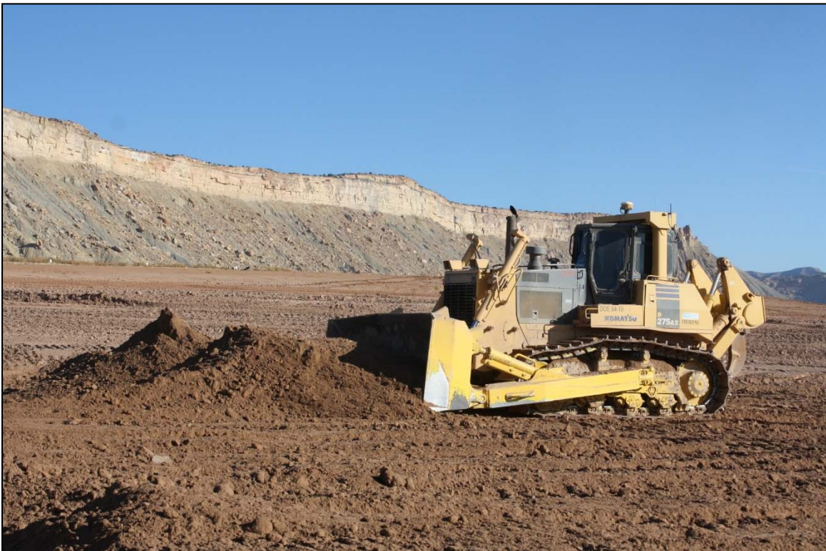
Photo 16. Dozer Placing Material December 2017
