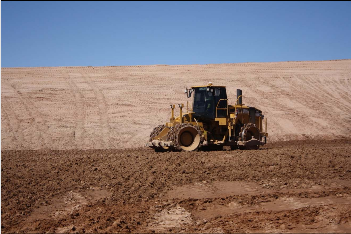
Photo 37. Compaction of Lift Area by Compactor April 2018
