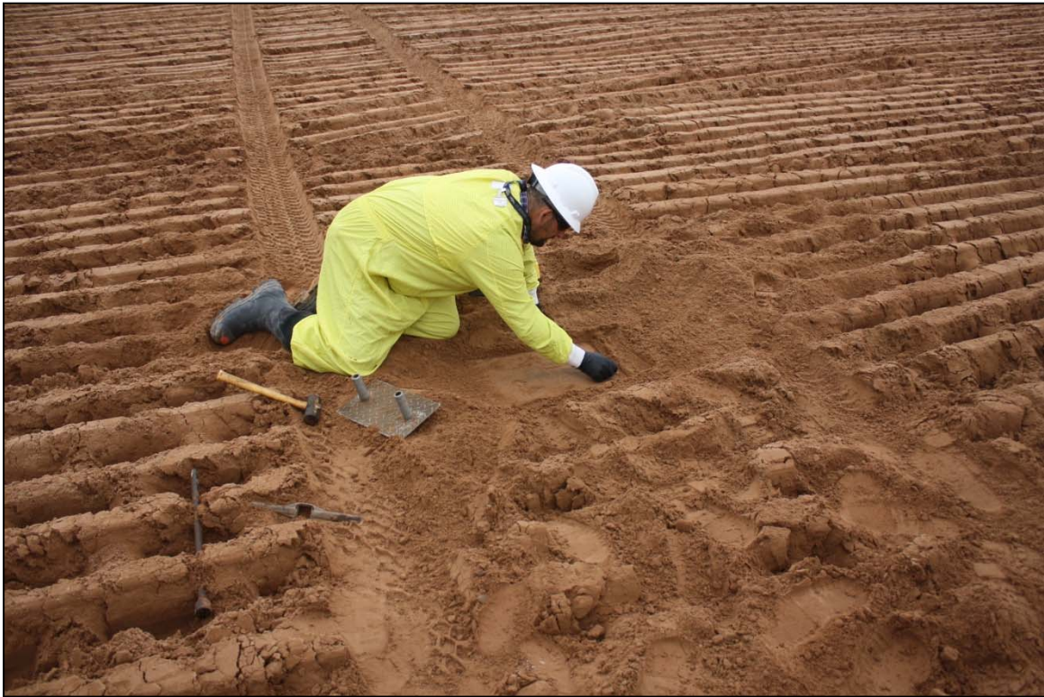
Photo 31. Moisture Density Site Preparation March 2018
