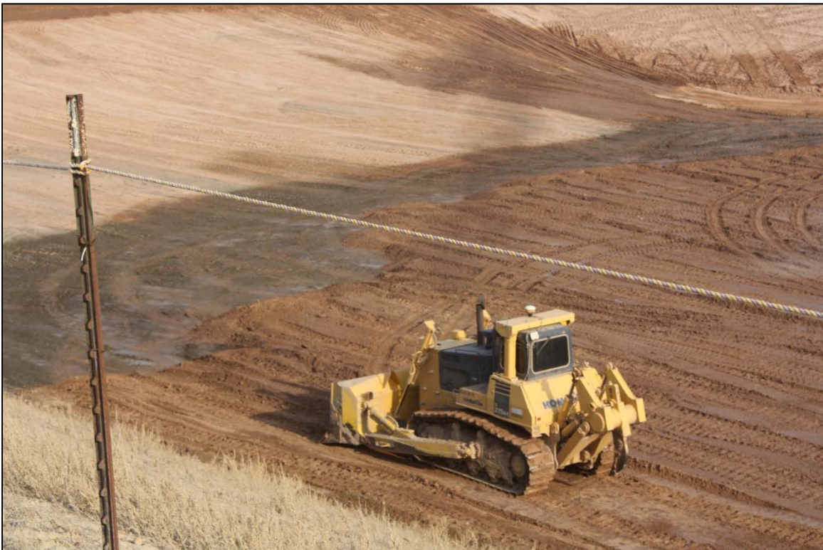
Photo 56. Dozer Placing Material on Lift Area August 2018
