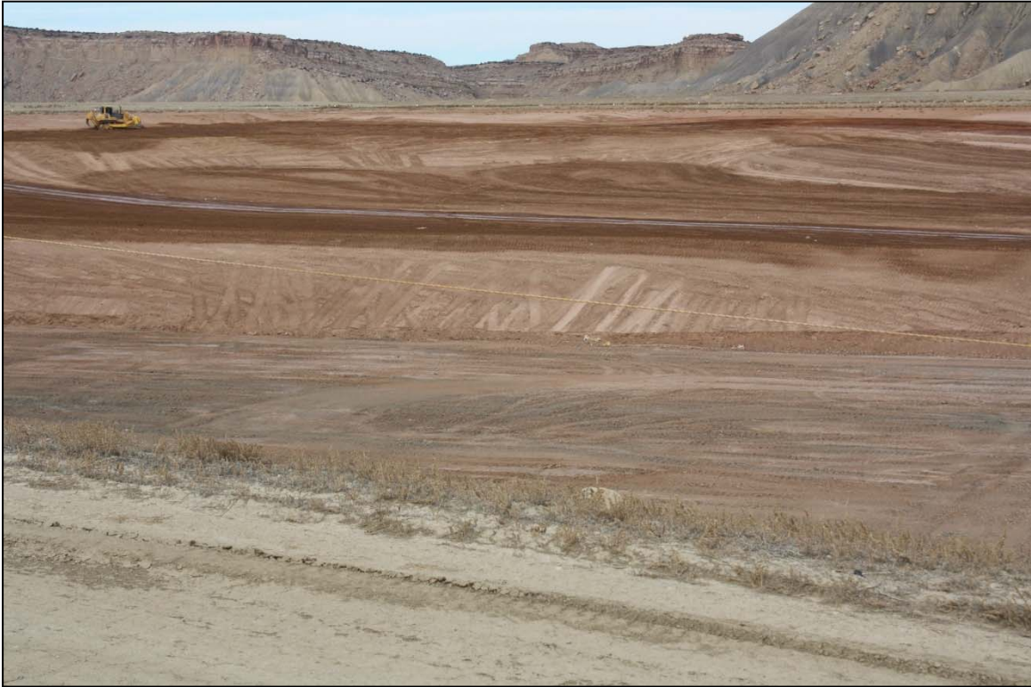
Photo 11. Moisturized Lift Prepared for Placement of Lifts November 2017
