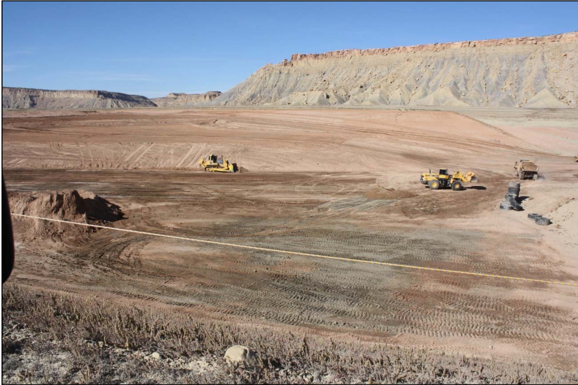
Photo 3. Multiple Disposal Cell Operations October 2017
