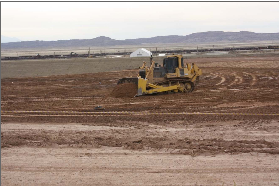
Photo 8. Dozer Placing Material November 2017
