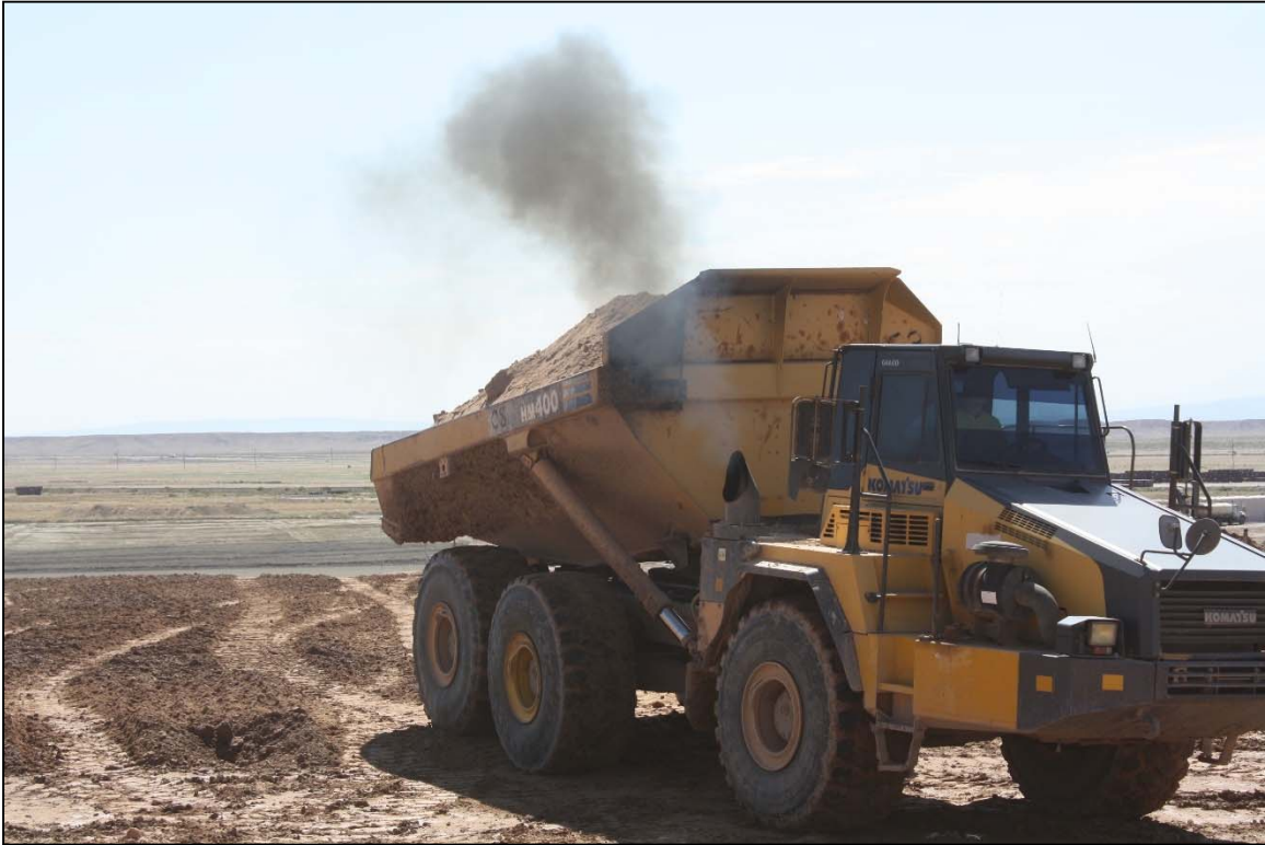
Photo 55. Haul Truck Dumping RRM in Lift Area August 2018
