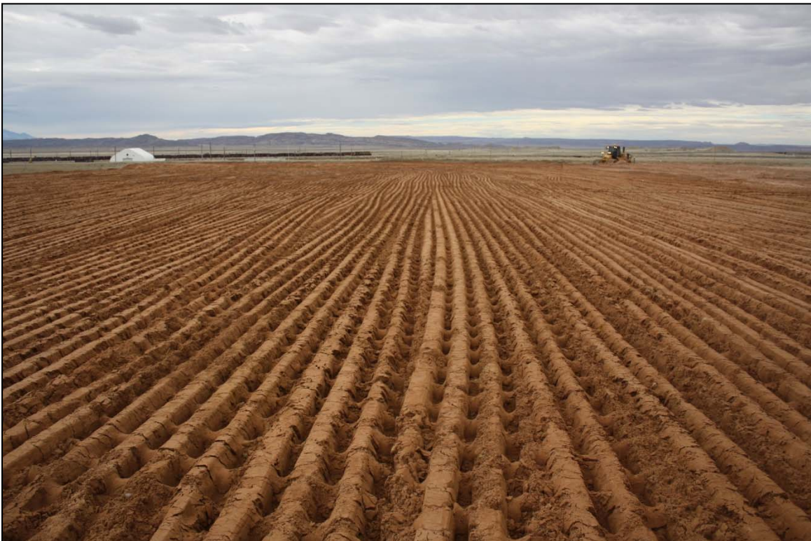
Photo 30. Scarified Lift Area March 2018
