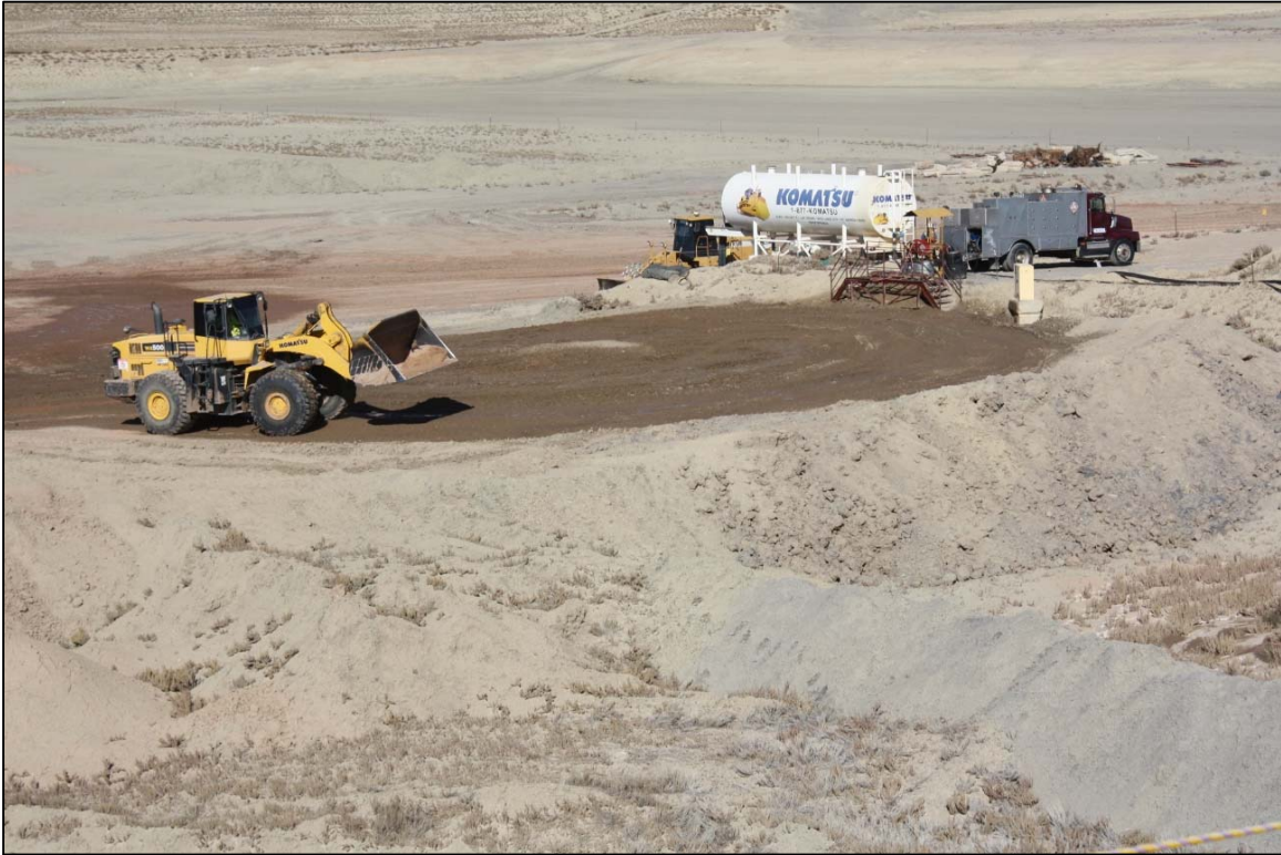
Photo 1. Loader Approaching Fuel Island October 2017
