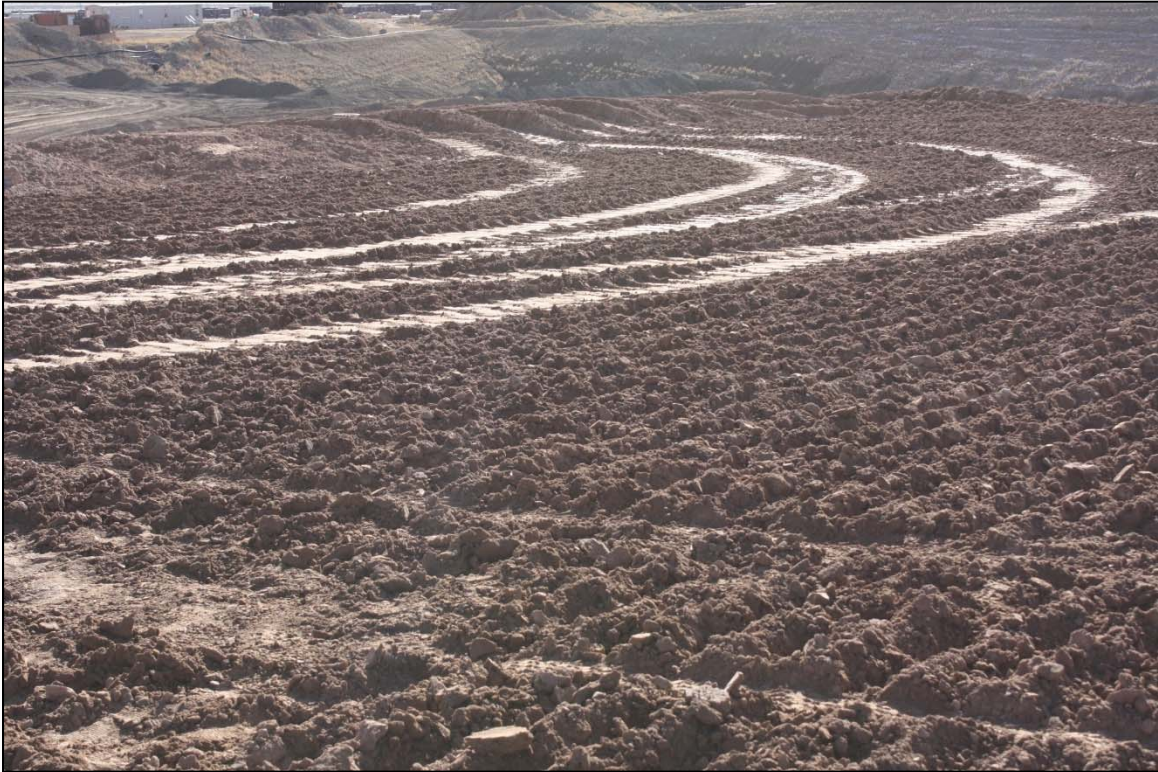
Photo 21. Compaction of Lift Area January 2018
