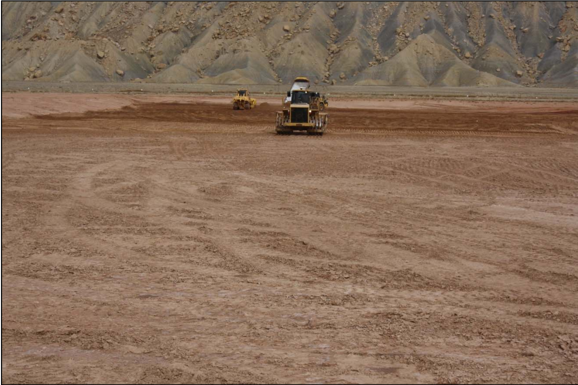
Photo 7. Compaction of Lift Area November 2017
