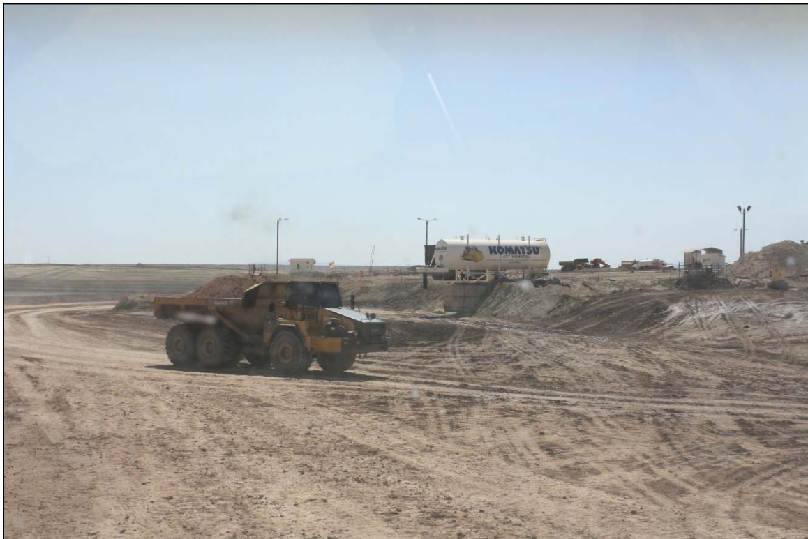
Photo42. Haul Truck on Haul Road to Disposal Cell June 2018
