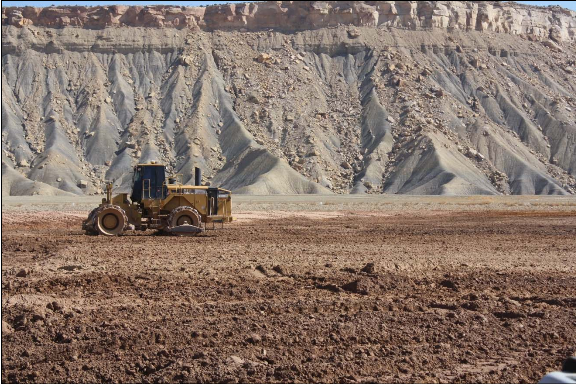
Photo 53. Compactor Compacting Material on a Lift July 2018
