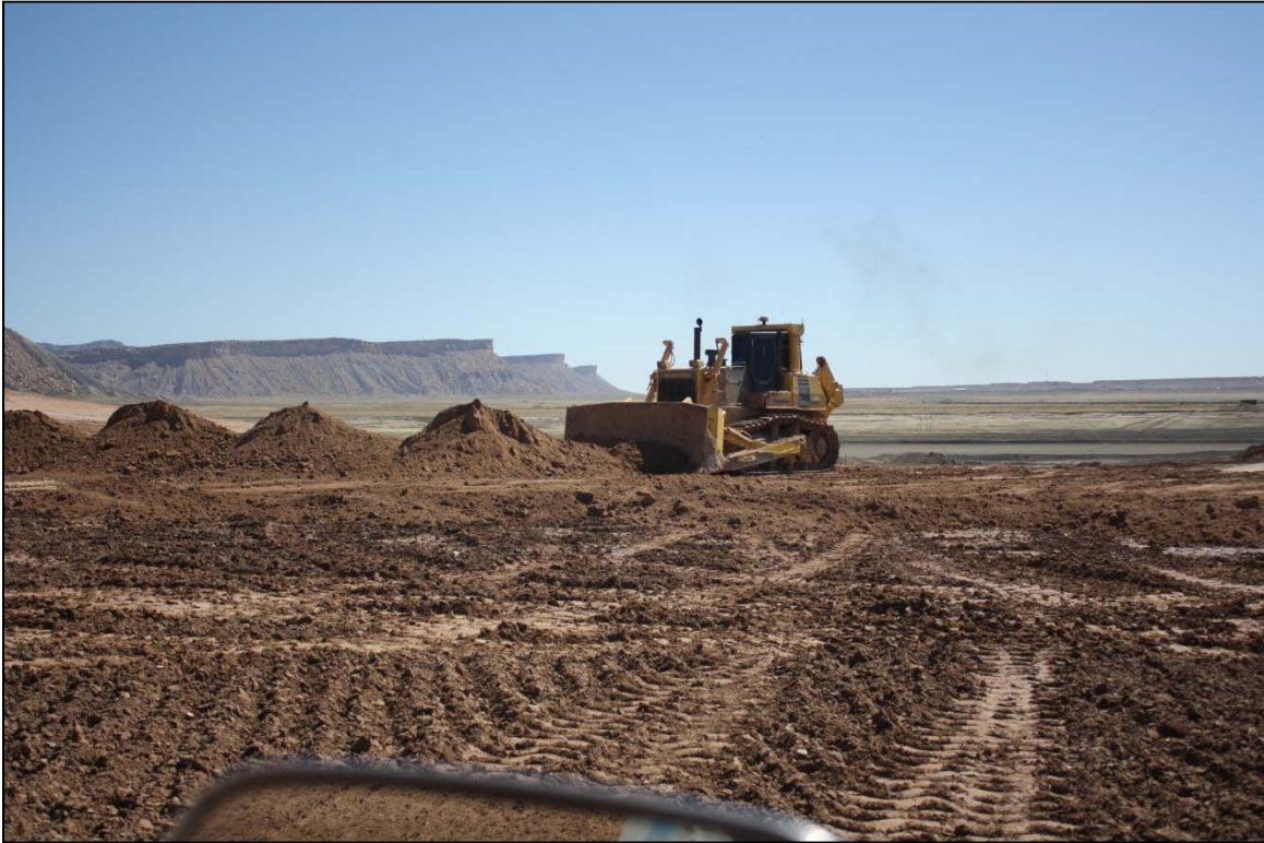
Photo 39. Dozer Placing RRM May 2018
