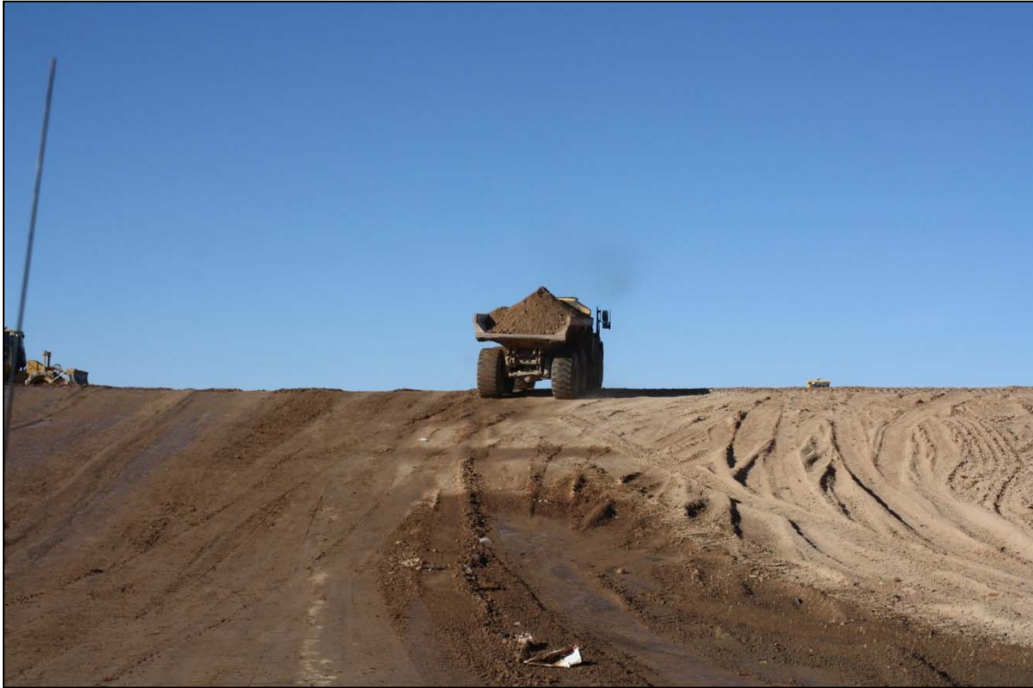
Photo 17. Haul Truck Hauling RRM to Lift Area December 2017
