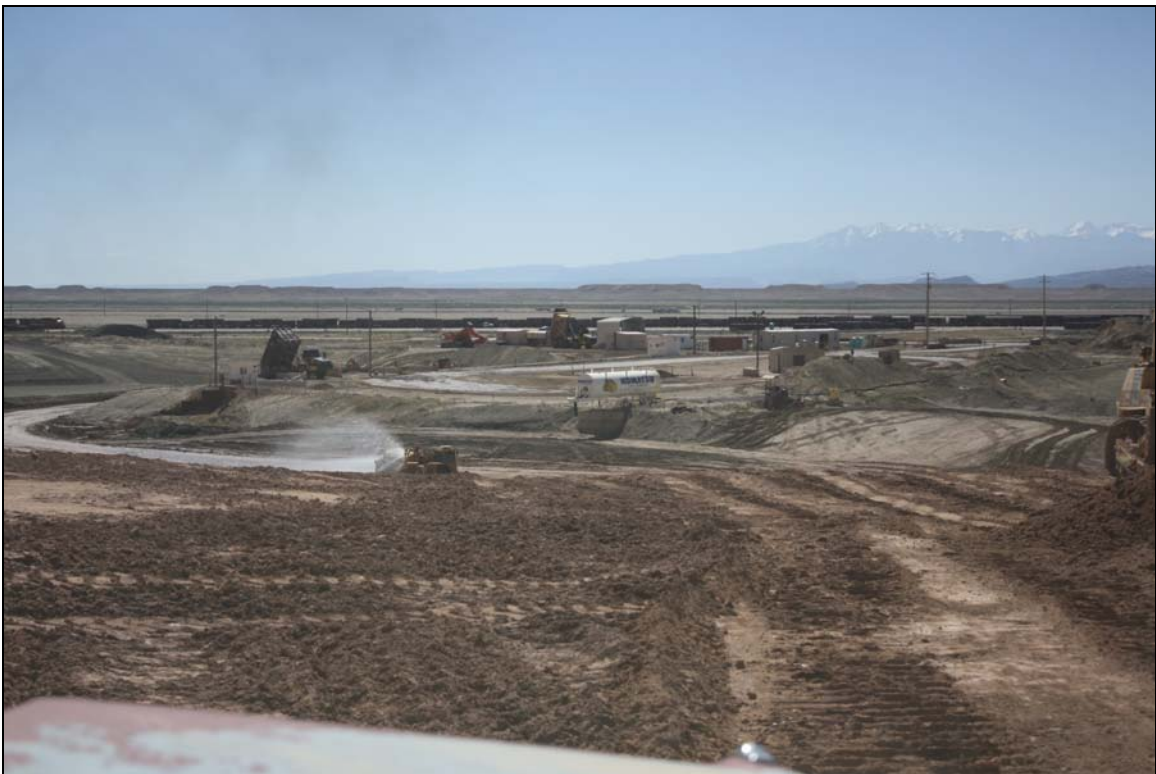
Photo 34. Water Wagon Watering Haul Routes April 2018
