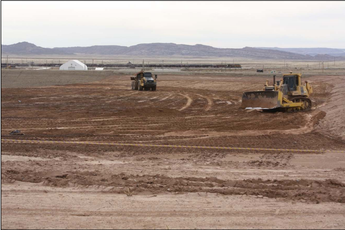
Photo 9. Haul Truck Approaching with Load November 2017
