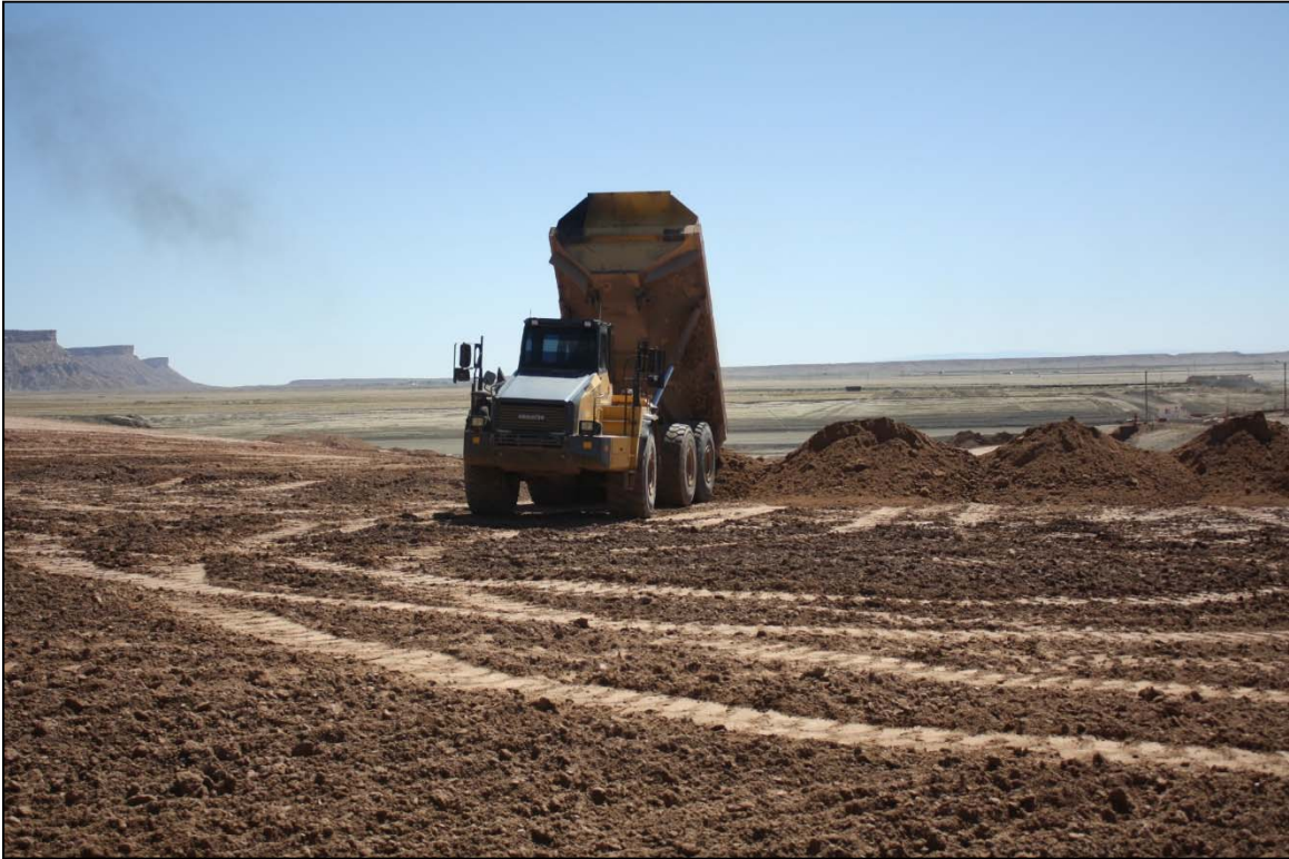
Photo 35. Haul Truck Placing Load on Lift April 2018
