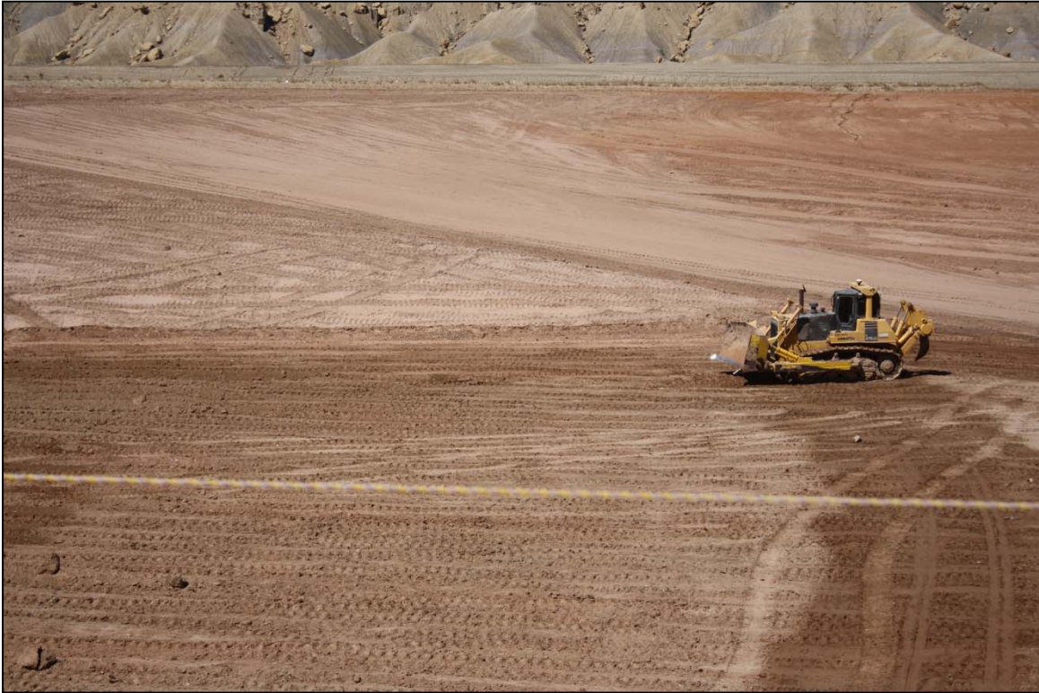
Photo 59. Dozer Placing RRM in Lift Area September 2018
