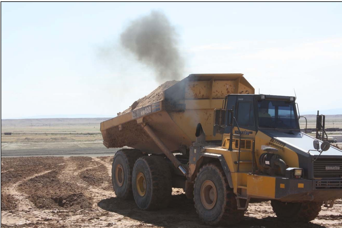
Photo 50. Haul Truck Preparing to Dump Material on Lift Area July 2018
