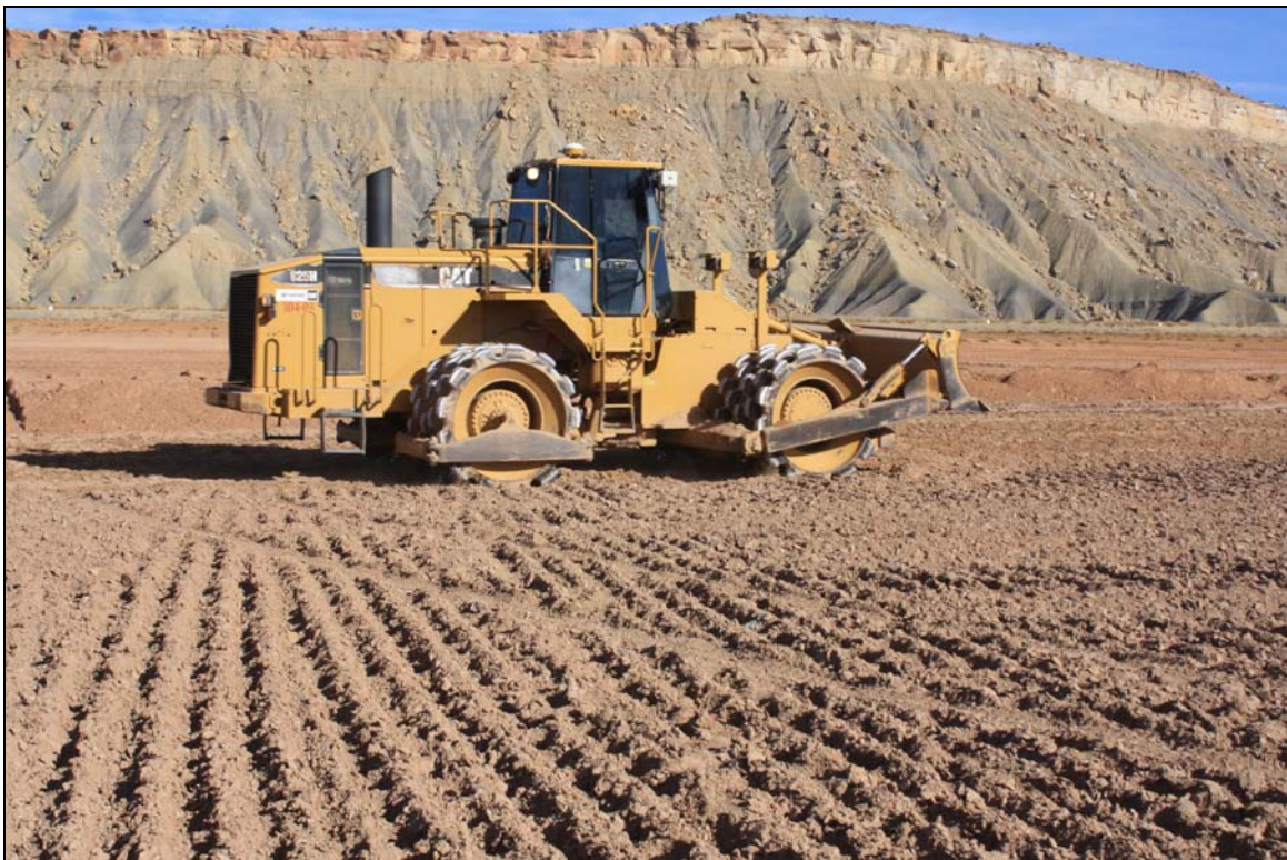
Photo 20. Scarified Lift Area January 2018
