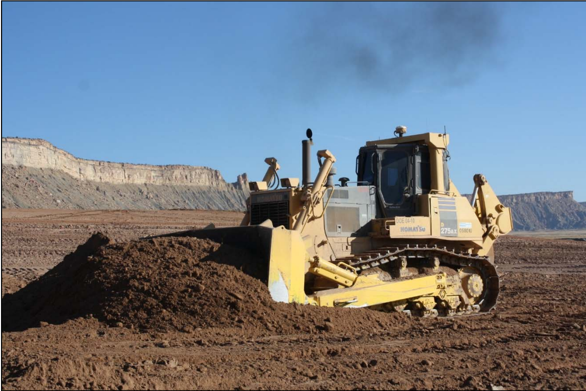
Photo 15. Dozer Pushing Material December 2017
