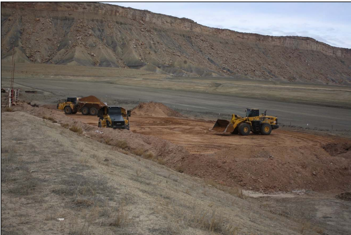
Photo 26. CA Loading Area at Dump Ramp March 2018
