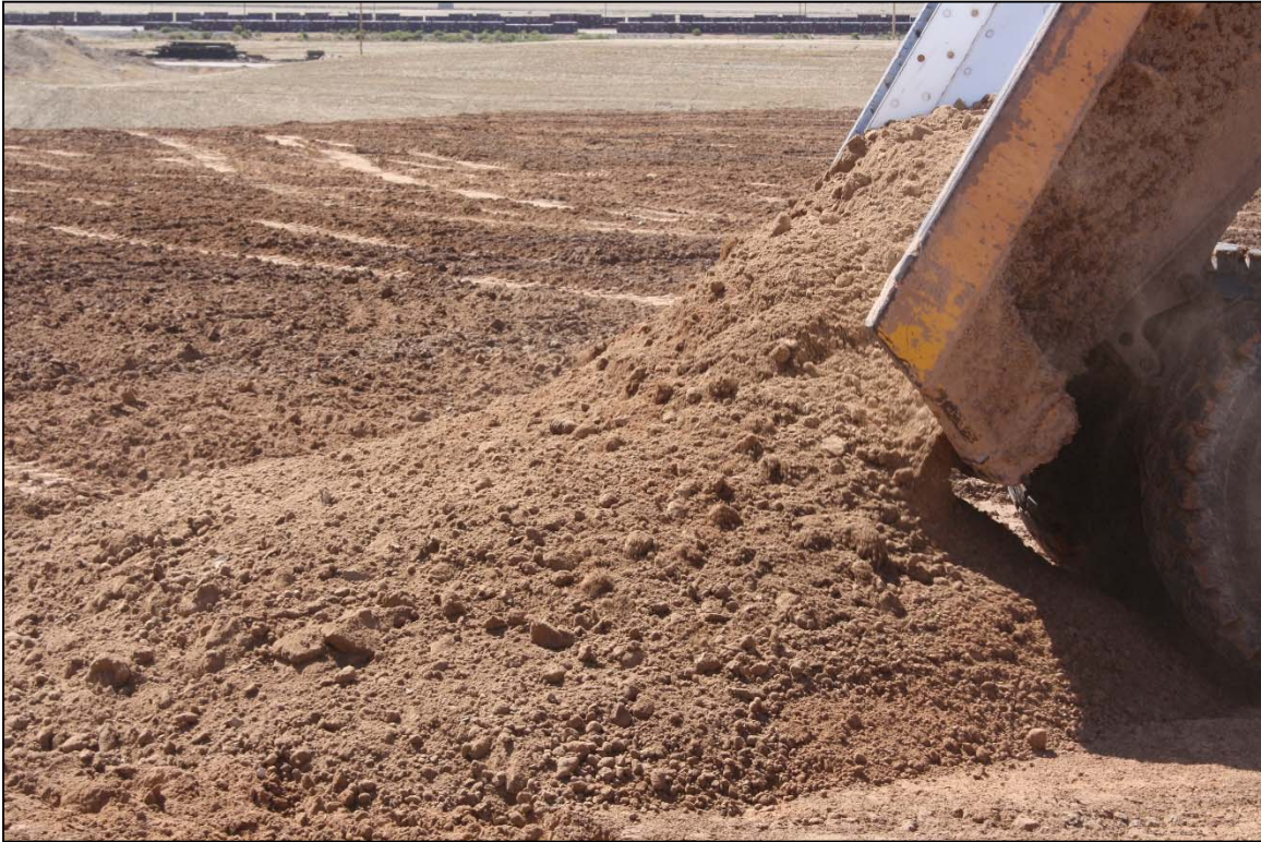
Photo 51. RRM Pile Placed on Lift Area July 2018
