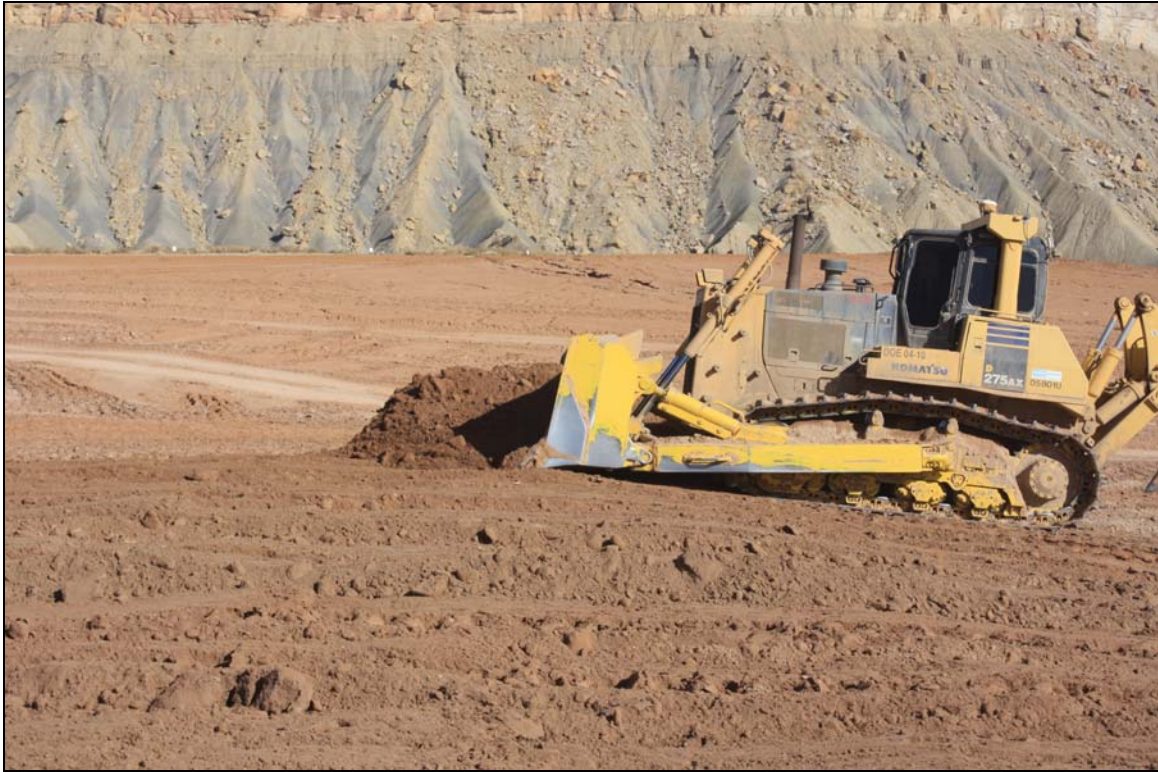
Photo 19. Dozer Placing Material January 2018
