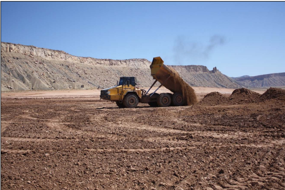
Photo 38. Placement of Material on Lift Area by Haul Truck May 2018
