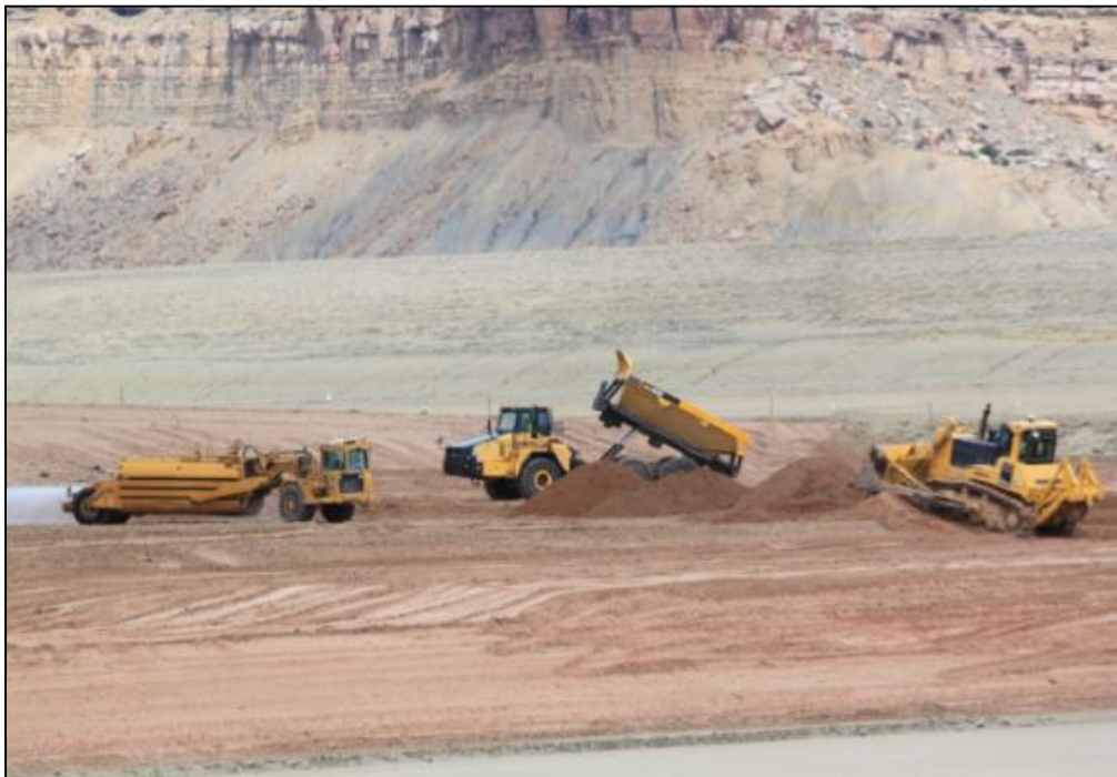
Photo 8. RRM Placement May 2013
