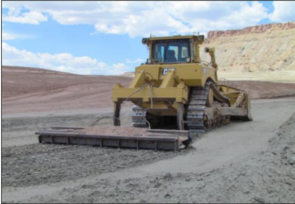
Photo 9. Conditioning RRM June 2013
