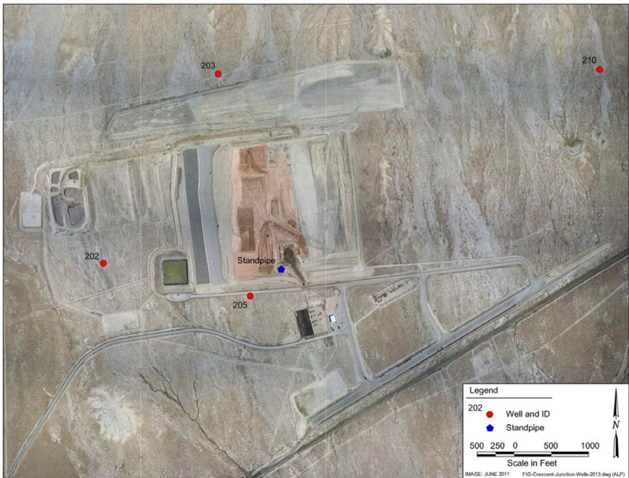
Figure 5. Locations of Monitoring Wells and Standpipe
