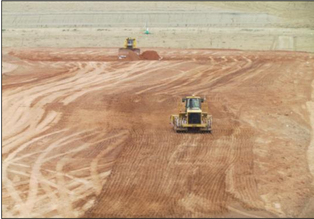
Photo 7. RRM Compaction May 2013
