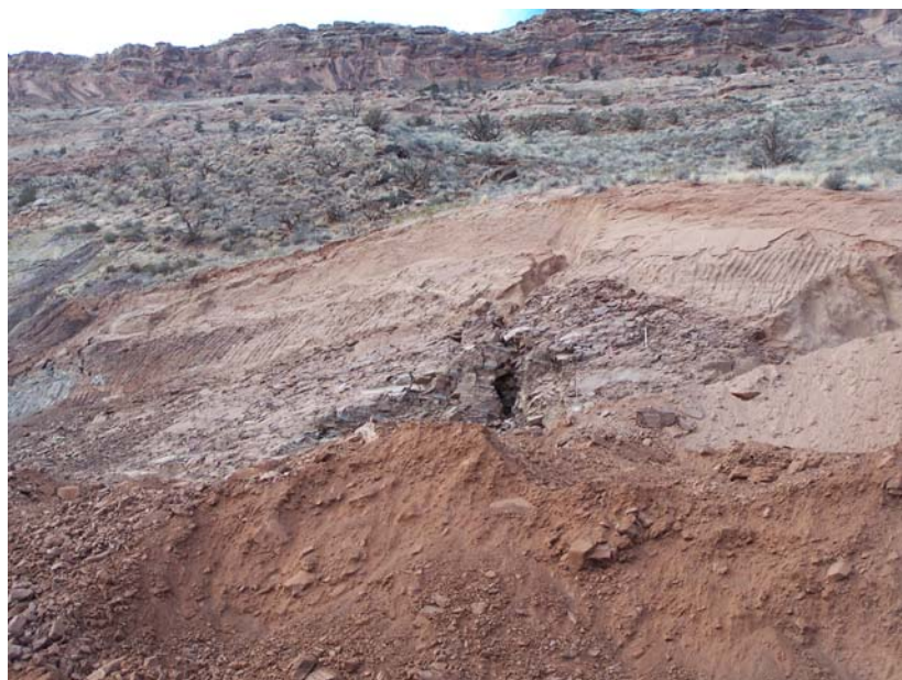
Photo 21. Hillslope One Day After February 2009 Slide
