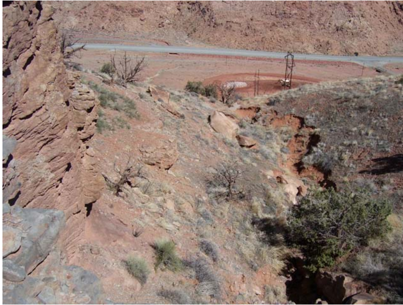
Photo 17. Looking Downslope at Drainage 3
