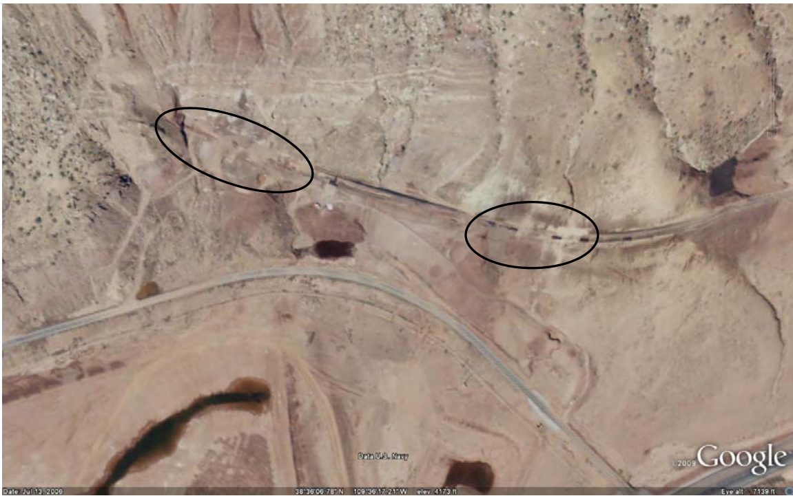
Photo 27. Rail Damage from July 2006 Flash Flood
