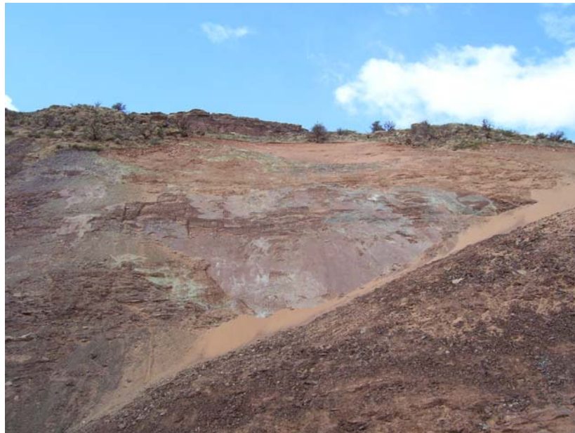
Photo 22. Hillslope Slide Area After Cleaning of Slumped Material
