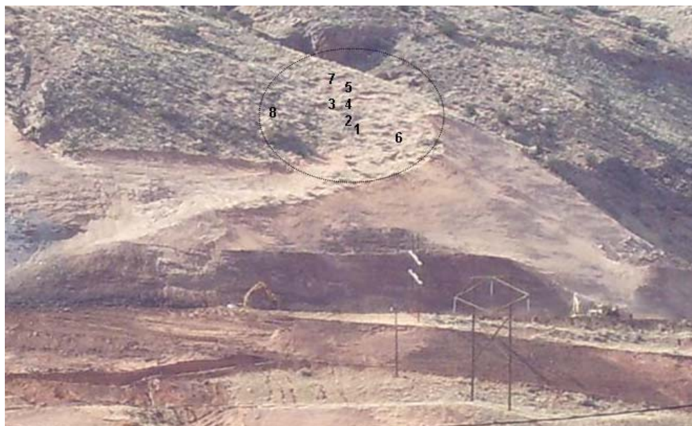
Photo 23. Staked Locations Monitored on Hillside
