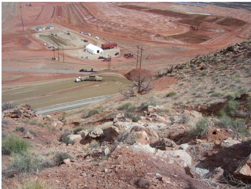
Photo 14. Drainage 2 Looking Downslope at Bedrock Above Excavation
