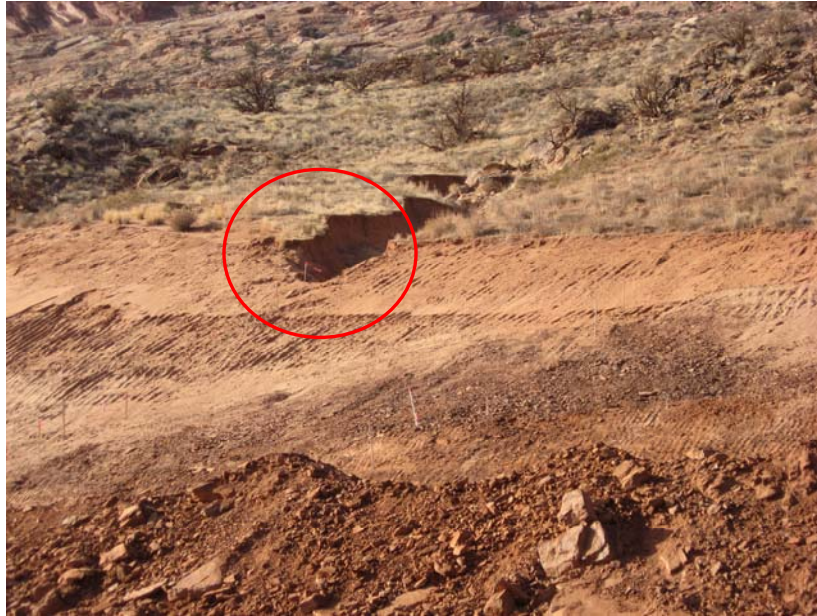
Photo 28. Hillside Excavation Showing Junction of Drainage Channel and Excavated Face
