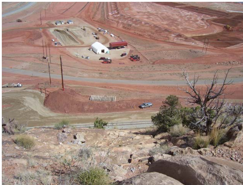
Photo 12. Looking Downslope from Drainage 1
