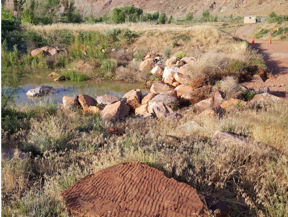
Photo B-1. River Water Backing Up into Lower Reach of Moab Wash
