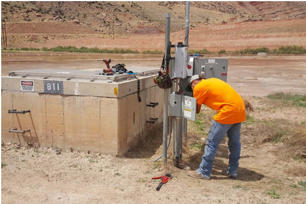
Photo C-4. Replacing Electrical Components on Well 0811
