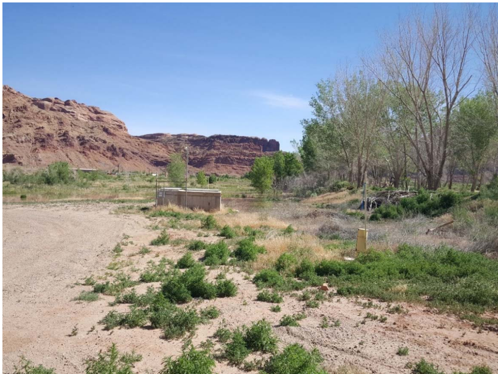
Photo B-14. Well 0813 Vault
