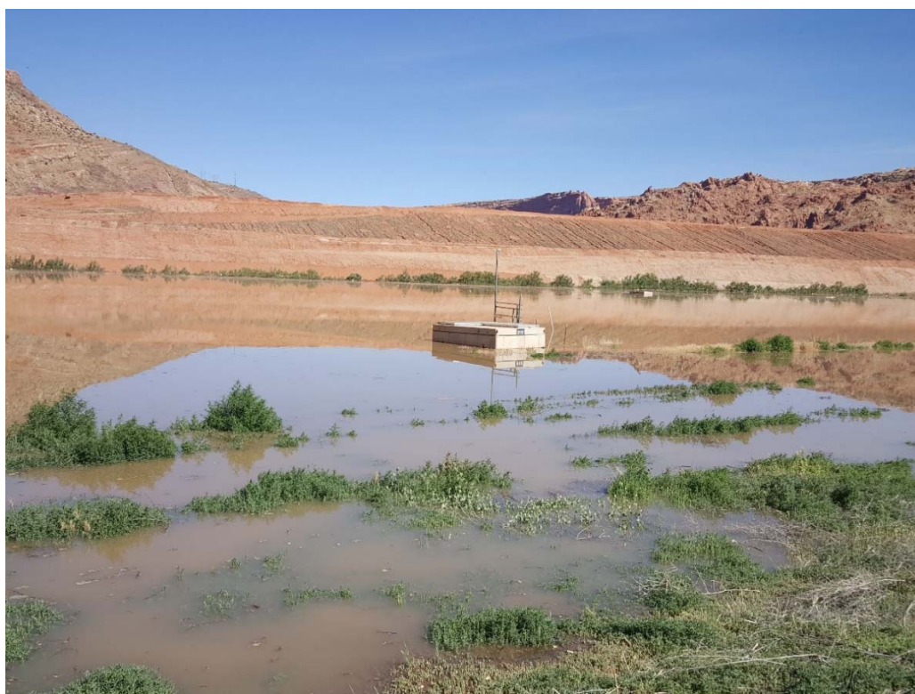
Photo B-12. Well 0810 Vault
