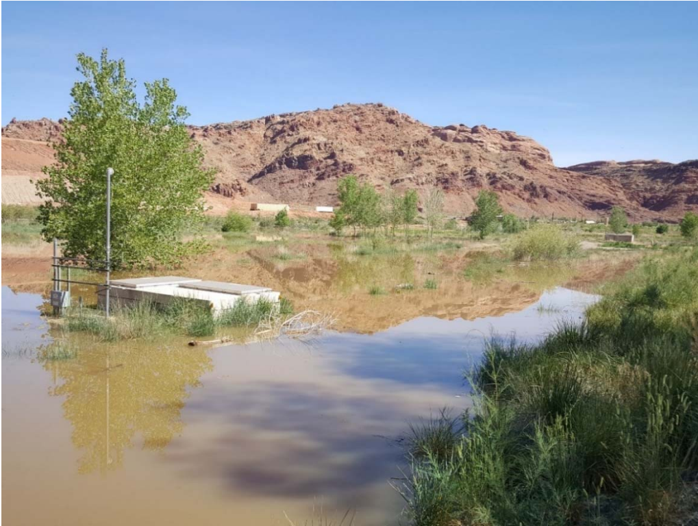
Photo B-13. Well 0812 Vault
