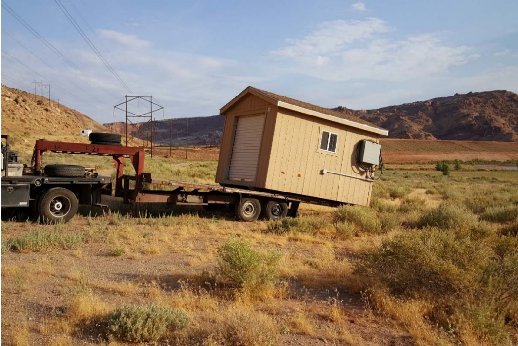
Photo C-3. Moving Pump House from Near Hwy 279 Gate
