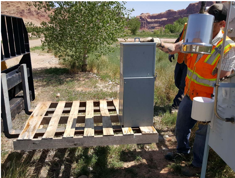
Photo B-4. Moving Well Field Power Center
