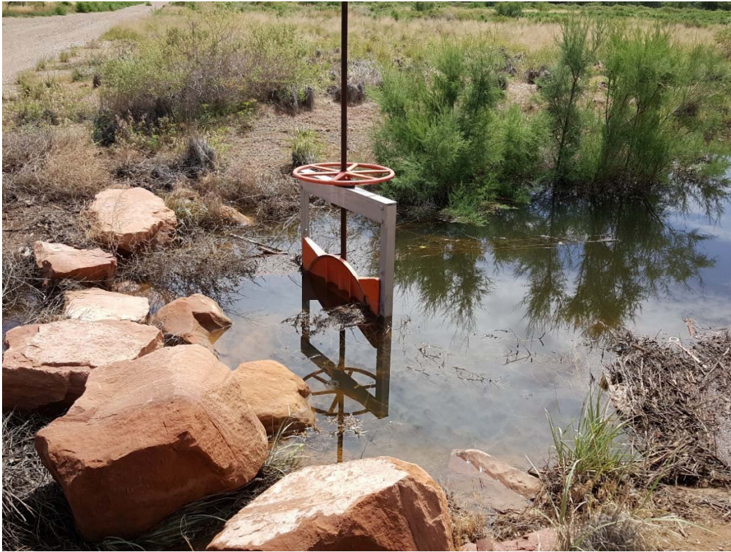
Photo B-21. Drainage Channel through South Off-pile Area
