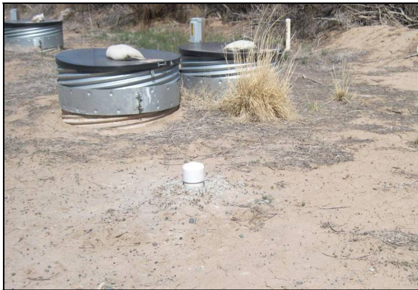
CF2 Remediation Well 0650
