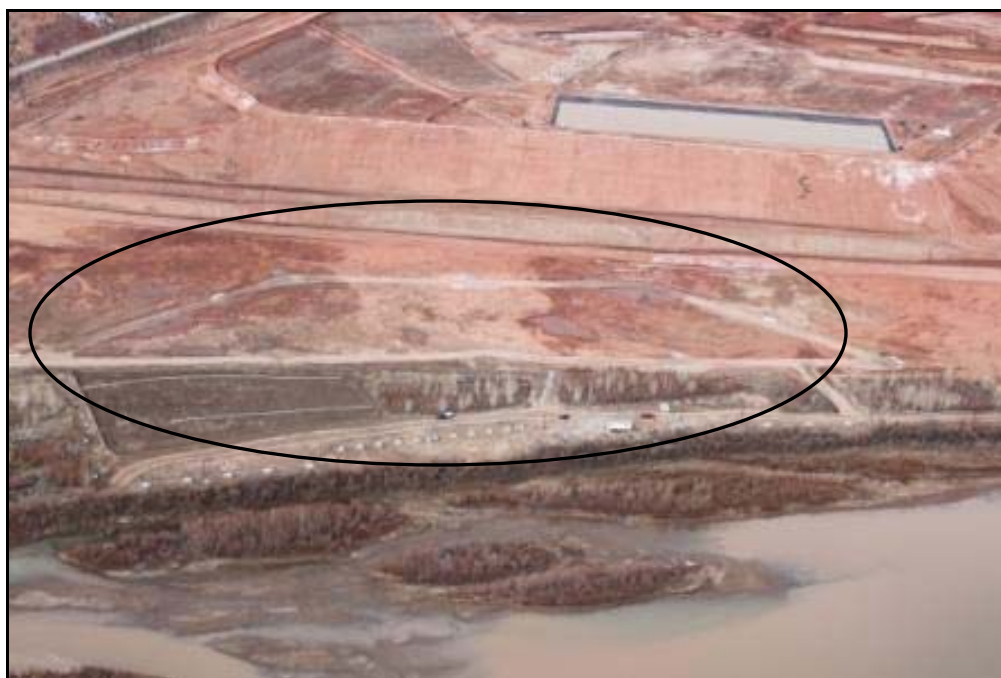
Photo 2. Location of Newly Remediated Off-pile Area Where CF5 Wells Were Installed
