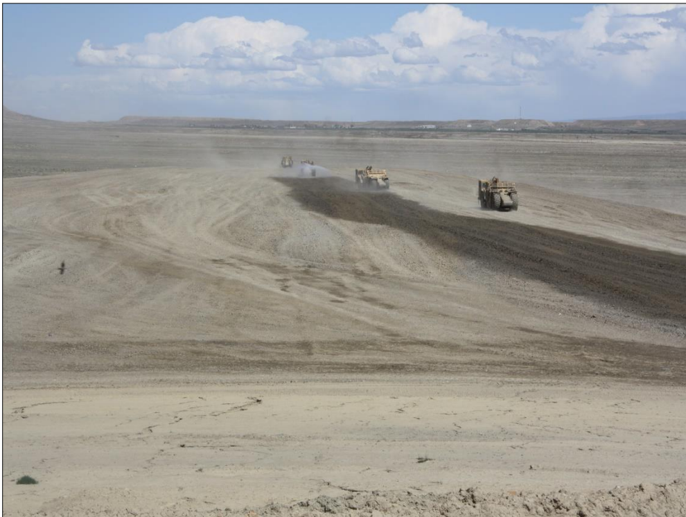
Photo 30. Spoils Embankment Placement April 20, 2017
