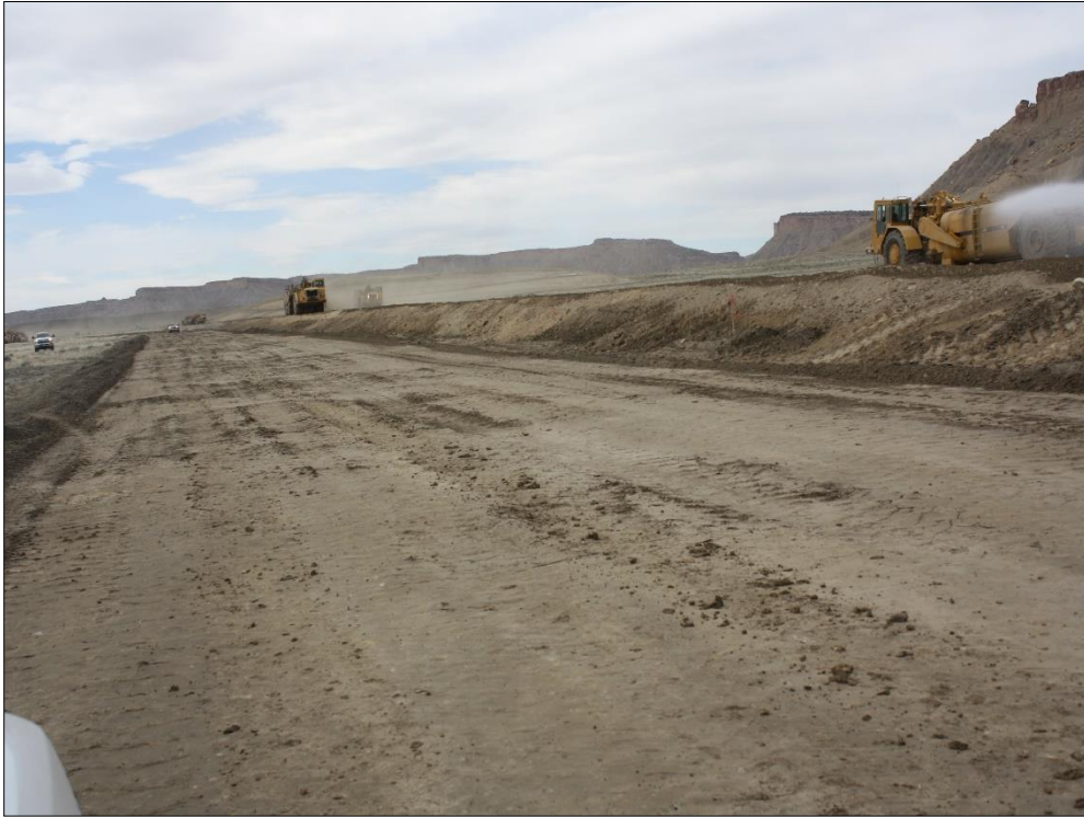
Photo 29. Spoils Embankment Placement March 21, 2017
