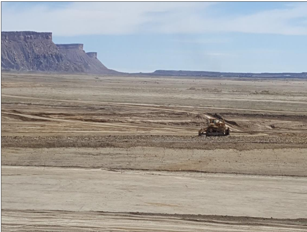
Photo 4. Phase 3b Cell Excavation April 7, 2017
