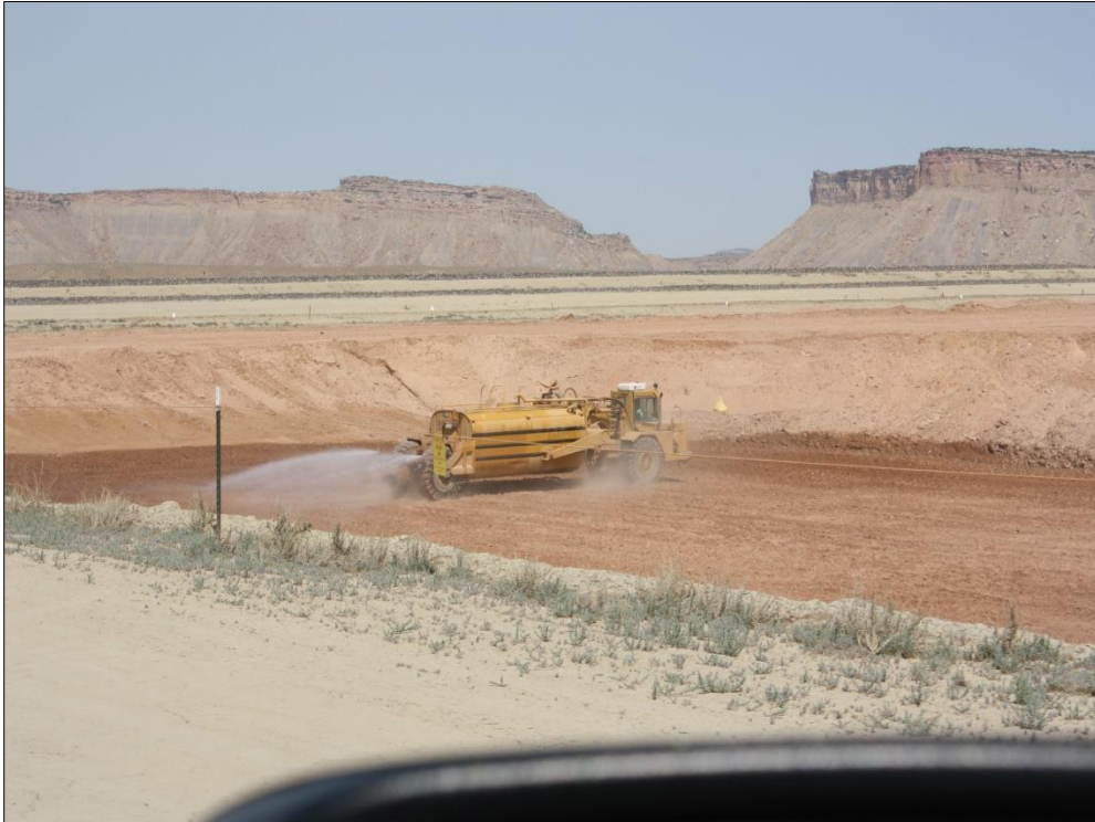
Photo 21. RRM Moisture Conditioning June 27, 2017
