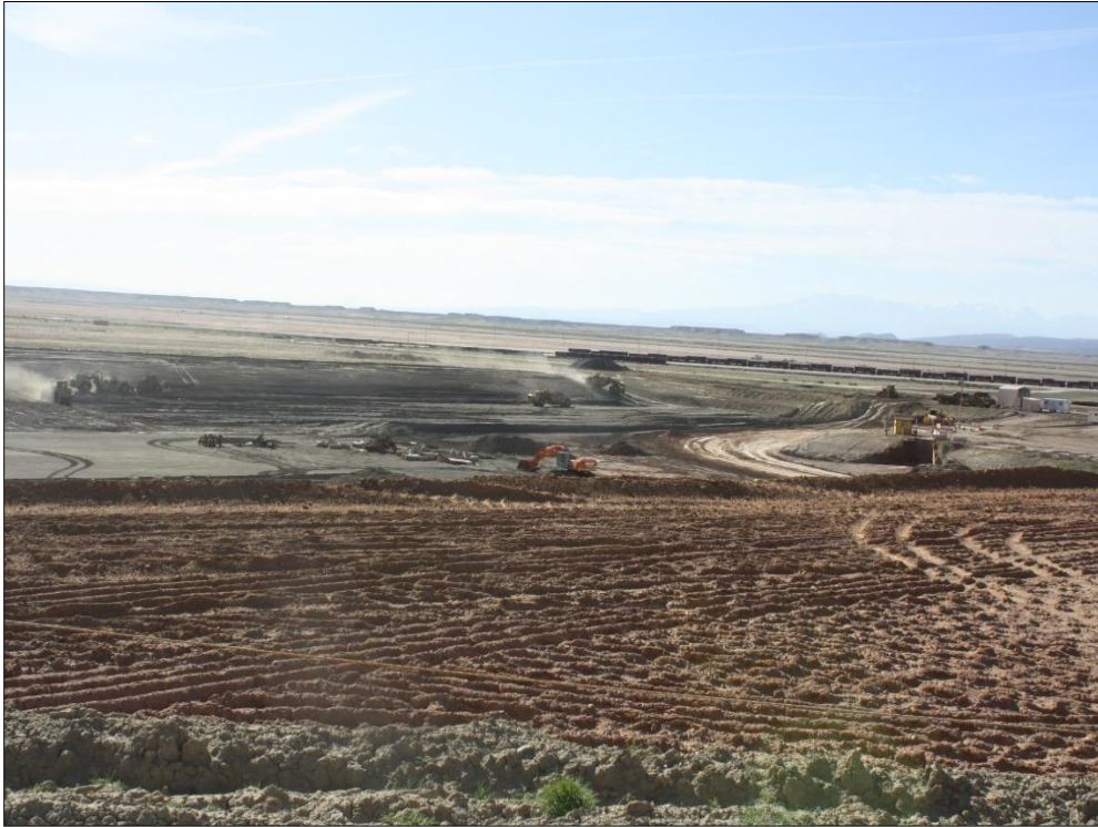
Photo 7. Phase 3b Cell Excavation May 15, 2017
