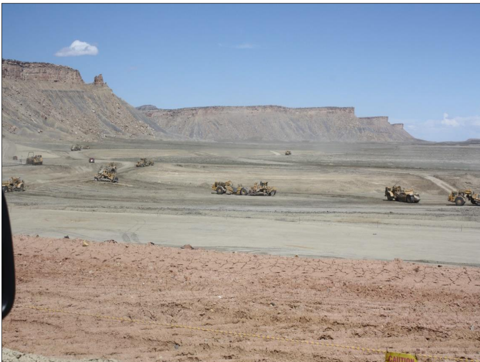
Photo 6. Phase 3b Cell Excavation April 20, 2017
