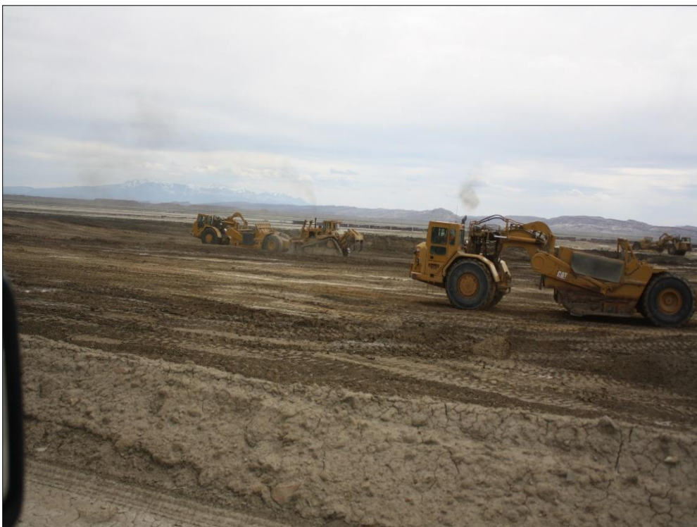
Photo 2. Phase 3b Cell Excavation March 21, 2017
