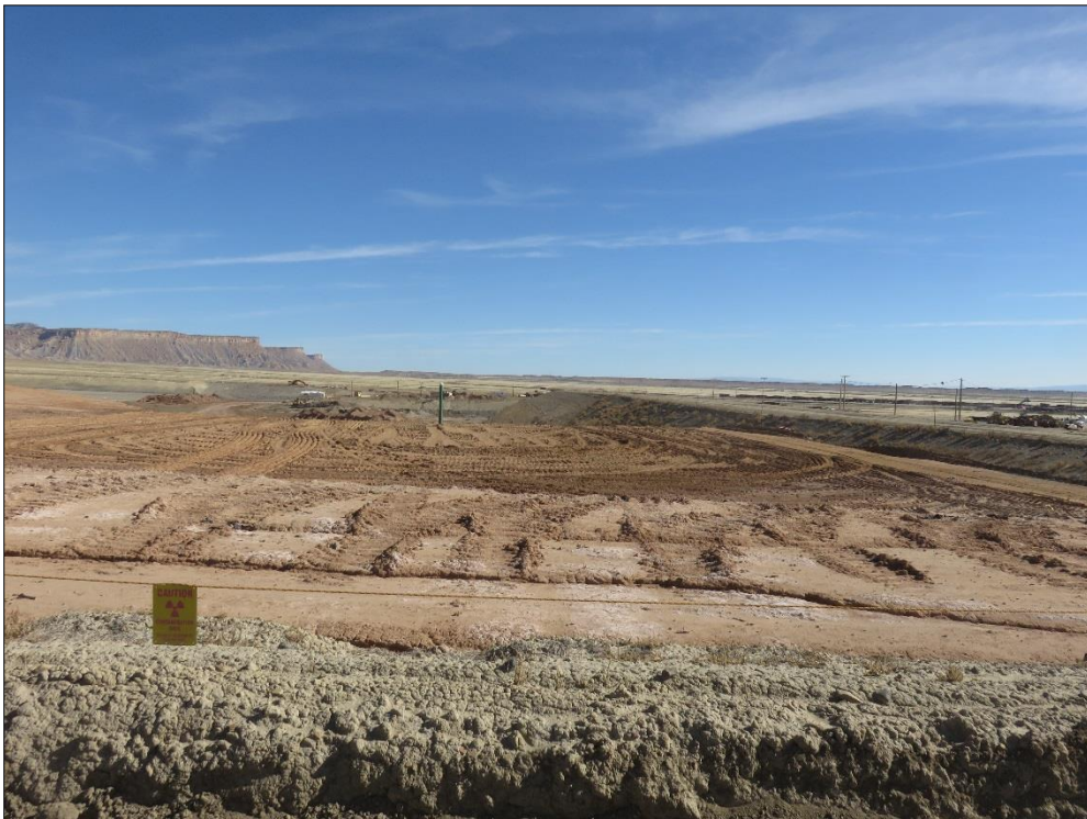
Photo 10. RRM Placement – Standpipe Compaction November 8, 2016
