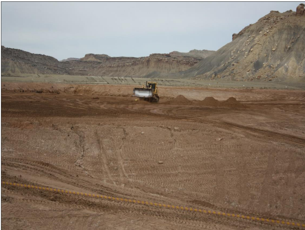
Photo 16. RRM Placement March 21, 2017
