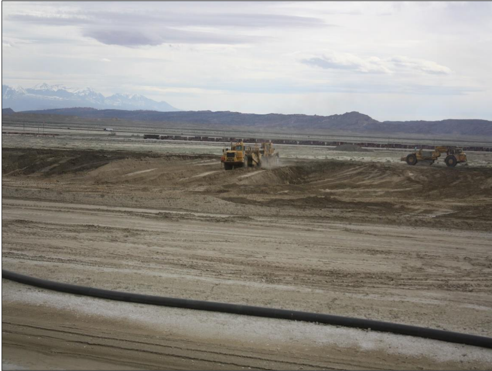
Photo 3. Phase 3b Cell Excavation March 22, 2017
