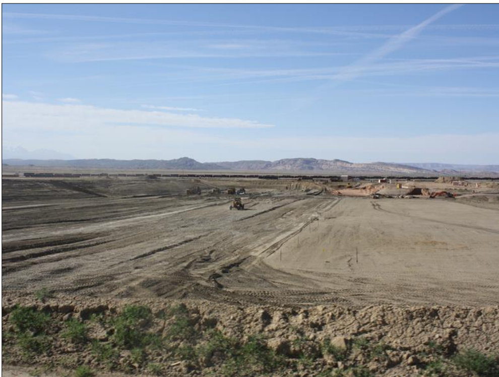
Photo 8. Phase 3b Cell Excavation May 15, 2017
