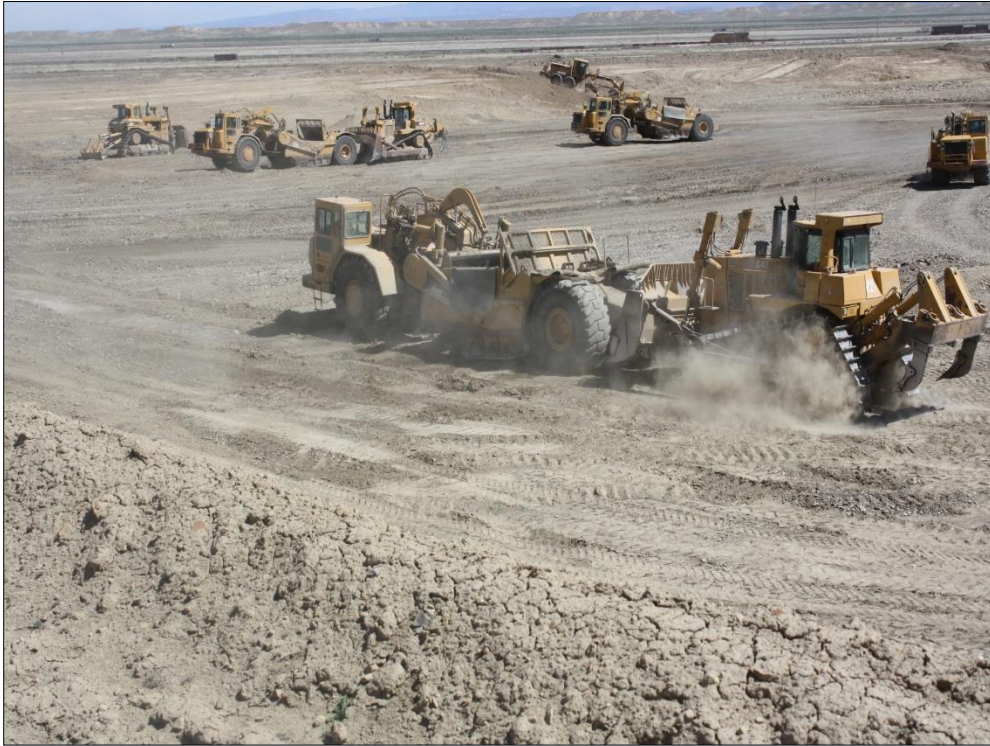
Photo 5. Phase 3b Cell Excavation April 20, 2017
