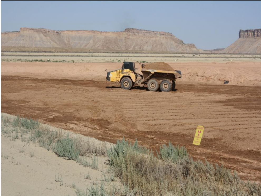
Photo 25. RRM Placement August 29, 2017
