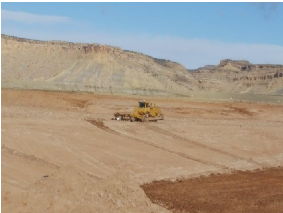
Photo 28. RRM Placement September 12, 2017
