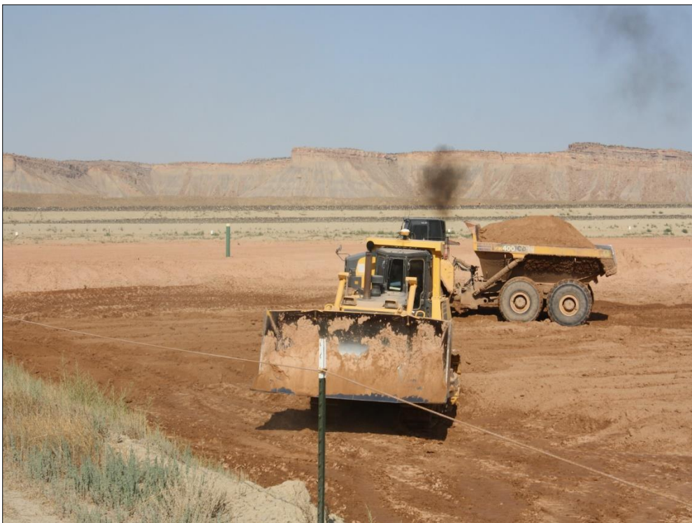
Photo 26. RRM Placement August 29, 2017
