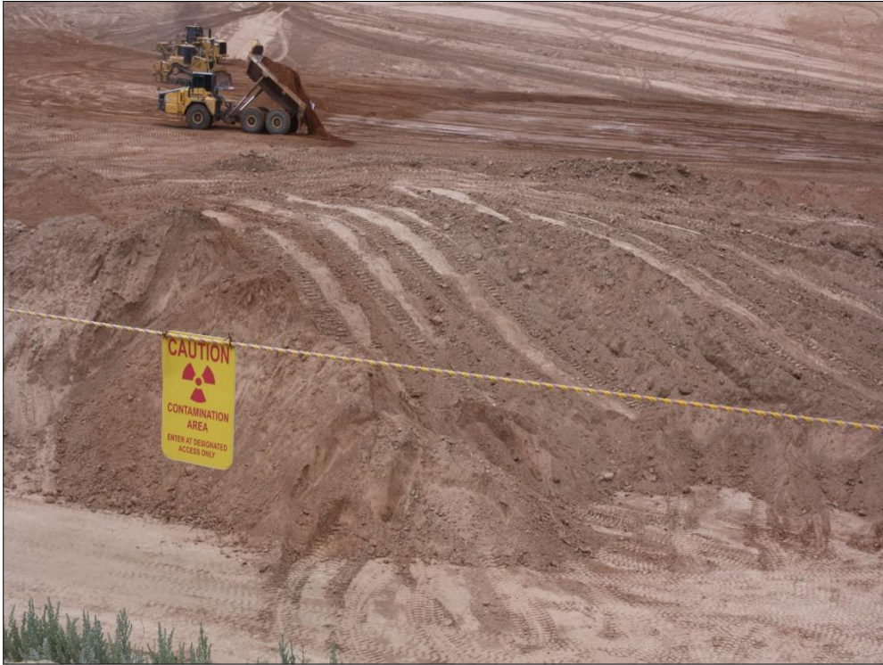
Photo 23. RRM Placement August 1, 2017
