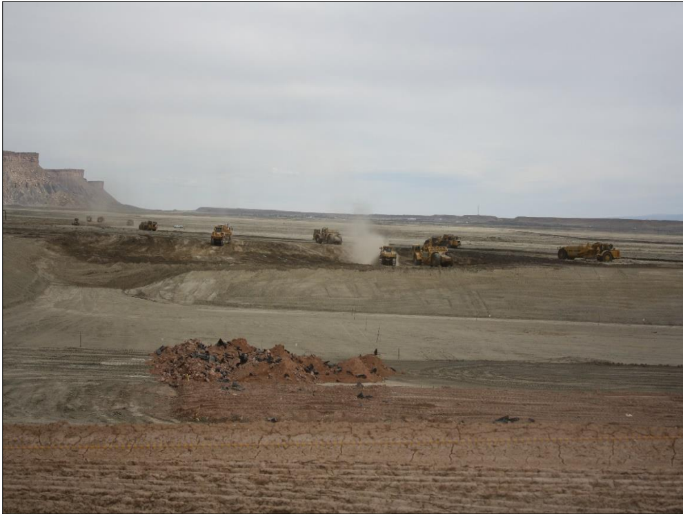
Photo 1. Phase 3b Cell Excavation March 21, 2017
