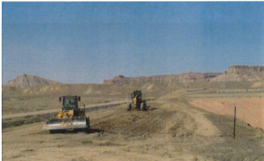
Photo 2 Compaction of Perimeter Berm Material
