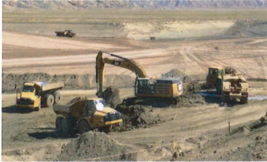
Photo 1 Excavation, Load Out, and Moisture Conditioning of the Old Dump Ramp
