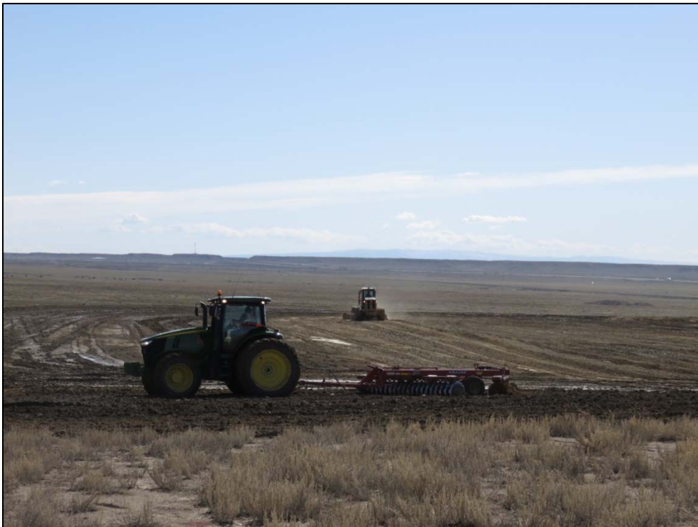
Photo 34. Spoils Embankment Placement April 5, 2016
