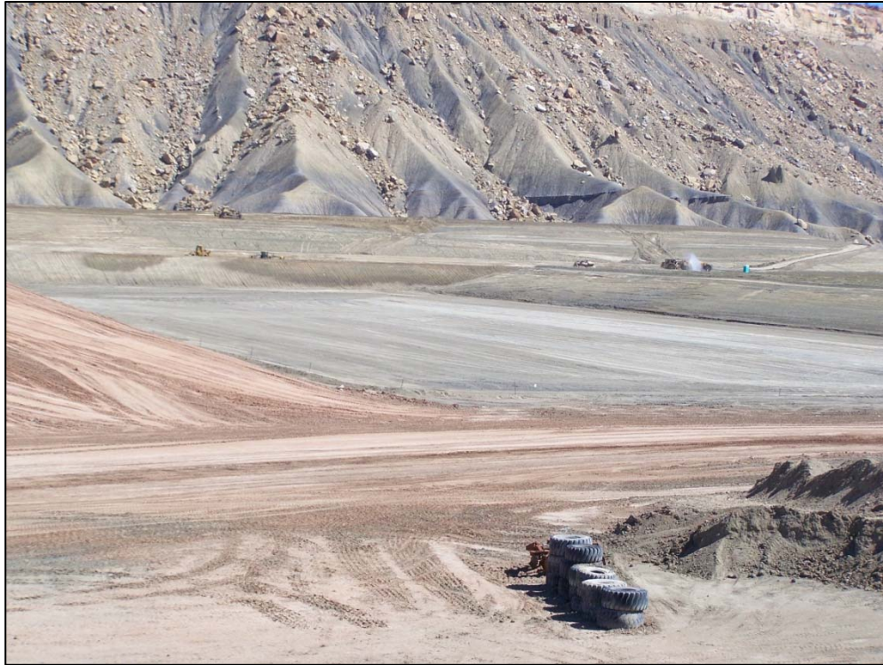
Photo 7. Phase 3a Cell Excavation May 12, 2016
