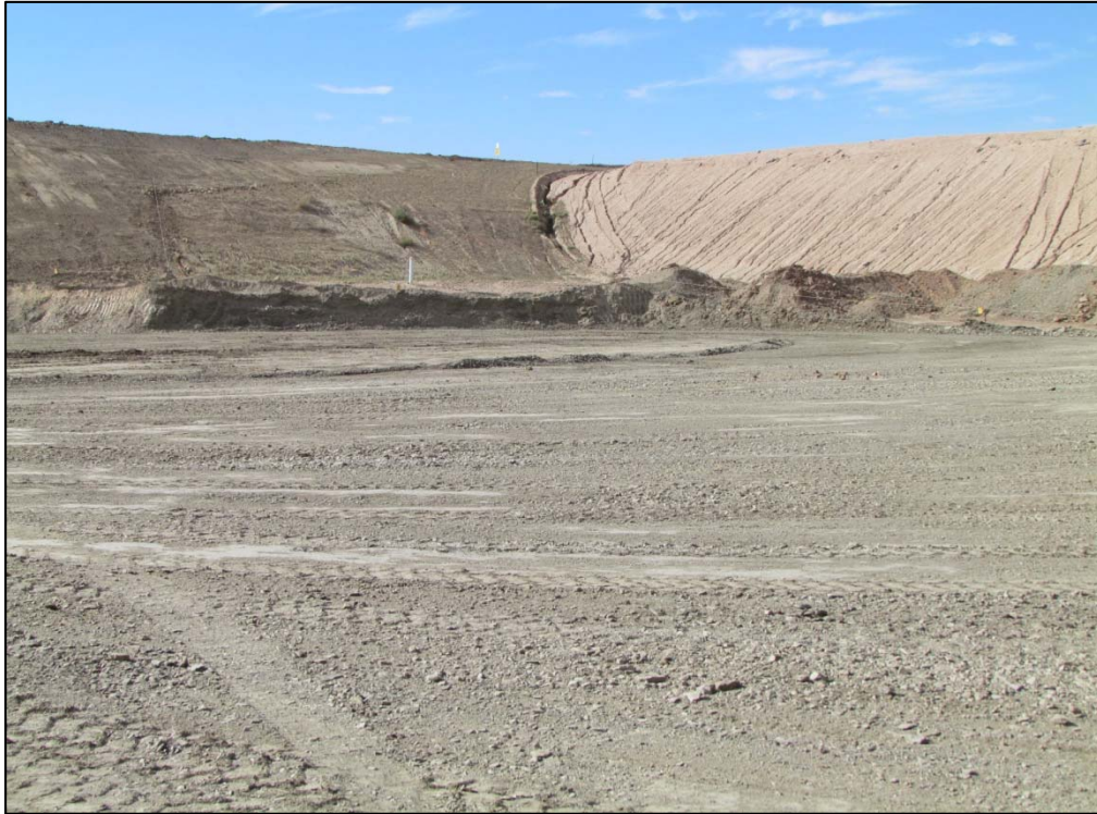
Photo 1. Removal of Former Dump Ramp in Phase 2 October 1, 2015
