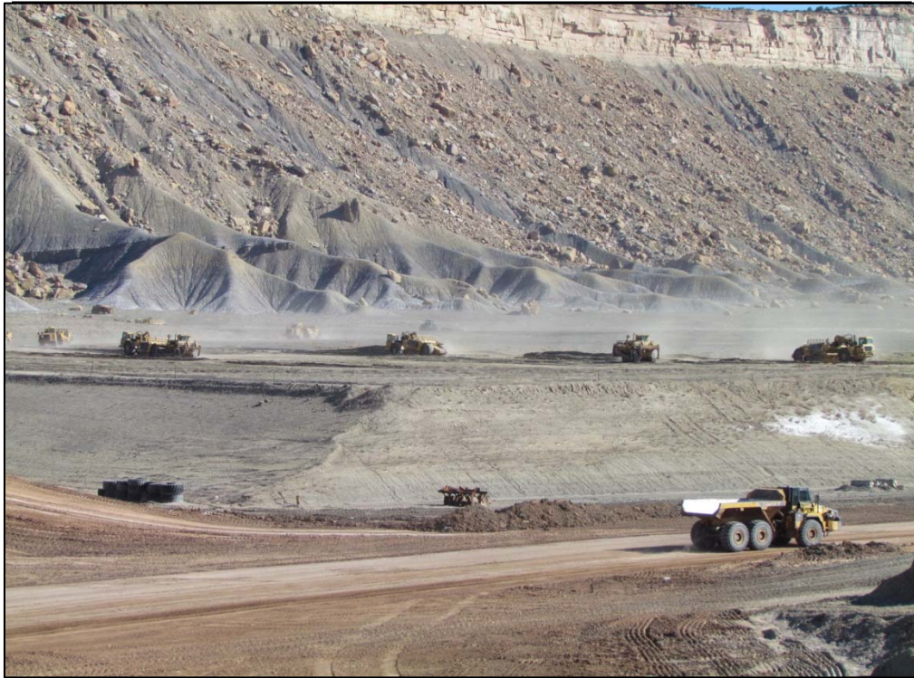
Photo 3. Phase 3a Cell Excavation March 22, 2016
