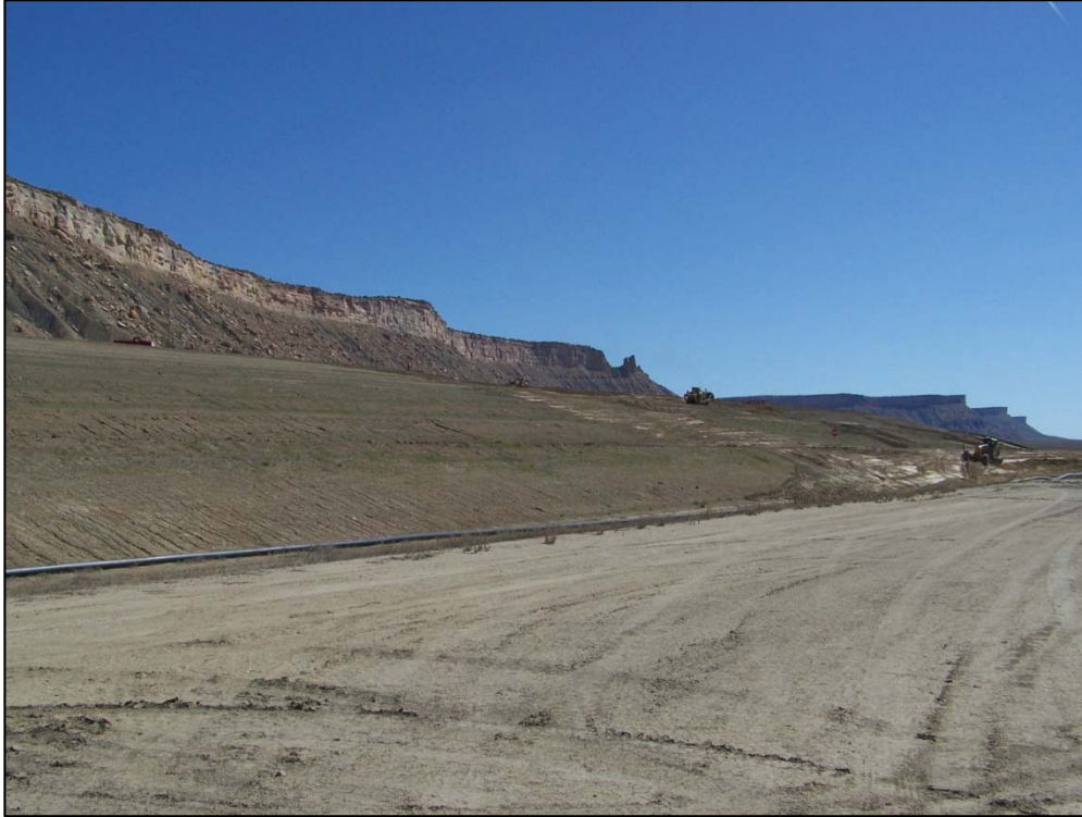
Photo 35. Spoils Embankment Placement May 12, 2016
