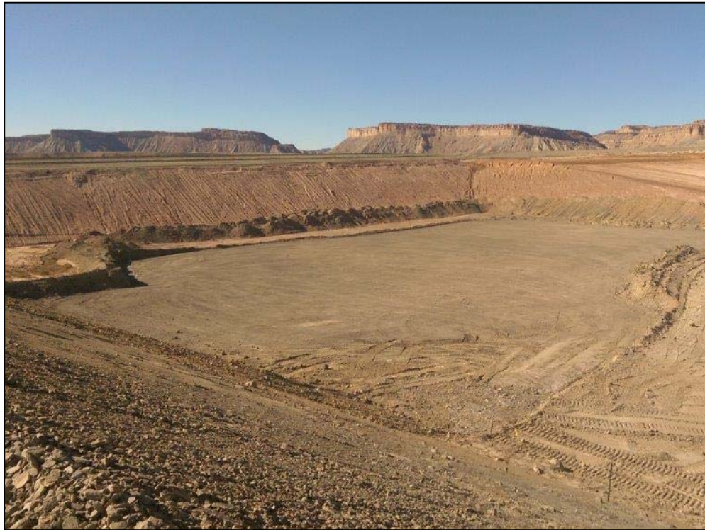
Photo 2. Removal of Former Dump Ramp in Phase 2 October 1, 2015
