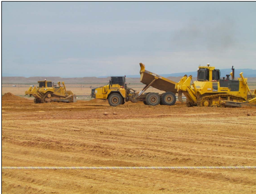
Photo 26. RRM Placement Top of Waste August 4, 2016
