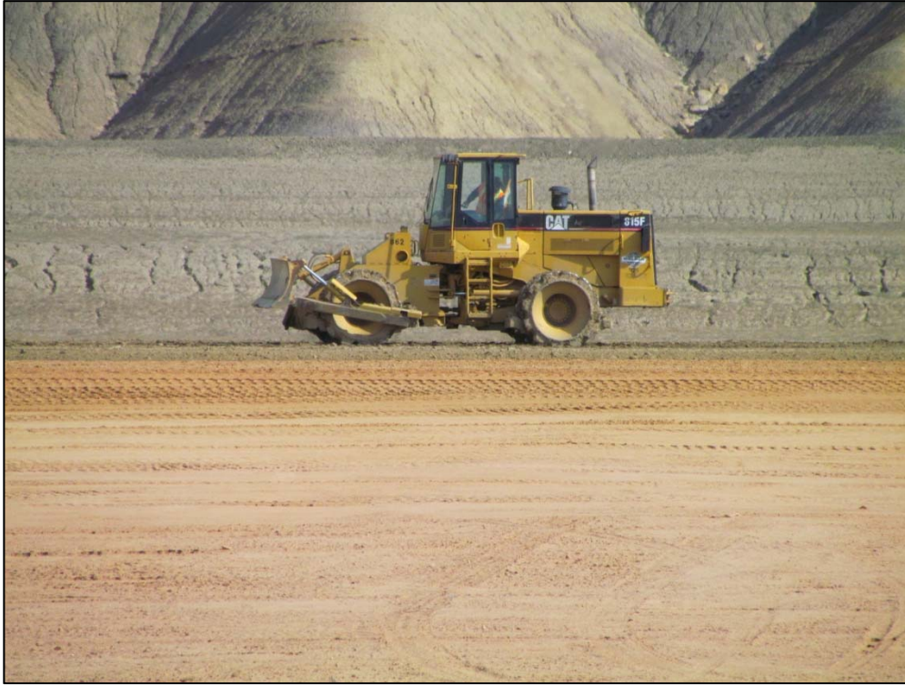
Photo 31. Interim Cover Placement August 25, 2016
