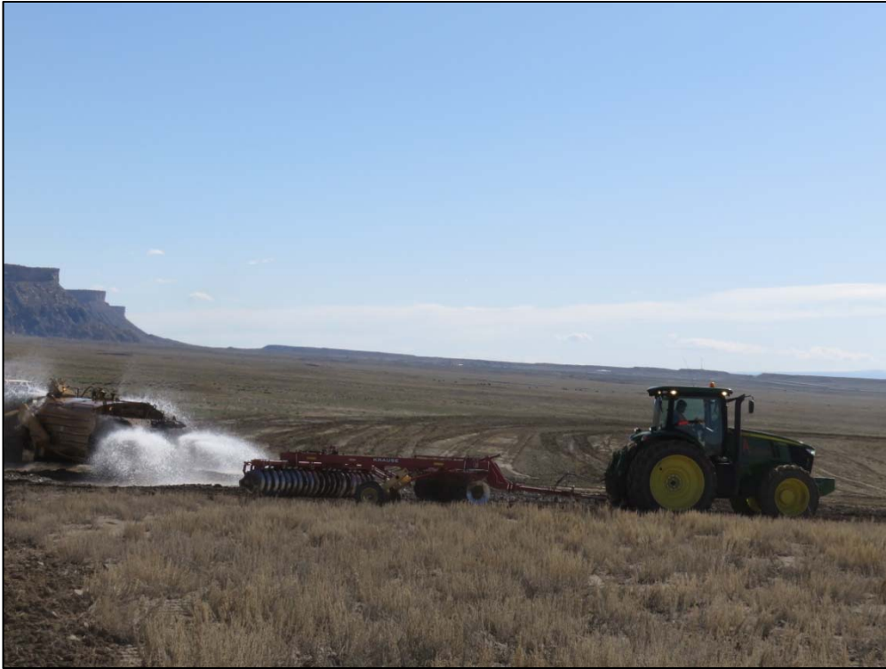
Photo 33. Spoils Embankment Placement April 5, 2016
