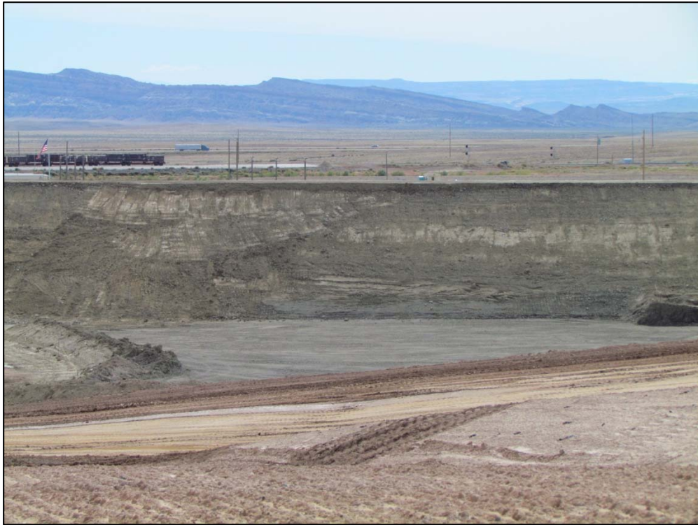
Photo 8. Perimeter Embankment October 8, 2015
