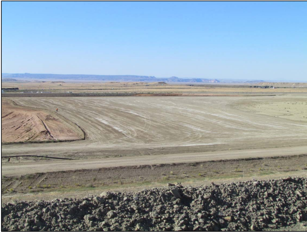
Photo 32. Completed Interim Cover September 8, 2016
