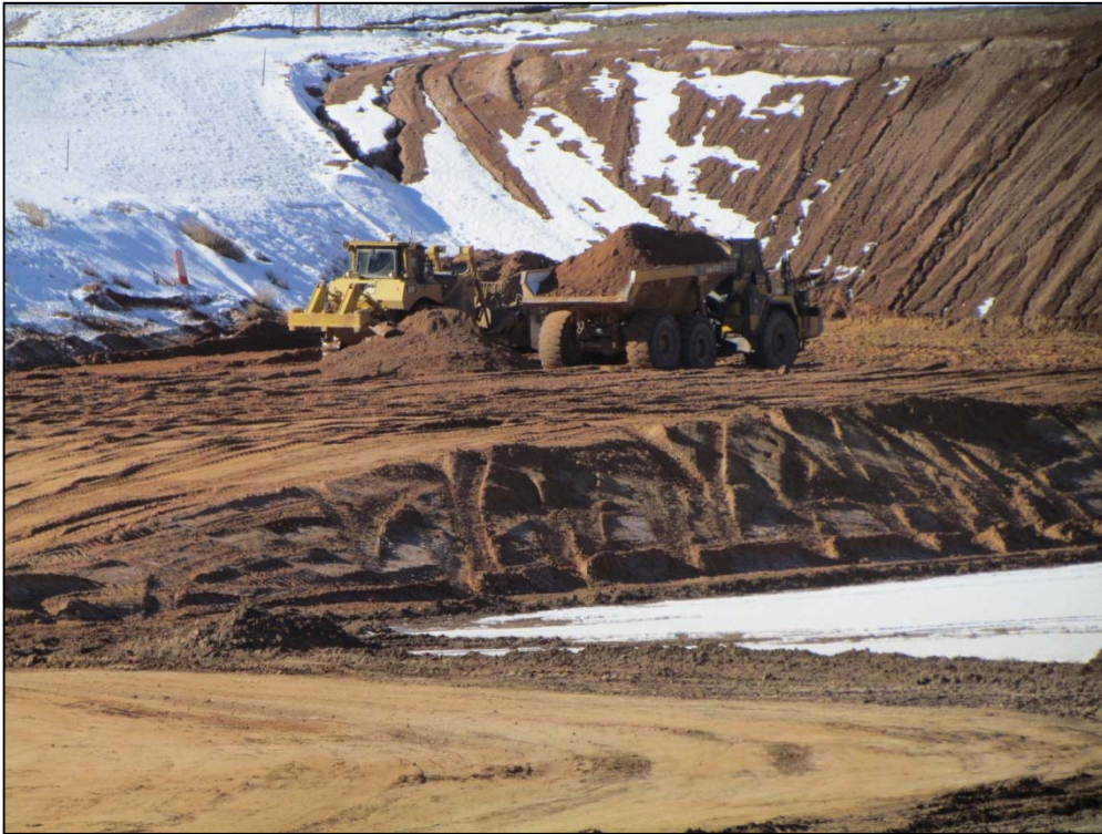
Photo 15. RRM Placement January 28, 2016
