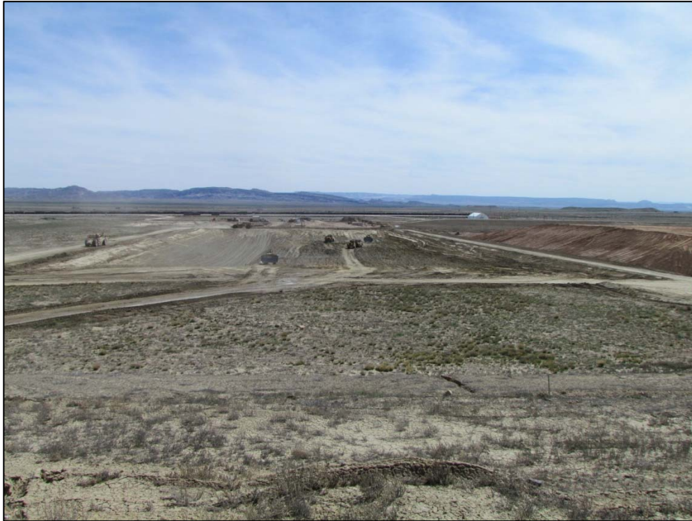
Photo 5. Phase 3a Cell Excavation April 7, 2016
