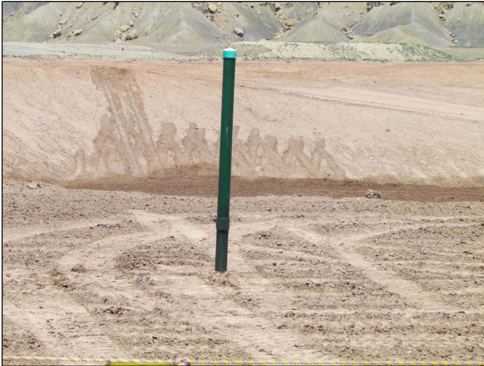
Photo 23. RRM Placement - Standpipe Compaction June 20, 2016
