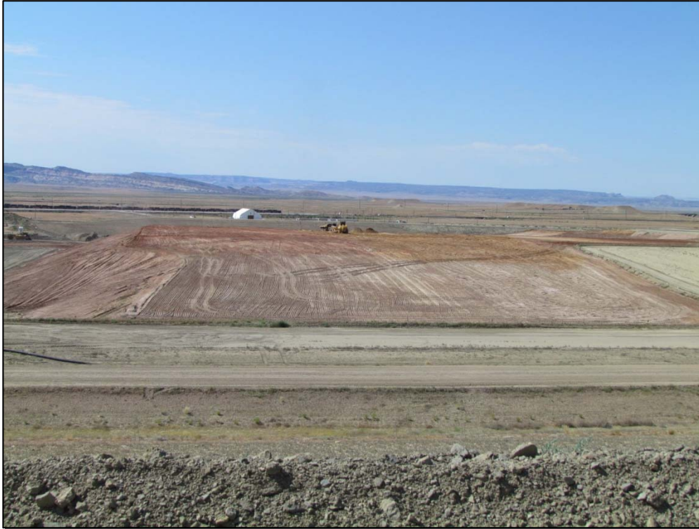
Photo 25. RRM Placement Top of Waste July 26, 2016
