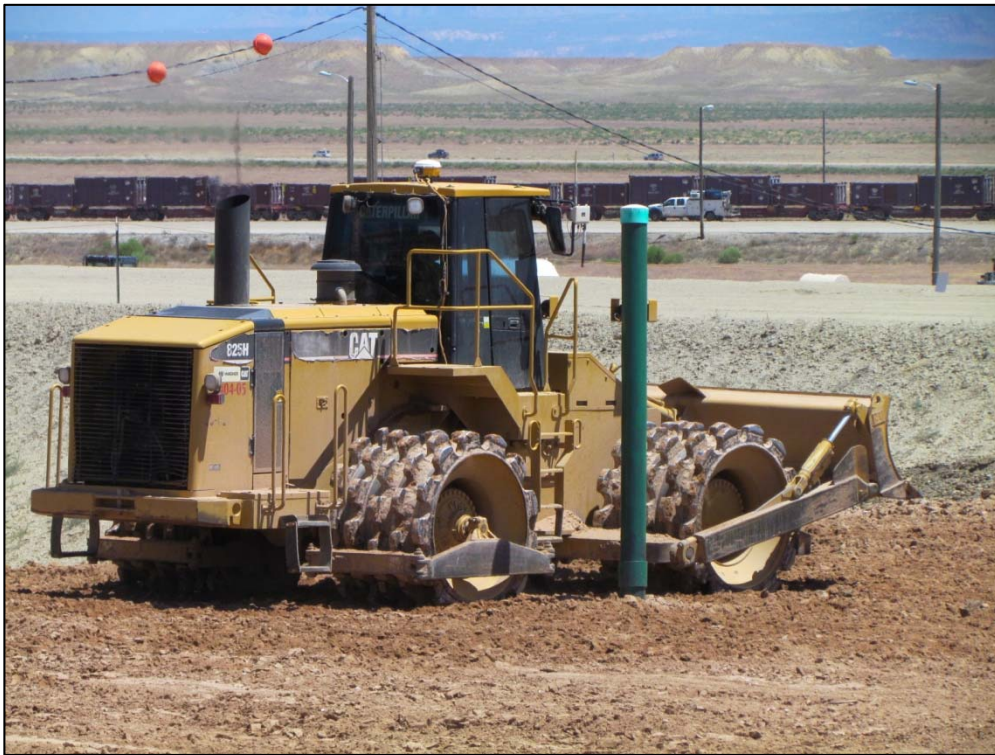
Photo 24. RRM Placement - Standpipe Compaction July 5, 2016
