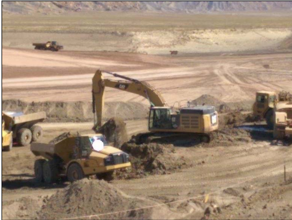
Photo 10. Perimeter Embankment October 2015
