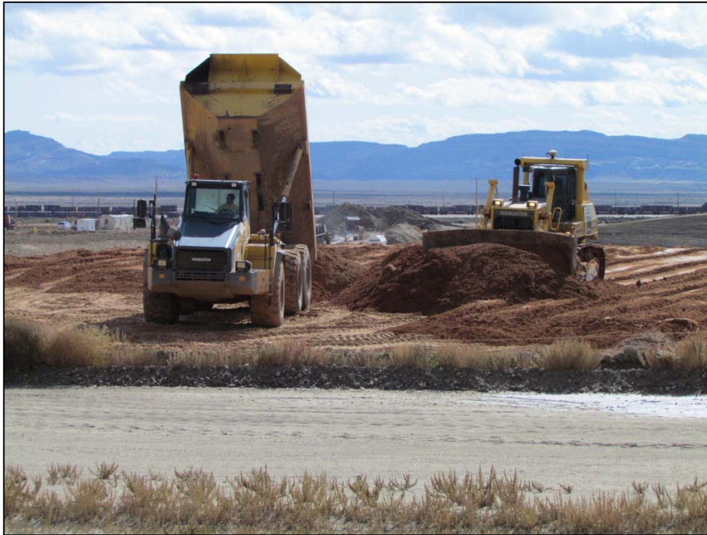
Photo 11. RRM Placement October 26, 2015
