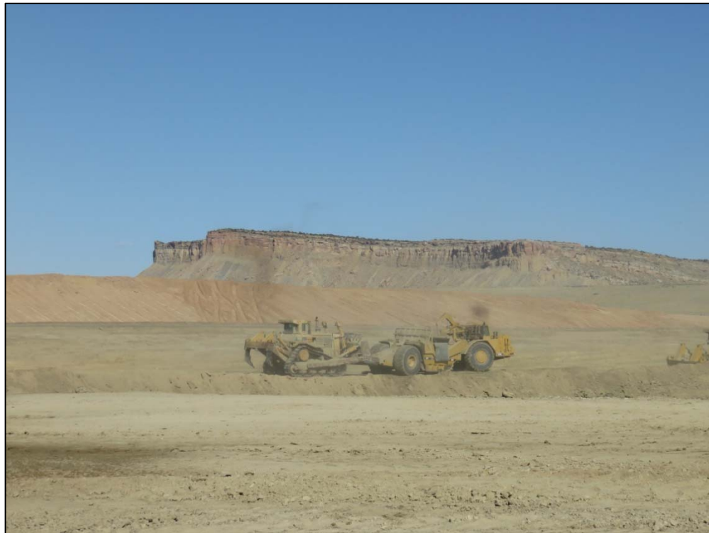
Photo 4. Phase 3a Cell Excavation April 5, 2016
