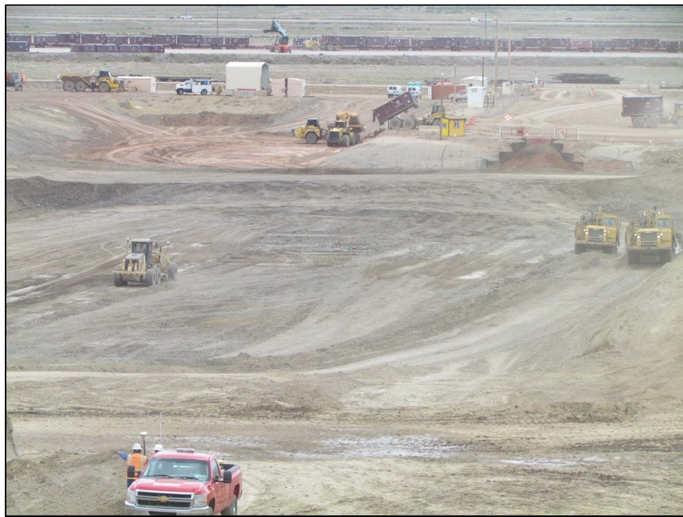
Photo 6. Phase 3a Cell Excavation April 18, 2016
