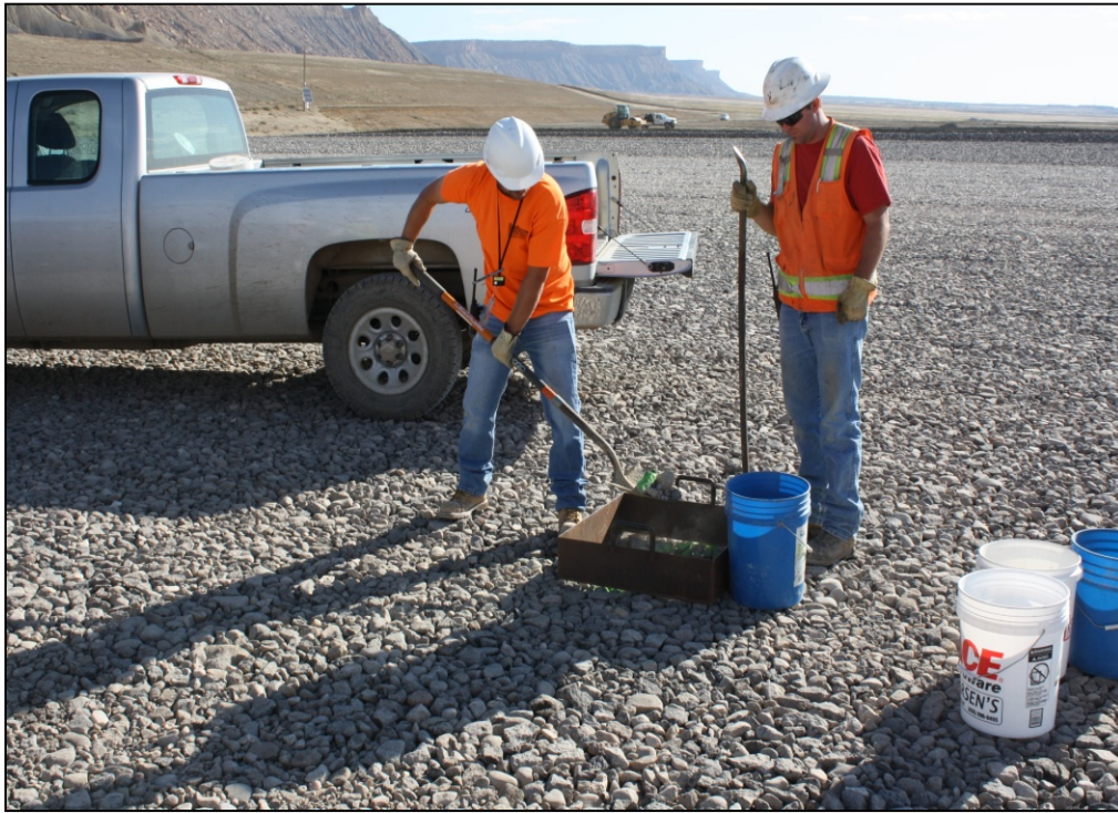
Photo 39. Infiltration and Biointrusion Barrier September 16, 2014
