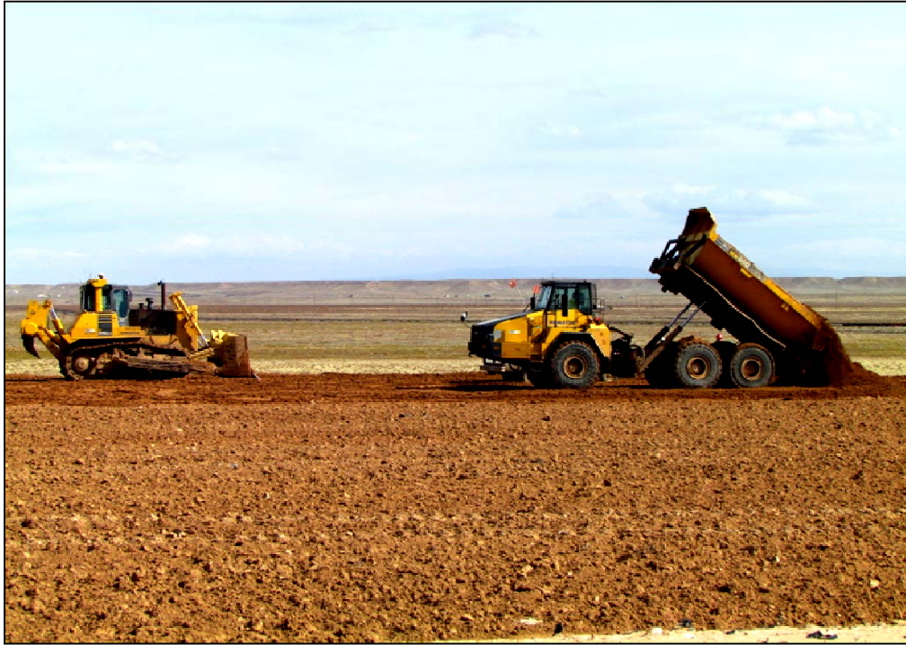
Photo 3. RRM Placement October 28, 2013
