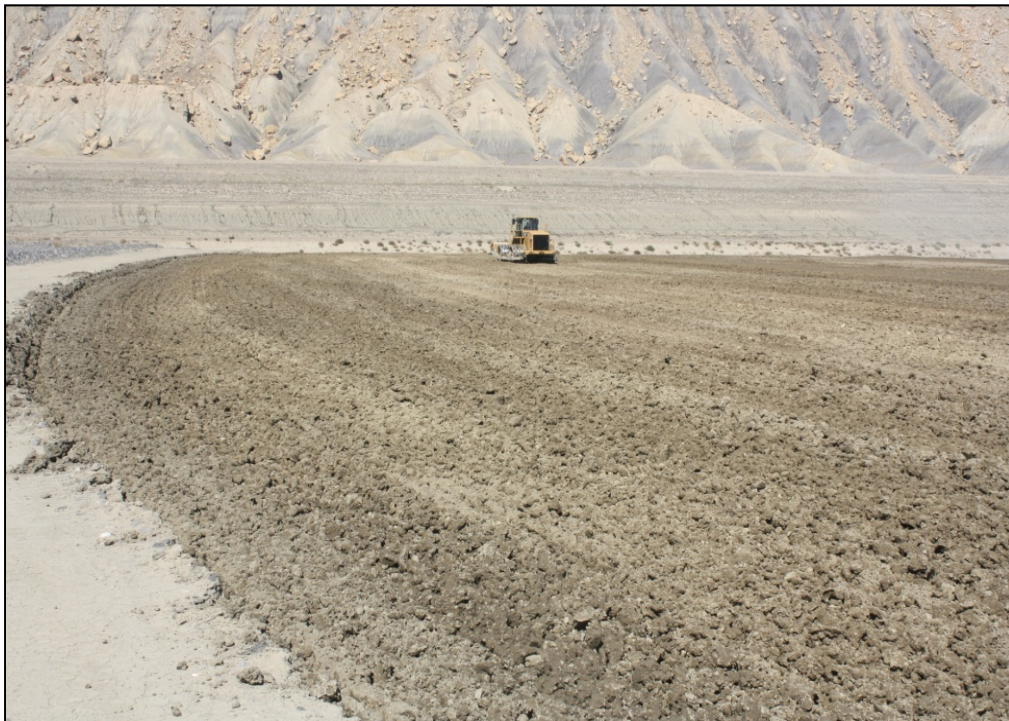
Photo 48. Frost Protection Layer September 25, 2014
