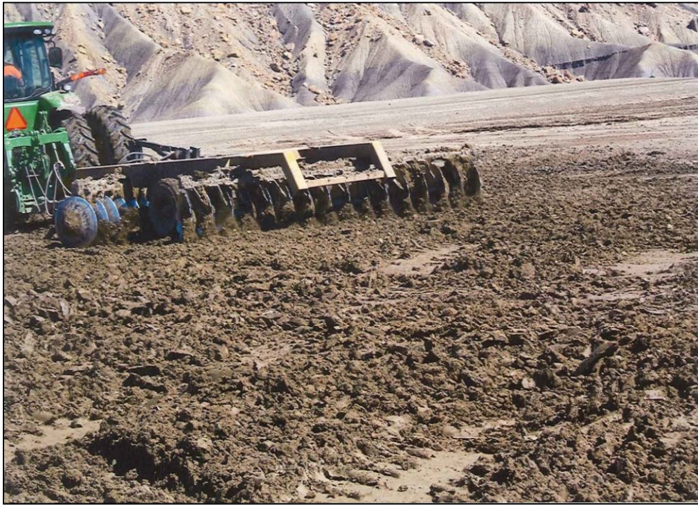
Photo 35. Radon Barrier September 23, 2014
