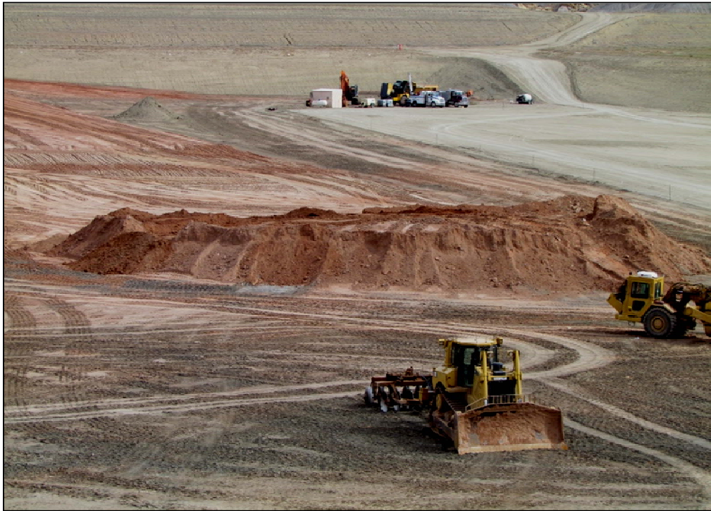
Photo 17. RRM Placement April 22, 2014
