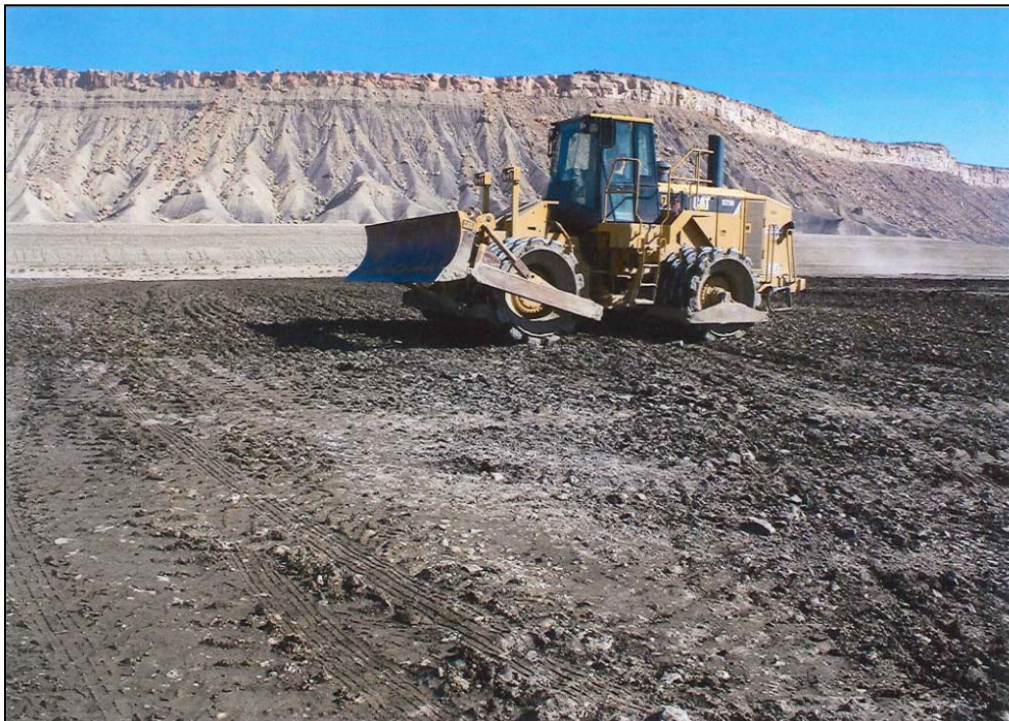
Photo 34. Radon Barrier September 18, 2014
