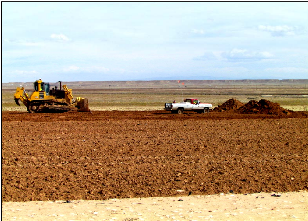
Photo 2. RRM Placement October 28, 2013
