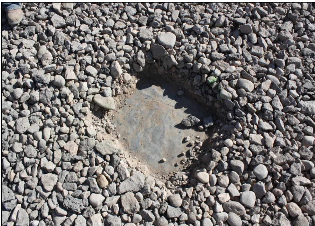
Photo 42. Infiltration and Biointrusion Barrier September 16, 2014
