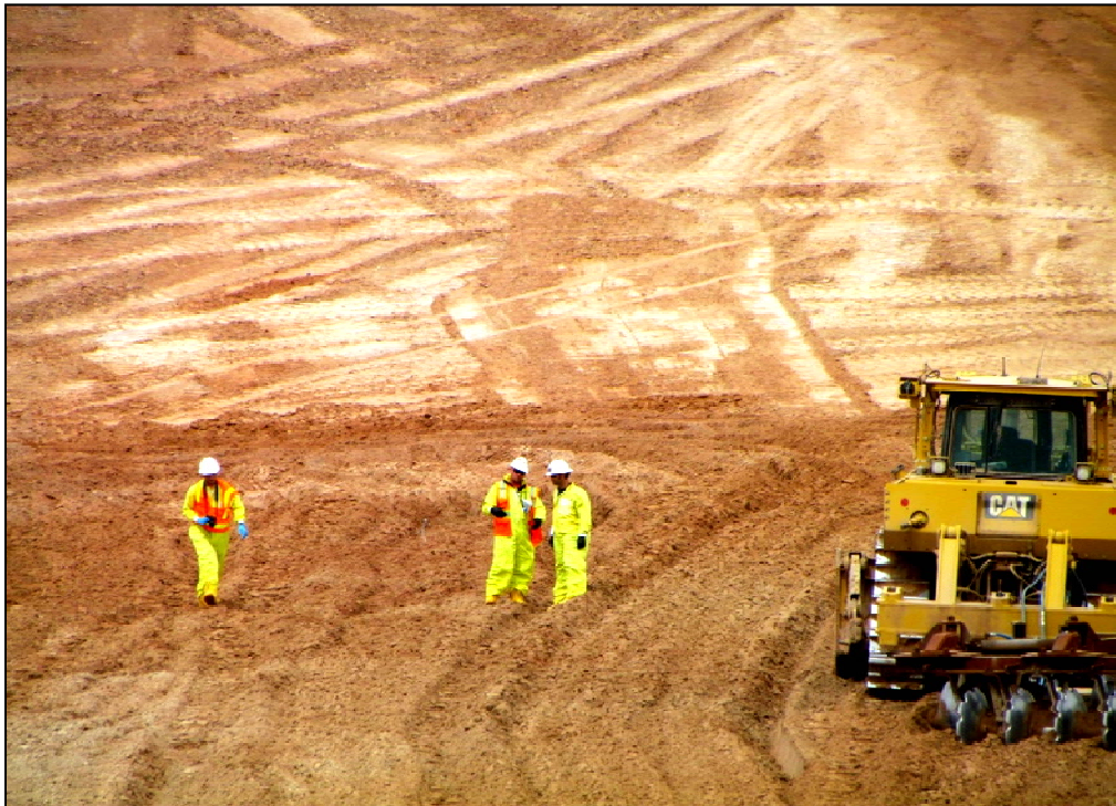
Photo 16. RRM Placement April 1, 2014
