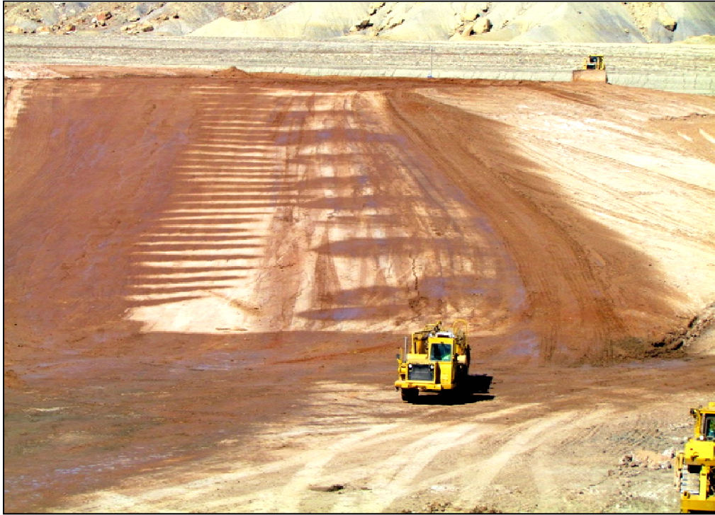
Photo 1. RRM Placement October 21, 2013
