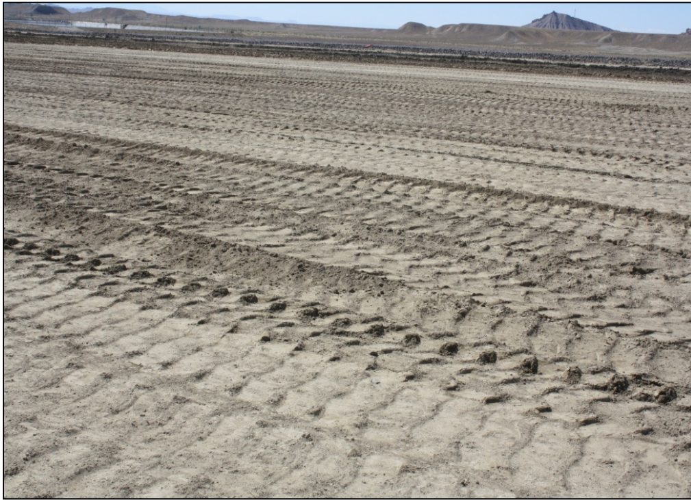
Photo 47. Frost Protection Layer September 25, 2014
