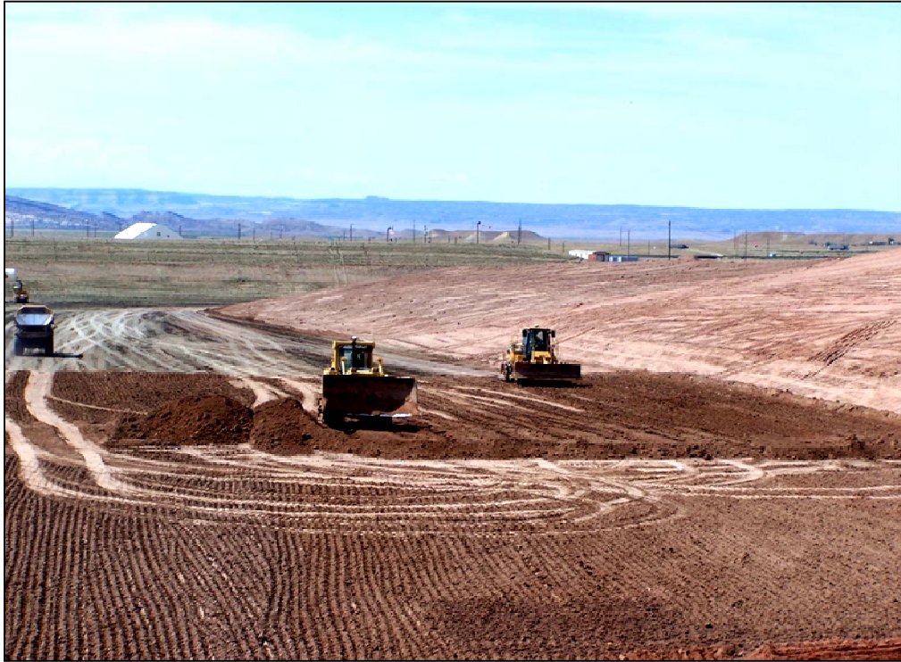
Photo 23. RRM Placement July 31, 2014
