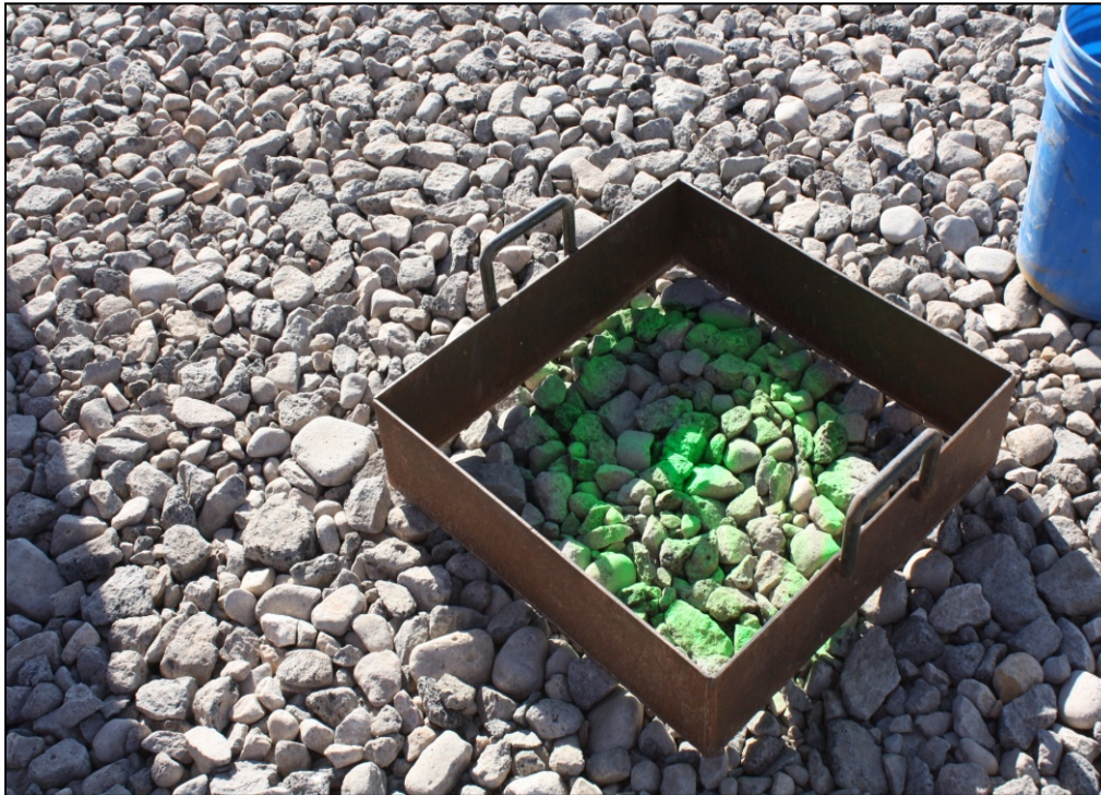
Photo 38. Infiltration and Biointrusion Barrier September 16, 2014
