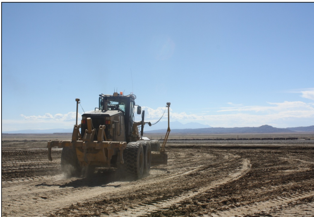
Photo 44. Frost Protection Layer September 19, 2014
