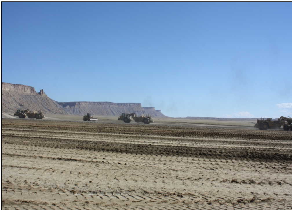
Photo 43. Frost Protection Layer September 19, 2014
