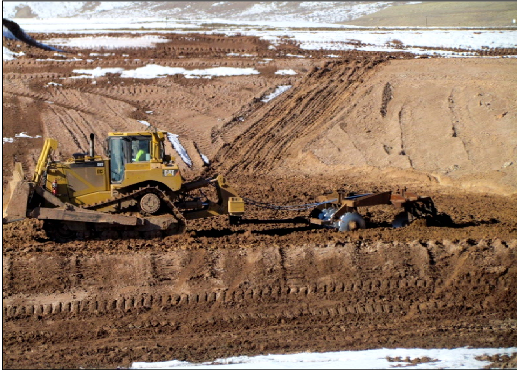
Photo 11. RRM Placement January 17, 2014
