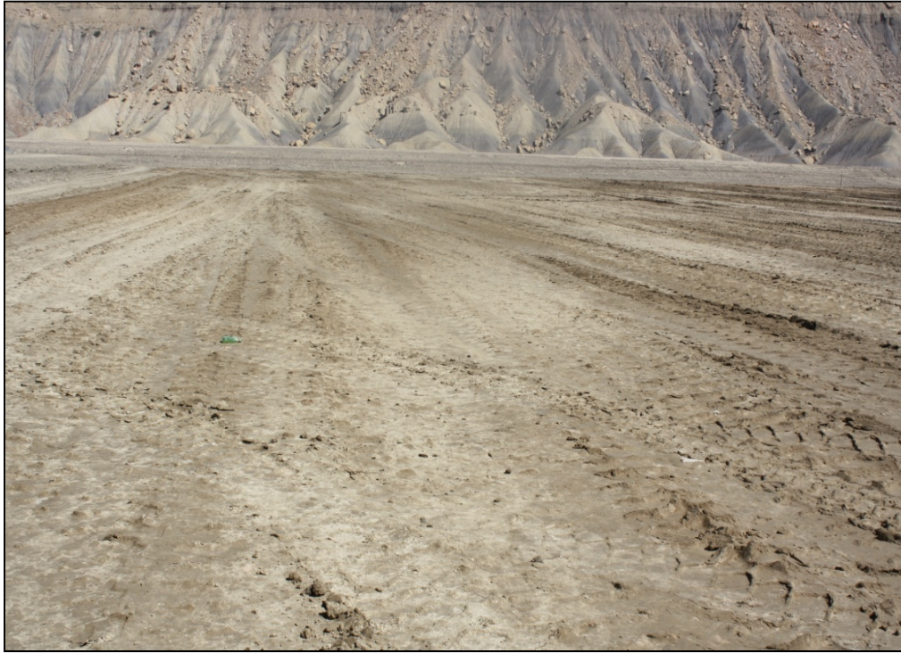
Photo 45. Frost Protection Layer September 19, 2014
