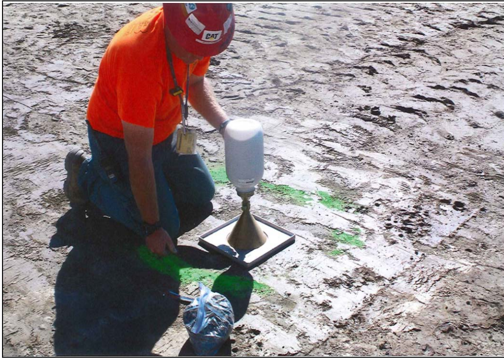
Photo 33. Radon Barrier September 18, 2014
