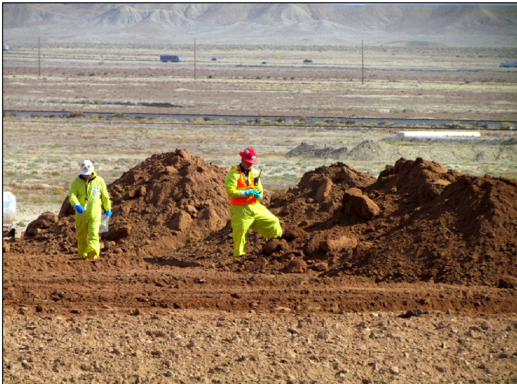
Photo 4. RRM Placement October 28, 2013
