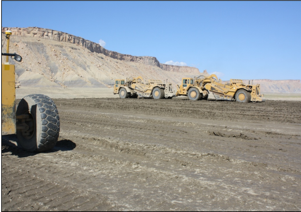
Photo 31. Radon Barrier September 10, 2014
