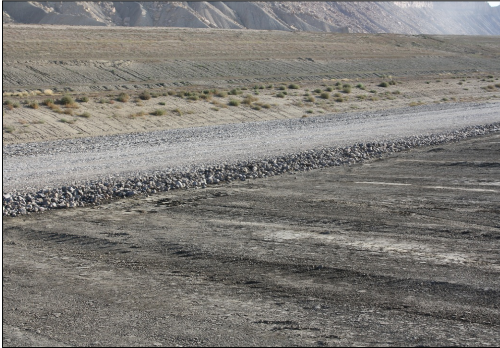
Photo 37. Infiltration and Biointrusion Barrier September 13, 2014
