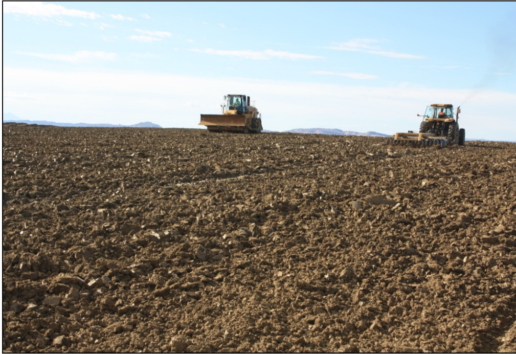
Photo 29. Radon Barrier August 2014
