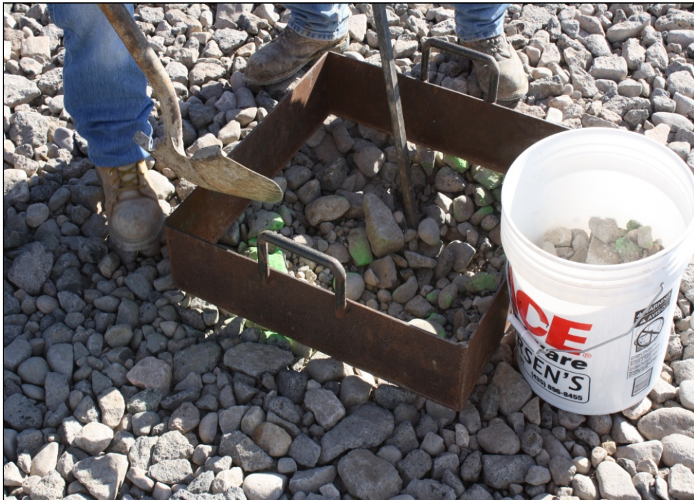
Photo 40. Infiltration and Biointrusion Barrier September 16, 2014
