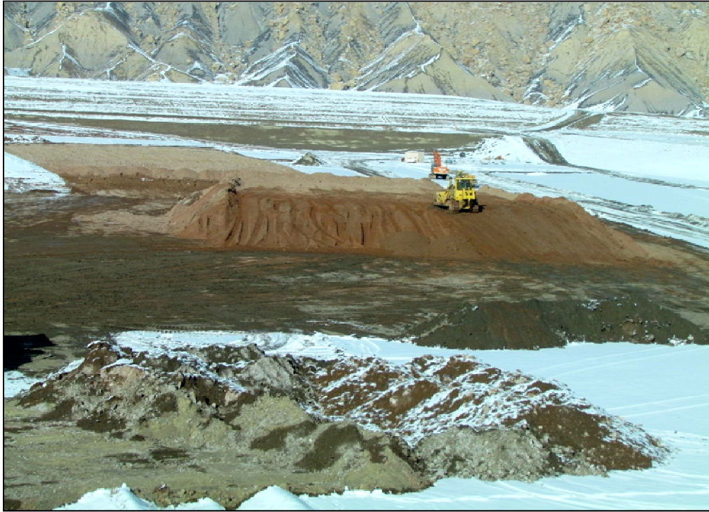
Photo 9. RRM Placement December 17, 2013
