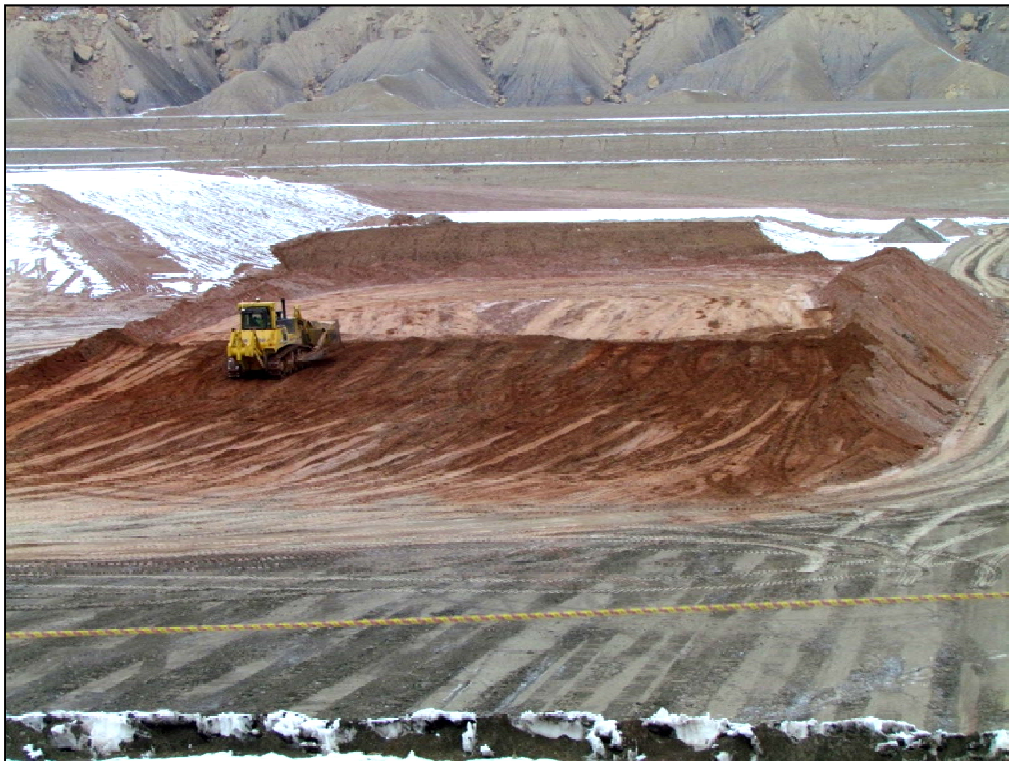
Photo 10. RRM Placement January 7, 2014
