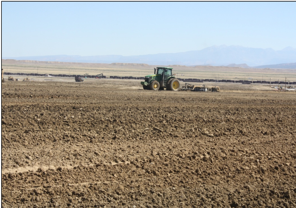
Photo 46. Frost Protection Layer September 25, 2014
