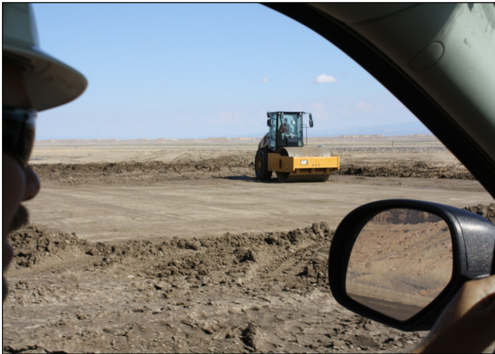
Photo 32. Radon Barrier September 10, 2014
