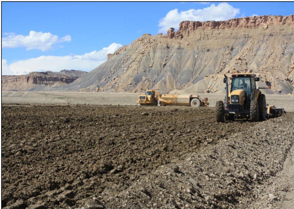
Photo 30. Radon Barrier August 2014
