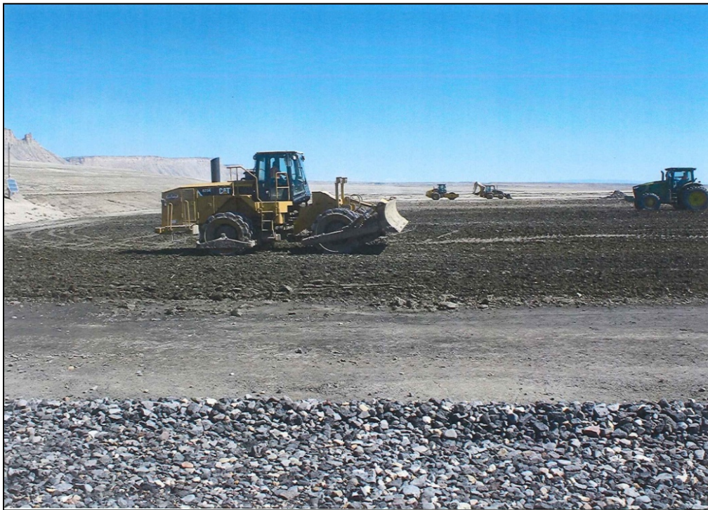
Photo 36. Radon Barrier September 26, 2014
