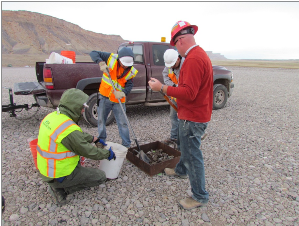
Photo 32. Biointrusion Barrier Sampling October 9, 2014
