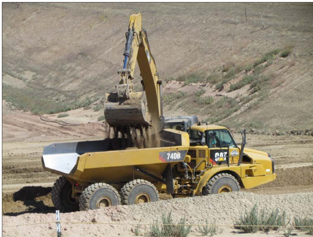
Photo 2. Dump Ramp Removal September 9, 2015
