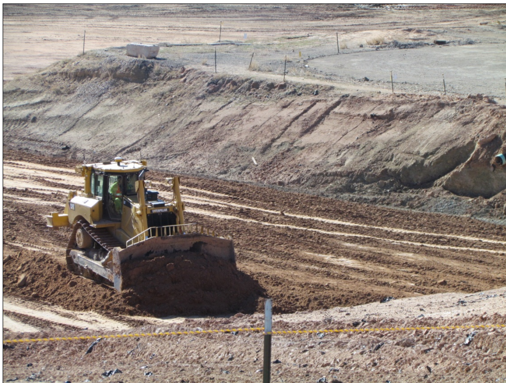
Photo 21. RRM Placement April 28, 2015
