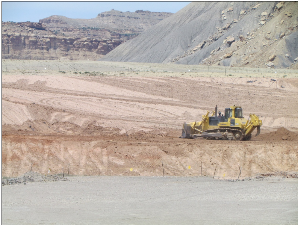
Photo 22. RRM Compaction June 23, 2015
