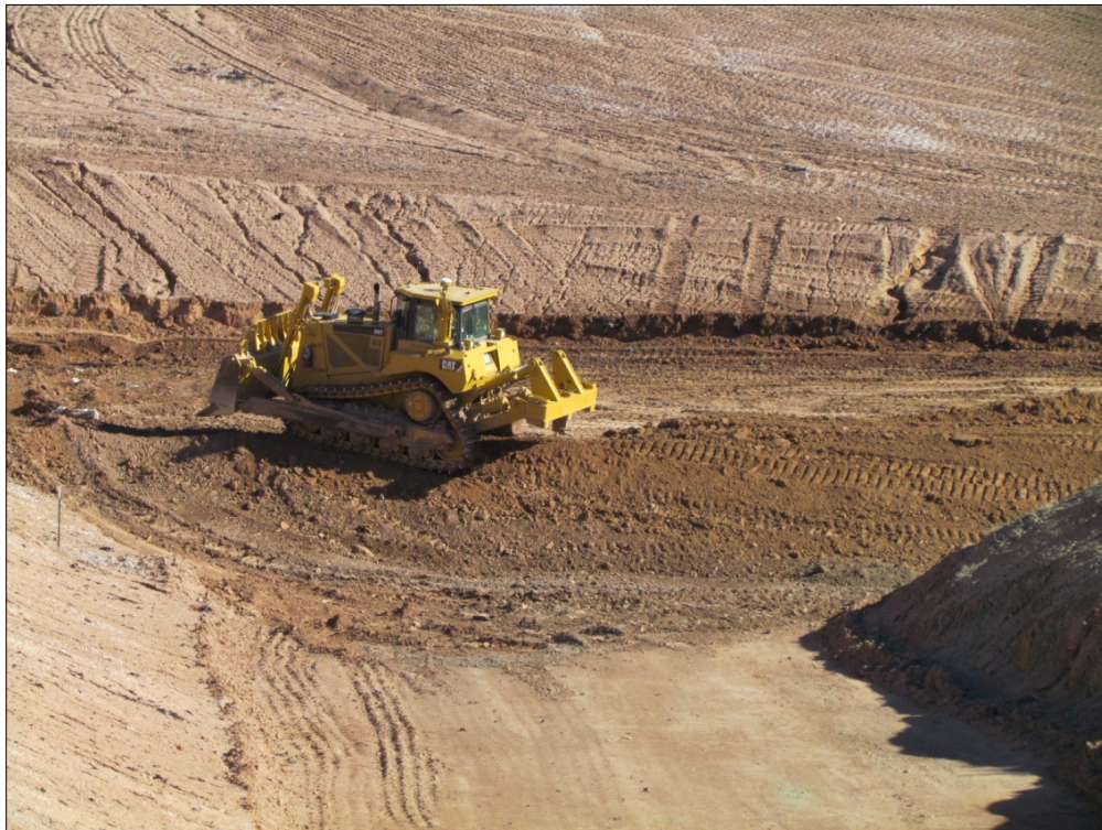
Photo 20. RRM Compaction April 28, 2015
