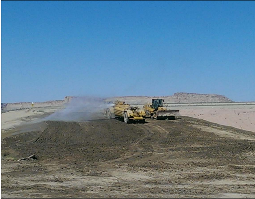
Photo 5. Compaction and Moisture Conditioning of Embankment Fill September 10, 2015
