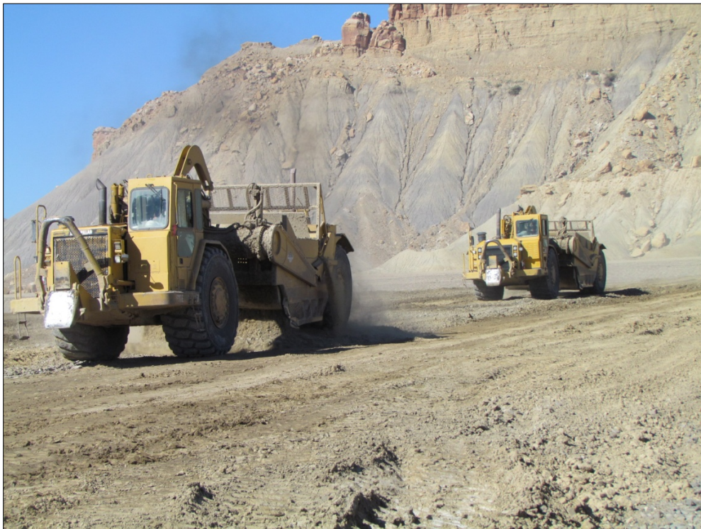
Photo 34. Frost Protection Layer Placement October 14, 2014
