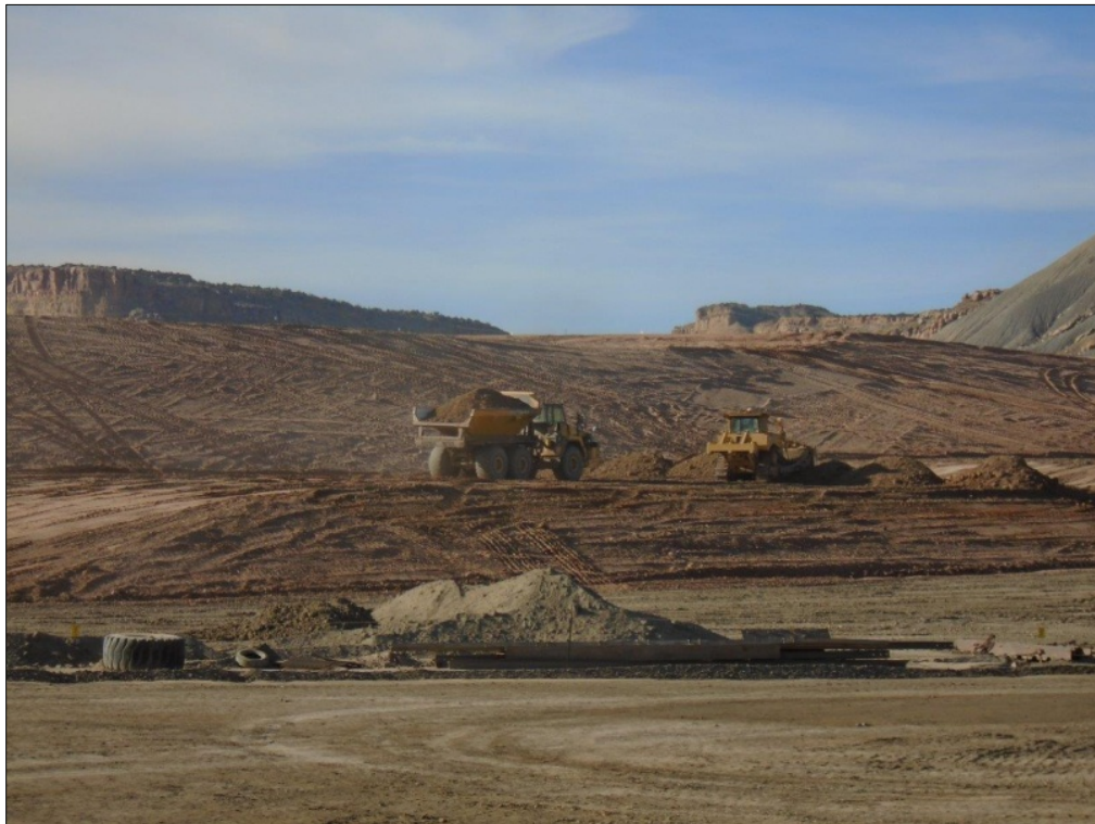
Photo 6. RRM Placement October 17, 2014
