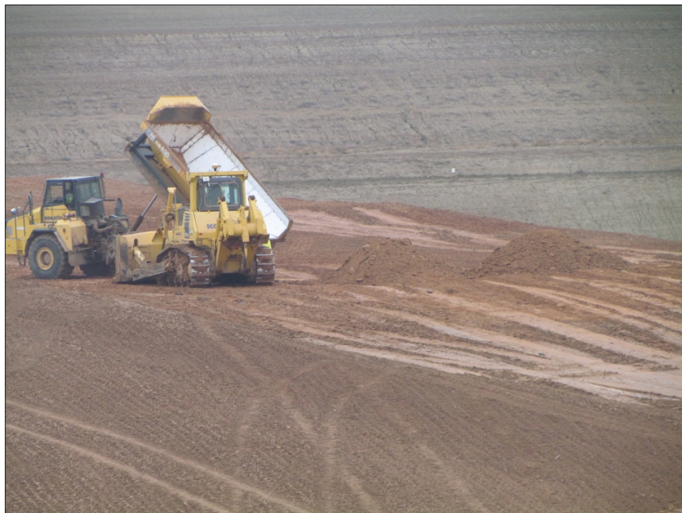
Photo 9. RRM Placement December 29, 2014
