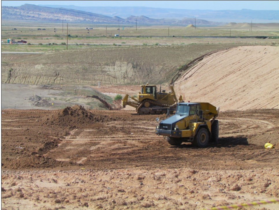
Photo 26. RRM Placement July 1, 2015
