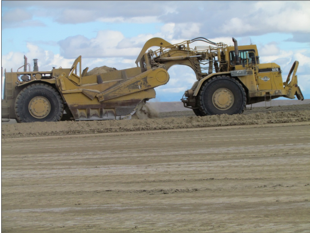
Photo 35. Frost Protection Layer Placement October 29, 2014
