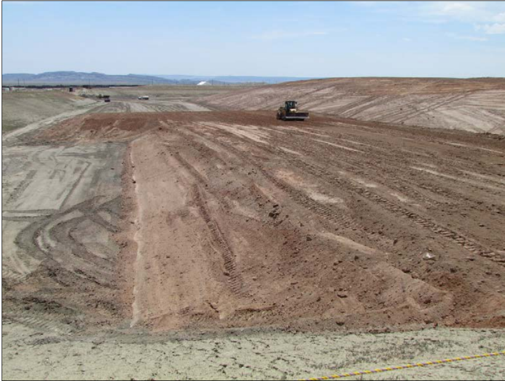
Photo 24. RRM Compaction June 23, 2015
