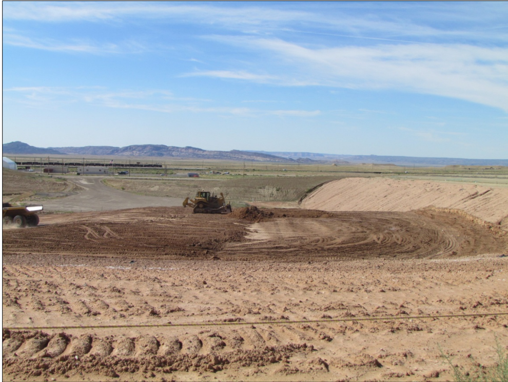
Photo 28. RRM Placement July 29, 2015
