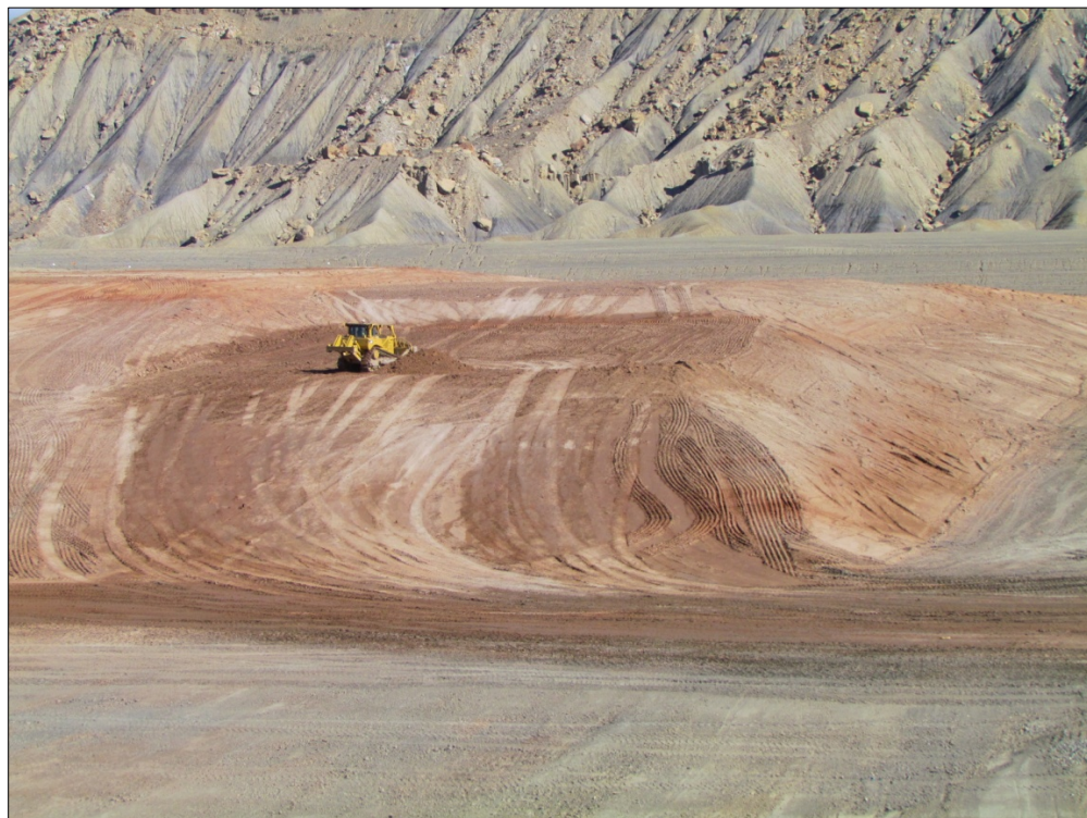
Photo 19. RRM Compaction April 15, 2015
