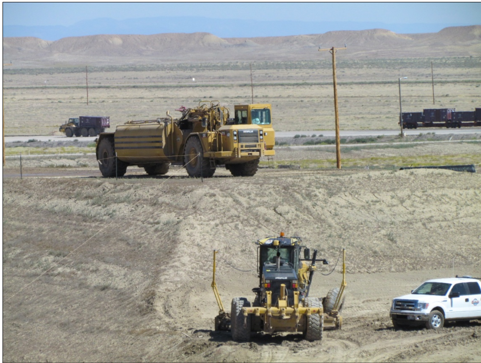
Photo 1. Preparing Material for Perimeter Embankment September 9, 2015
