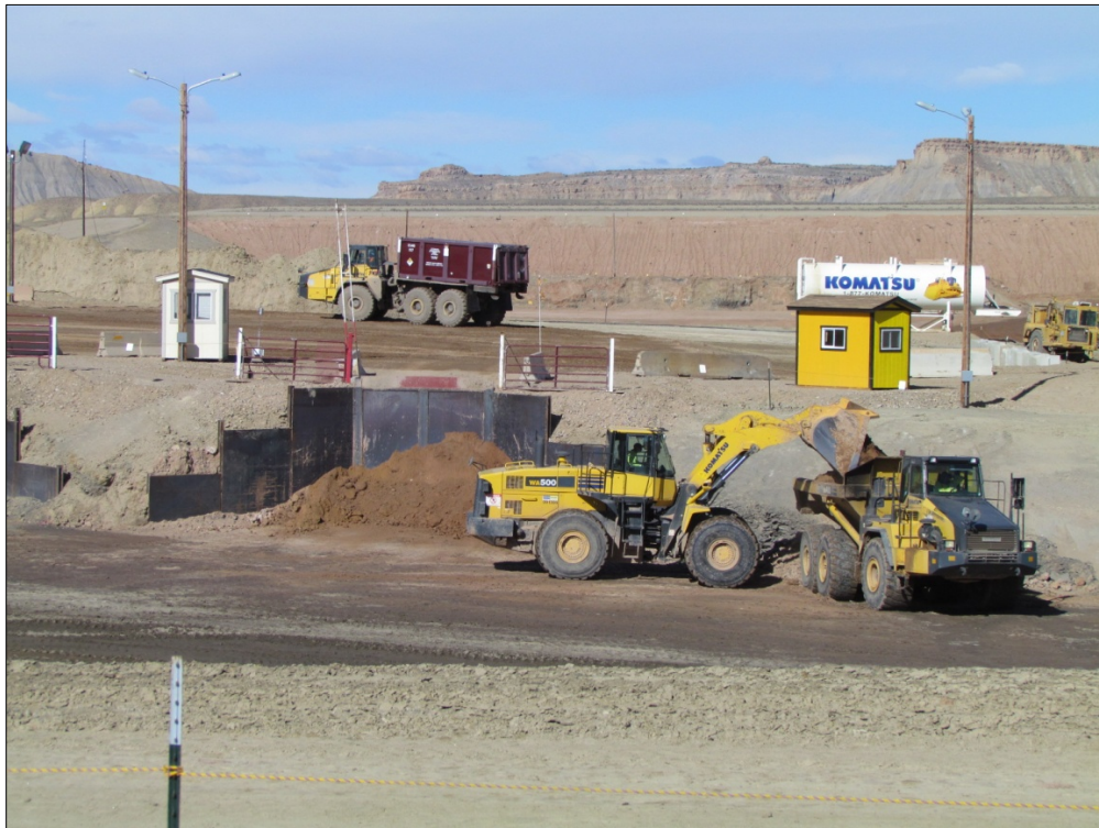
Photo 18. RRM Placement April 15, 2015
