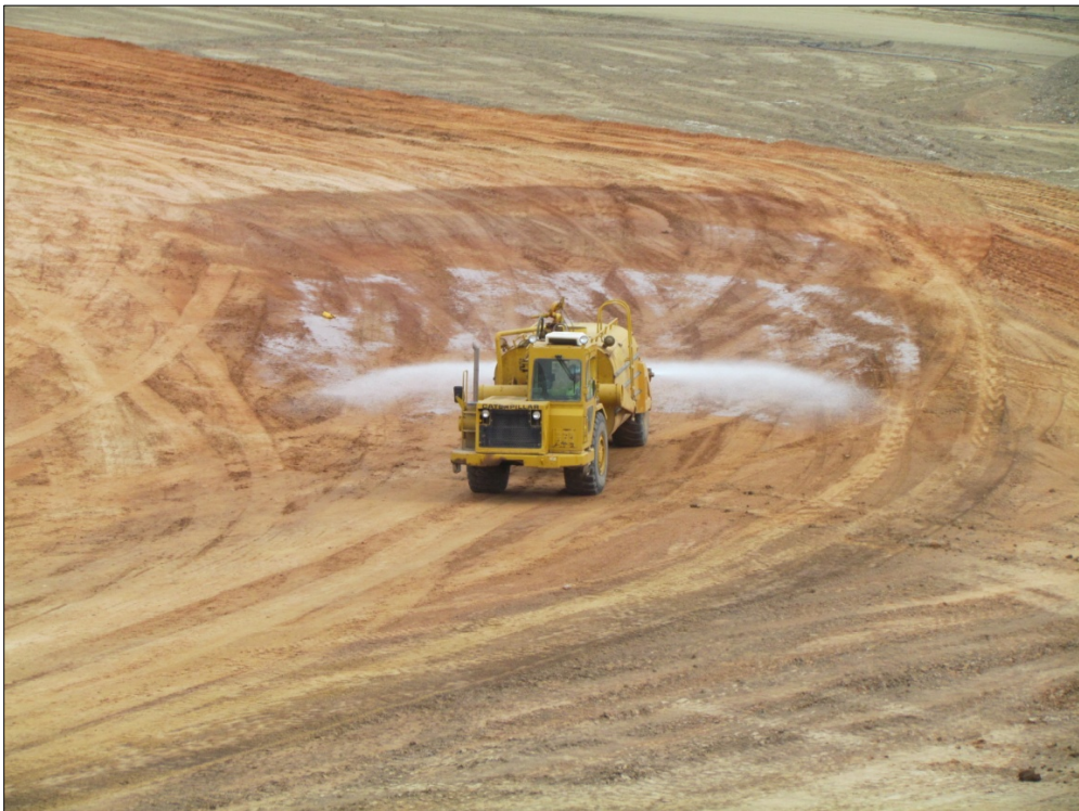
Photo 17. Dust Control March 11, 2015
