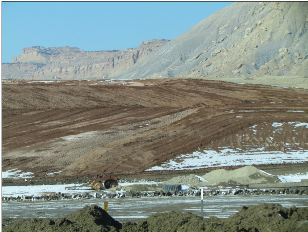
Photo 12. RRM Placement January 8, 2015
