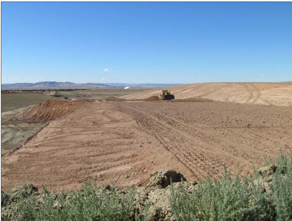
Photo 27. RRM Placement July 22, 2015
