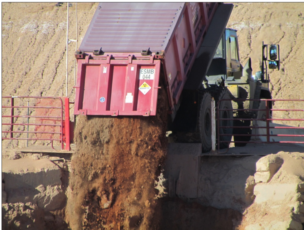
Photo 7. Modified Container Dumping November 6, 2014
