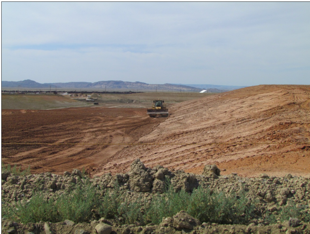
Photo 25. RRM Placement July 1, 2015
