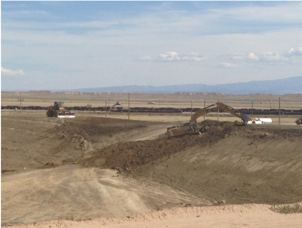
Photo 3. Embankment Construction September 28, 2015
