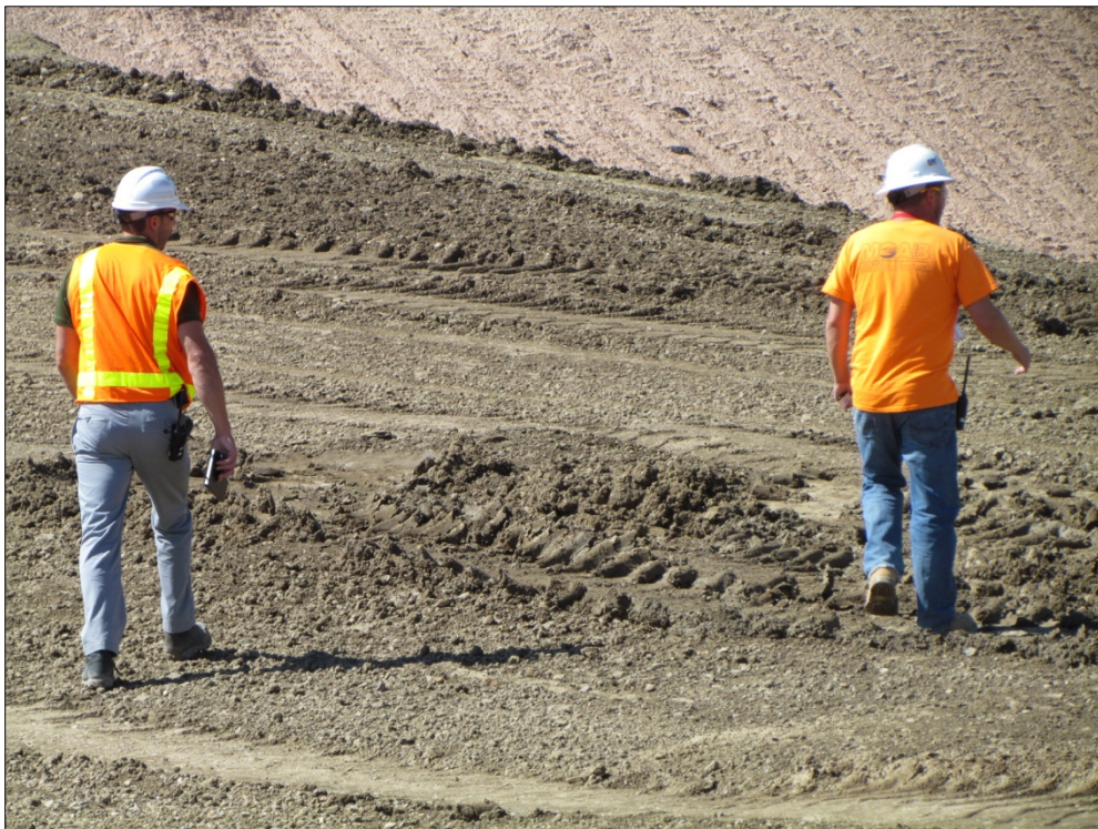
Photo 4. QC Embankment Inspection September 9, 2015
