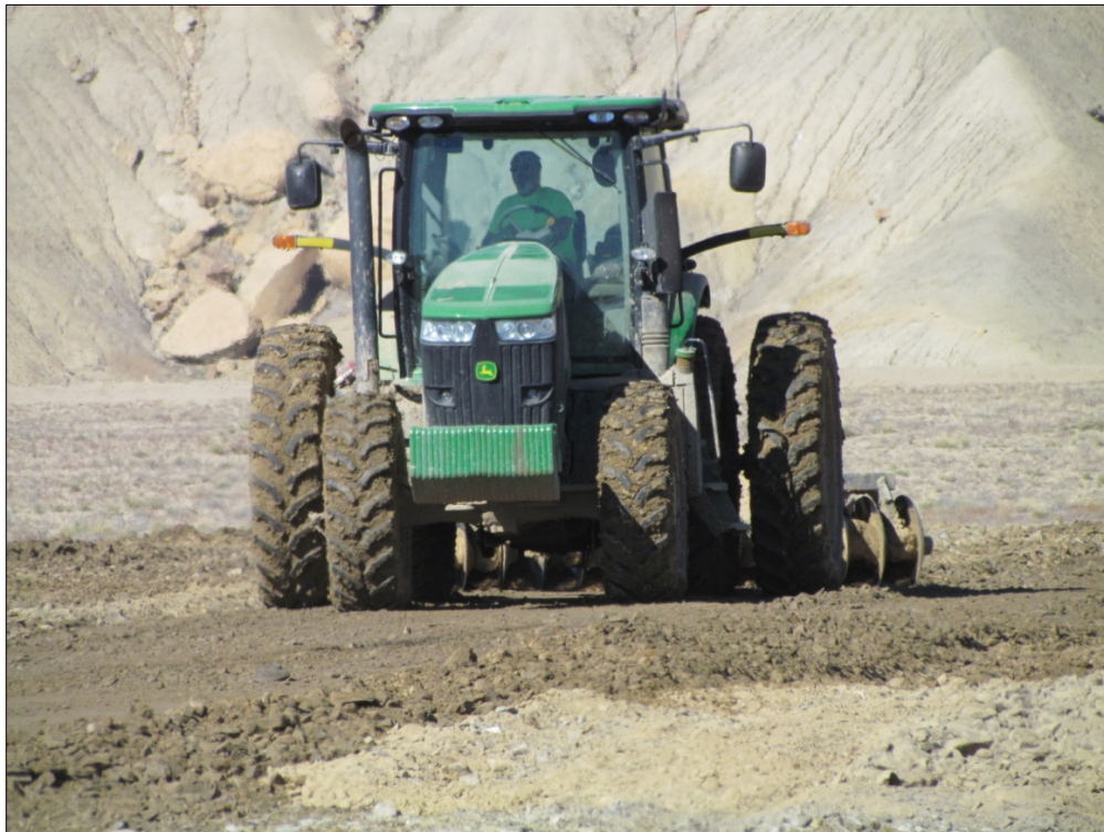
Photo 33. Frost Protection Layer Placement October 14, 2014
