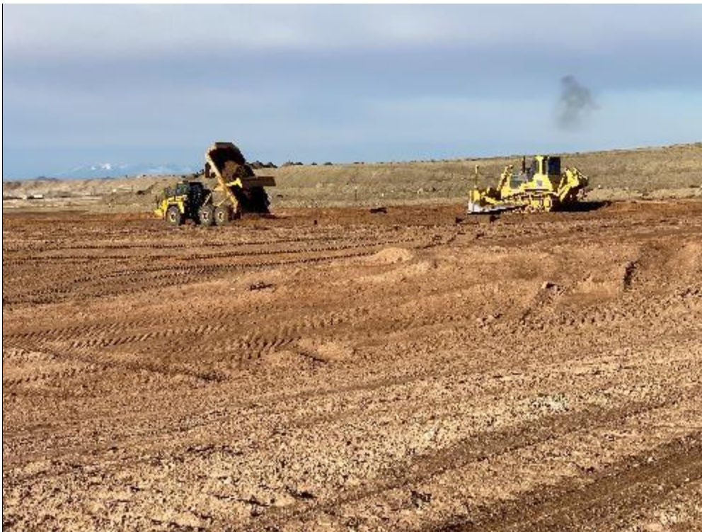
Photo 38. Debris Being Covered March 2021
