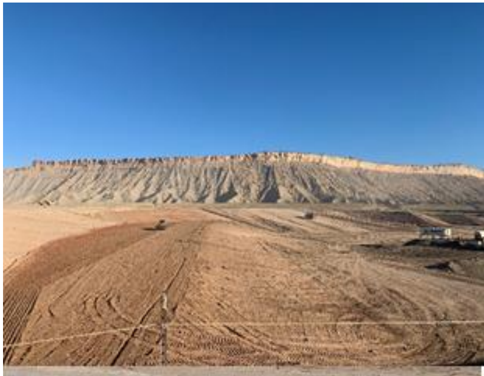
Photo 19. Placement of RRM October 2020
