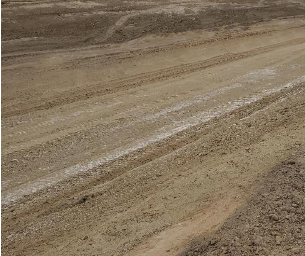
Photo 17. Completed Cell Excavation February 2021
