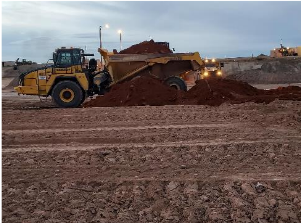
Photo 28. RRM Debris Lift December 2020
