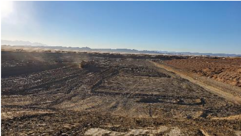
Photo 12. Cell Excavation December 2020
