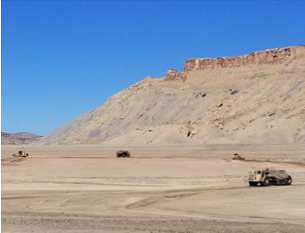
Photo 3. Phase 3 Cell Excavation October 2020
