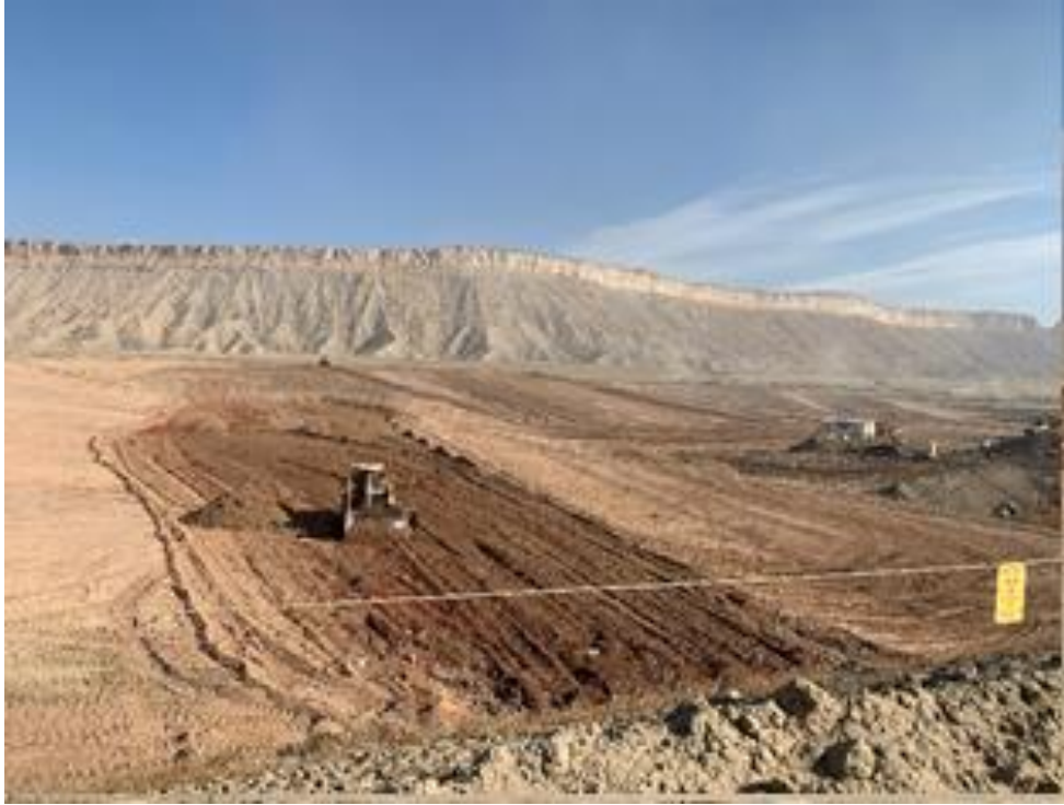
Photo 18. Dozer placing material October 2020
