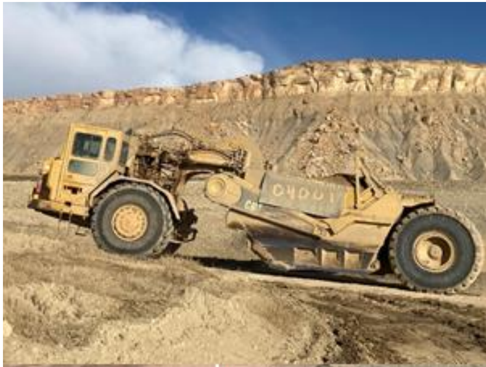
Photo 80. Scraper Hauling Spoils Embankment Material January 2021
