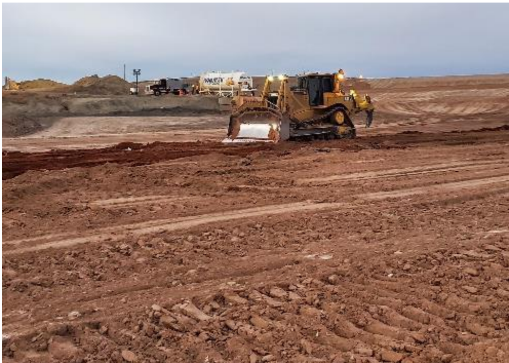
Photo 27. Placing a Debris Lift December 2020
