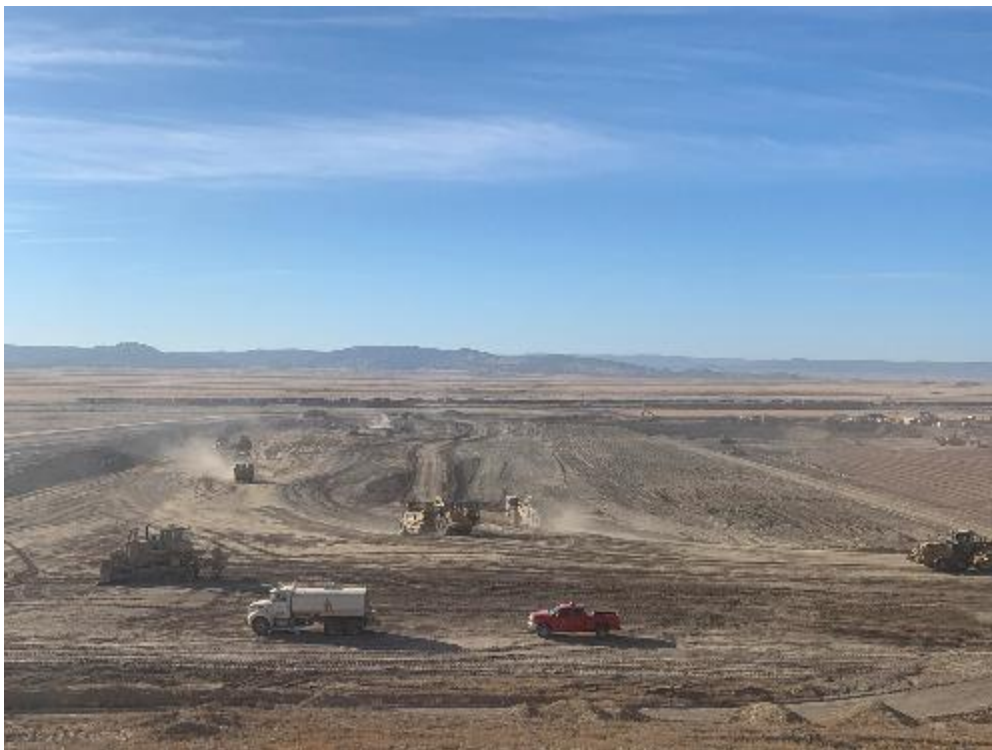
Photo 2. Phase 3 Cell Excavation October 2020
