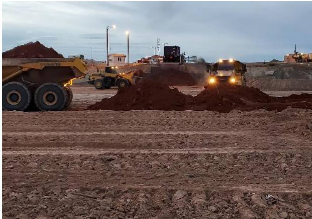
Photo 29. Material being placed December 2020
