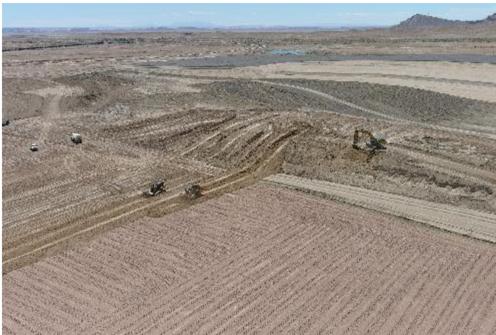
Photo 68. Pushing Out of the Stock Pile May 2021
