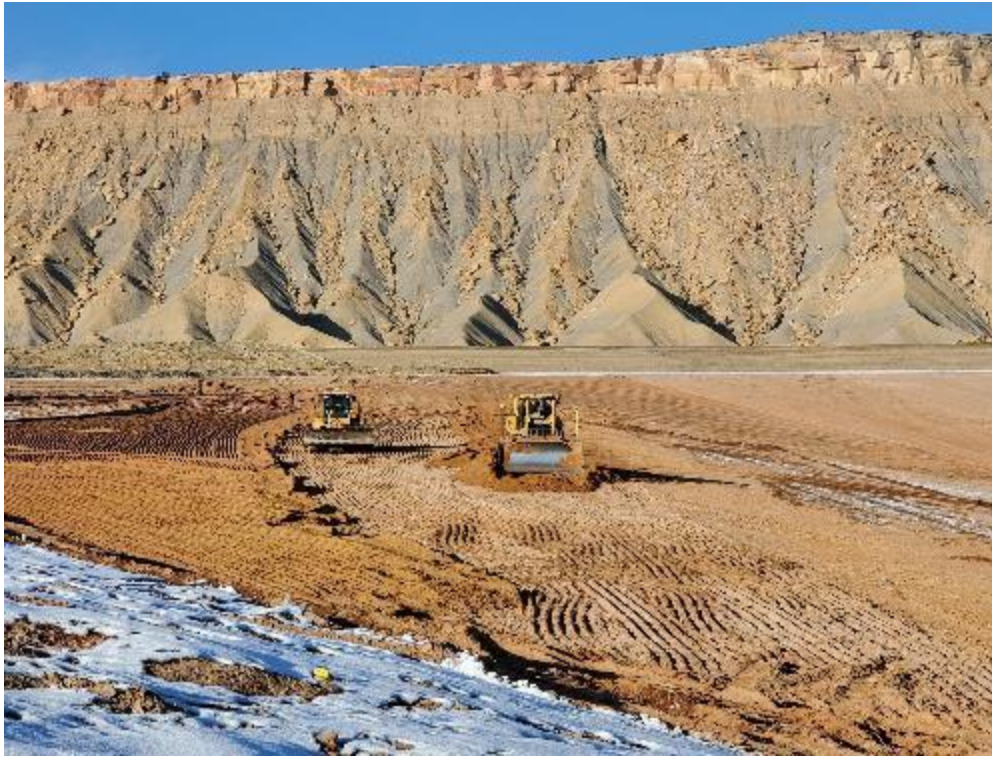
Photo 32. Equipment Placing RRM January 2021
