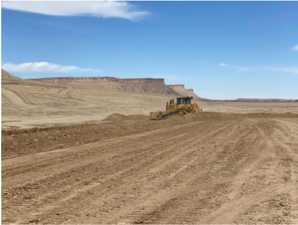
Photo 71. Dozer Pushing Interim Cover Material June 2021
