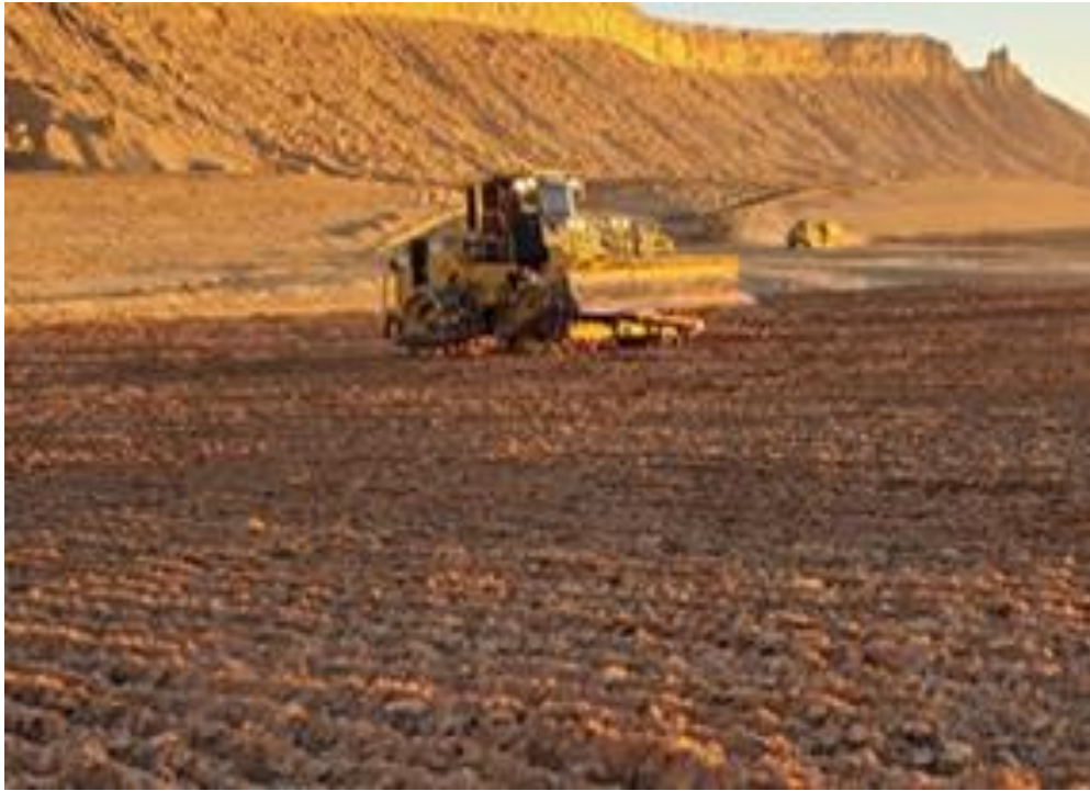
Photo 24. RRM Compaction December 2020
