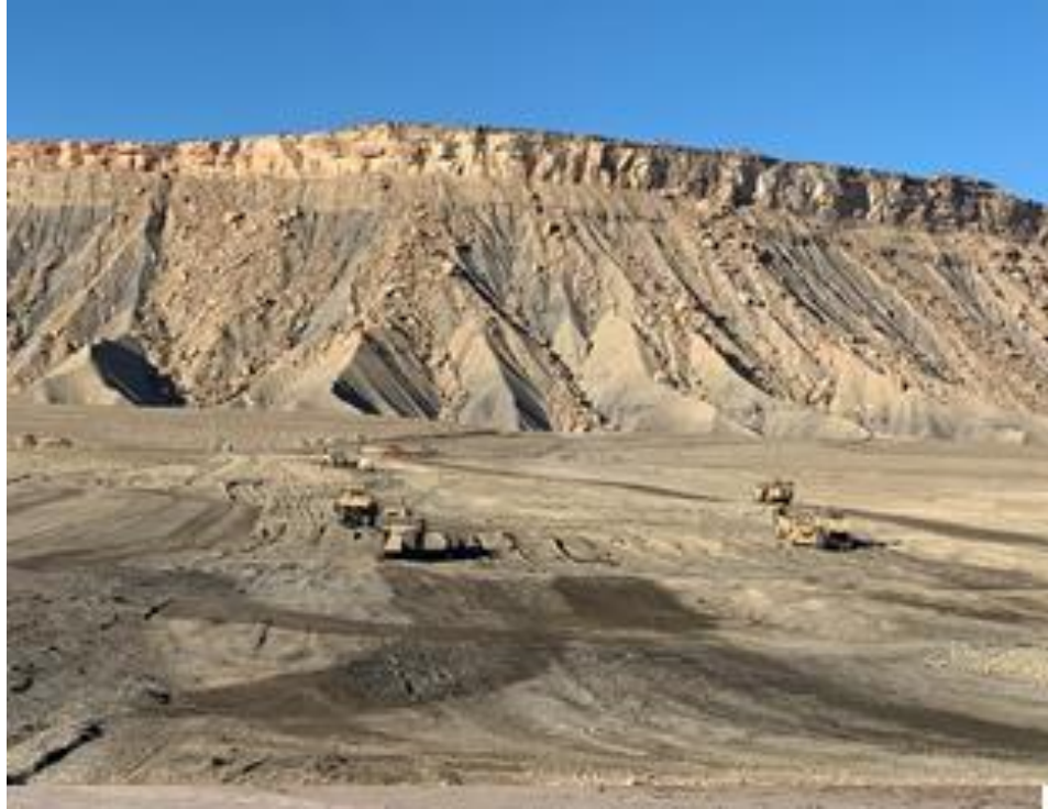
Photo 5. Cell Excavation November 2020
