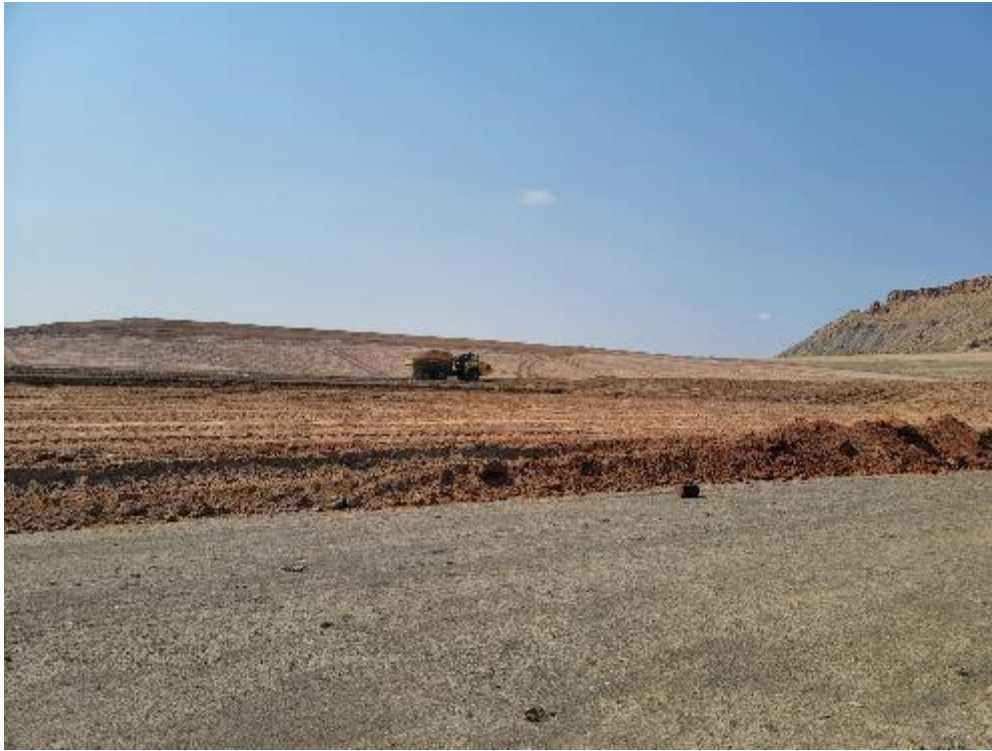
Photo 61. Placement of Debris Lift September 2021
