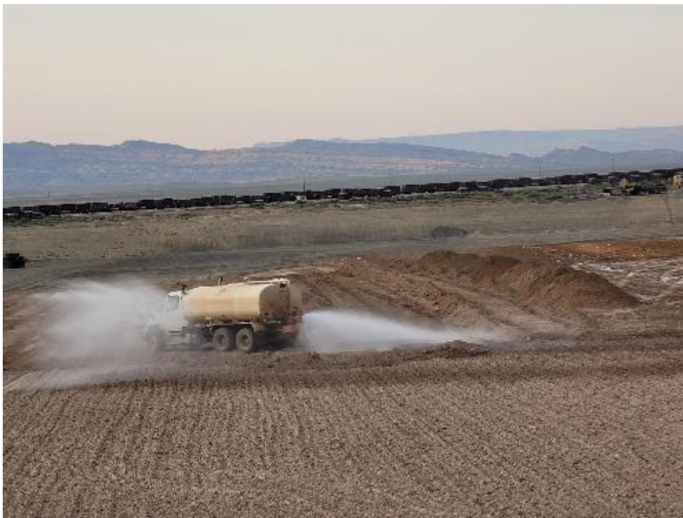
Photo 62. Dust Suppression and Moisture Conditioning September 2021
