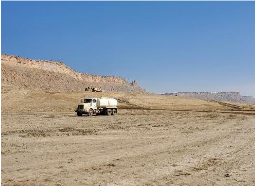
Photo 75. Spoils Embankment Construction October 2020
