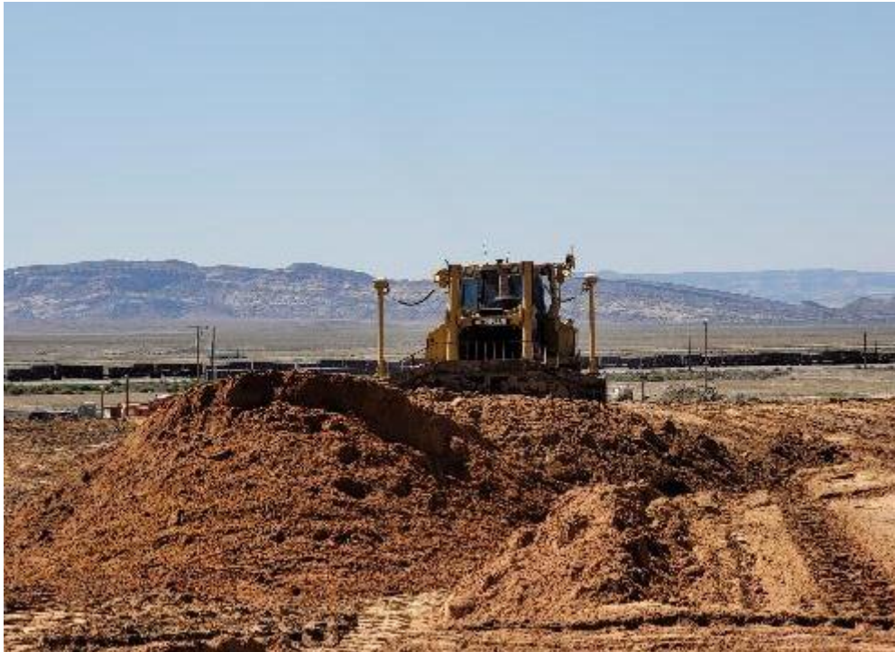
Photo 59. Dozer Pushing Material on RRM Lift August 2021
