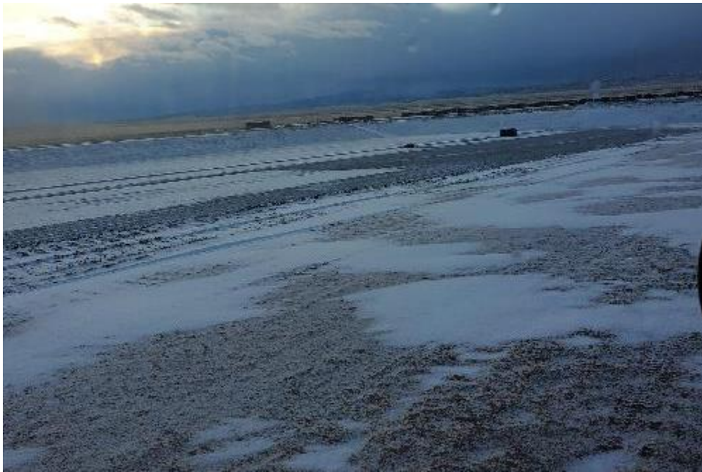
Photo 14. Cell Excavation January 2021
