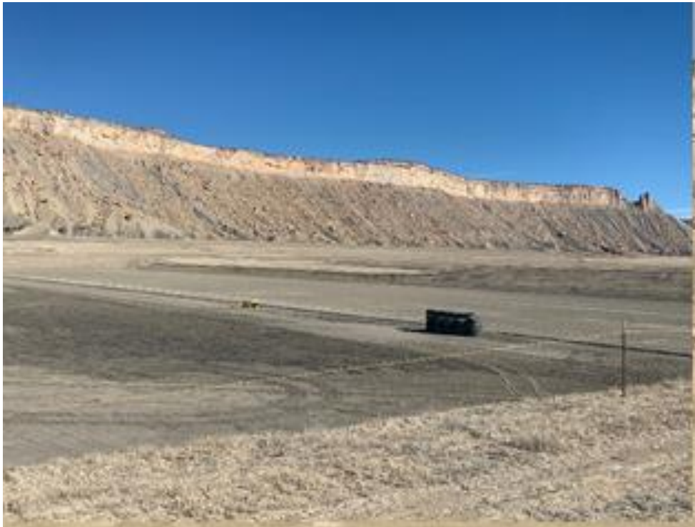
Photo 16. Cell Excavation February 2021
