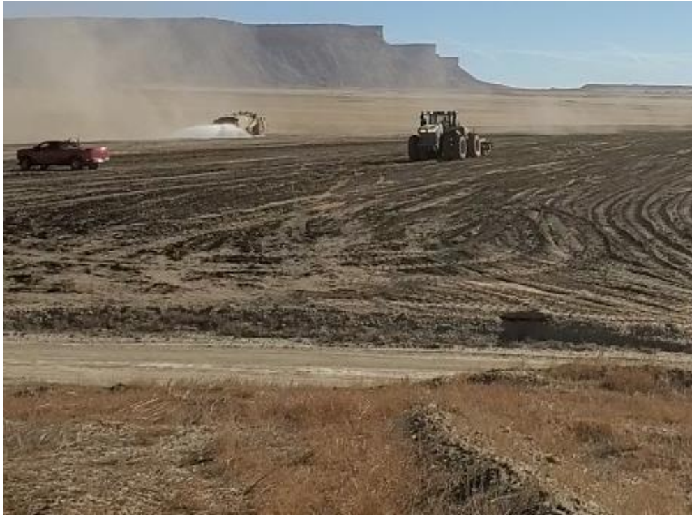
Photo 77. Constructing Spoils Embankment November 2020
