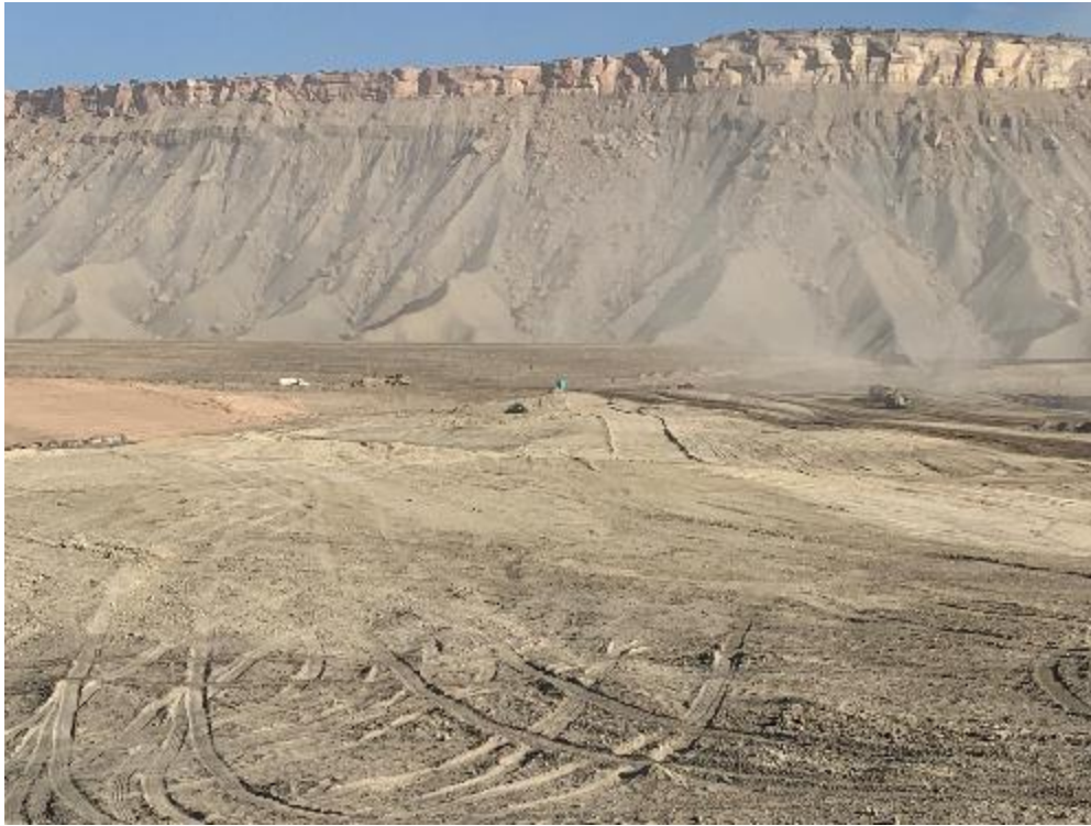
Photo 1. Phase 3 Cell Excavation October 2020
