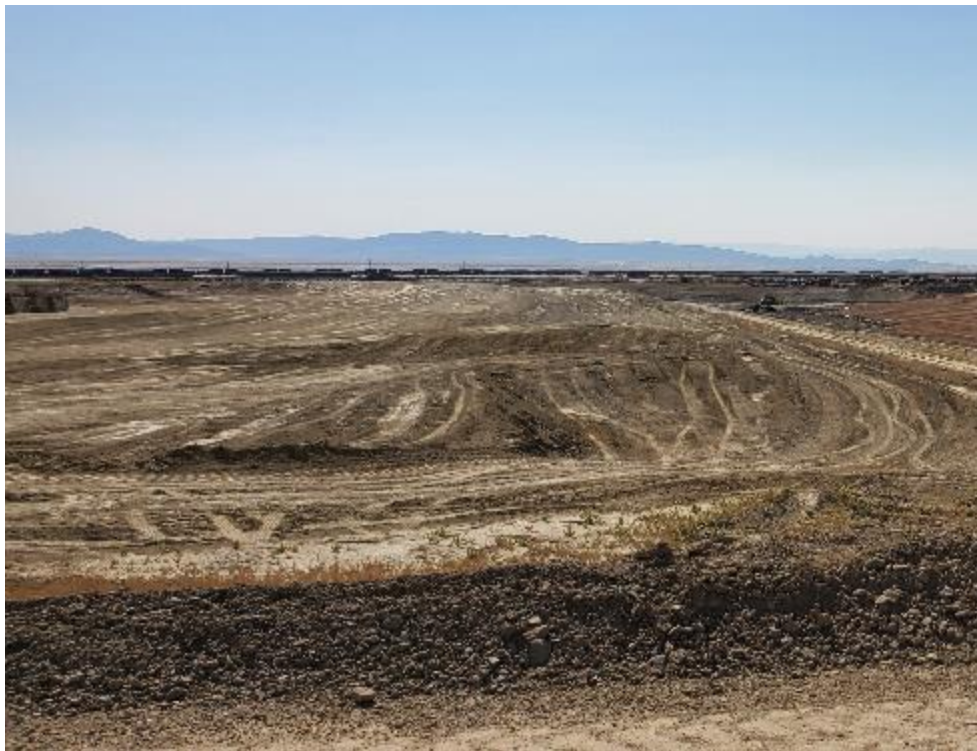
Photo 4. Phase 3 Cell Excavation October 2020
