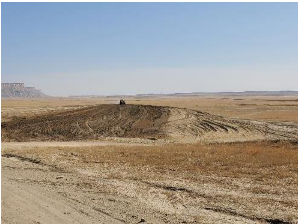
Photo 74. Placing Spoils Embankment Lift October 2020
