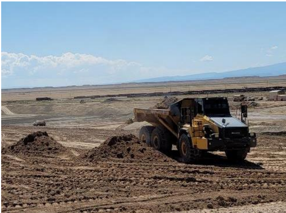
Photo 54. Hauling RRM for Placement July 2021
