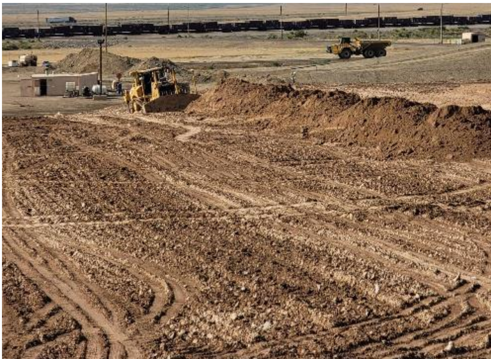
Photo 50. Dozer Placing RRM on Active Lift Area June 2021
