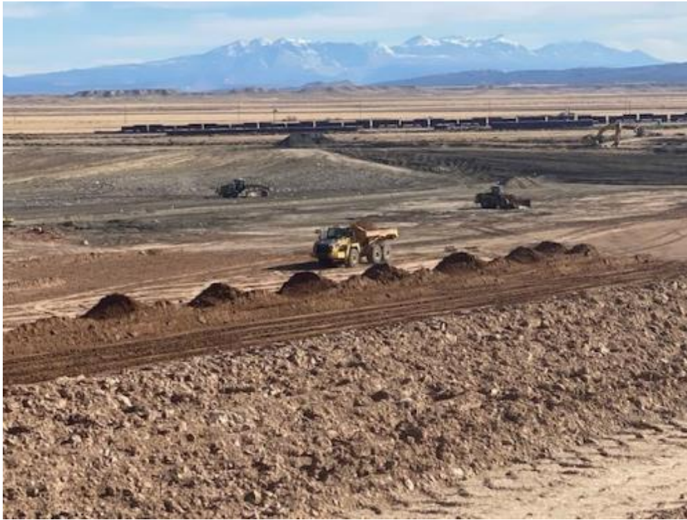
Photo 22. RRM ready for placement November 2020
