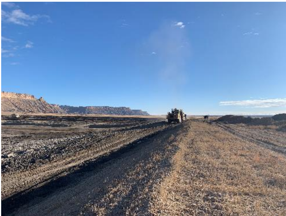
Photo 8. Cell Excavation November 2020
