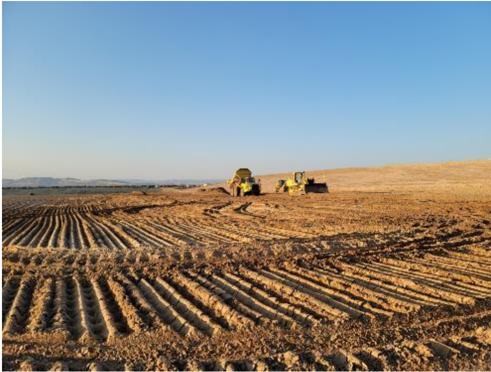
Photo 63. Pushing and Dumping RRM September 2021
