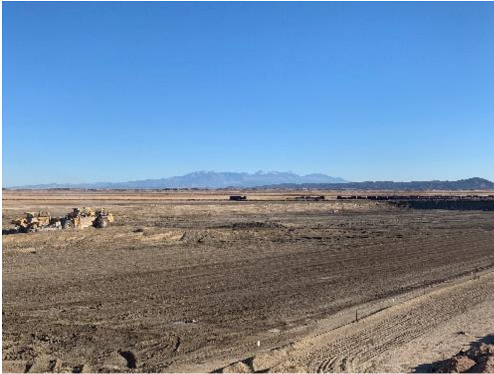
Photo 9. Cell Excavation December 2020
