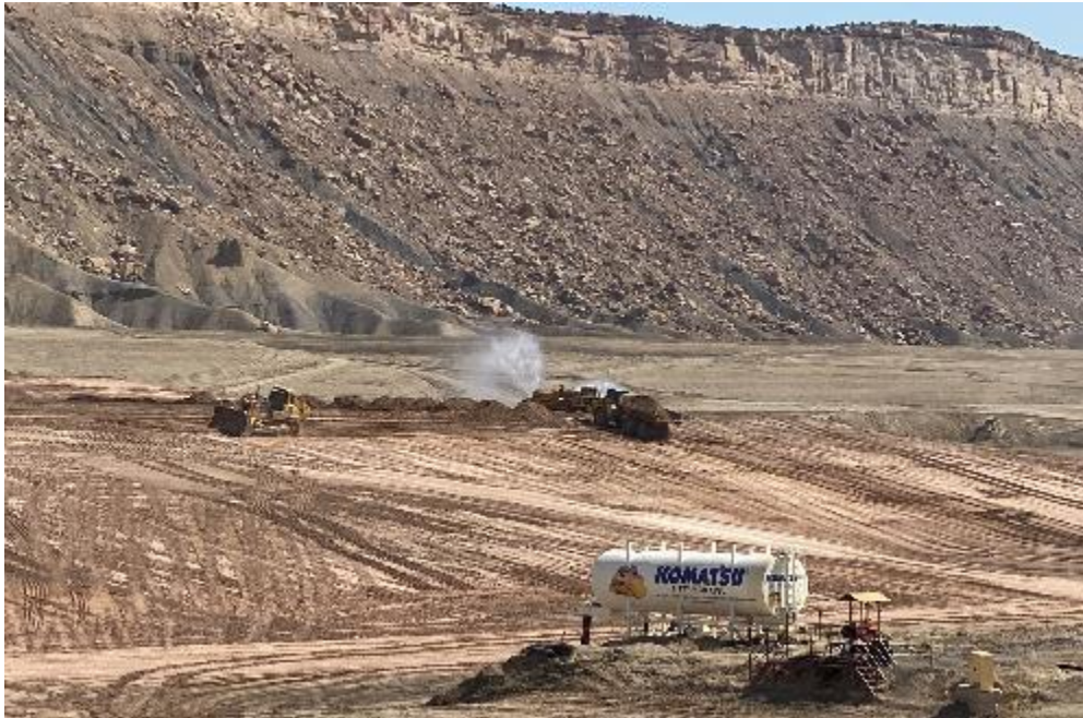
Photo 49. Placing RRM June 2021
