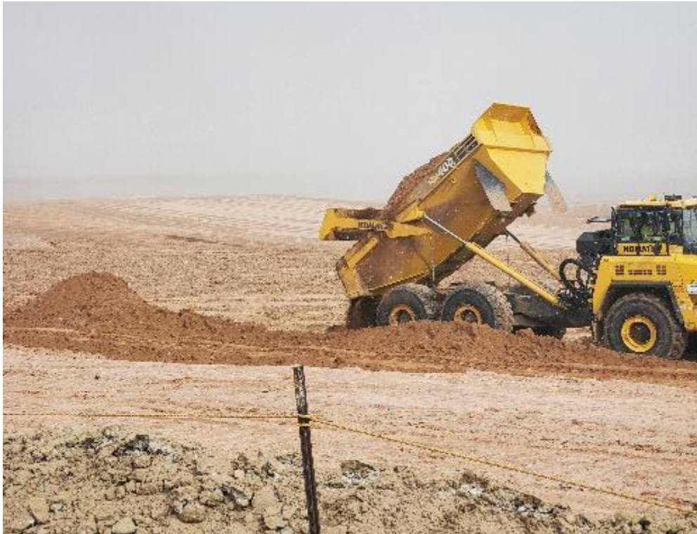
Photo 35. Soils Placement February 2021
