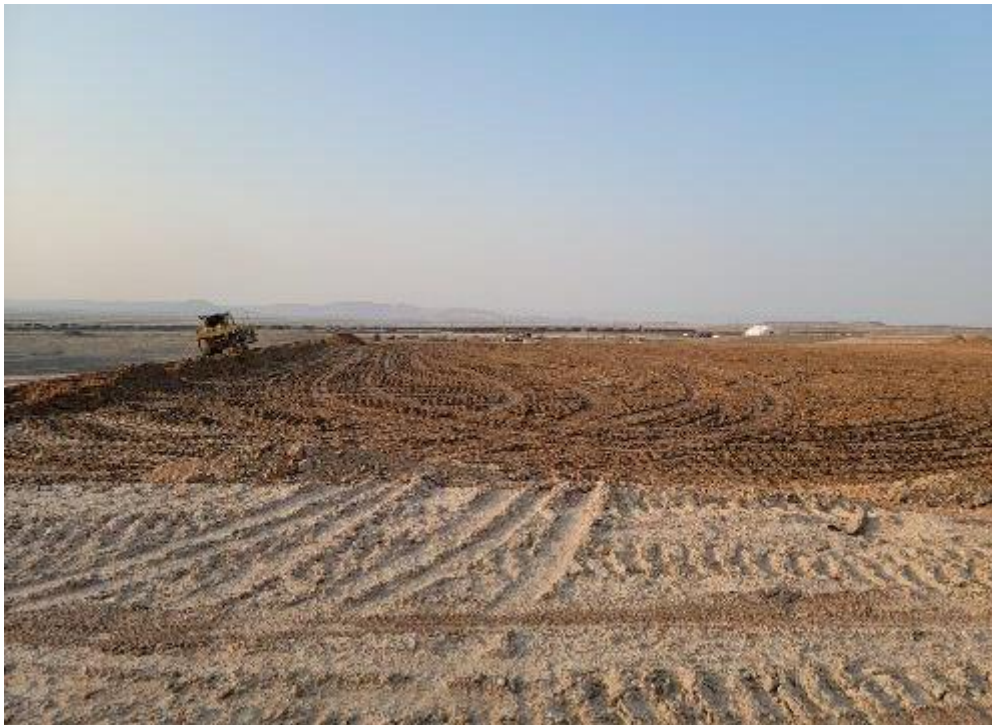
Photo 60. Looking South at the Disposal Cell August 2021
