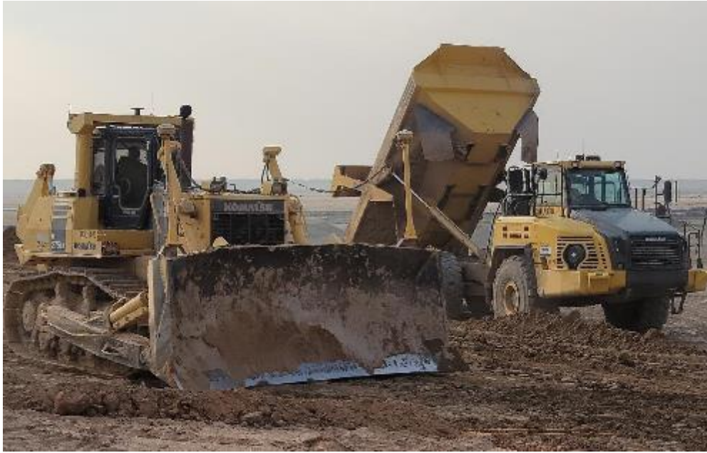
Photo 55. Equipment Preparing RRM Lift July 2021
