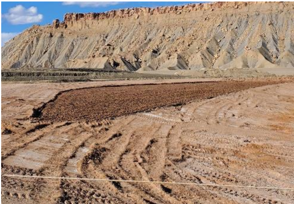
Photo 36. RRM Lift February 2021
