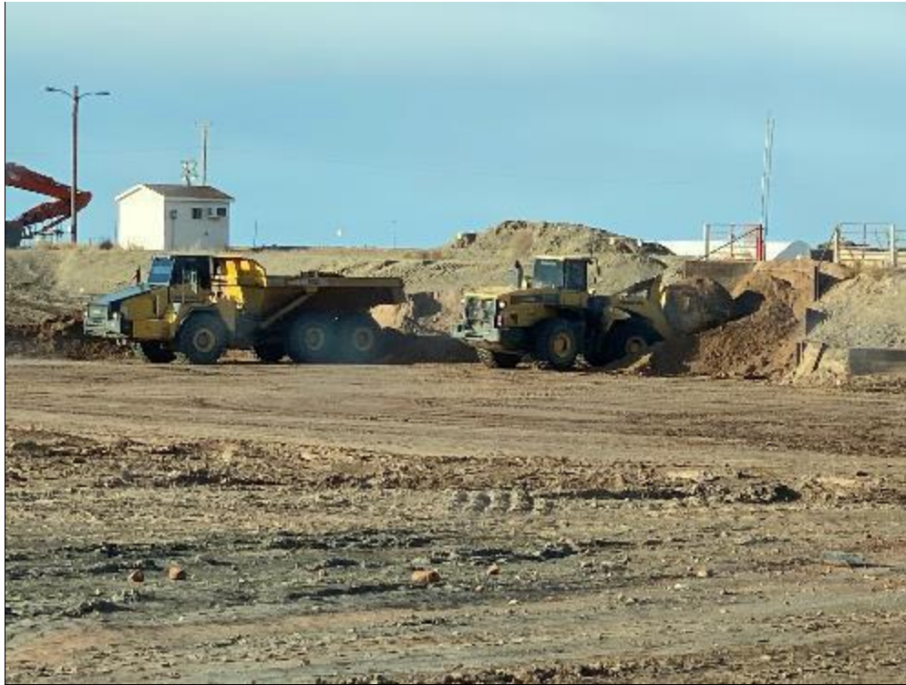
Photo 39. RRM Loadout March 2021
