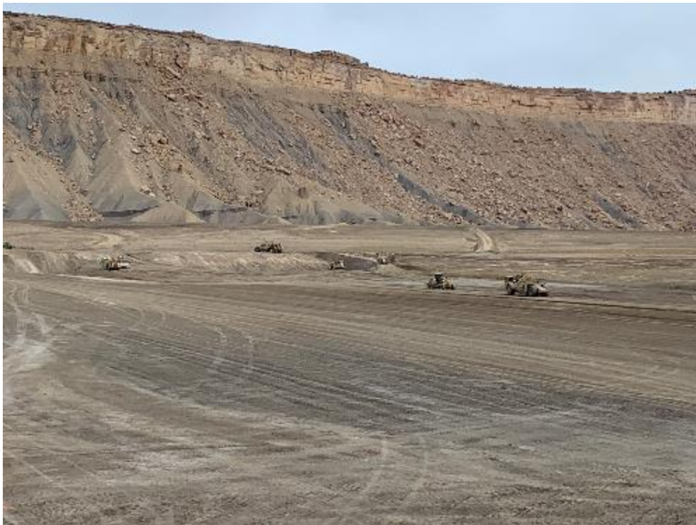
Photo 10. Cell Excavation December 2020
