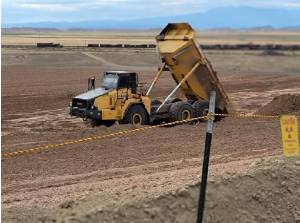
Photo 51. Haul Truck Dumping RRM of Lift Area June 2021
