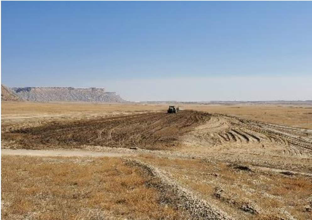
Photo 73. Constructing Spoils Embankment October 2020
