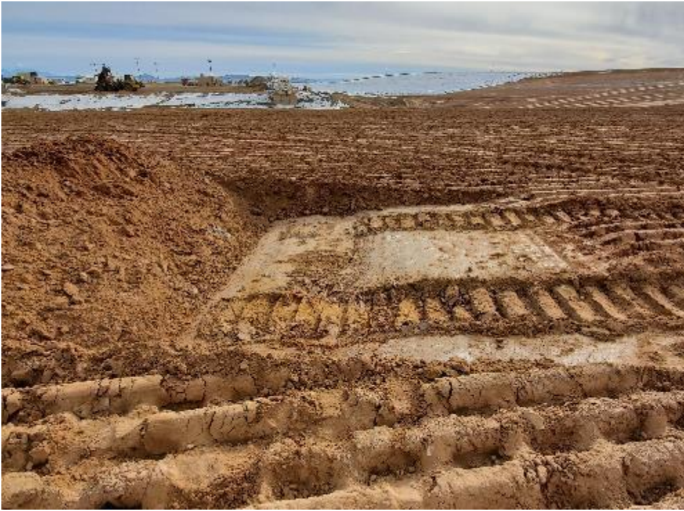
Photo 30. Lift Prepared for In-place Density Test January 2021
