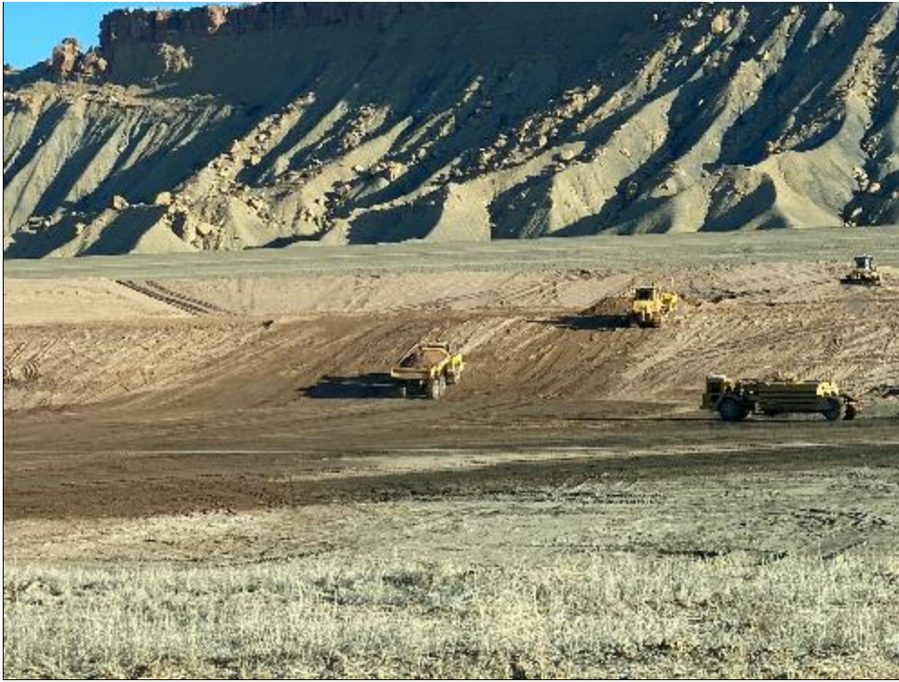
Photo 41. Hauling RRM for Placement April 2021
