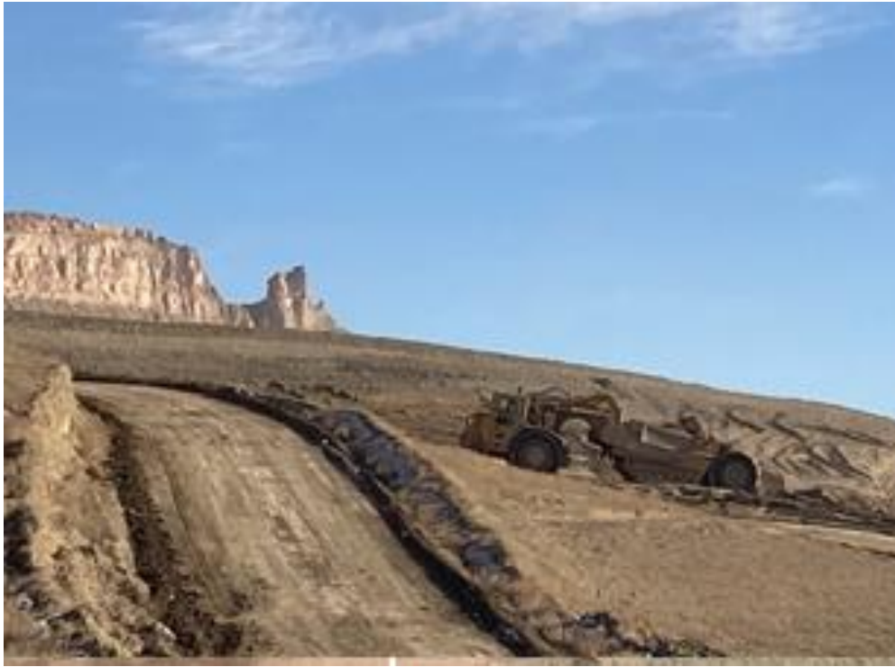
Photo 79. Transporting Material to Spoils Embankment January 2021
