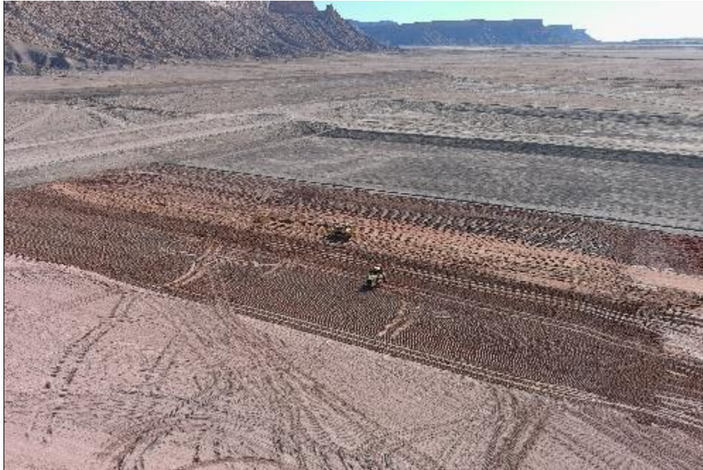
Photo 45. Aerial Photo of RRM being Placed May 2021
