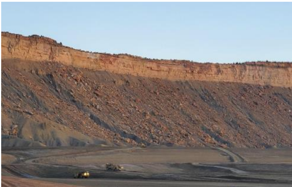
Photo 78. Transporting Material to Spoils Embankment December 2020
