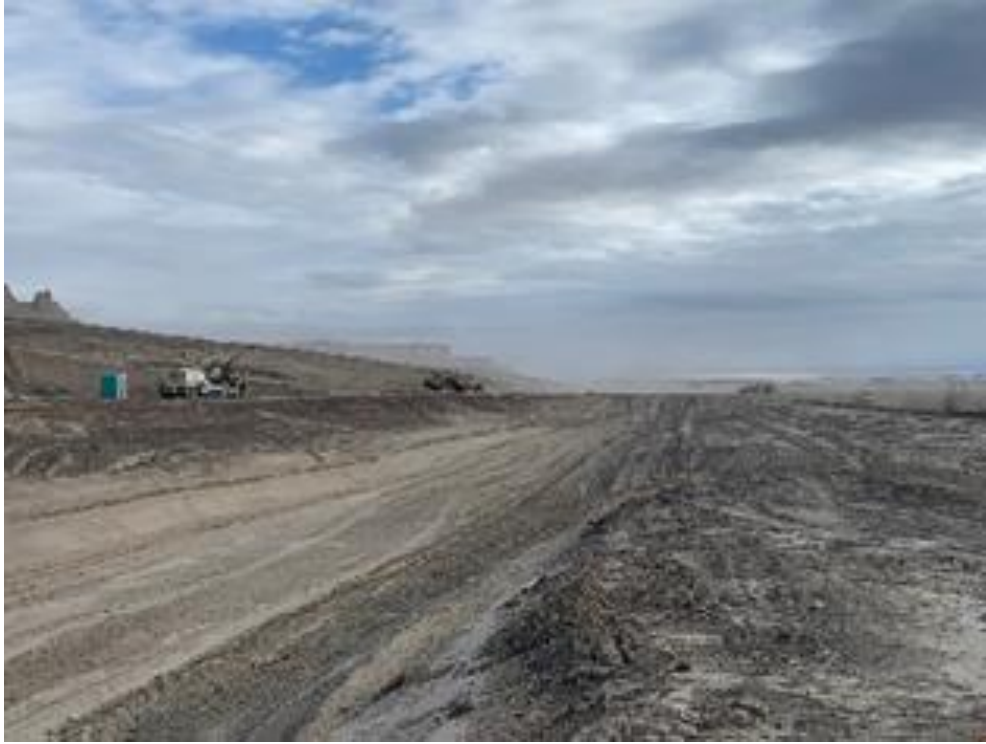
Photo 13. Cell Excavation January 2021
