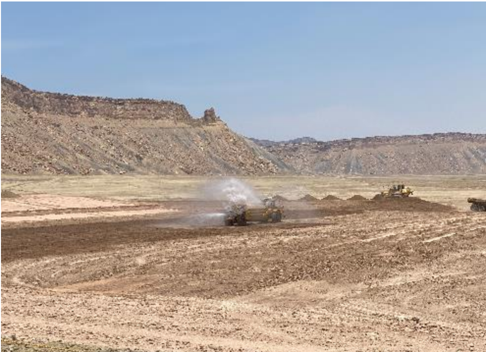
Photo 52. Watering Area for Dust Control June 2021
