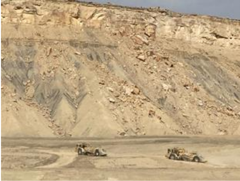
Photo 15. Cell Excavation February 2021
