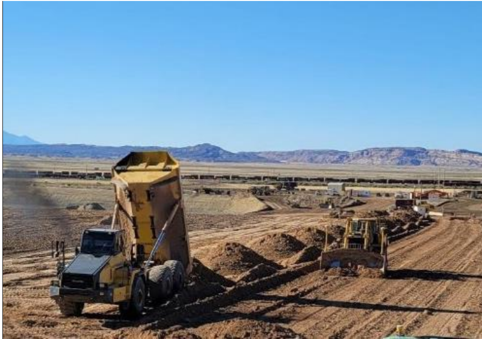
Photo 47. Placement of Material on Lift Area by Haul Truck May 2021
