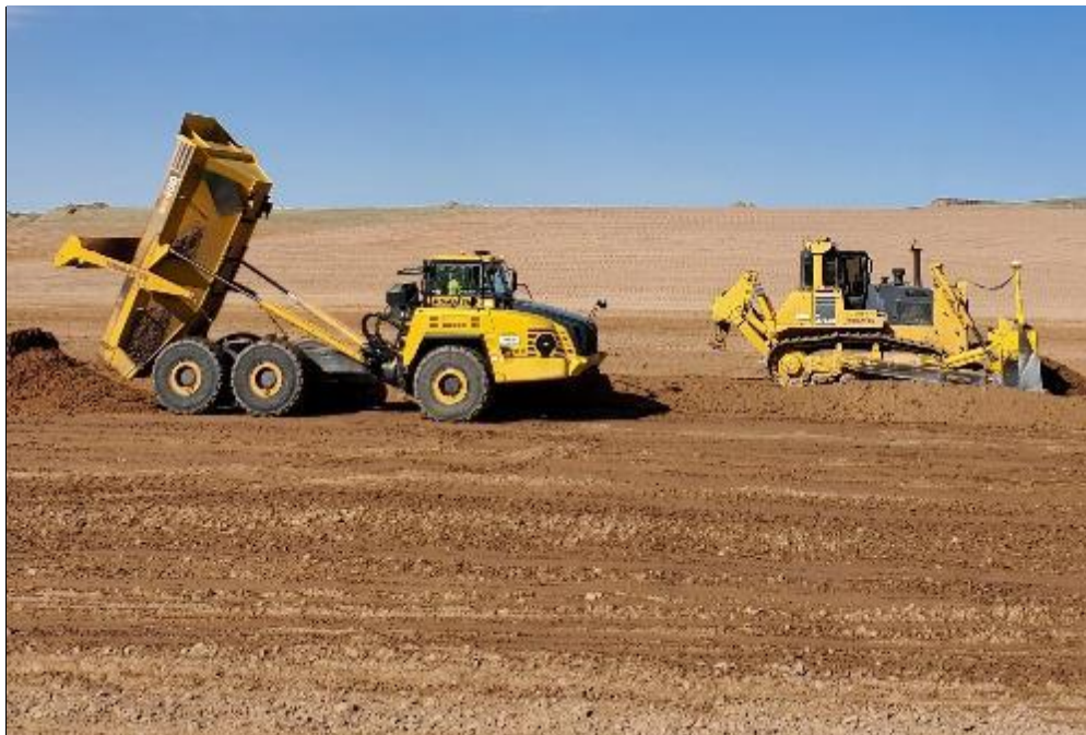
Photo 44. Equipment Placing RRM Material on Lift Area April 2021
