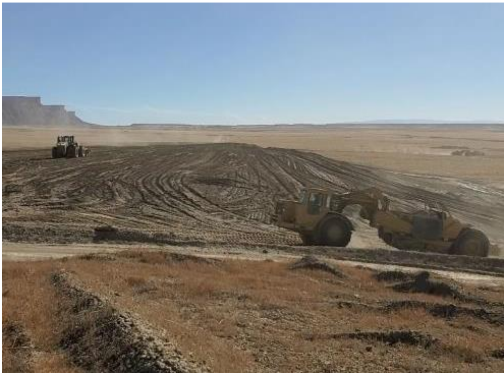
Photo 76. Hauling Material for Placement on Spoils Embankment November 2020
