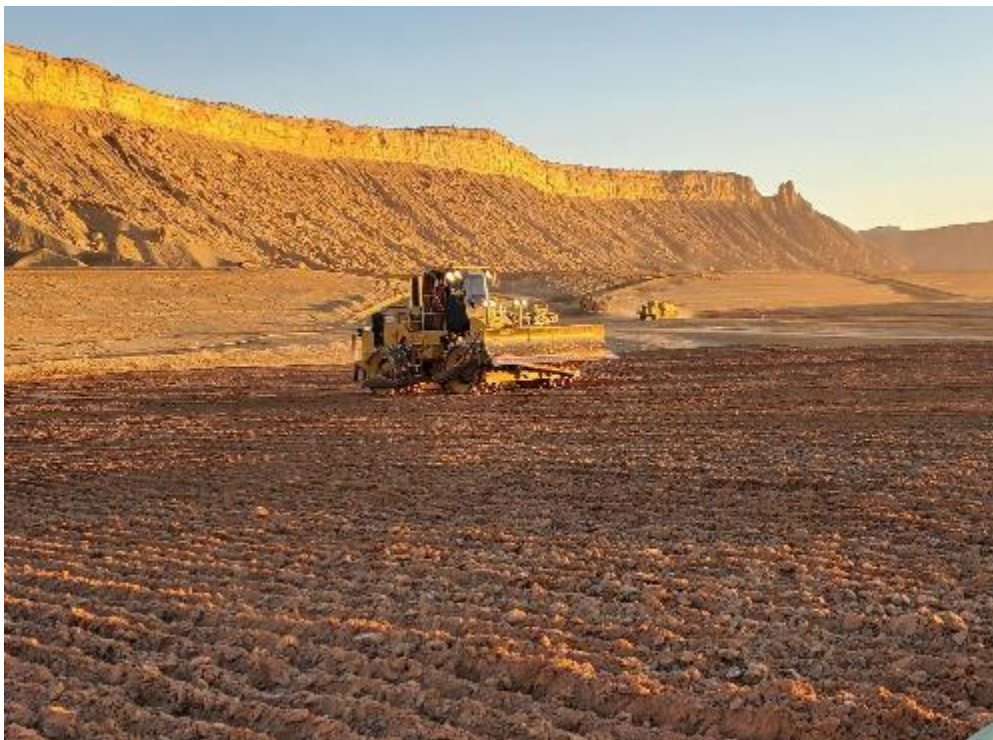
Photo 25. Breaking up Frost December 2020
