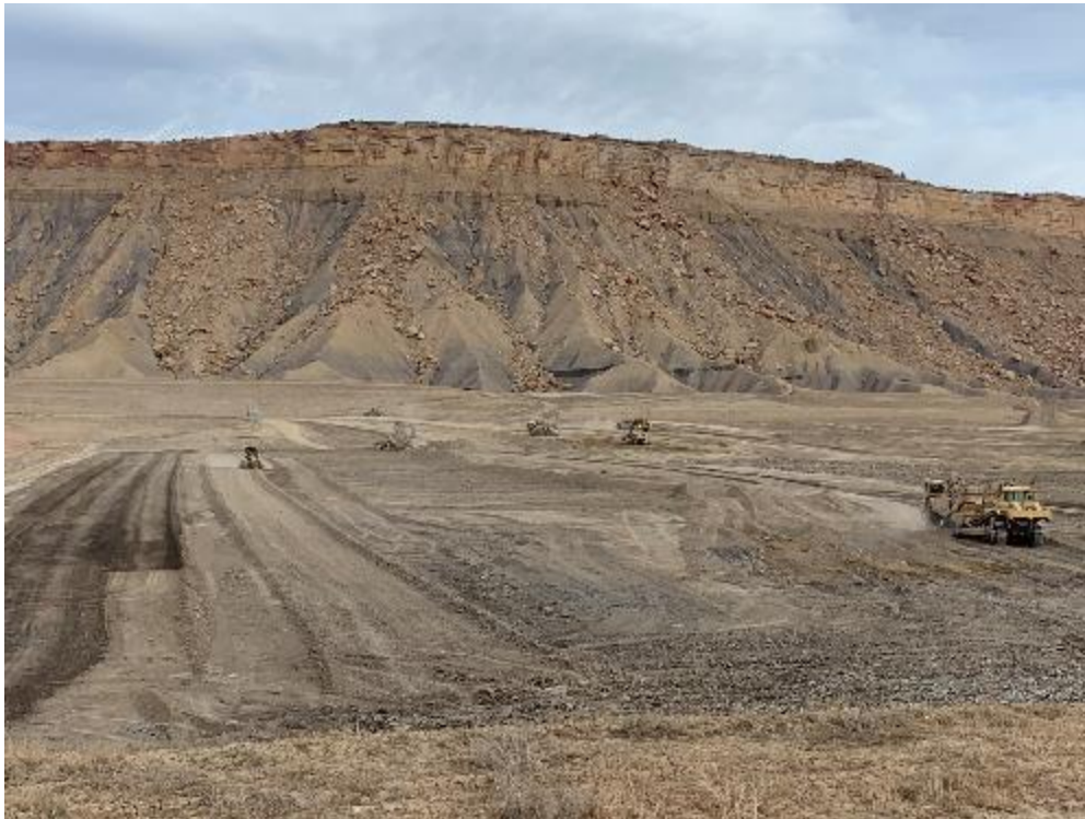
Photo 6. Cell Excavation November 2020
