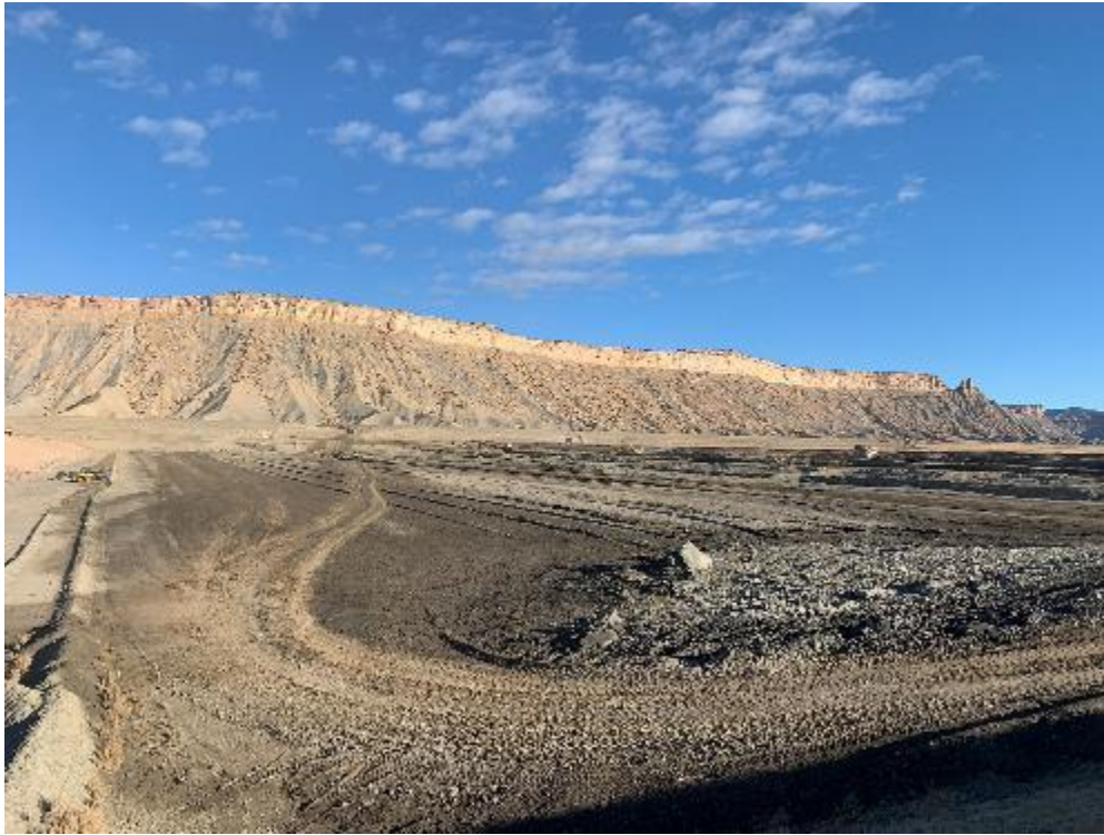
Photo 7. Cell Excavation November 2020
