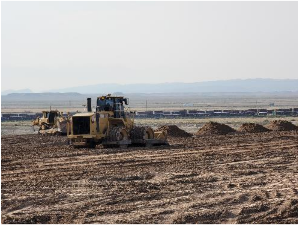
Photo 57. Compaction of 4 th RRM Lift in Top 7 Feet August 2021
