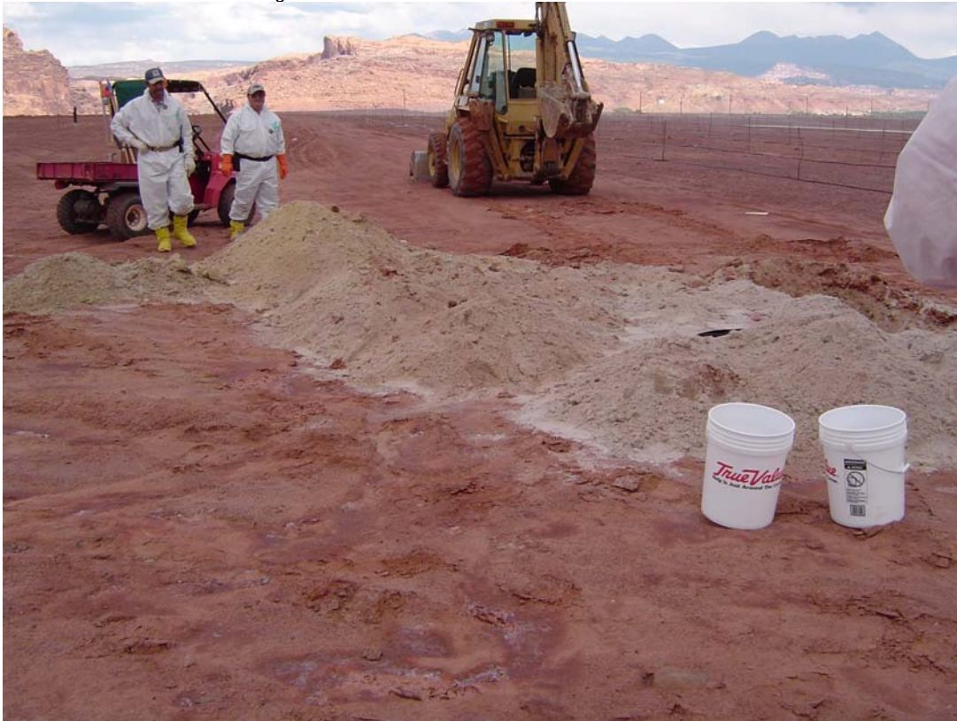
2. Photo of GATP-02 cuttings on the ground surface.
