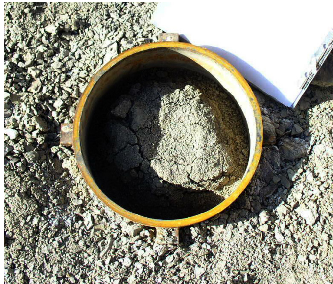
Figure 6. Channel Along Ring Exterior Filled with Spoils Prior to Testing
