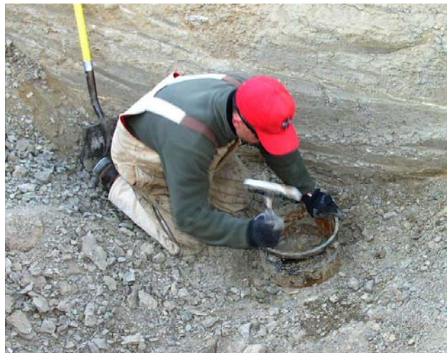
Figure 2. Excavating Circular Channel into Weathered Mancos Shale to Place AEP Ring
