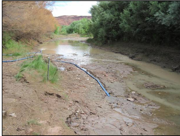
Photo D-9. CF4 Channel; Initial Action Diverting Water Through Gravel Bar (view to north)
