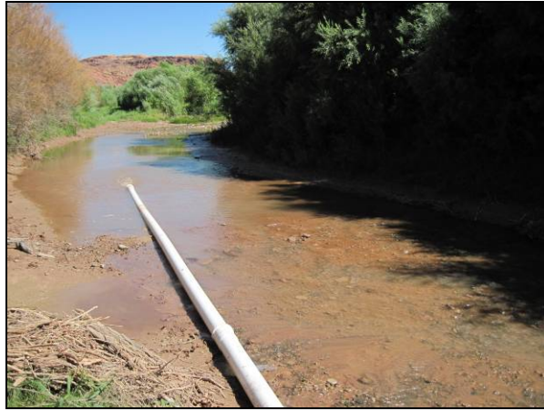
Photo D-16. CF4 Channel With Initial Action Piping (view to north)
