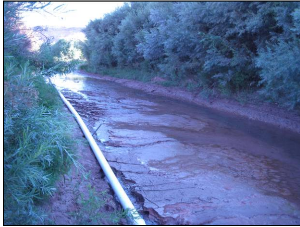
Photo D-18. CF4 Channel With Initial Action Piping (view to north)
