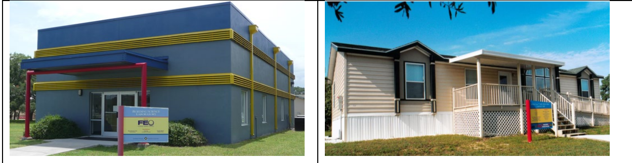
Figure C-1. Pilot System A was installed in the Manufactured Housing Lab (right) and Pilot System C was installed in the Building Science Lab (left).
