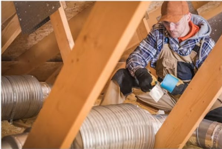
Duct Sealing
