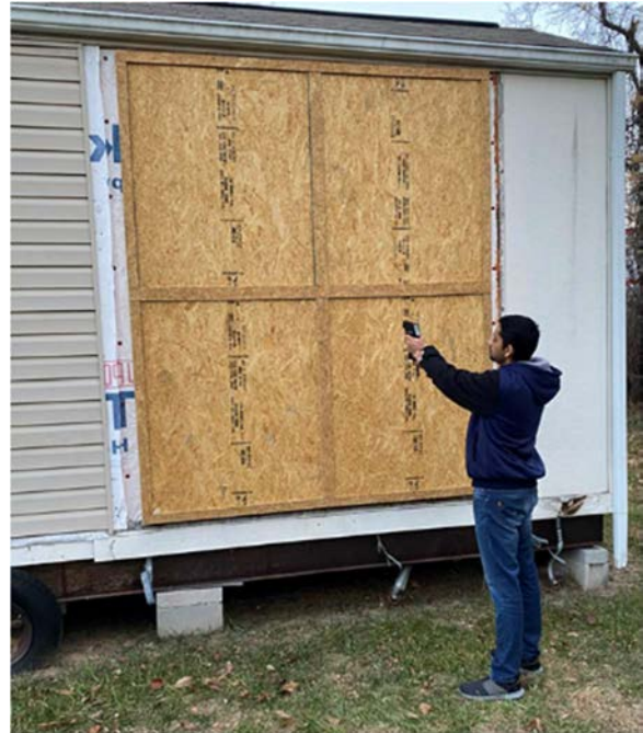
Figure 38: Thermal imaging should be the final quality inspection of the installation
