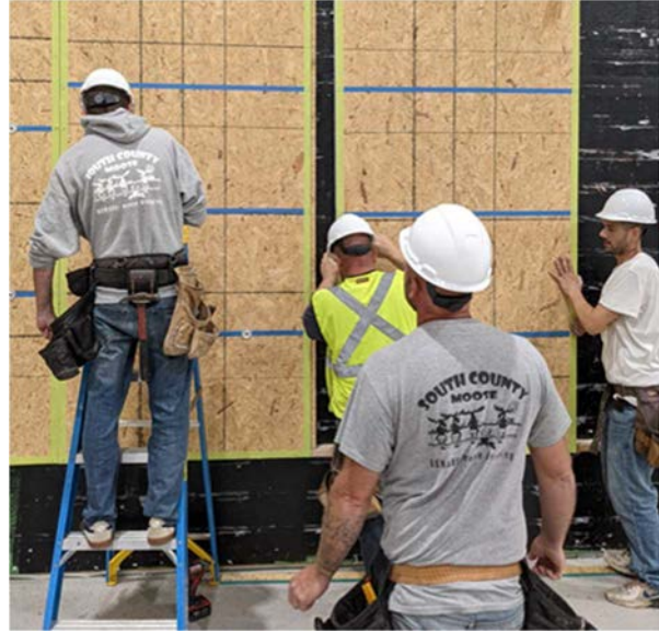
Figure 34: Installation of Mock-Up Panels
