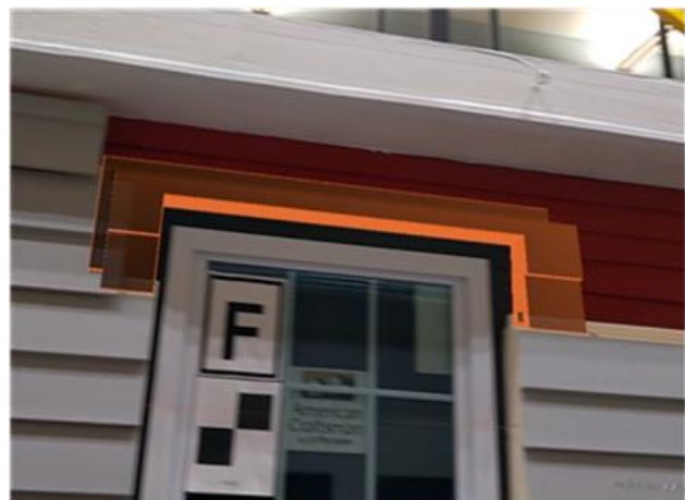
Figure 16: AR highlights for the worker the next PB to install and, when prompted, shows where to install it (note: the PB highlighted on pallet differs from that projected on the wall).
