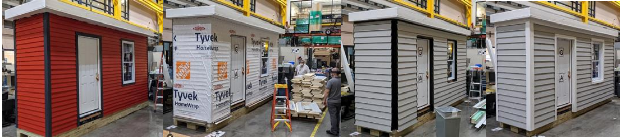
Figure 2: Complete installation of the PB system on the mock-up wall.
