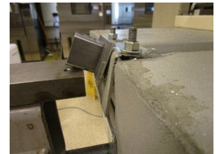
6B FIC Flexural Test Failure Mode Detail
