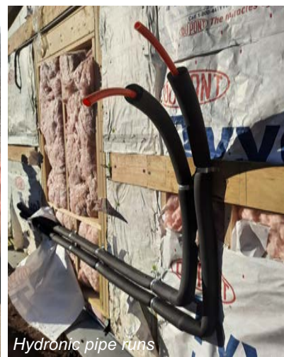
Panel fit test. Note: Wood ledgers designed for BEST facility test only; not intended for future implementation.
