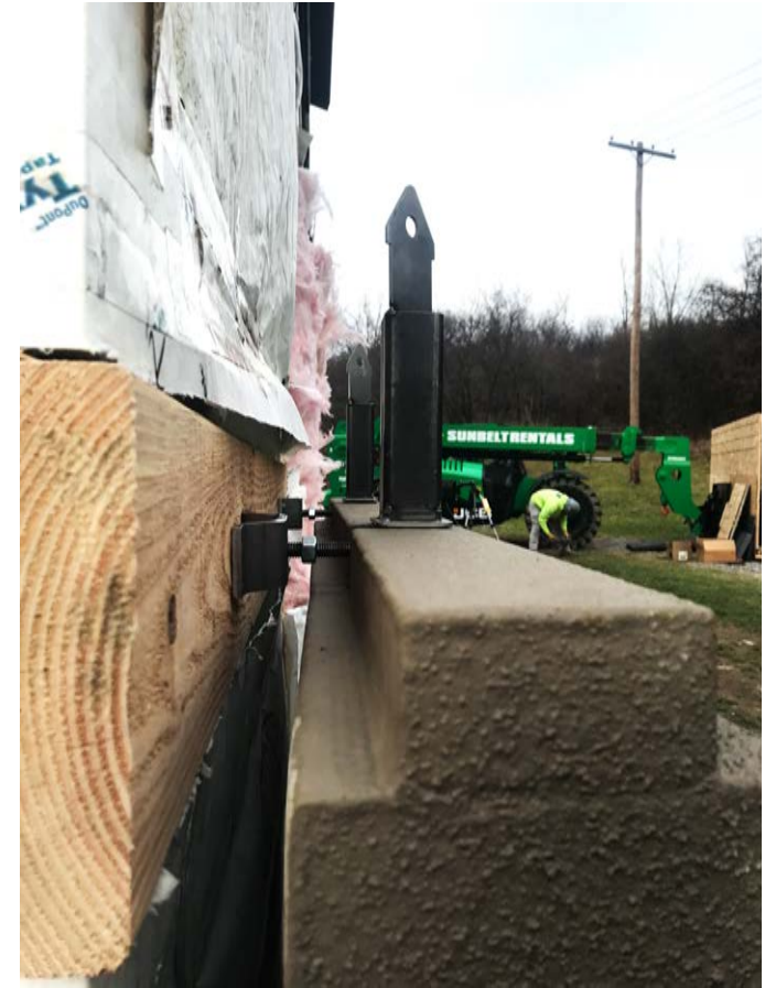
Full-scale prototype installation partial mock-up showing service cavity and adjustable attachment system.
