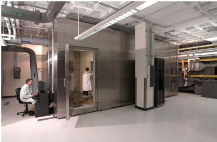
Building Energy and Environmental Systems Laboratory (BEESL), Syracuse University
