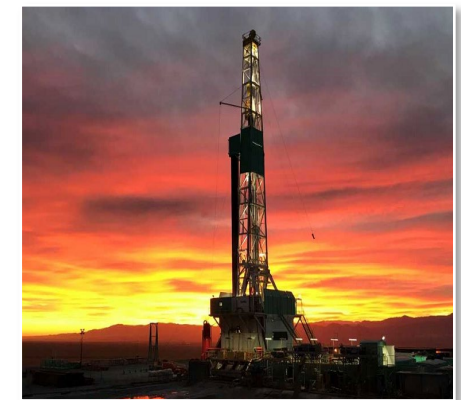
A drilling rig at the FORGE site outside of Milford, Utah
