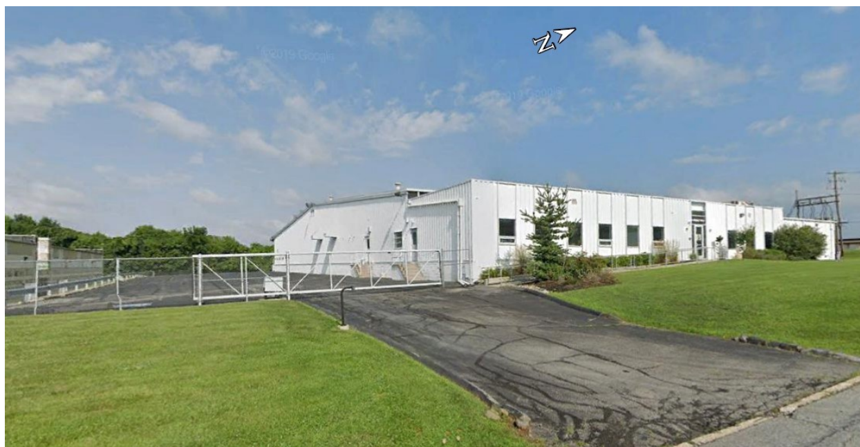
Figure 2-7 Bethlehem Apparatus Building 945 (foreground) and Building 935 (rear left)
