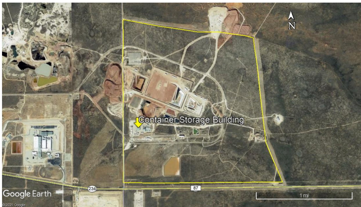
Figure 3-2 Aerial View of WCS Container Storage Building
