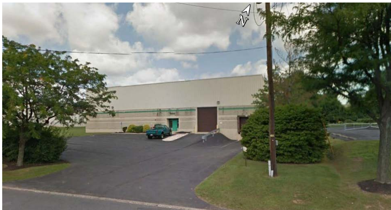
Figure 2-8 Bethlehem Apparatus Building 1055
