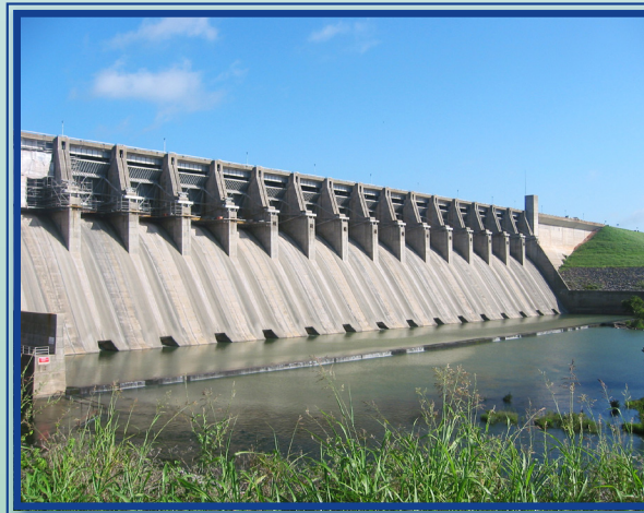
Whitney Dam was fully rehabilitated using $32 million in customer funding, resulting in an uprate of 13 MW.
