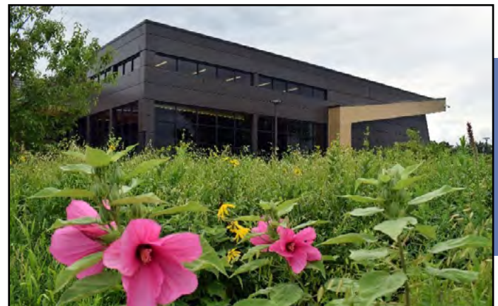
New Weldon Spring Site Interpretive Center near St. Charles, Missouri.
