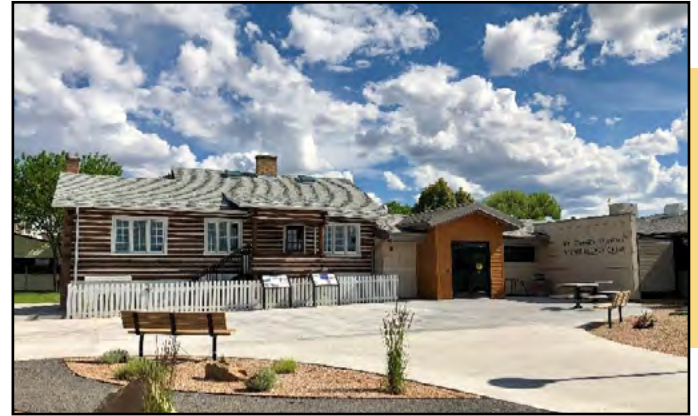
Atomic Legacy Cabin in Grand Junction, Colorado.
