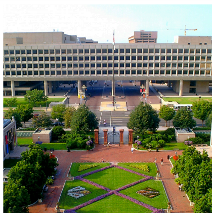
DOE's Forrestal Building in Washington, D.C.
