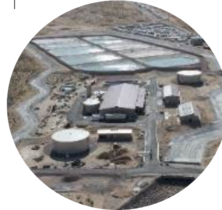
Ft. Irwin, CA Water Treatment Plant (MILCON)
