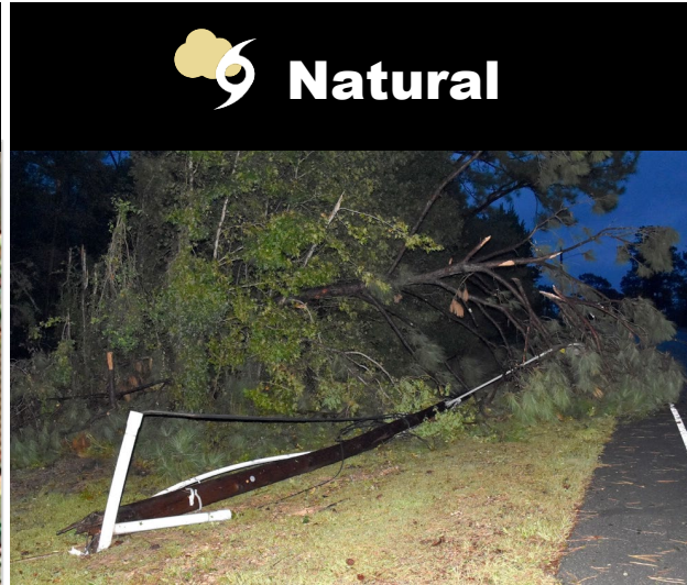
Power lines knocked down during Hurricane Delta, October 2020, Ft Polk, LA
