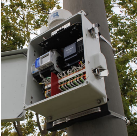
FIGURE 27. INSTALLATION OF A MICRO-SYNCHROPHASOR ON A DISTRIBUTION POLE (SOURCE: ARPA-E)
