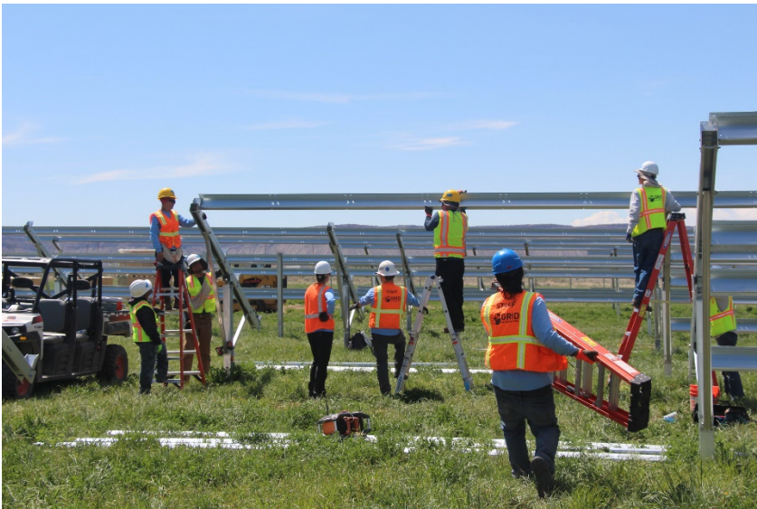
Interns, Grid Employees and Volunteers during construction
