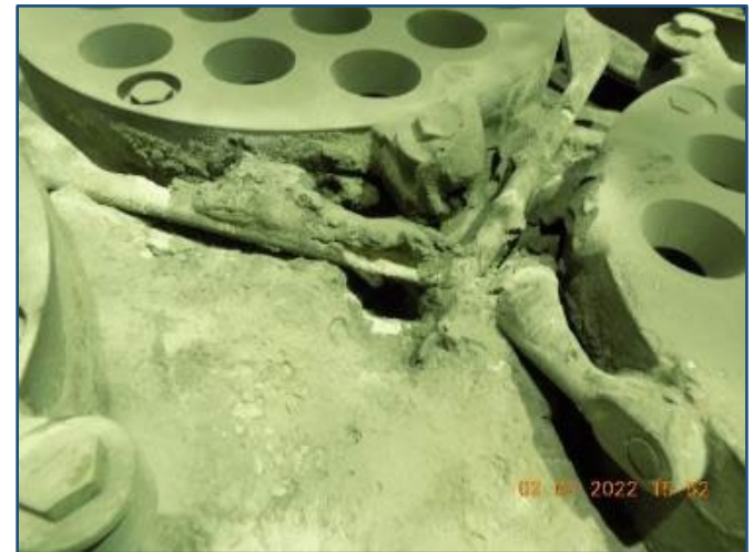
Closeup of carbonate accumulation on tube sheet near bundle #18
