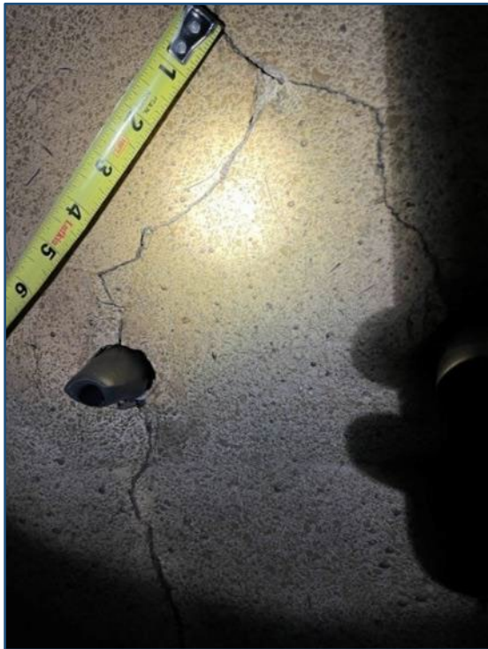
Shallow cracks in refractory
