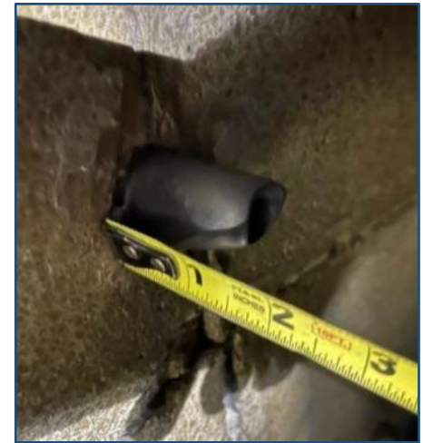
Eroded CRR piping penetration
