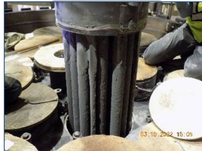
PGF bundles relatively clean with no bridging/excessive material build up indicating effective blowbacks
