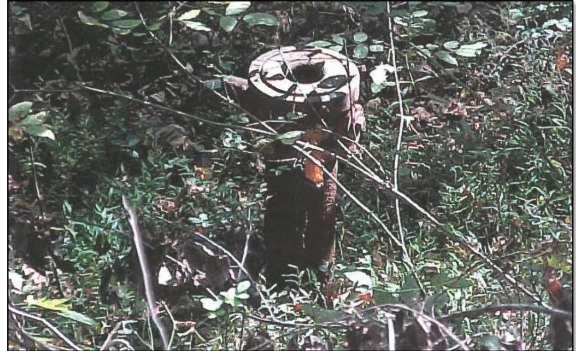
Orphaned well in Kanawha County, West Virginia – October 2005 (West Virginia Surface Owners' Rights Association, 2018)
