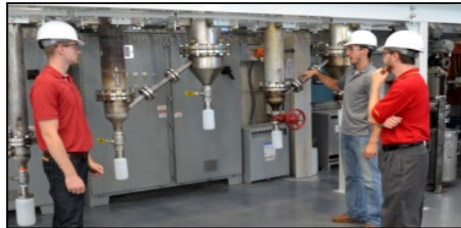
Autothermal pyrolysis pilot plant (15-20 kg/h) supported design of demonstration plant
