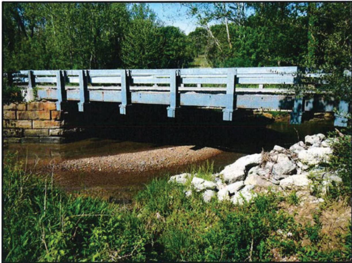
Photo 1 – Elevation view looking southeast.
