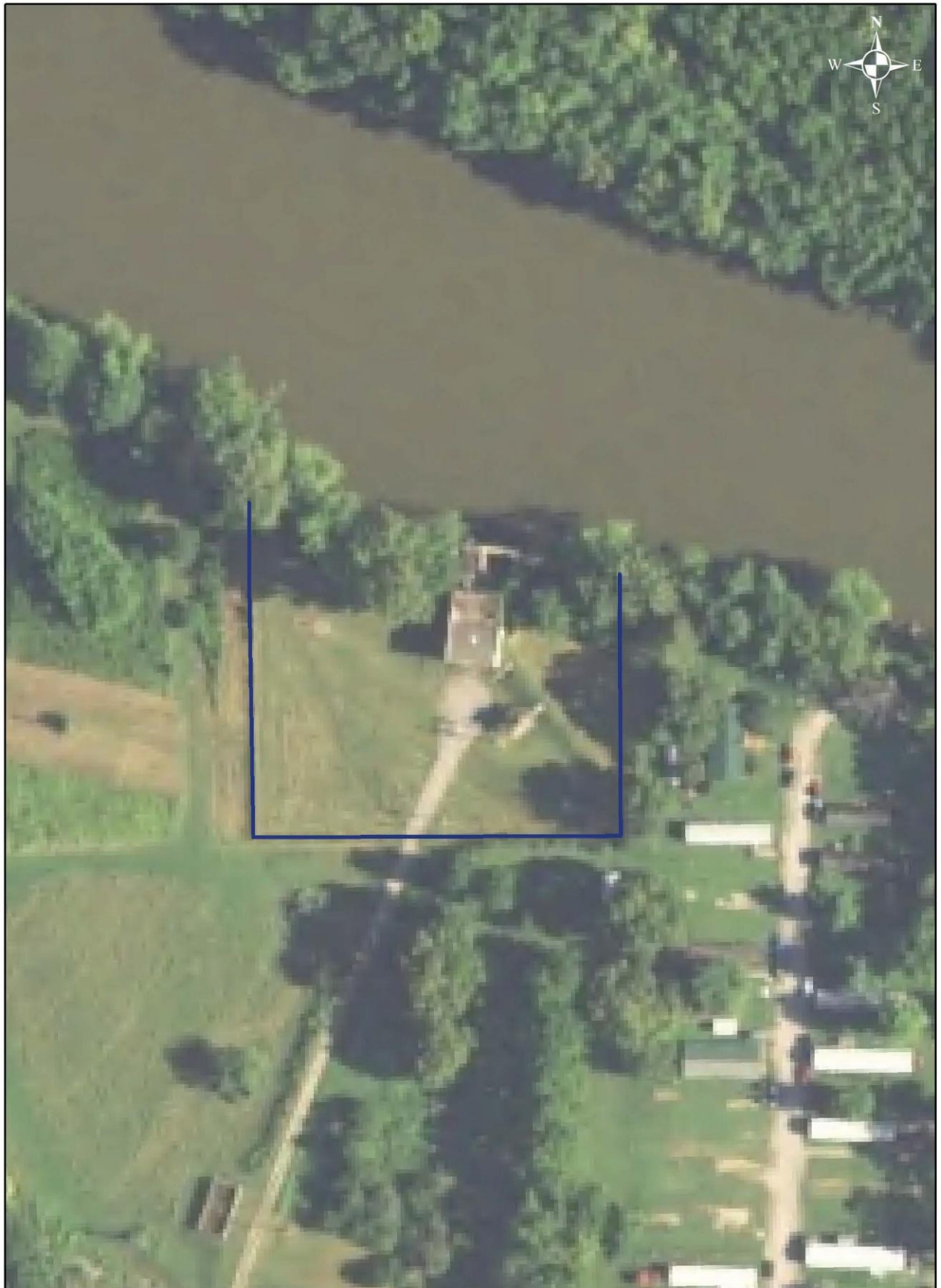
X-608 / Pump House
