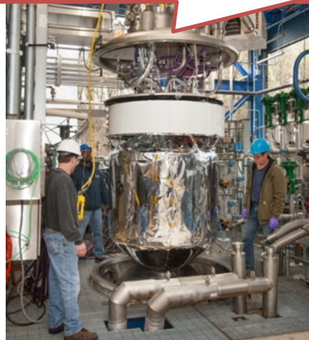
ZBO Test Article at the Small Multi-Purpose Research Facility (SMiRF) (GRC)
