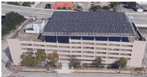
Figure1. Photovoltaic System at the Site
